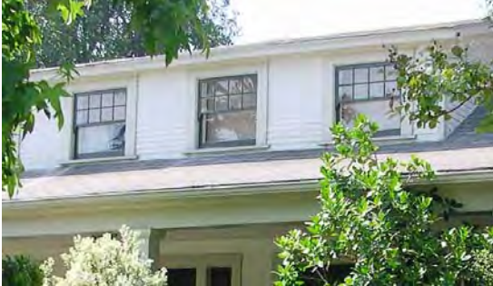
The historic windows on this home add to its character.
