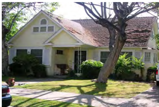
830 Melrose Hill, constructed in 1918.
