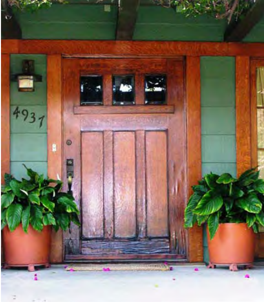
The loss of this door would have a negative effect on the character of this house.
