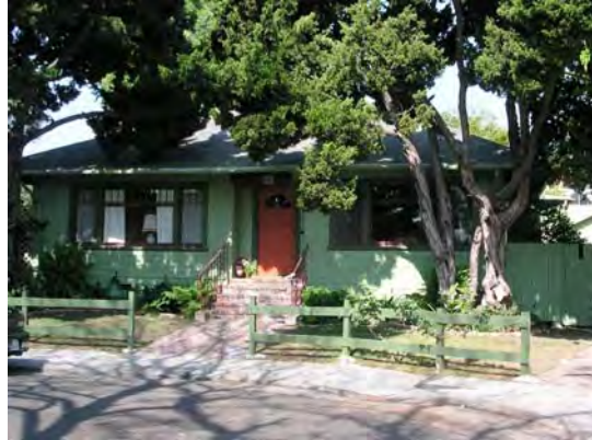
837 Melrose Hill, constructed in 1914.
