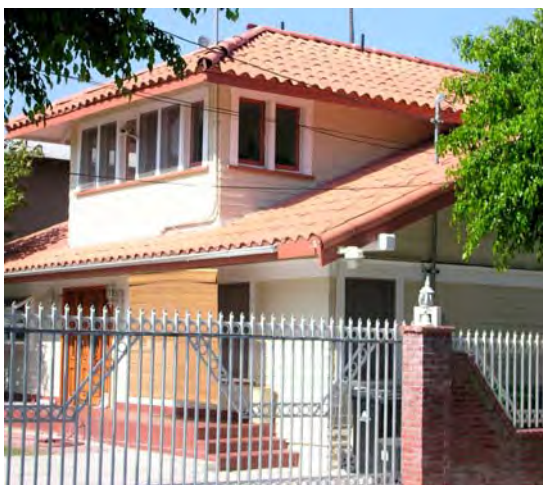
Inappropriate materials can also destroy the historic character of a structure. In this case, clay tiles should not be used on a Craftsman style home.
