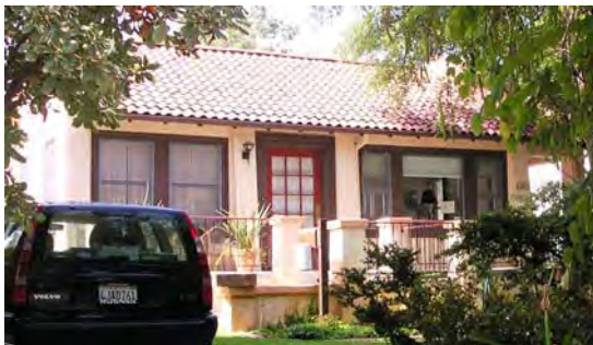
A clay tile roof is appropriate on a Mission Revival style home.
