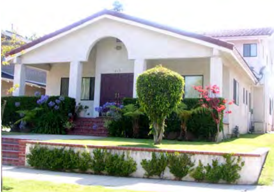
This front yard addition destroys the historic character of the main structure. Additions should always be placed at the rear of structures.
