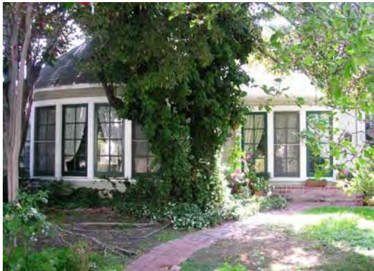
824 Melrose Hill, constructed in 1919.
