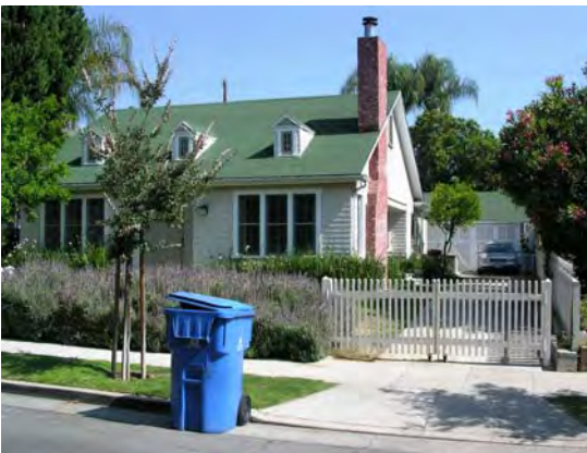
4947 Melrose Hill, constructed in 1918.
