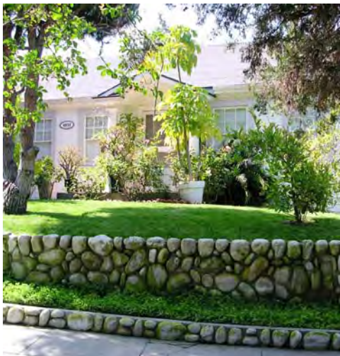
This historic retaining wall creates a consistent streetscape and neighborhood identity.
