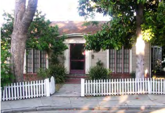
836 Melrose Hill, constructed in 1917.
