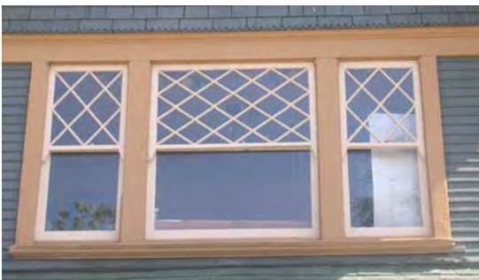
The decorative windows on this structure add to its historic character.
