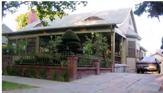
808 Melrose Hill, constructed in 1920.
