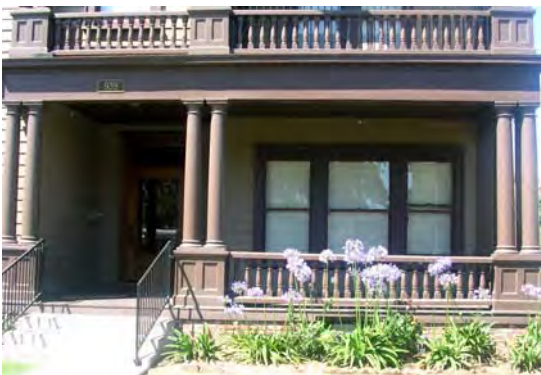
Adding a simple railing to improve safety is appropriate. However, the railing should match the existing porch in material and color.
