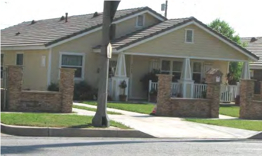
These infill homes use materials and paint colors that are similar to those used historically.
