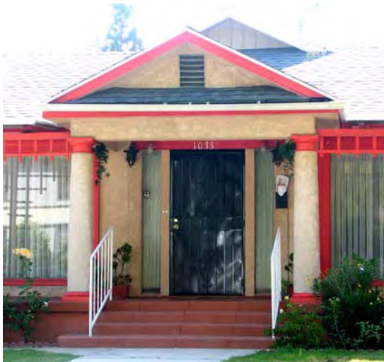
A security door disfigures this entryway.
