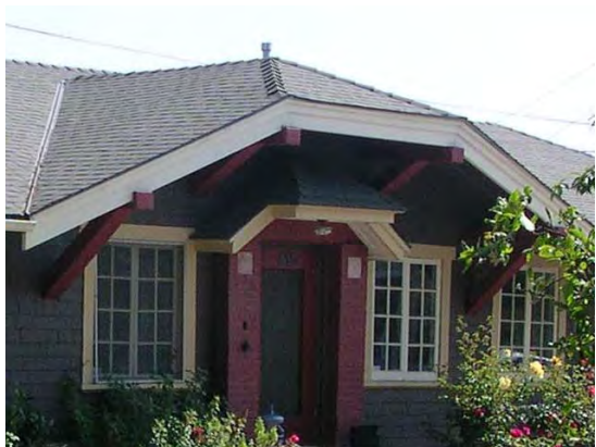
This complex roof system includes a medium pitched gable roof with the main ridge parallel to the front, a cross gable section that projects over the entrance and terminates with a jerkinhead, or clipped gable, and a cantilevered clipped gable roof over the entrance door.
