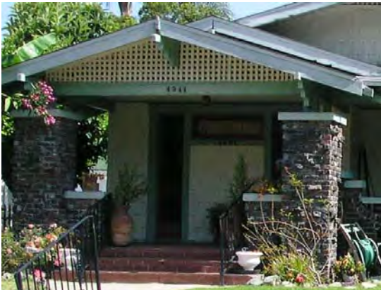
The clinker brick posts are common on Craftsman style bungalows. Painting them or altering them in another way would negatively affect the character of the home.
