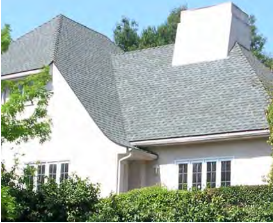
Stucco texture is based on stucco type and application. Historic stucco was always applied by hand, and never sprayed on. When replacing stucco, it is important to match the original texture and finish.
