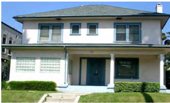
This porch has been filled in and inappropriate glass-block windows installed.
