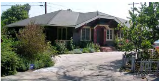
840 Melrose Hill, constructed in 1913.
