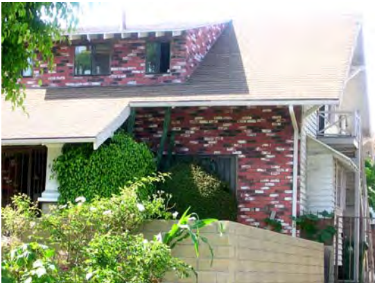
It is inappropriate to cover wood siding or other details with vinyl, stucco, or other materials. It is inappropriate to repair wood siding by adding new material that does not match the original.
