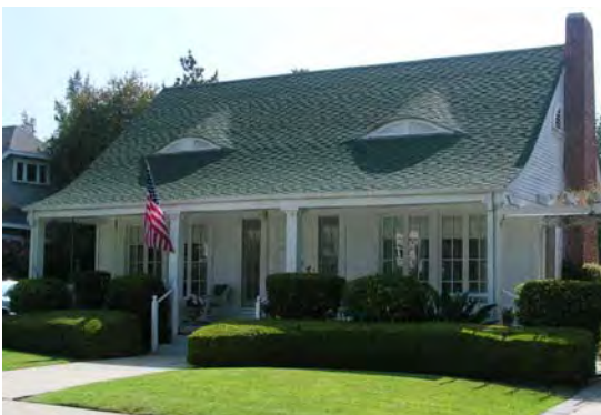
The porch is a significant element of this home. It is a full width porch covered by an extension of the main roof, four square wood columns and a central entrance door.
