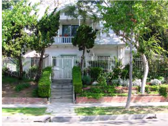
4935 Marathon Street, constructed in 1917. Ownership changed several times between 1920 and 1936 when August J. O'Conner became owner.
