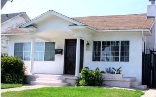
These replacement windows are inappropriate. When putting new windows on the front facade of a home, the new windows should match the historic windows in size, shape, arrangement of panes, materials, hardware, method of construction, and profile.
