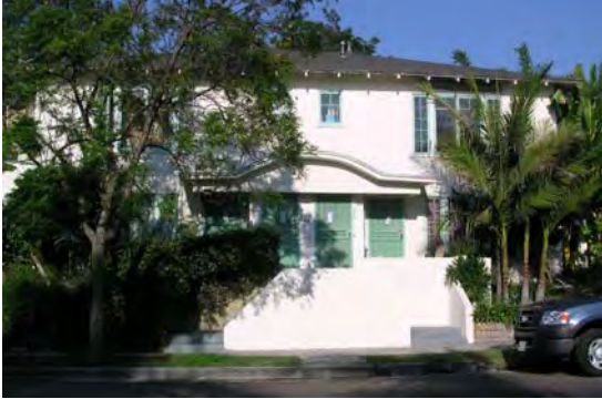
720-726 North Oxford Avenue, constructed in 1917 as a two-story, four family residence.
