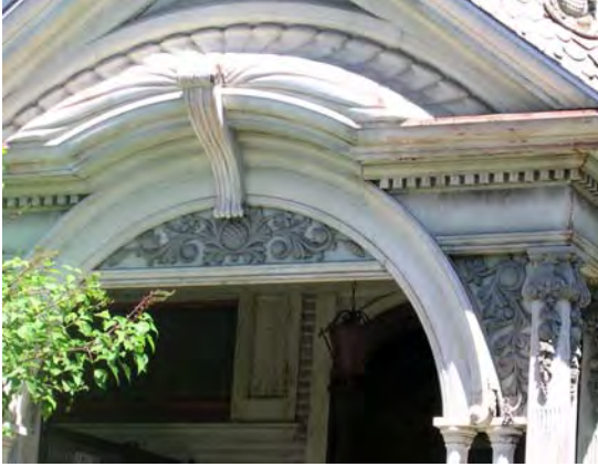
This porch is defined with decorative wood work.
