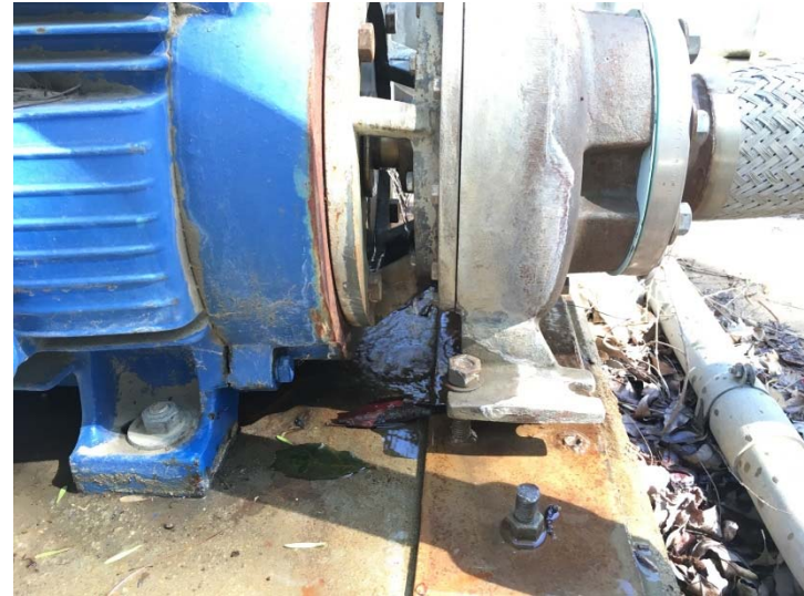
Photo 166: Potable Water Leak – Booster Pump Seal and Valve: April 19, 2016
