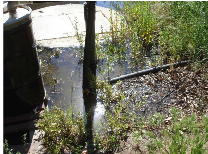
Photo 168: Portable Water Leak Ponding: April 19, 2016
