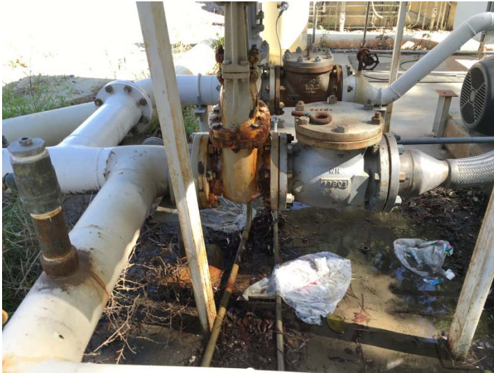
Photo 165: Potable Water Leak – Booster Pump Seal and Valve: April 19, 2016
