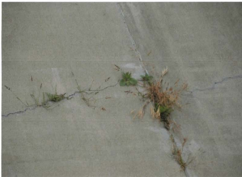
Photo 4a and 4b: Vegetation in cracks on wall of in Terminal Basin
