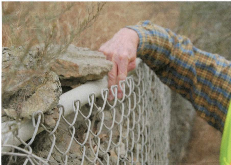
Photo 5a and 5b: Soil against fence a retaining wall along San Fernando Road
