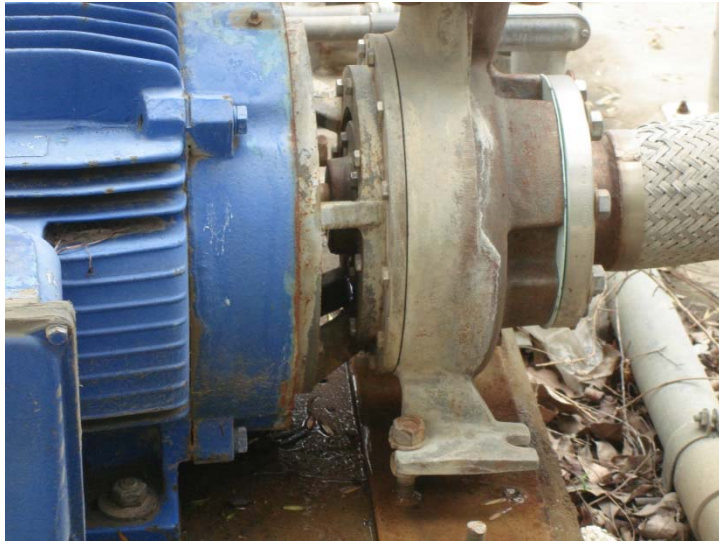
Photo 169: Potable Water Booster Pump Seal Leak: May 10, 2016
