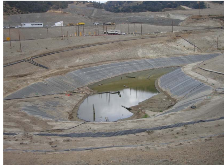
Photo 62: City Lined Drainage Lift Area: May 25, 2016
