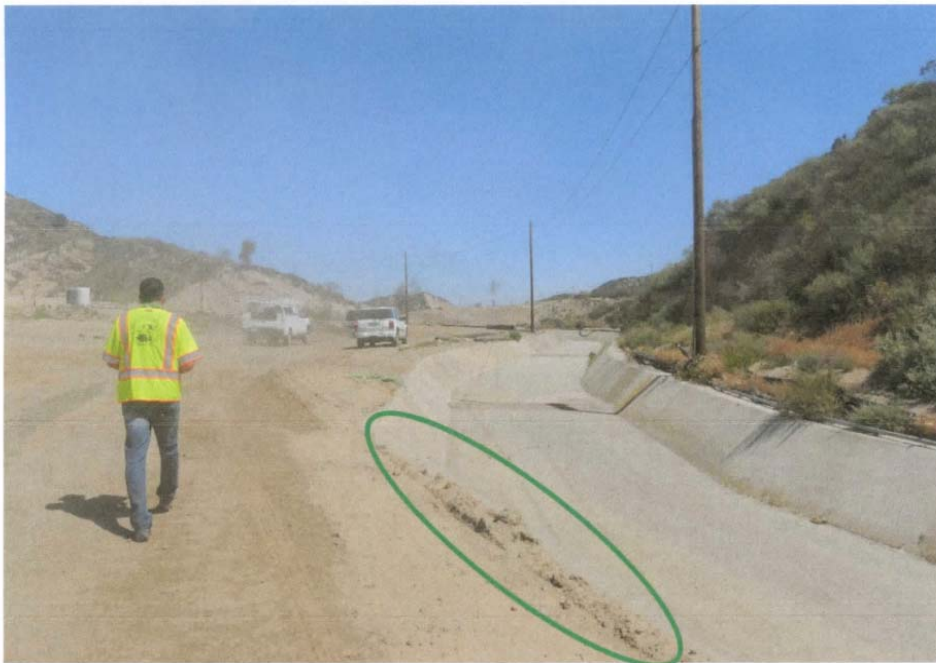
Figure 4: Separation between edge of concrete channel and soil has been backfilled
