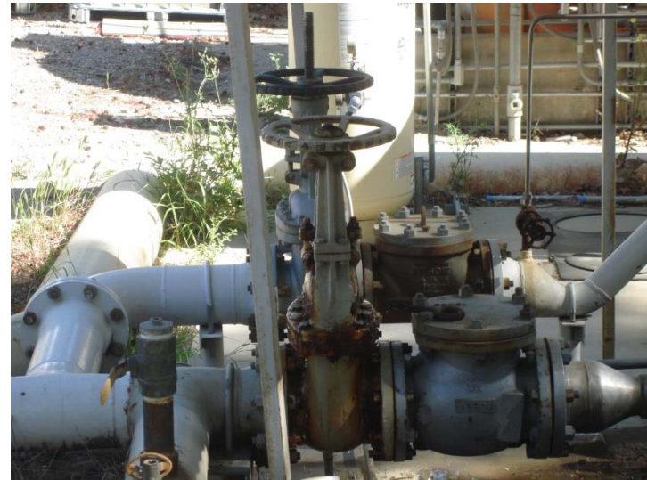
Photo 164: Potable Water Leak – Booster Pump Seal and Valve: April 19, 2016
