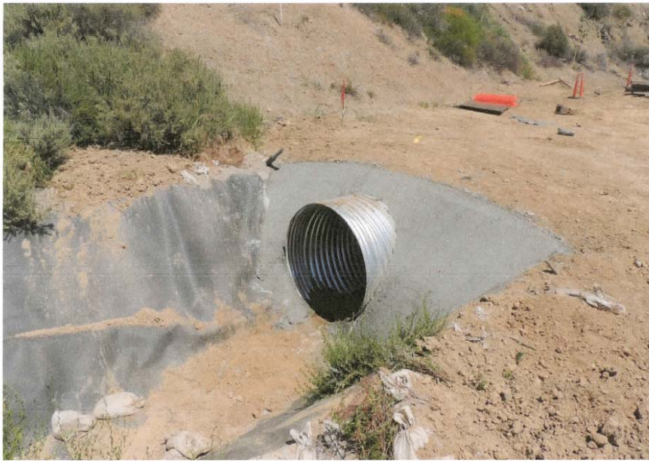
Photo 3: Connection geomembrane-shotcrete at drainage pipe intake
