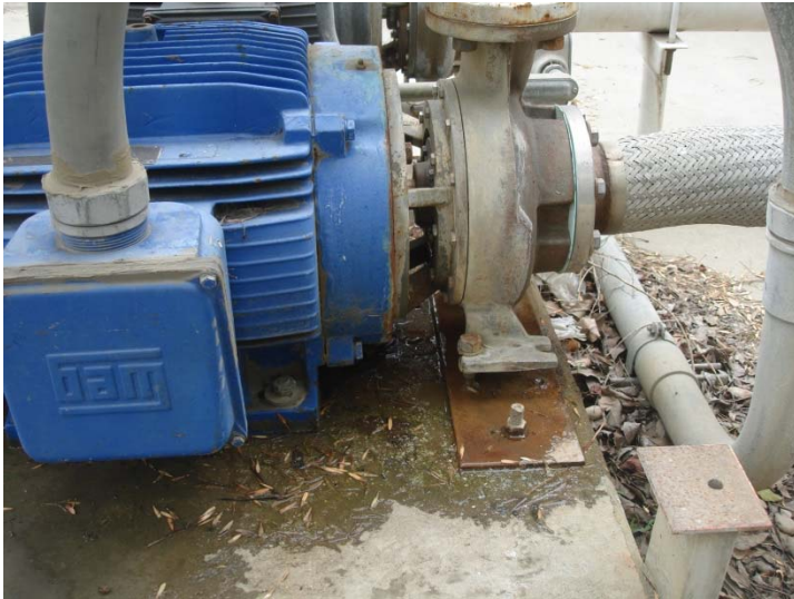
Photo 173: Potable Water Booster Pump Seal Leak: May 25, 2016
