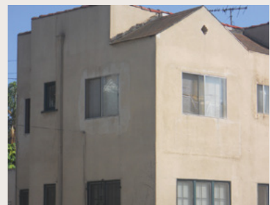
Windows and doors should not be mounted flush with the exterior wall finish as shown here, they must be setback or have a frame detail that provides some relief and shadow.
