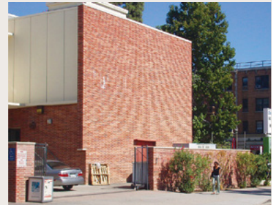
A tall masonry wall matching the color and finish of the main building screens most of a ground mounted electrical cabinet that would otherwise be visible from the public right-of-way.
