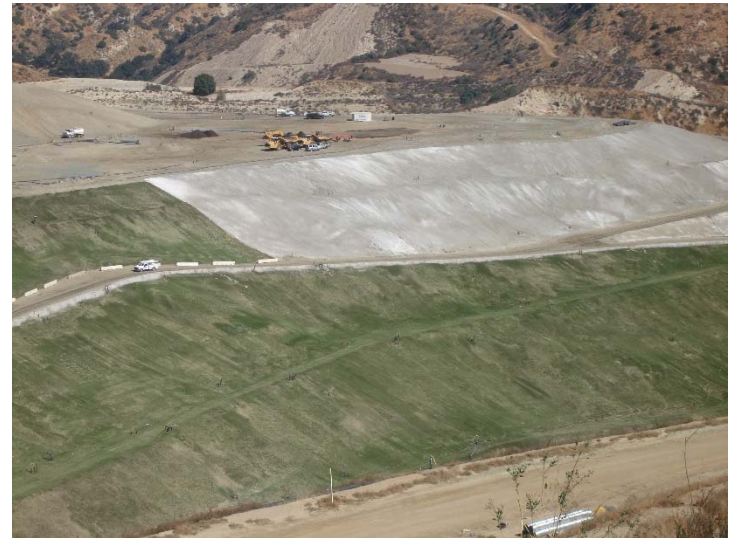
Photo 200: Closure Turf & Posi-Shell: October 26, 2017
