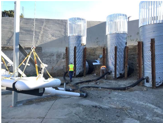
Photo 515: Terminal Basin New Skimmer Risers Outlet System: December 12, 2017
