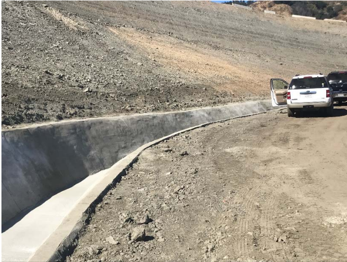
Photo 333: New Concrete Westside Drainage Channel: October 26, 2017
