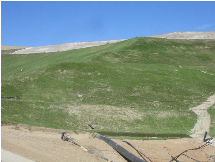
Photo 231: Closure Turf & Posi-Shell: December 12, 2017
