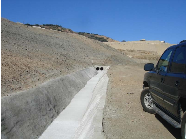
Photo 339: New Concrete Westside Drainage Channel: October 26, 2017
