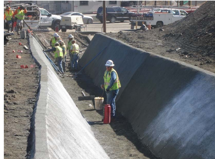
Photo 330: New Concrete Westside Drainage Channel: October 26, 2017
