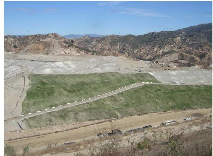
Photo 204: Closure Turf & Posi-Shell: November 7, 2017
