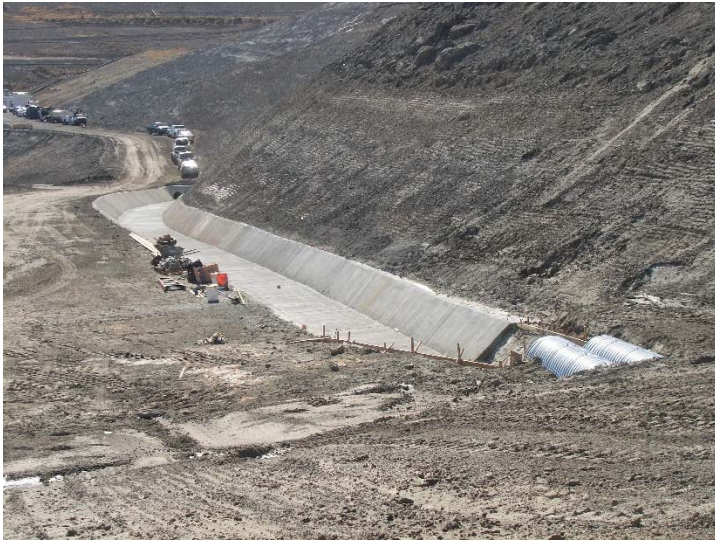
Photo 341: New Concrete Westside Drainage Channel: October 26, 2017
