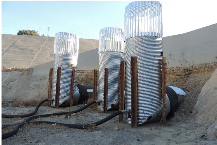
Photo 513: Terminal Basin New Skimmer Risers Outlet System: December 12, 2017
