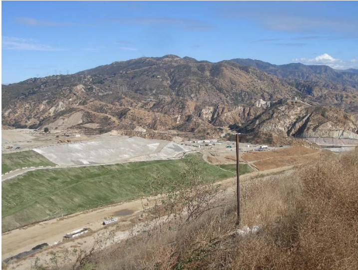
Photo 205: Closure Turf & Posi-Shell: November 7, 2017
