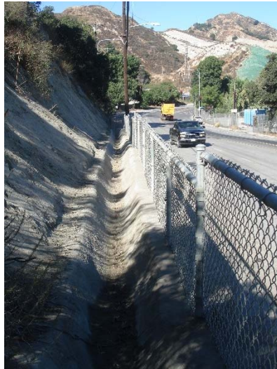
Photo 565: Frontage Retaining Wall on San Fernando Road Plugged Drainage: November 7, 2017
