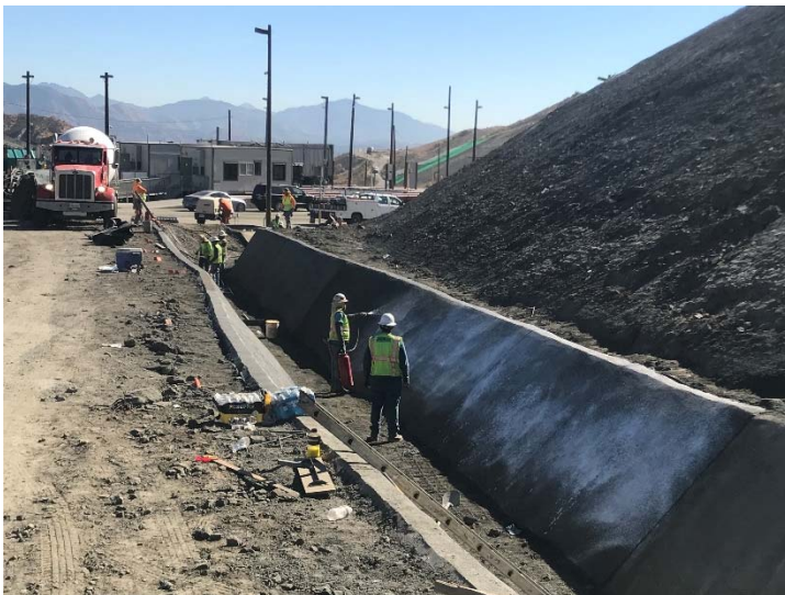
Photo 331: New Concrete Westside Drainage Channel: October 26, 2017
