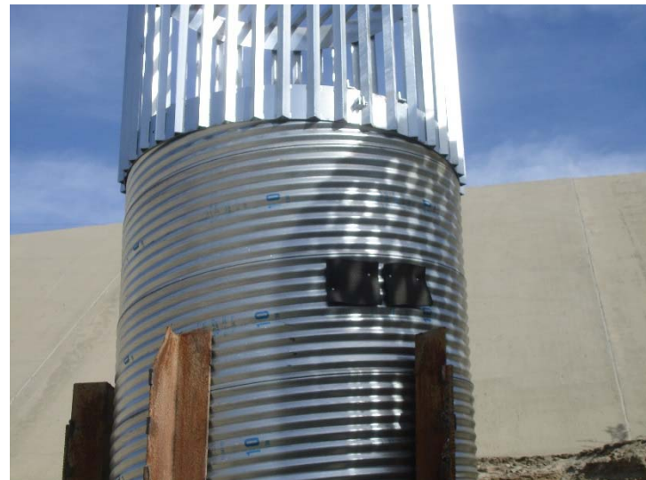
Photo 500: Terminal Basin New Skimmer Risers Low Flow Outlet: November 21, 2017
