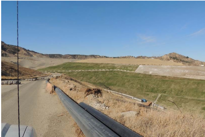
Photo 225: Closure Turf & Posi-Shell: December 12, 2017
