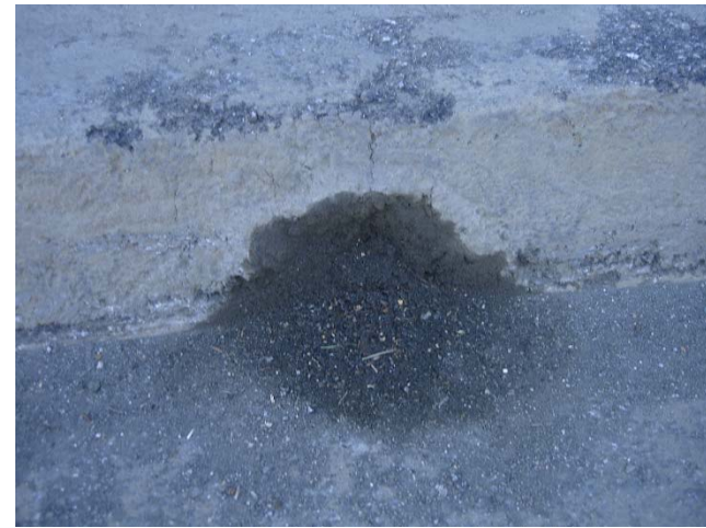
Photo 572: Frontage Retaining Wall on San Fernando Road Plugged Drainage: November 7, 2017
