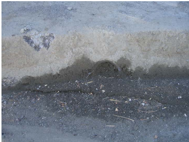
Photo 571: Frontage Retaining Wall on San Fernando Road Plugged Drainage: November 7, 2017
