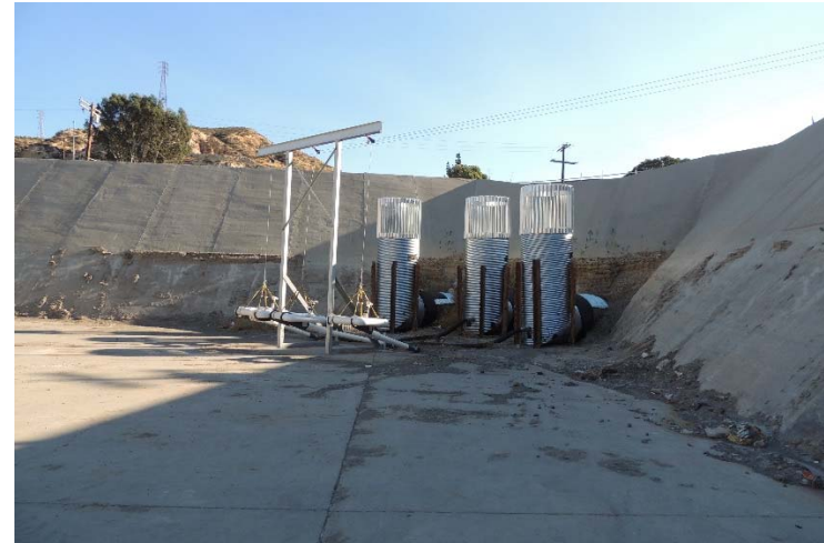
Photo 514: Terminal Basin New Skimmer Risers Outlet System: December 12, 2017
