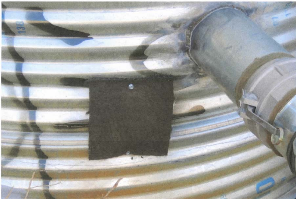
Photo 10: Drain Holes with Geocomposite Patch on Riser at Terminal Basin
