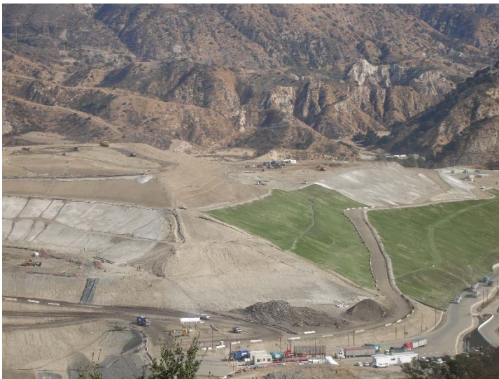
Photo 215: Closure Turf & Posi-Shell: November 21, 2017
