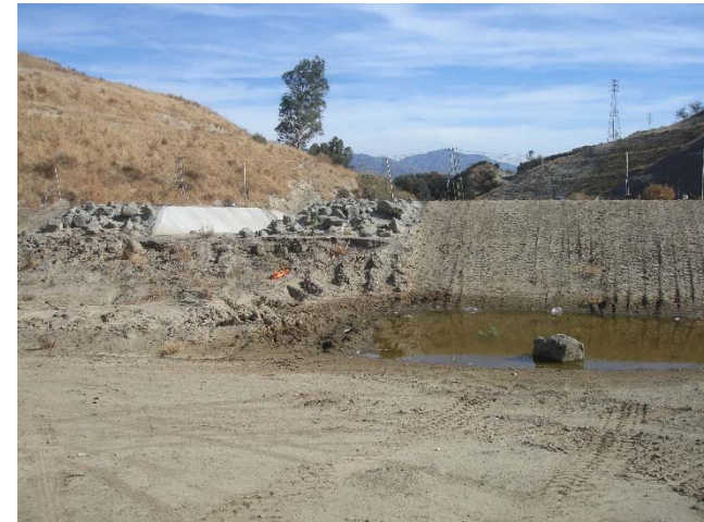
Photo 264: Basin CC3B Plugged Low Flow-Outlet: November 21, 2017
