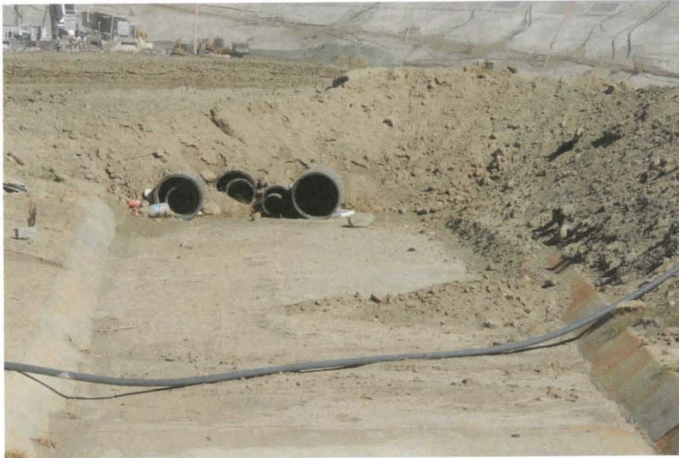
Photo 9: Partially obstructed channel downstream of basin A
