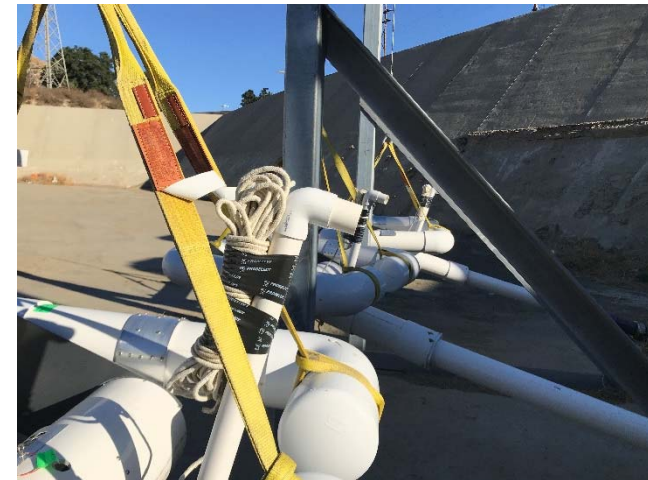
Photo 516: Terminal Basin New Skimmer Risers Outlet System: December 12, 2017
