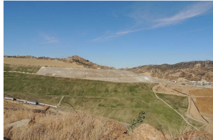
Photo 226: Closure Turf & Posi-Shell: December 12, 2017
