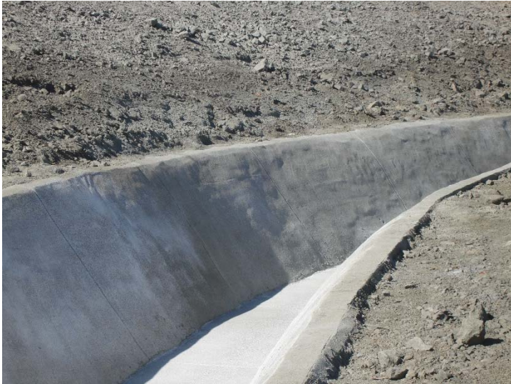
Photo 337: New Concrete Westside Drainage Channel: October 26, 2017
