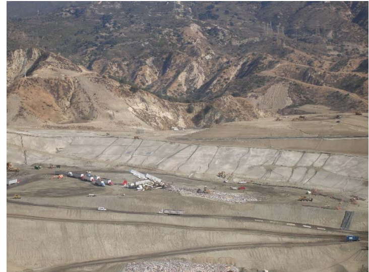
Photo 214: Closure Turf & Posi-Shell: November 21, 2017
