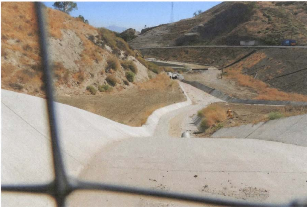
Photo 4: Spillway and blocked pipe on apron at temporary earthen basin near terminal basin
