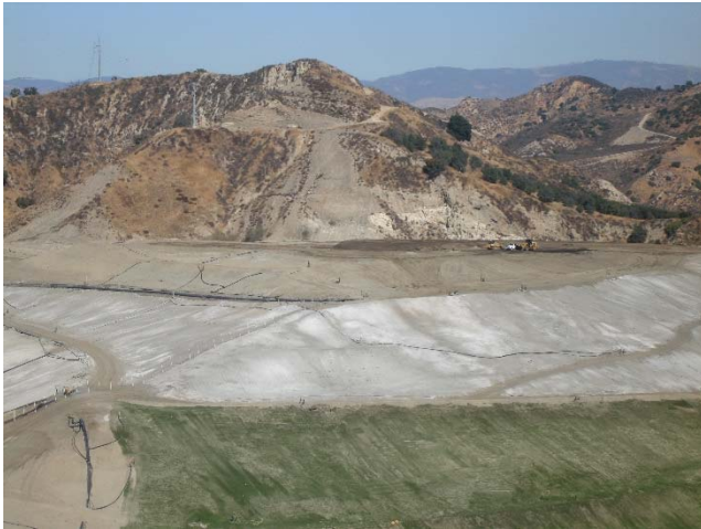
Photo 193: Closure Turf & Posi-Shell: October 26, 2017
