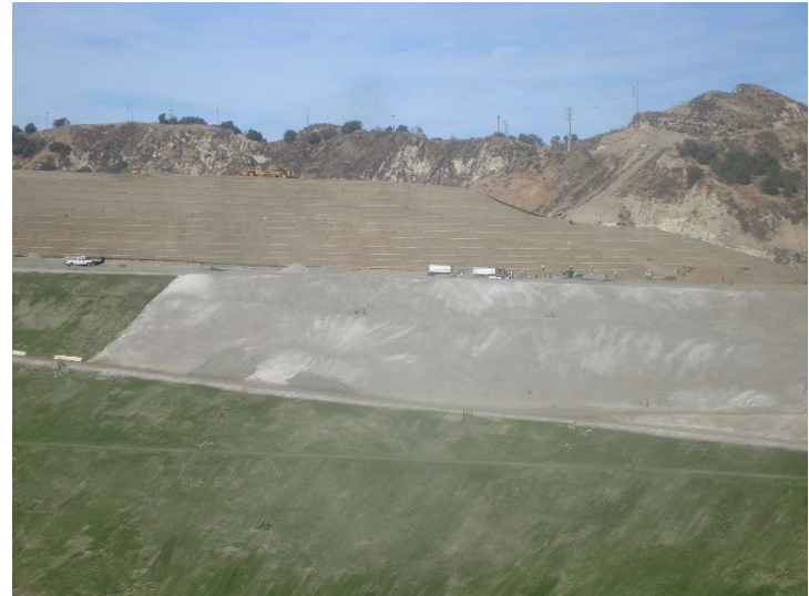
Photo 218: Closure Turf & Posi-Shell: November 21, 2017
