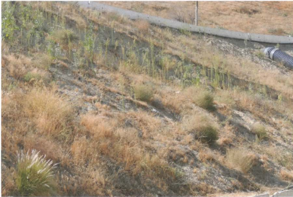
Photo 15: Sloughing on embankment of main access road near entrance of Terminal Basin
