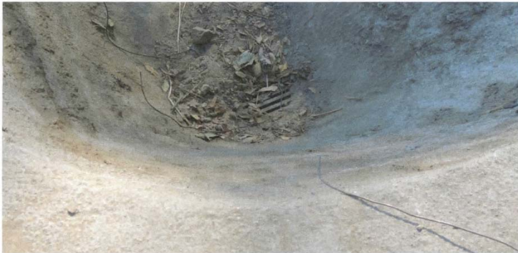
Photo 19: Cleaning operations at wall on San Fernando Road – Cleared drain intake at swale
