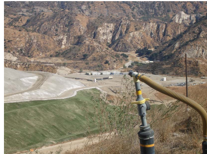
Photo 196: Closure Turf & Posi-Shell: October 26, 2017
