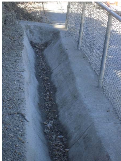
Photo 567: Frontage Retaining Wall on San Fernando Road Plugged Drainage: November 7, 2017
