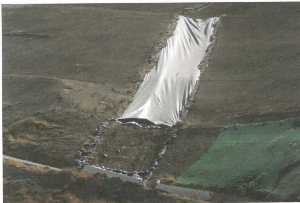
Photo 12: Geomembrane Slip-side Needing Repair on Old City Landfill Slope
