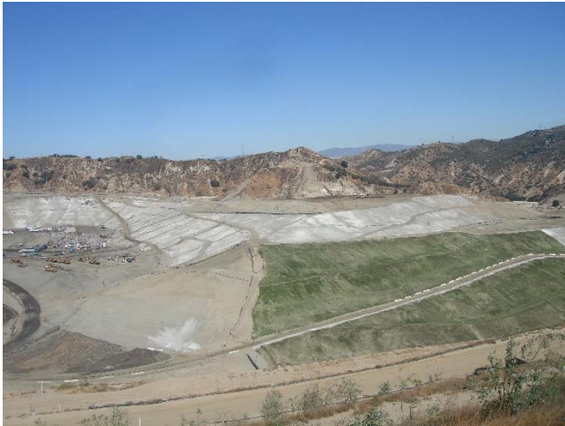
Photo 189: Closure Turf & Posi-Shell: October 26, 2017
