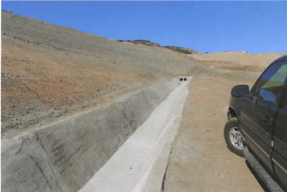
Photo 13: New V-ditch along access road bordering cell CC4 Phase 2
