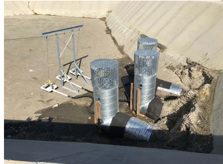
Photo 490: Terminal Basin New Skimmer Risers: November 7, 2017
