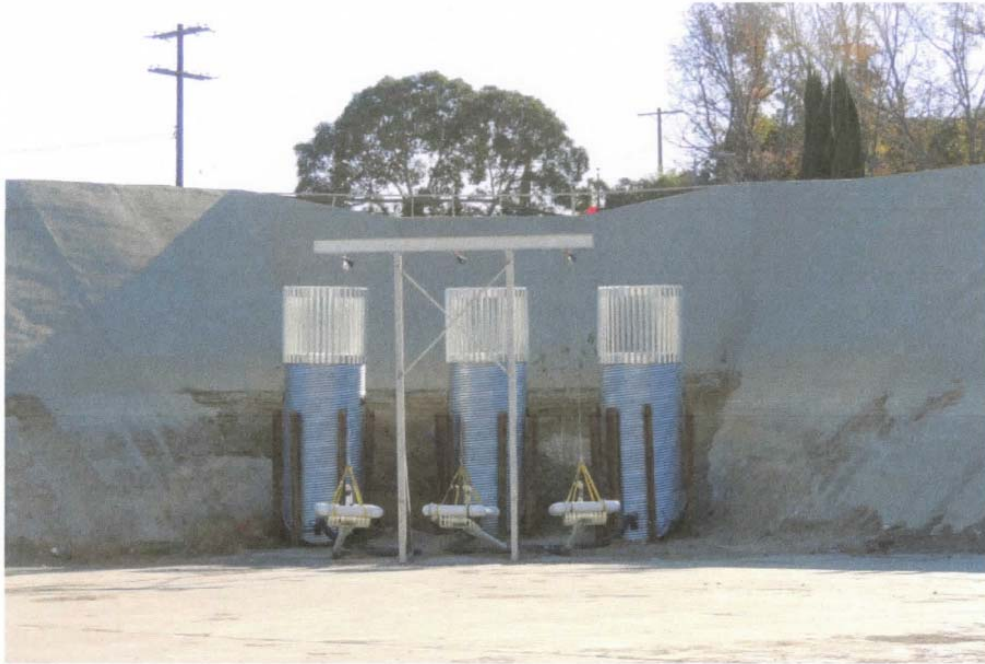
Photo 9: Skimmers in Terminal Basin
