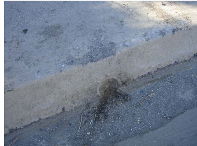
Photo 570: Frontage Retaining Wall on San Fernando Road Plugged Drainage: November 7, 2017
