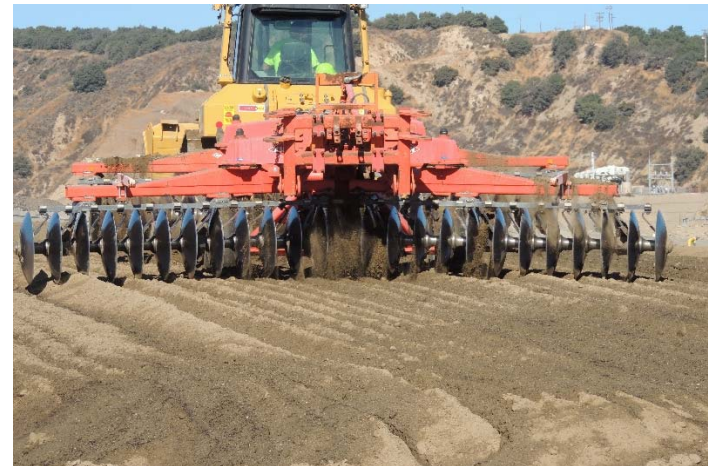
Photo 184: CC3A Top Deck Soil Amending: October 26, 2017
