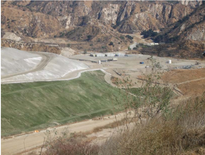
Photo 201: Closure Turf & Posi-Shell: October 26, 2017
