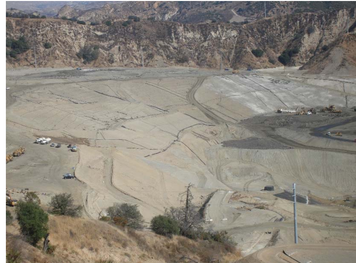
Photo 210: Closure Turf & Posi-Shell: November 21, 2017
