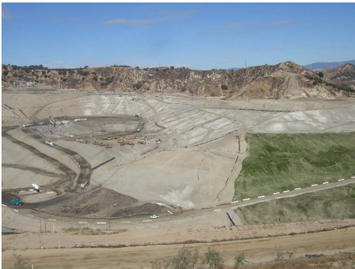
Photo 203: Closure Turf & Posi-Shell: November 7, 2017
