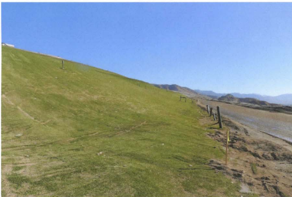
Photo 16: Repaired breakout on Closure Turf along access road to deck of Cell CC3b
