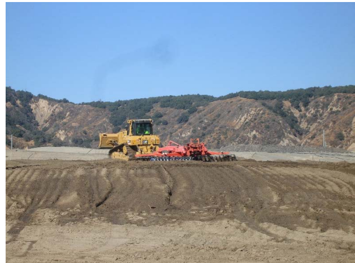
Photo 180: CC3A Top Deck Soil Amending: October 26, 2017
