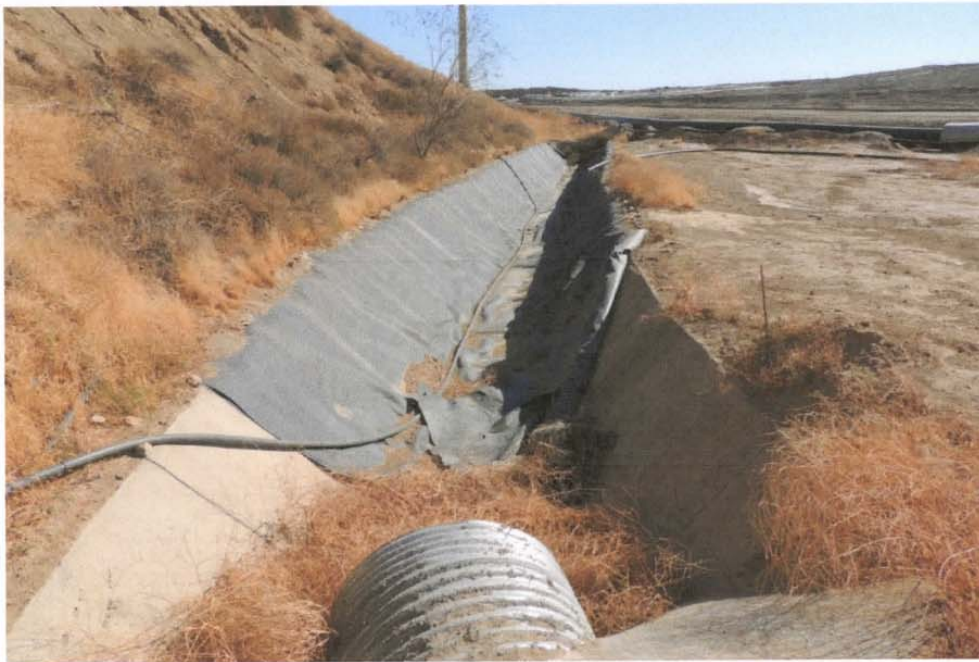
Photo 8: Torn-up Geomembrane, Tumbleweeds, and Soil in Channel between Basin B and D
