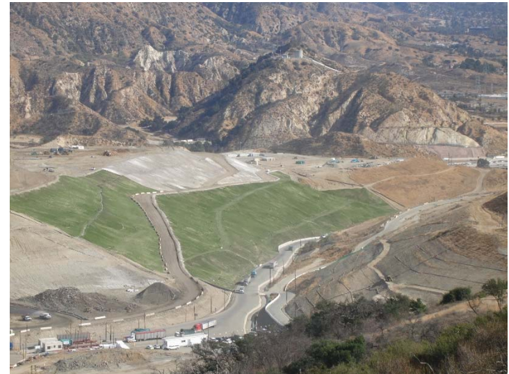
Photo 216: Closure Turf & Posi-Shell: November 21, 2017
