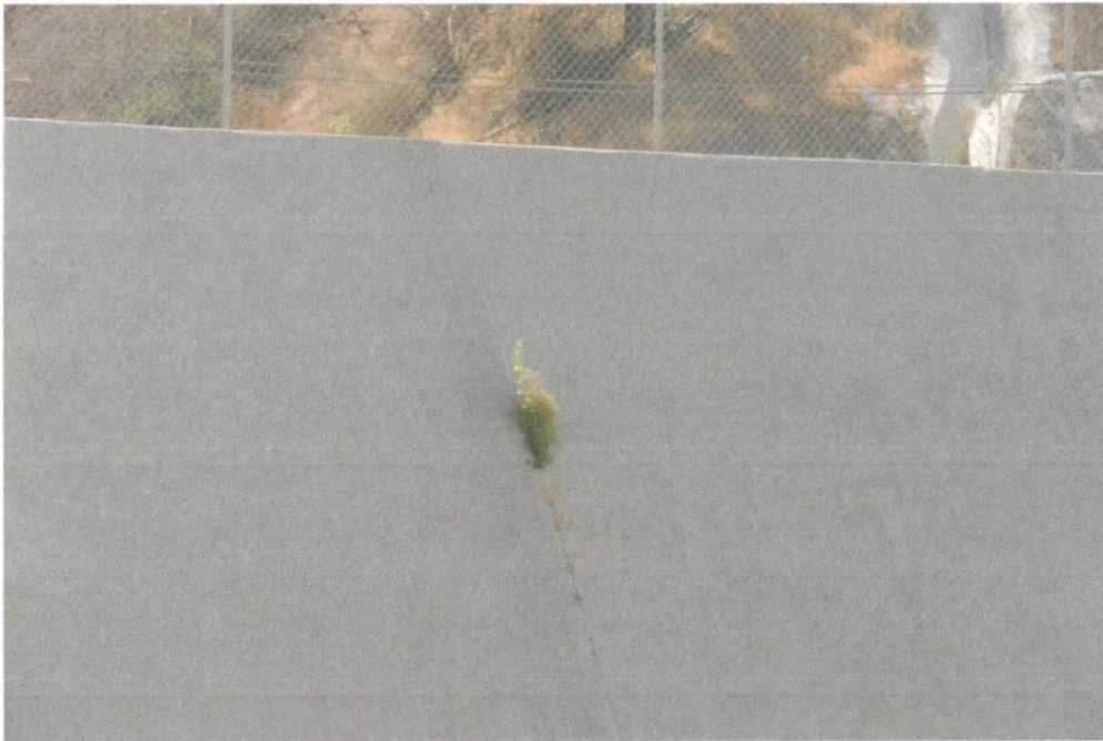
Photo 11: Weeds in crack on shotcrete wall of Terminal Basin
