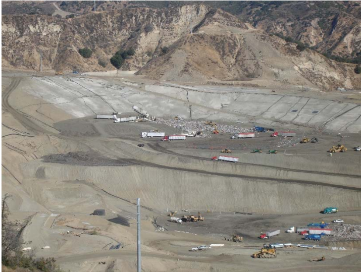
Photo 221: Closure Turf & Posi-Shell: December 12, 2017
