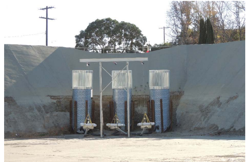
Photo 510: Terminal Basin New Skimmer Risers Outlet System: December 12, 2017
