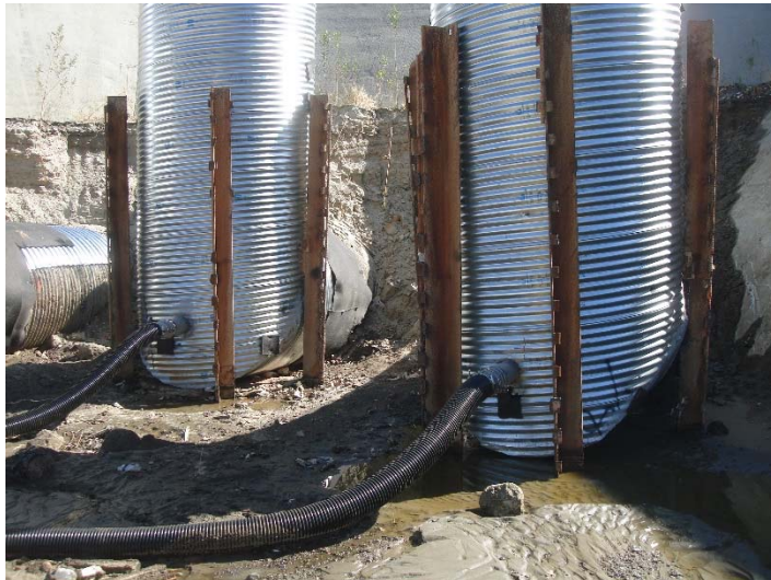
Photo 495: Terminal Basin New Skimmer Risers: November 7, 2017
