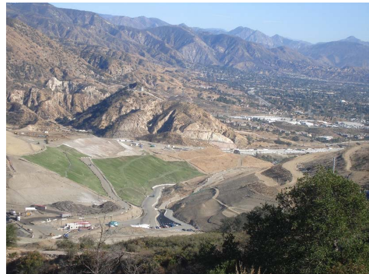
Photo 224: Closure Turf & Posi-Shell: December 12, 2017
