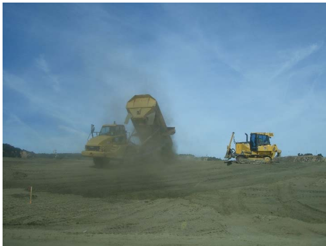
Photo 187: CC3A Top Deck Soil Amending: November 21, 2017
