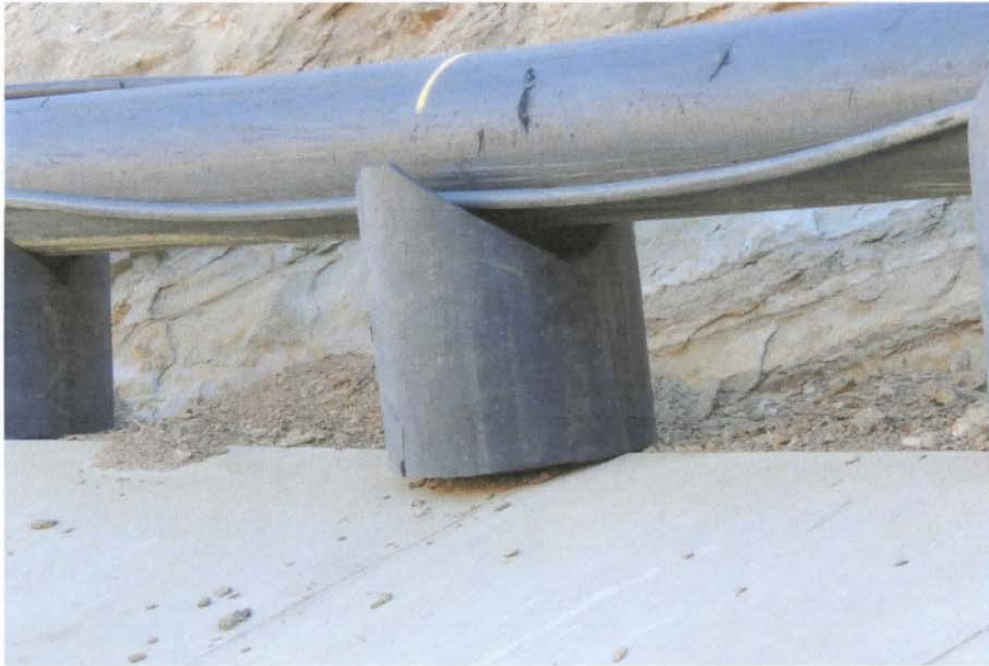
Photo 5: Potentially Unstable HDPE Supports for Gas Header at Basin A
