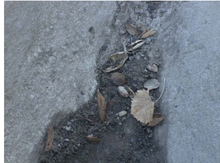
Photo 566: Frontage Retaining Wall on San Fernando Road Plugged Drainage: November 7, 2017
