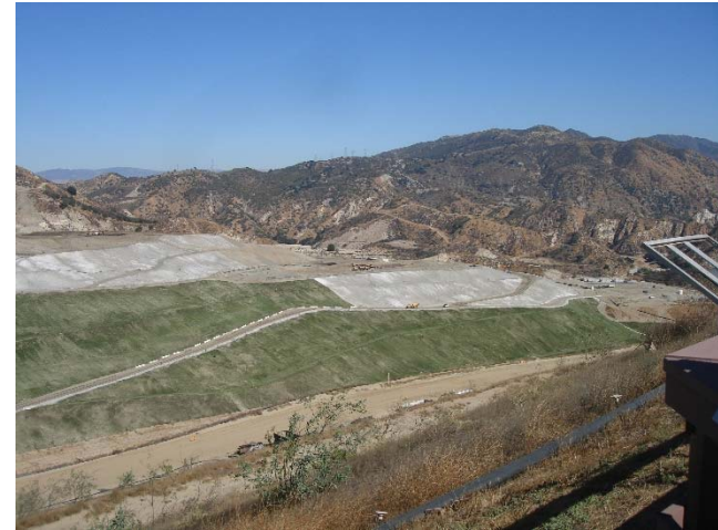
Photo 190: Closure Turf & Posi-Shell: October 26, 2017
