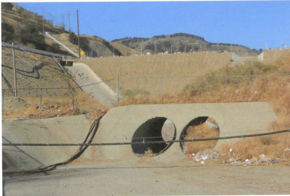
Photo 11: Culvert into Terminal Basin plugged with Tumbleweed
