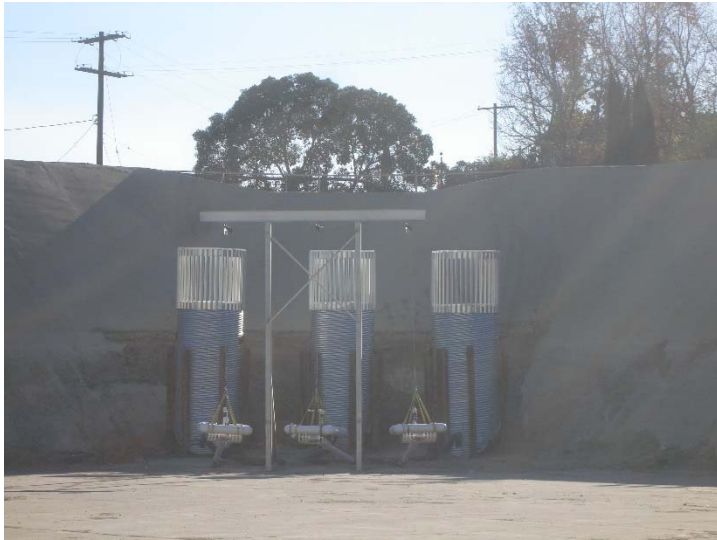
Photo 509: Terminal Basin New Skimmer Risers Outlet System: December 12, 2017
