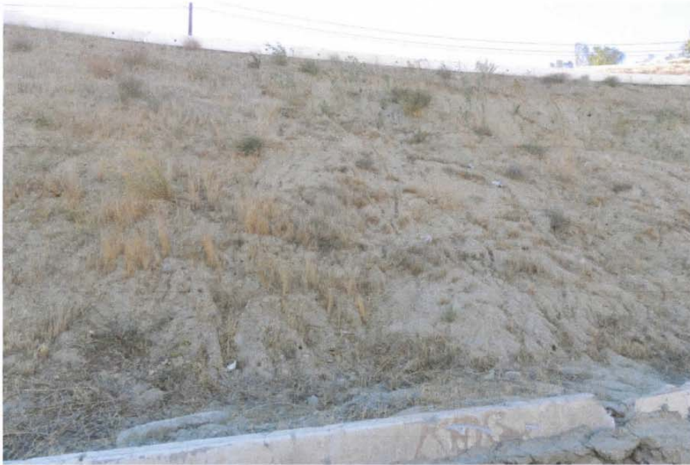
Photo 13: Sloughing on embankment of main access road near entrance of Terminal Basin
