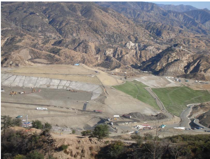
Photo 223: Closure Turf & Posi-Shell & Top Deck Revegetation: December 12, 2017
