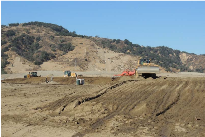
Photo 183: CC3A Top Deck Soil Amending: October 26, 2017
