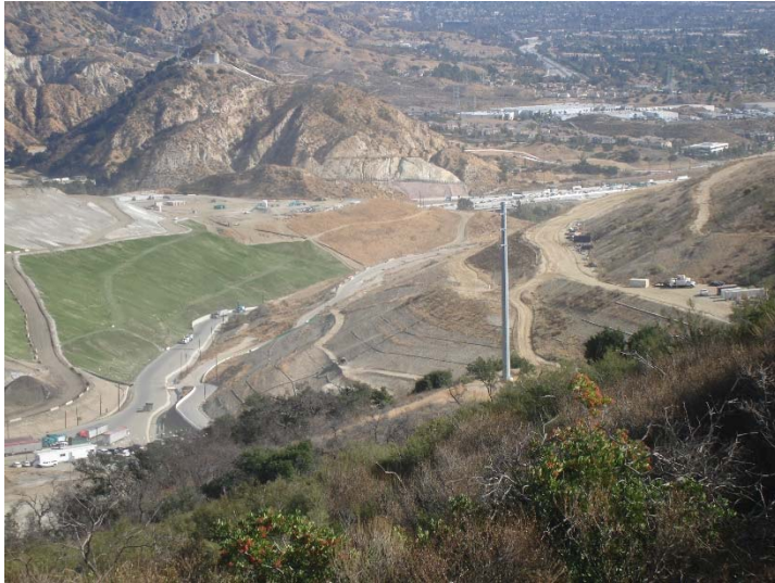
Photo 213: Closure Turf & Posi-Shell: November 21, 2017
