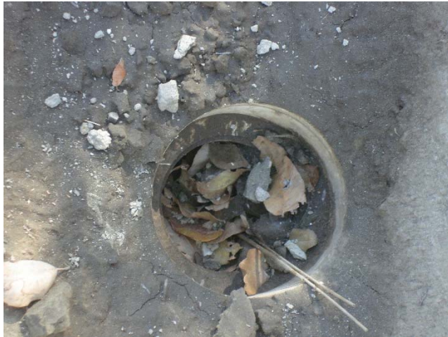
Photo 569: Frontage Retaining Wall on San Fernando Road Plugged Drainage: November 7, 2017
