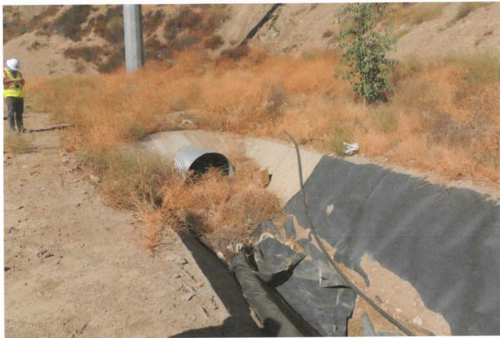
Photo 10: Torn-up geomembrane, tumbleweeds, and soil in Channel between Basin B and D
