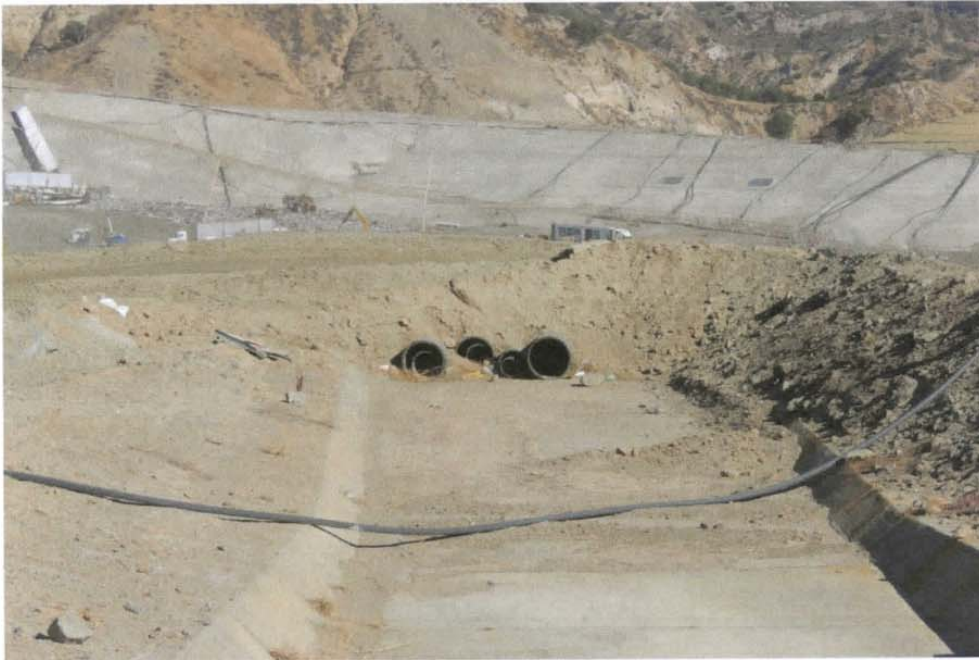
Photo 7: Partially Obstructed Channel Downstream of Basin A
