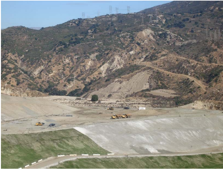
Photo 209: Closure Turf & Posi-Shell: November 7, 2017
