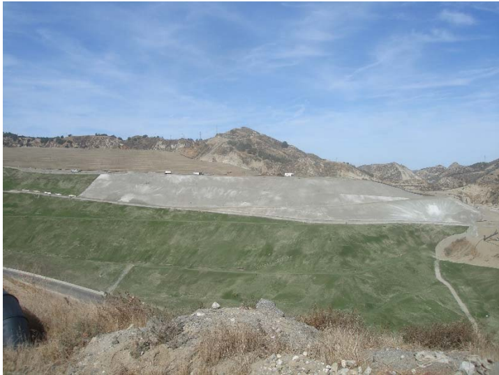
Photo 217: Closure Turf & Posi-Shell: November 21, 2017
