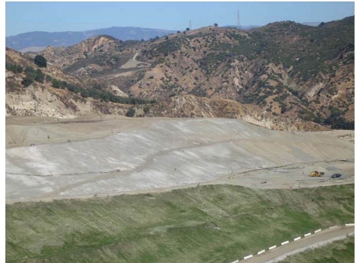
Photo 208: Closure Turf & Posi-Shell: November 7, 2017
