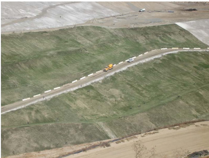
Photo 199: Closure Turf & Posi-Shell: October 26, 2017
