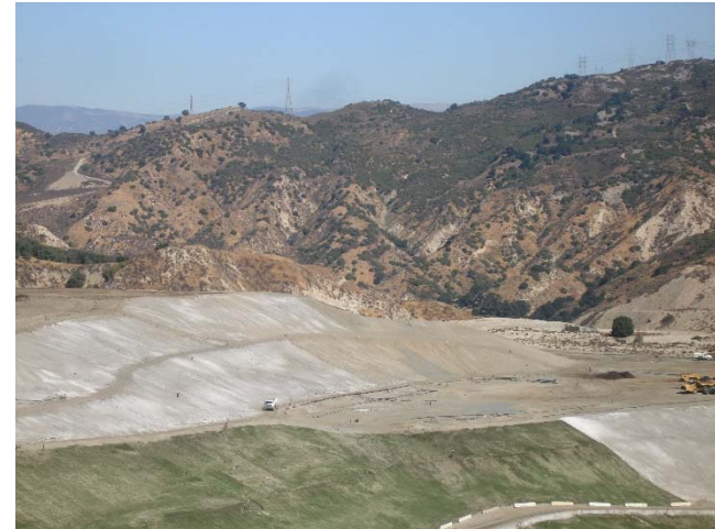
Photo 194: Closure Turf & Posi-Shell: October 26, 2017
