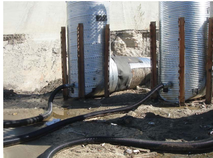
Photo 494: Terminal Basin New Skimmer Risers: November 7, 2017
