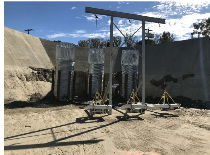
Photo 488: Terminal Basin New Skimmer Risers: November 7, 2017
