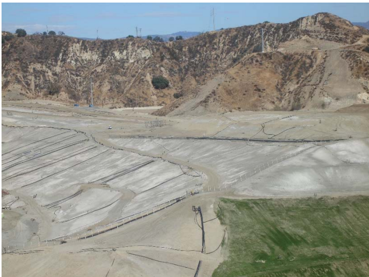
Photo 207: Closure Turf & Posi-Shell: November 7, 2017
