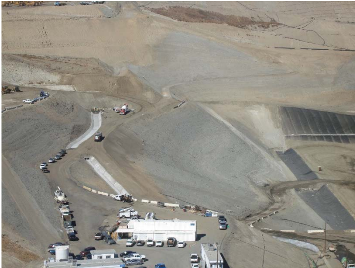
Photo 329: New Concrete Westside Drainage Channel: October 26, 2017
