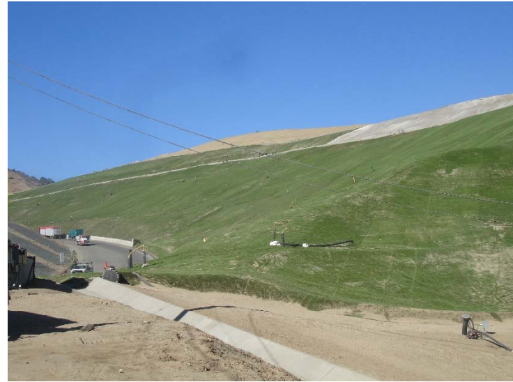
Photo 230: Closure Turf & Posi-Shell: December 12, 2017
