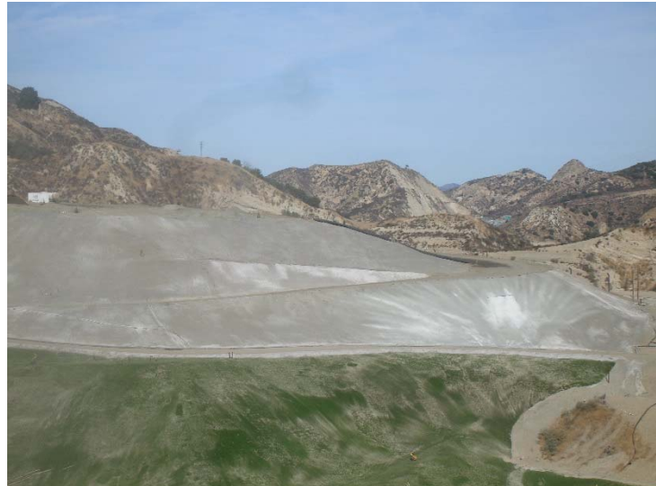
Photo 220: Closure Turf & Posi-Shell: November 21, 2017
