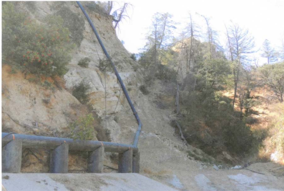
Photo 7: HDPE supports for gas header at Basin A
