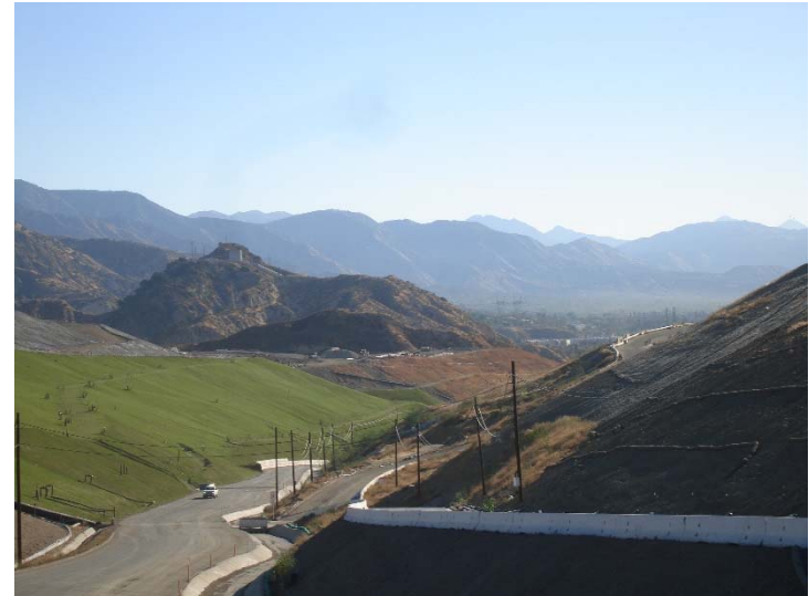
Photo 202: Closure Turf & Posi-Shell: October 26, 2017
