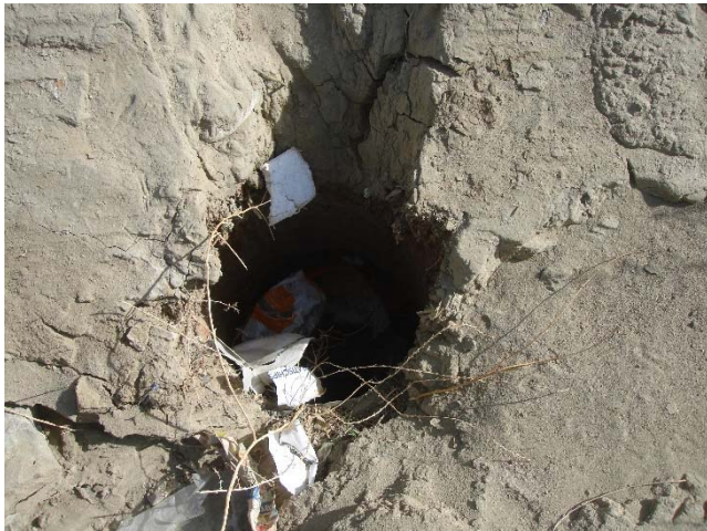
Photo 263: Basin CC3B Plugged Low Flow-Outlet: November 21, 2017
