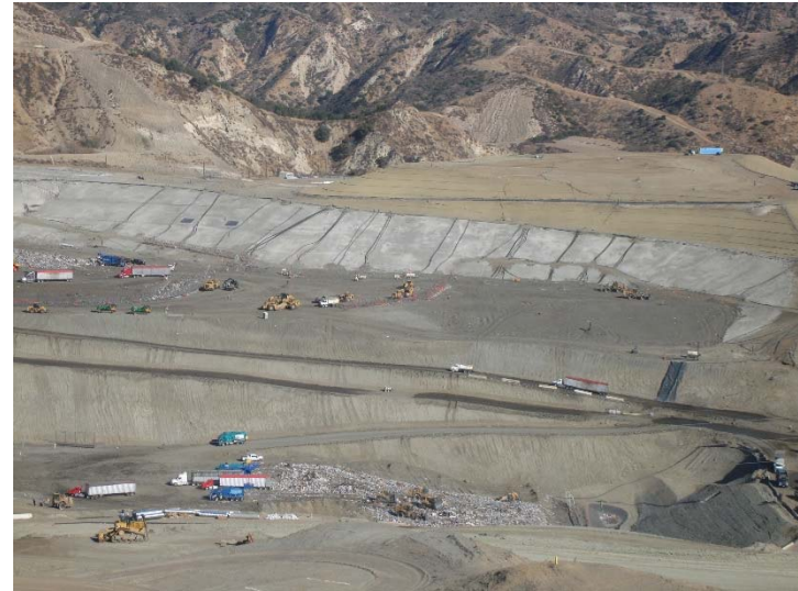
Photo 222: Closure Turf & Posi-Shell & Top Deck Revegetation: December 12, 2017
