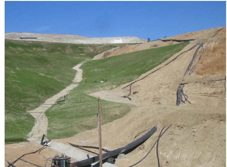
Photo 232: Closure Turf & Posi-Shell: December 12, 2017
