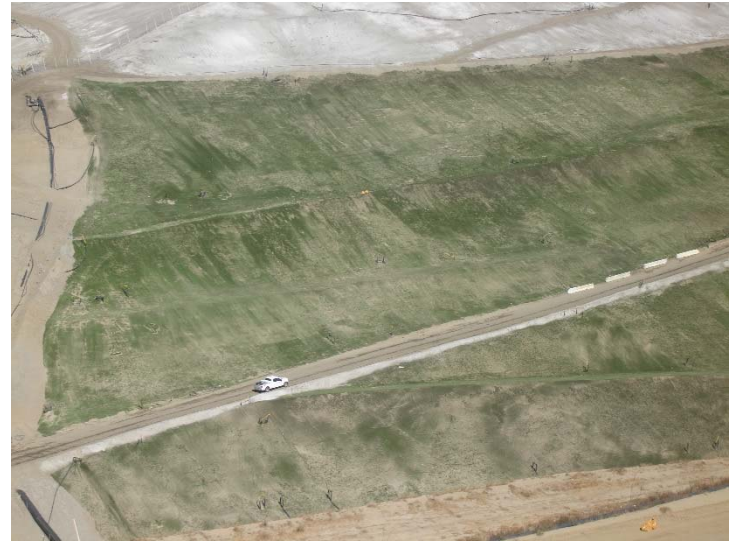
Photo 198: Closure Turf & Posi-Shell: October 26, 2017
