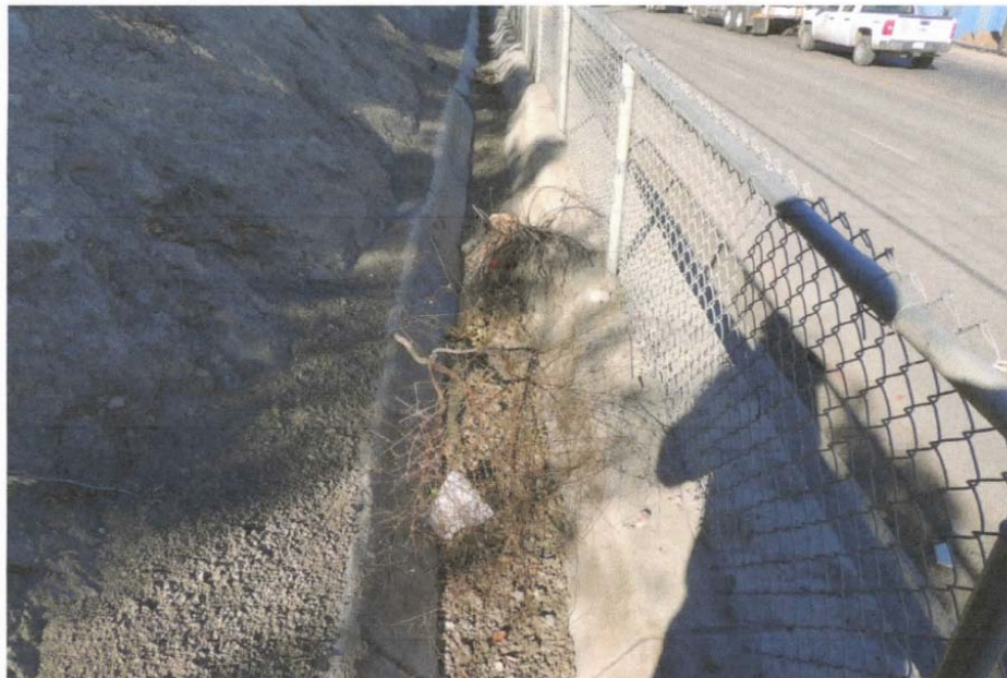
Photo 16: Soil Accumulating in Drainage Ditch on Top of San Fernando Wall
