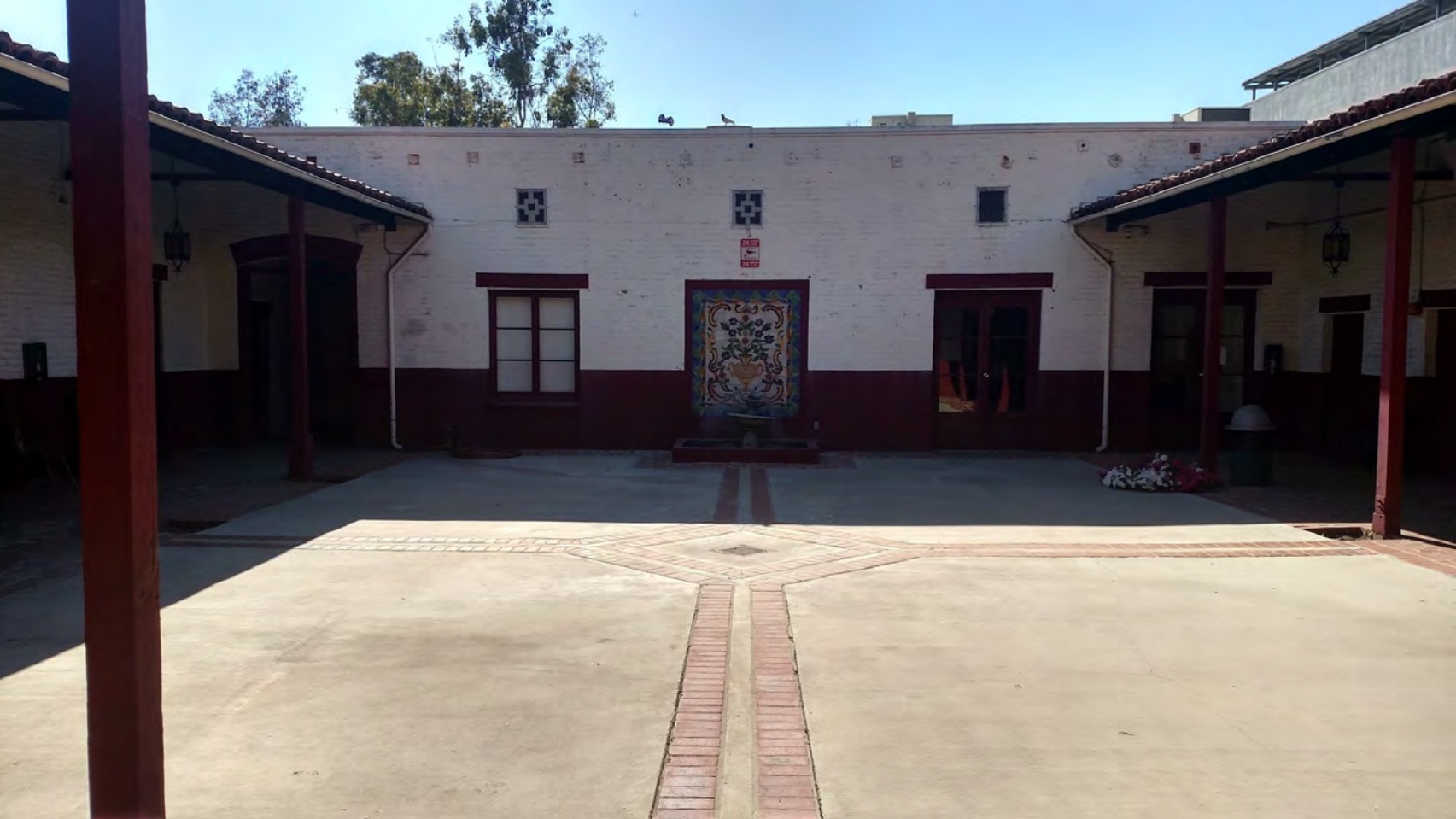
Main courtyard, view west. Photo by: Andrea Griego, 2019.
