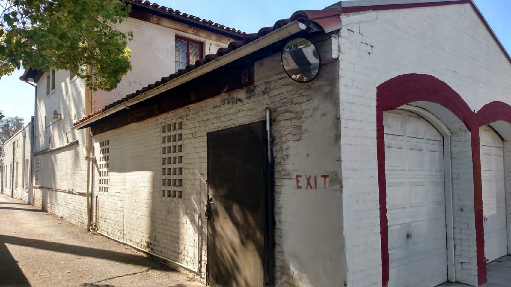
Secondary elevation (south), view facing northwest. Photo by: Andrea Griego, 2019.
