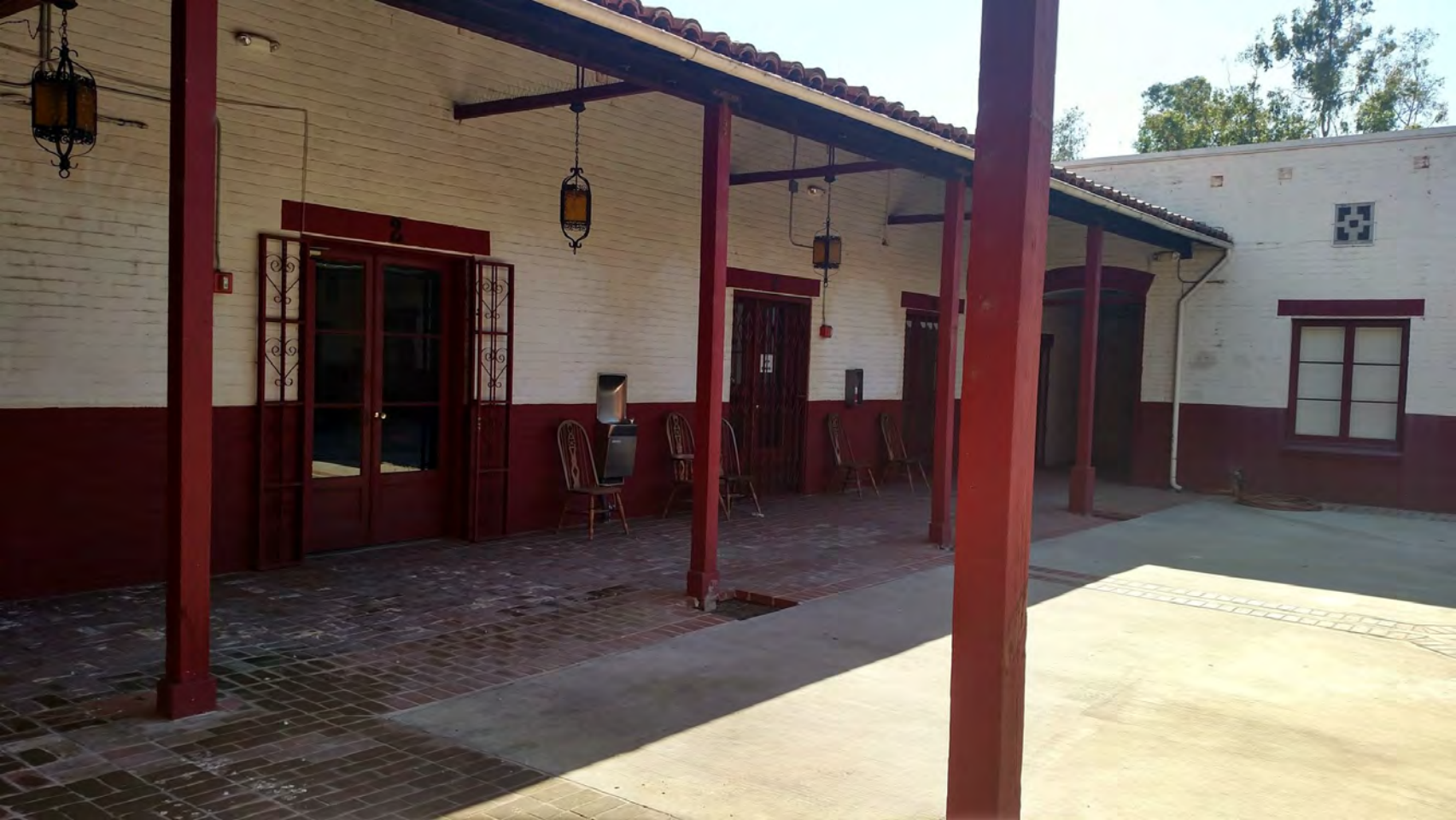
Main courtyard, view southwest. Photo by: Andrea Griego, 2019.
