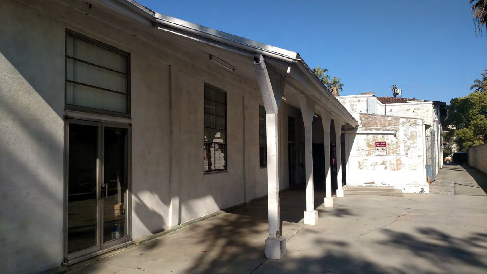
Covered walkway at south facade, view northeast. Photo by: M. Rosalind Sagara/L.A. Conservancy, 2019.
