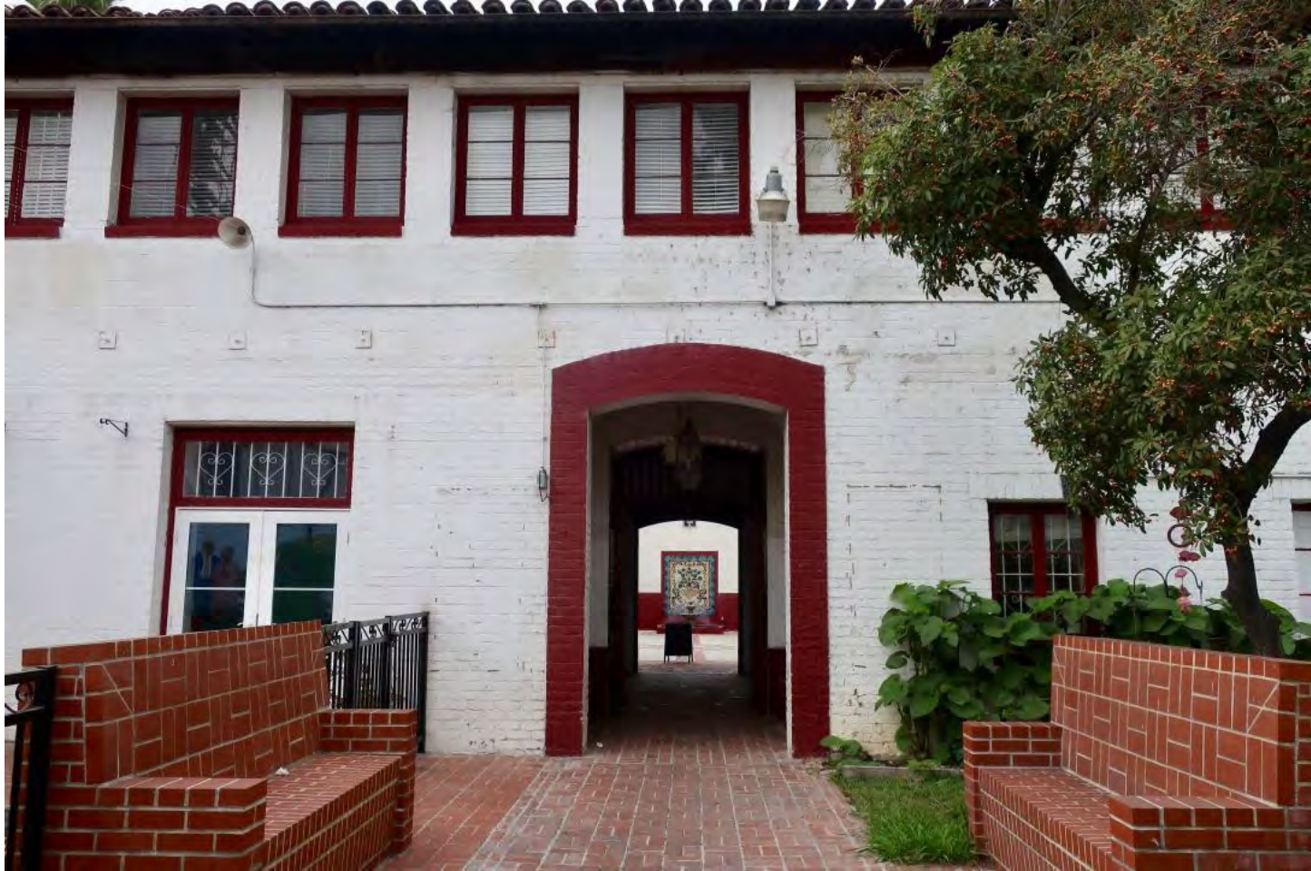
Forecourt, view west. Photo by Laura Dominguez, 2017.
