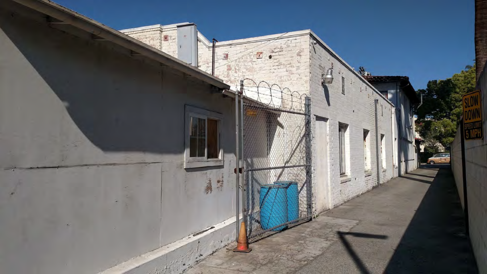
Secondary elevation (south), view east. Photo by: Andrea Griego, 2019.
