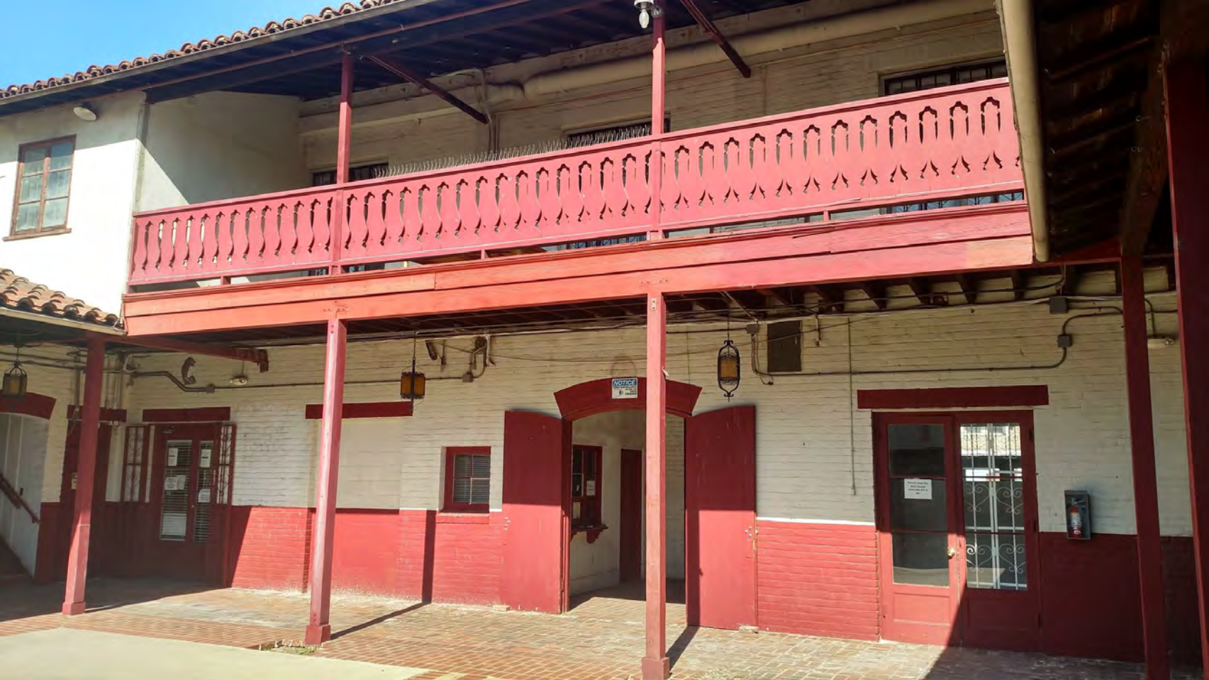
Balcony on north courtyard facade, view northeast. Photo by: Andrea Griego, 2019.
