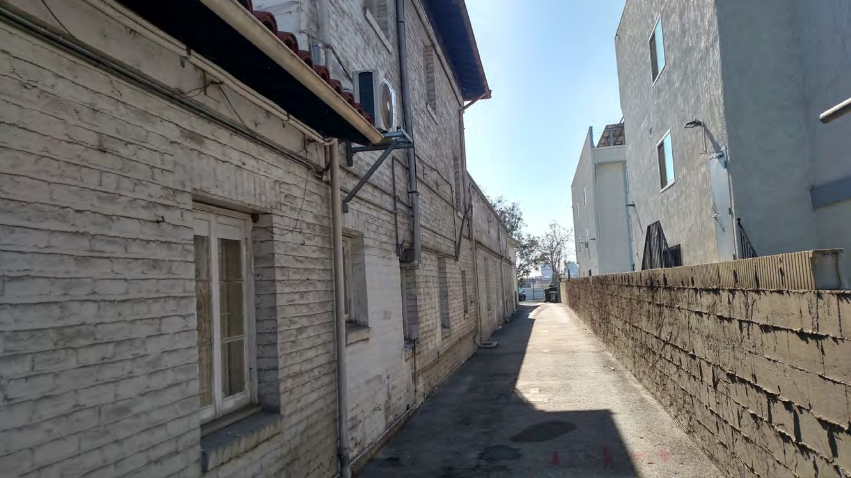
Secondary elevation (north), view west. Photo by: Andrea Griego, 2019.
