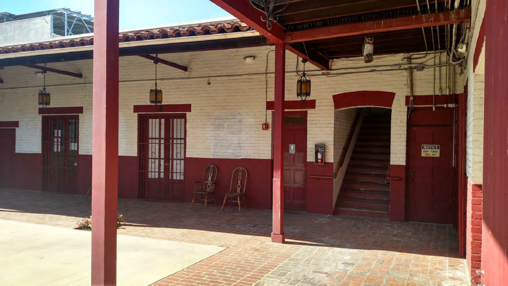
Main courtyard, view north exiting entry hallway. Photo by: Andrea Griego, 2019.
