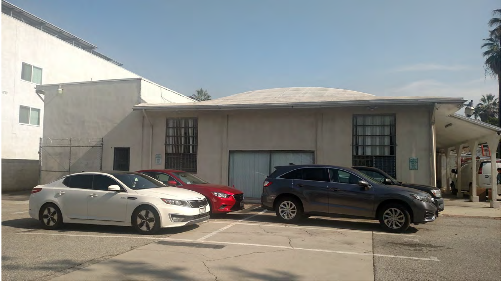
Rear (west) facade, view east. Photo by: Andrea Griego, 2019.
