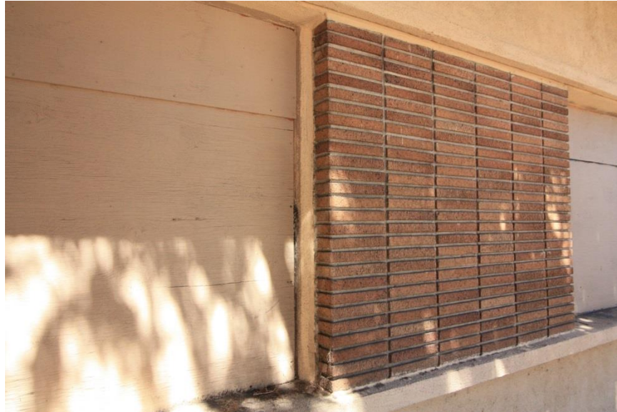
Figure 12. Brick veneer panel located within the stucco window casings along the south elevation. View north. (ESA PCR 2016)
