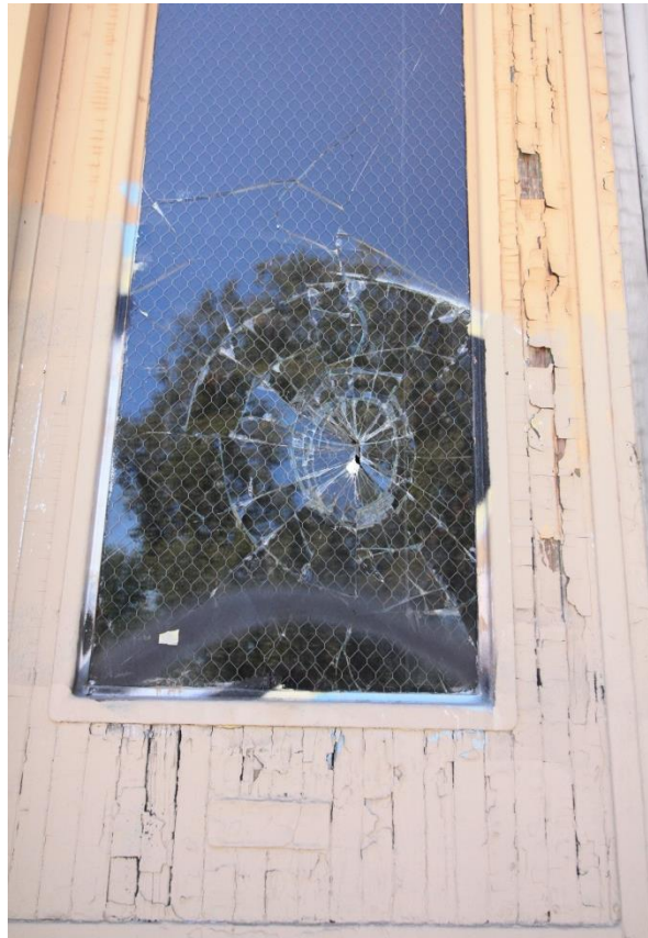
Figure 6. original chicken-wire glass set in the cascading wood garage doors, view west (ESA PCR 2016)
