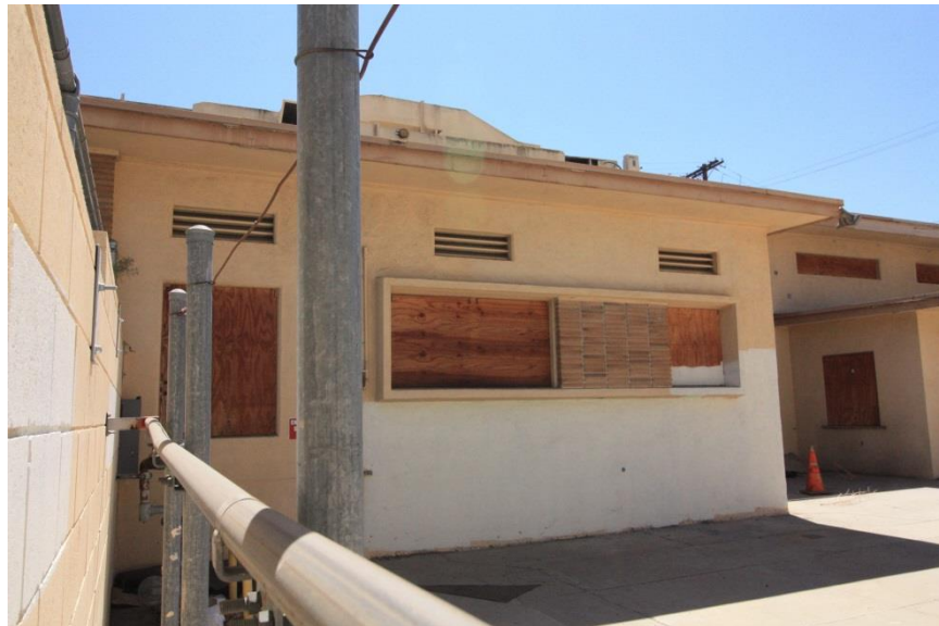
Figure 8. Distinctive stucco window casings with brick panel, view south (ESA PCR 2016)
