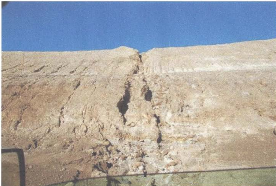
Photo 14: Damage to fill supporting road to Flare 3 from erosion gully shown in Photo 14
