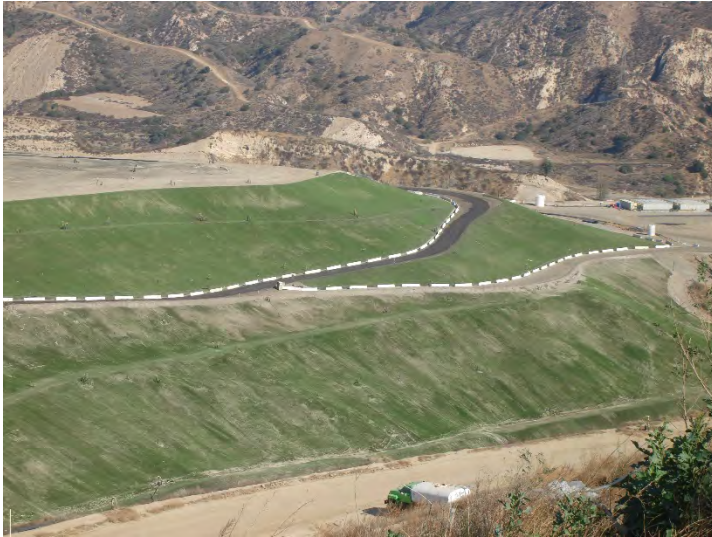
Photo 165: Posi-Shell and Closure Turf: November 20, 2018
