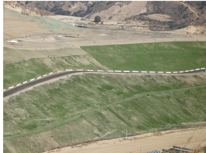
Photo 164: Posi-Shell and Closure Turf: November 20, 2018
