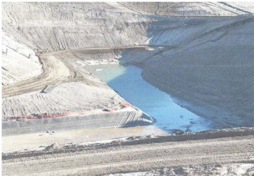
Photo 12: Pumping of water out of moat around Cell CC4 Part 2
