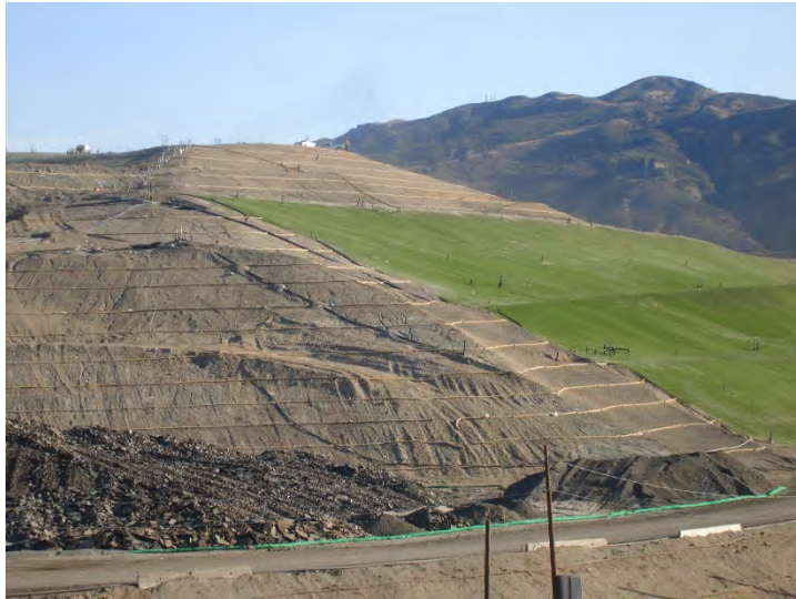
Photo 169: Posi-Shell and Closure Turf: November 20, 2018
