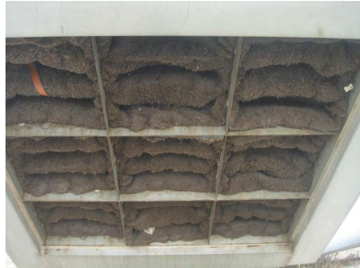
Photo 366: Flare 9 Blower Intake Air Filter: September 25, 2018
