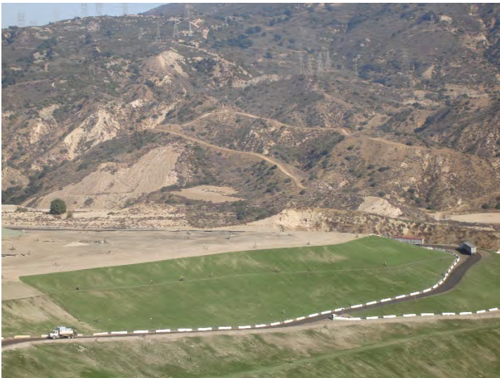
Photo 167: Posi-Shell and Closure Turf: November 20, 2018
