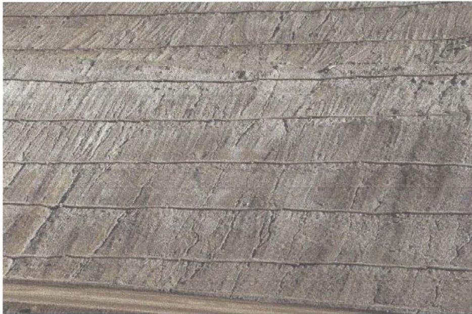
Photo 15: Minor erosion gullies on wattle protected slopes
