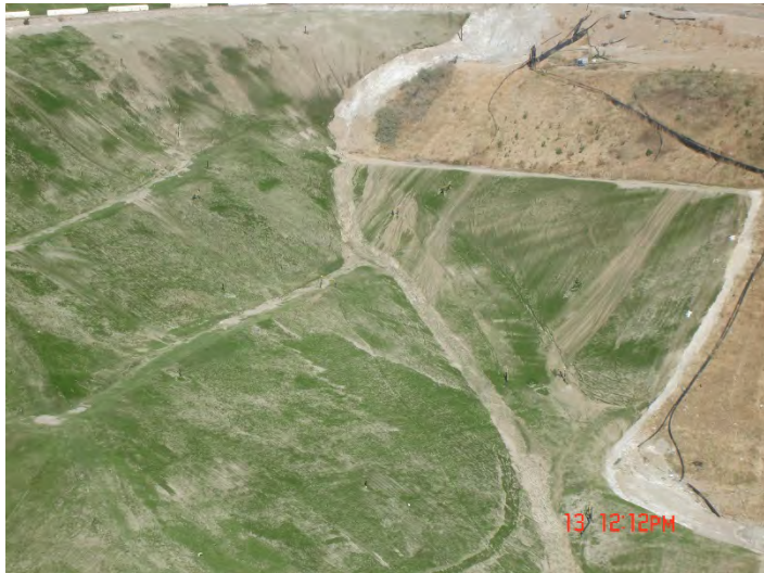
Photo 179: Posi-Shell and Closure Turf: December 13, 2018
