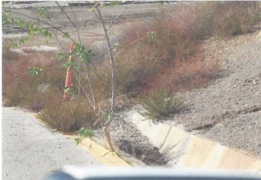
Photo 11: Sediments blocking drainage of ditch along access road to Flares 9-11
