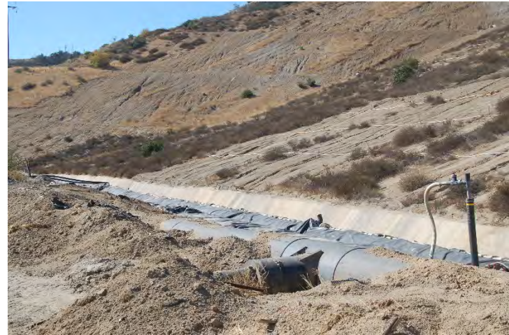
Photo 286: Sacrificial Liner Replacement Near County Sage: October 13, 2018
