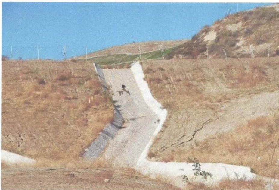
Photo 6: Erosion gullies on downstream side of embankment of cell CC3 basin have reappeared
