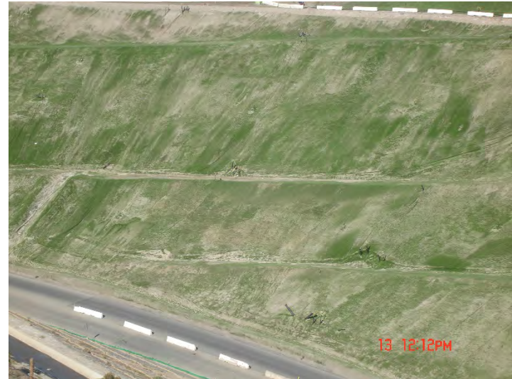
Photo 178: Posi-Shell and Closure Turf: December 13, 2018
