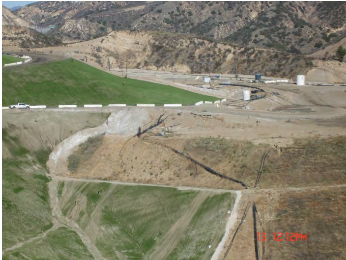
Photo 177: Posi-Shell and Closure Turf: December 13, 2018
