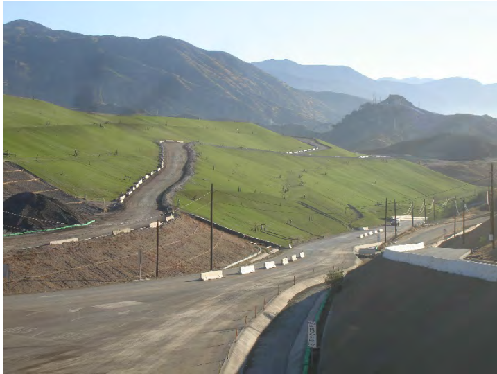
Photo 153: Posi-Shell and Closure Turf: October 23, 2018
