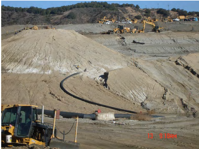
Photo 73: County Soil Stockpile Erosion Near CC-4 Parts 1&2: December 13, 2018
