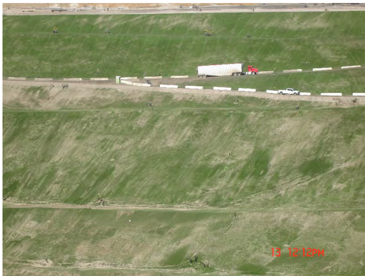
Photo 175: Posi-Shell and Closure Turf: December 13, 2018
