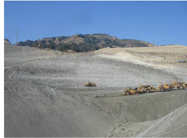
Photo 104: CC4 Part 3 Buttress Excavation Area: November 6, 2018
