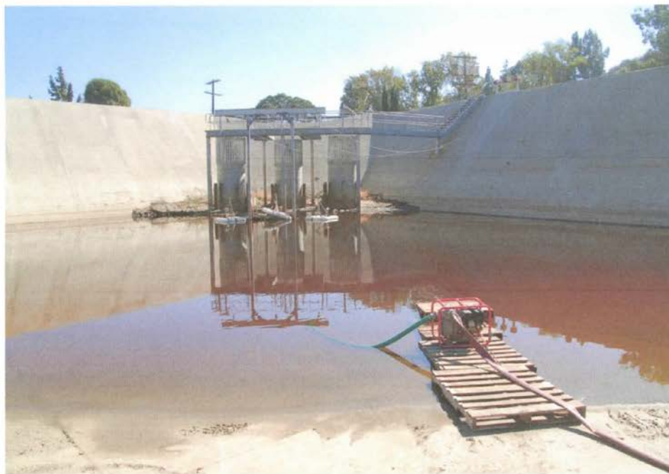
Photo 6: Lowered skimmers and ponding water at Terminal basin
