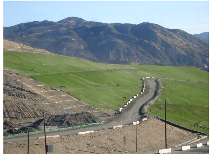
Photo 170: Posi-Shell and Closure Turf: November 20, 2018
