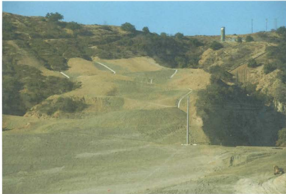
Photo 15: Shotcrete ditches on slope beneath Flare 3
