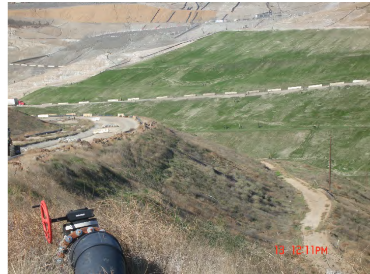
Photo 172: Posi-Shell and Closure Turf: December 13, 2018
