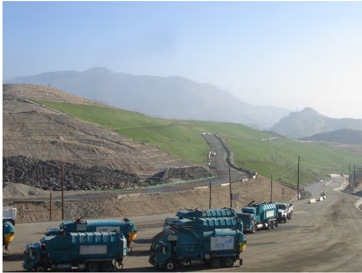
Photo 157: Posi-Shell and Closure Turf: November 6, 2018
