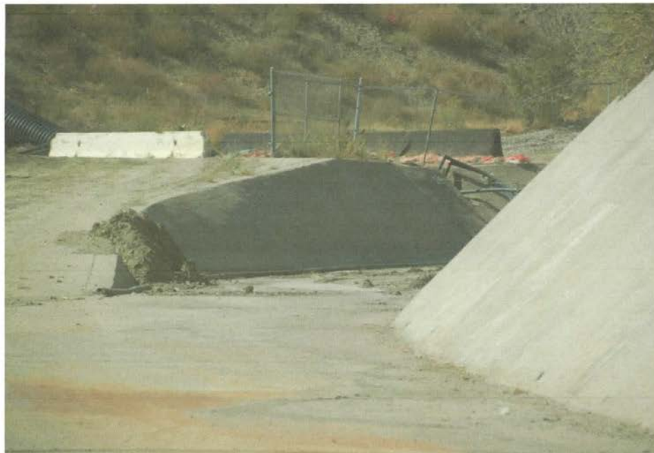
Photo 8: Earth check dam removed at Terminal basin
