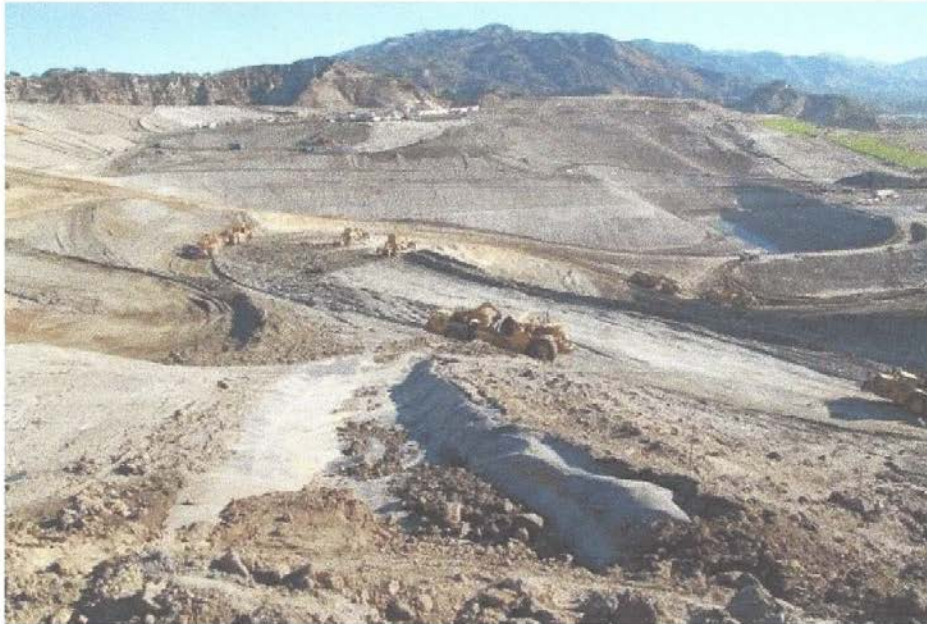
Photo 9: Lined swale to drain Basin A towards temporary basin at toe of buttress
