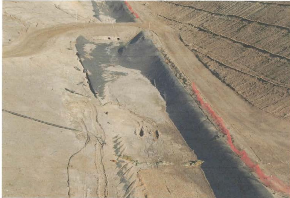
Photo 11: Sediments in moat around Cell CC4 Part 2
