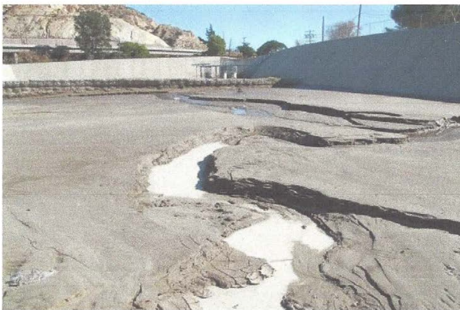
Photo 4: Sediment behind the separator gabion wall of Terminal Basin
