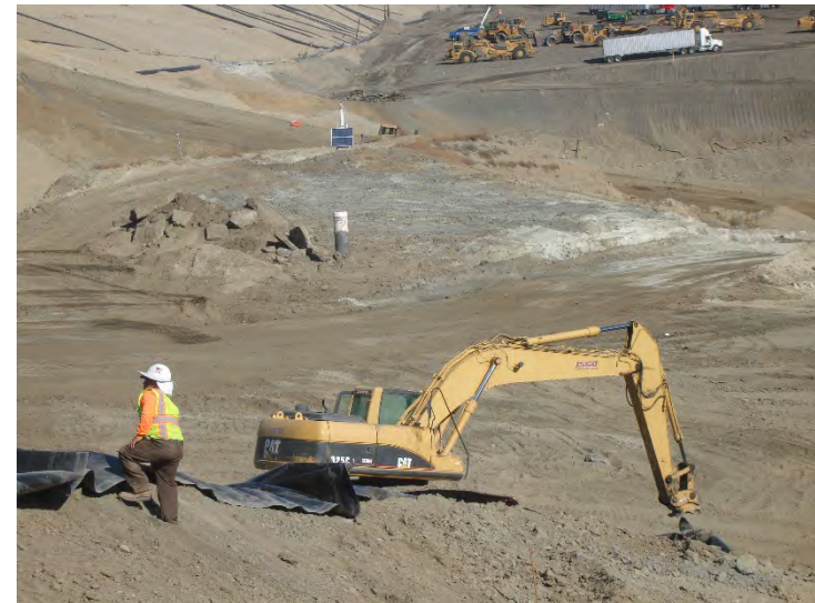
Photo 24: Basin A Temporary Outlet HDPE Channel: November 20, 2018
