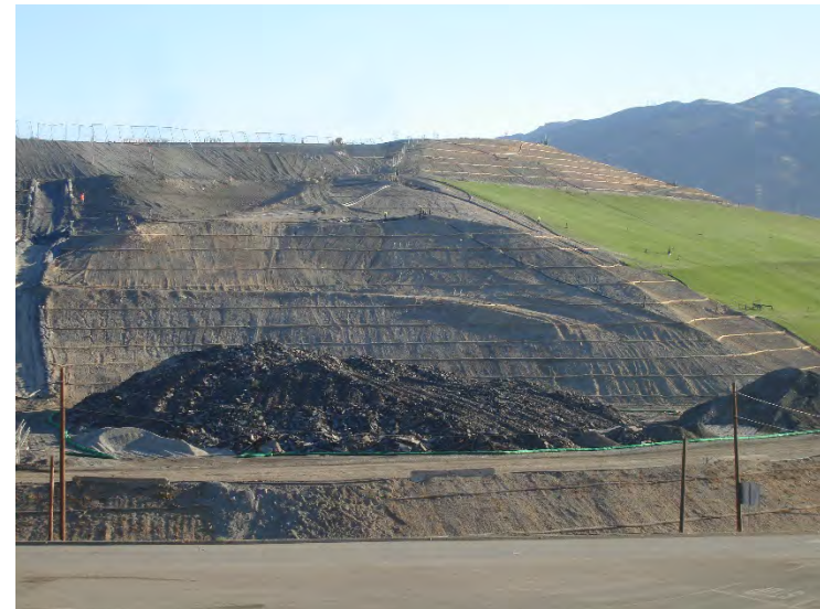
Photo 152: Posi-Shell and Closure Turf: October 23, 2018
