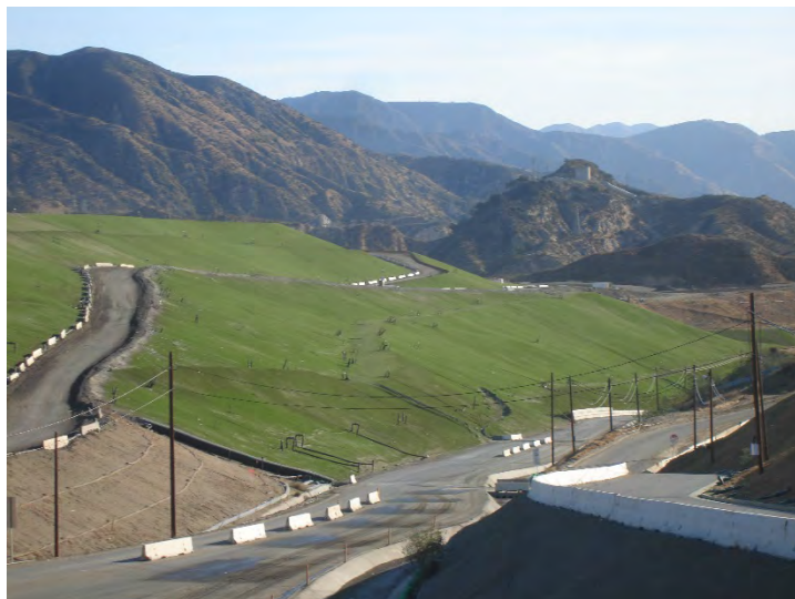
Photo 171: Posi-Shell and Closure Turf: November 20, 2018
