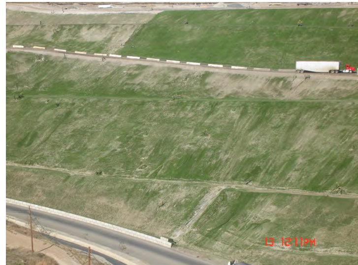
Photo 174: Posi-Shell and Closure Turf: December 13, 2018
