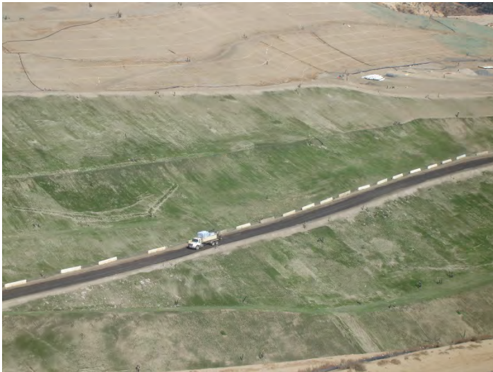
Photo 163: Posi-Shell and Closure Turf: November 20, 2018
