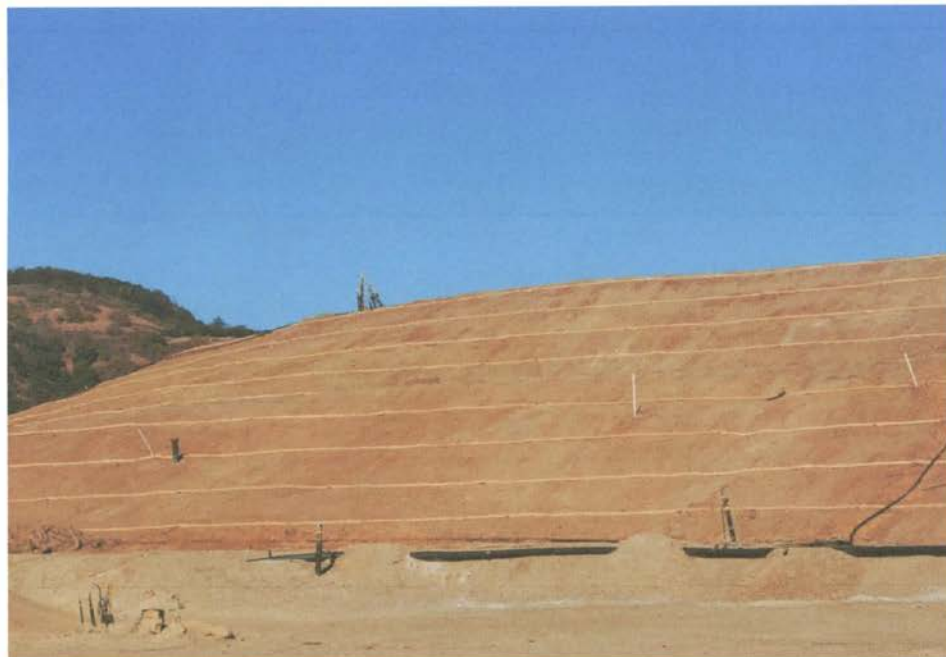
Photo 13: Erosion protection BMPs behind the administration buildings
