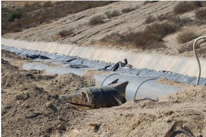
Photo 285: Sacrificial Liner Replacement Near County Sage: October 13, 2018
