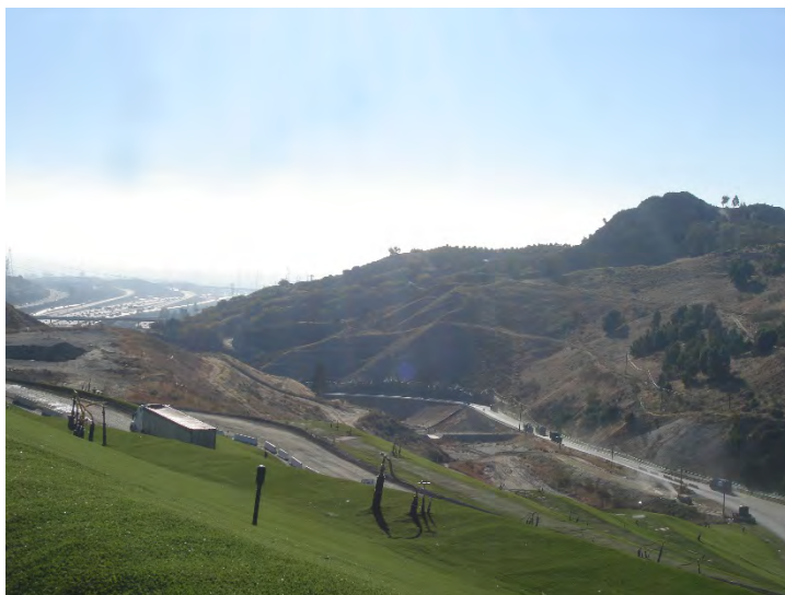
Photo 155: Posi-Shell and Closure Turf: October 23, 2018
