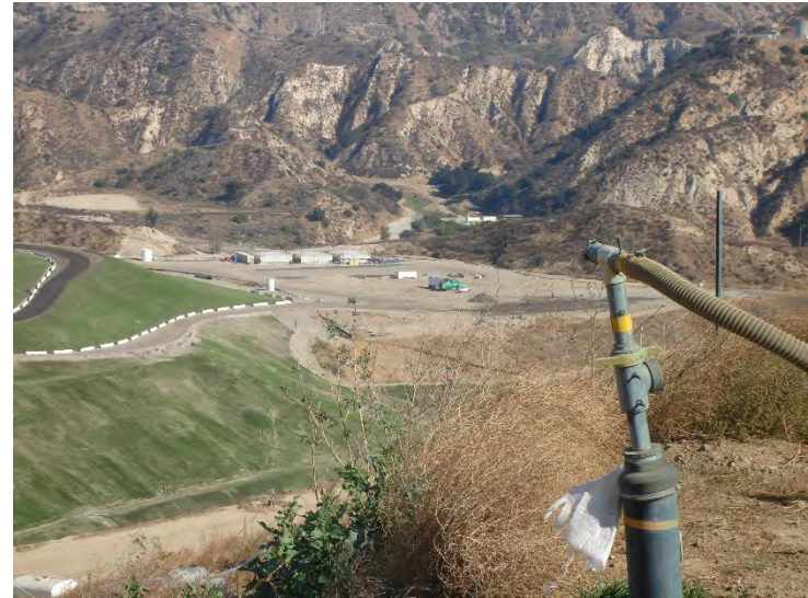
Photo 166: Posi-Shell and Closure Turf: November 20, 2018
