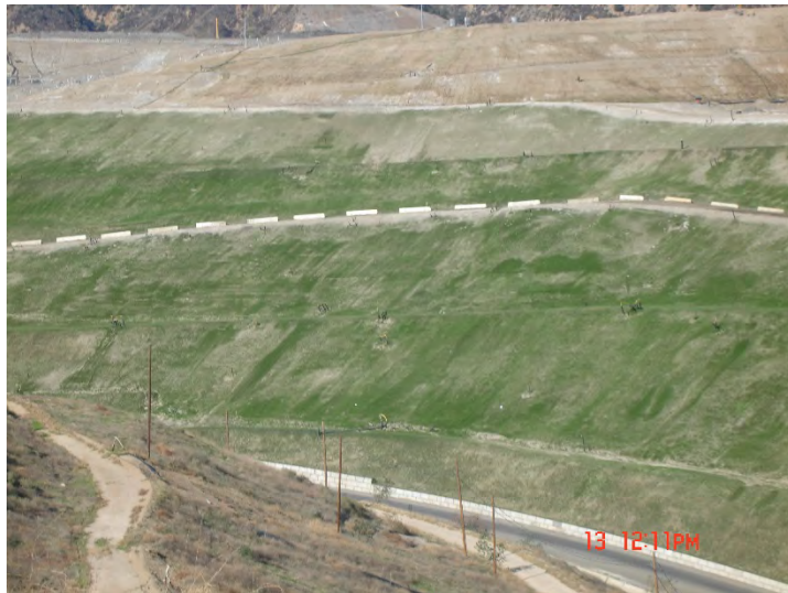
Photo 173: Posi-Shell and Closure Turf: December 13, 2018
