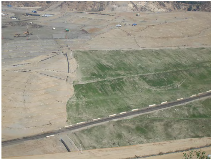
Photo 159: Posi-Shell and Closure Turf: November 6, 2018
