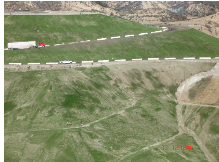
Photo 176: Posi-Shell and Closure Turf: December 13, 2018
