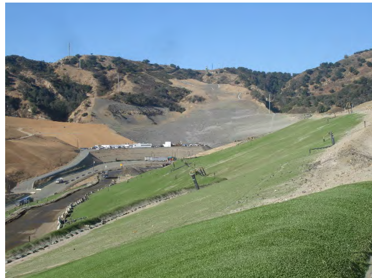
Photo 156: Posi-Shell and Closure Turf: October 23, 2018
