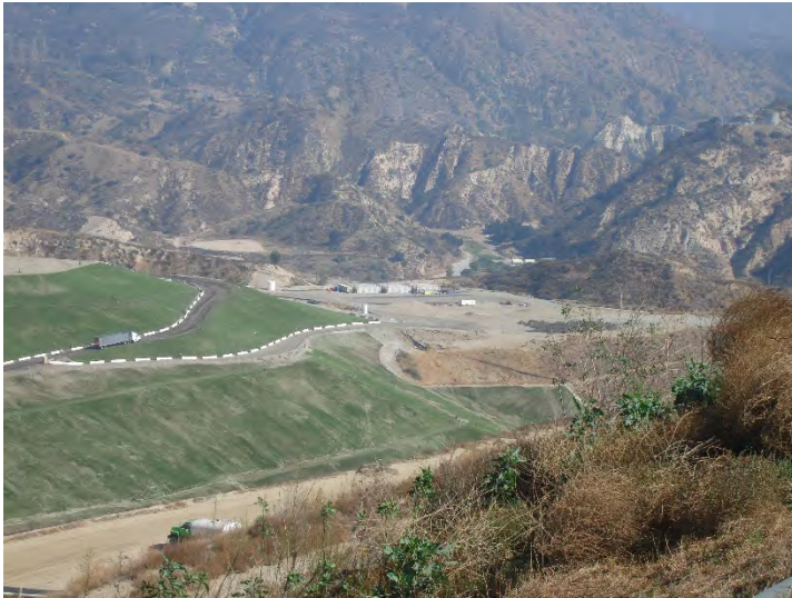
Photo 161: Posi-Shell and Closure Turf: November 6, 2018
