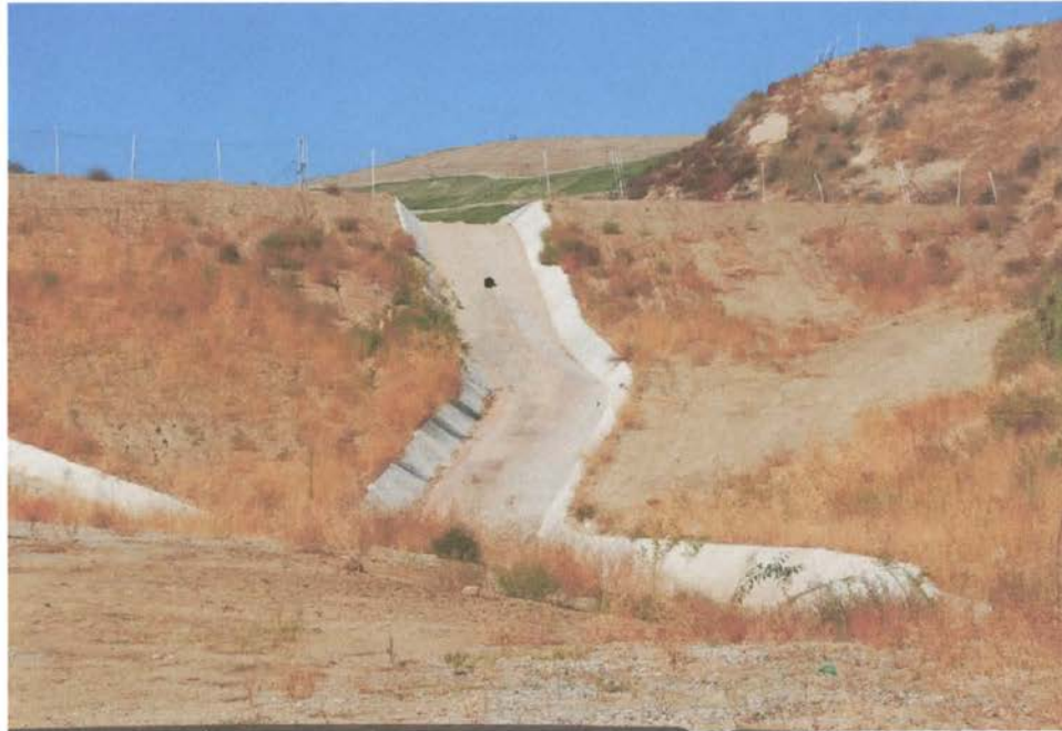
Photo 9: Repaired erosion gullies on downstream side of embankment of cell CC3 basin
