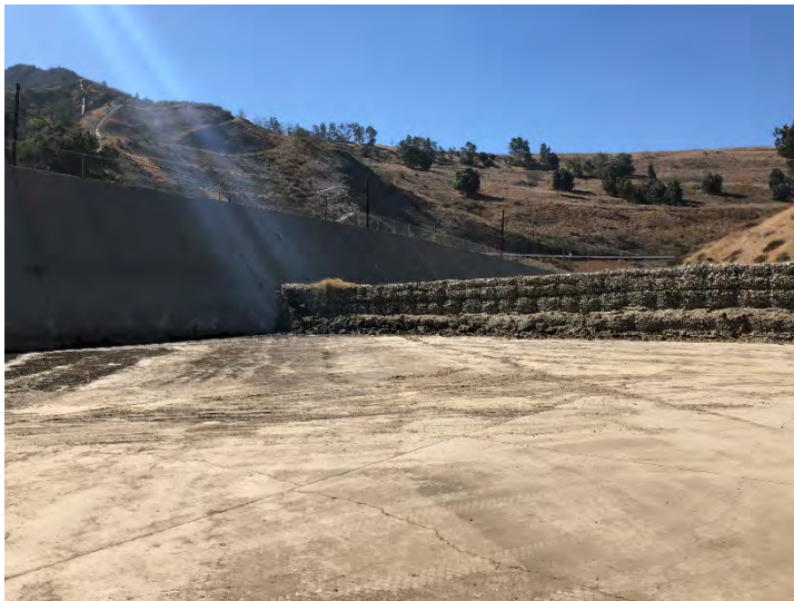
Photo 387: Terminal Basin Gabion Wall: July 24, 2018
