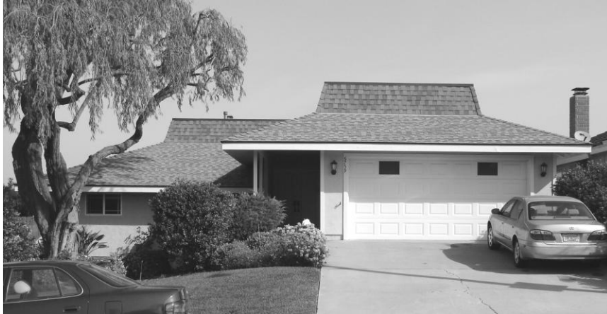
San Diego, ca. 1971. The inverted-Mansard roof conjures a tropical or South-Pacific association.
