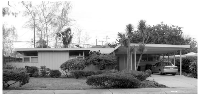
The Meadows tract, Palo Alto, Santa Clara County. Built ca. 1953 by Burke and Wyatt.
