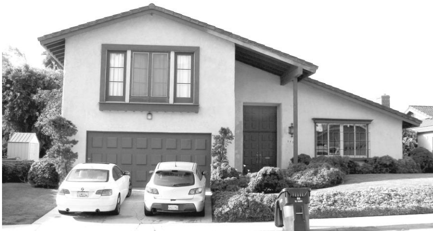
San Simeon tract, San Diego, ca. 1968. This sweeping-roof house is given a Spanish accent with a heavily paneled garage door and front door. Note also the deeply recessed front door, suggesting walls of thick adobe construction. (In fact, the walls are stucco over conventional wood framing.)
