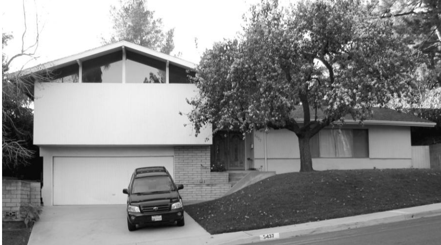
Pinecrest tract in Glendale, Los Angeles County, ca. 1967. The form is typical of California split-levels, with the garage lower than the main living level and the upper level above the garage.
