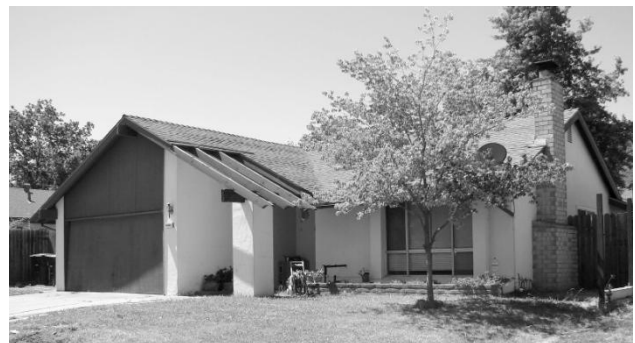
North Ridge tract, Sacramento County. Built ca. 1971 by Larchmont Homes.
