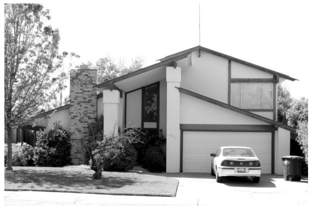
North Ridge tract, Sacramento County. Built ca. 1971 by Larchmont Homes.
