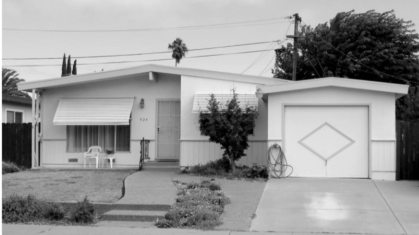
Fairfield, Solano County, ca. 1952. The one-piece, tilt-up garage door with decorative wood trim is typical of Postwar Minimal houses.
