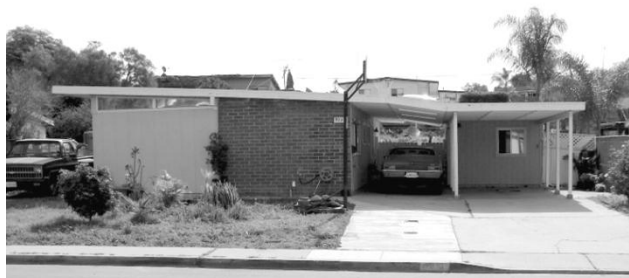
Country Club Park tract, Chula Vista, San Diego County. Built ca. 1954 by Sam Berger Construction.
