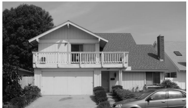
San Diego. Built ca. 1972 by Larwin Construction.
