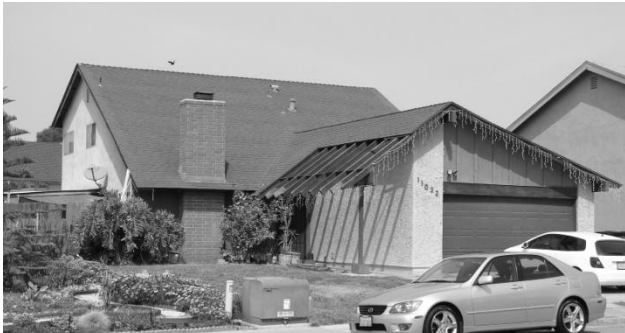
San Diego. Built ca. 1972 by Larwin Construction.
