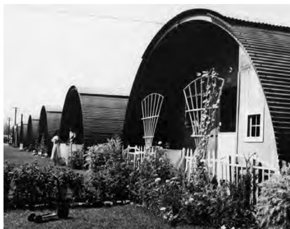
Quonset hut duplex residences at Rodger Young Village, 1950. (Leonard Nadel, photographer. Courtesy of the Los Angeles Public Library.)
