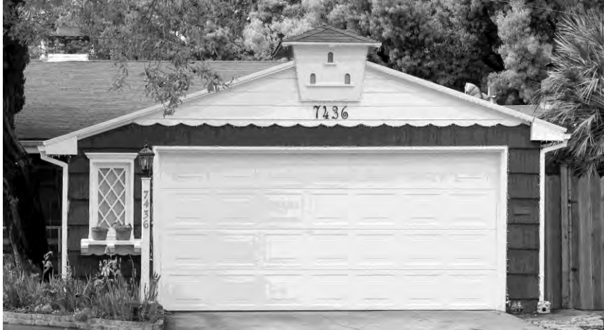
The four-panel, roll-up door on this Storybook house is a later replacement, but does not significantly detract from the overall character of the house.
