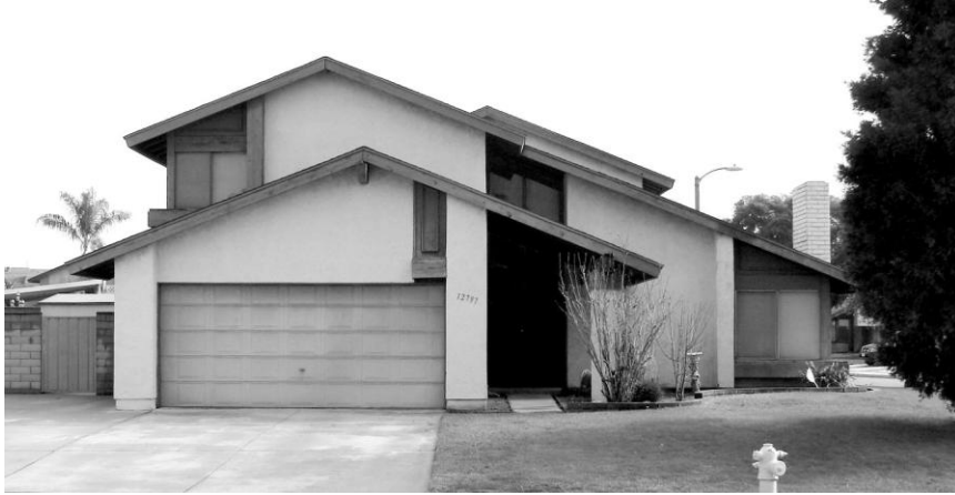
Chino, San Bernardino County. Built ca. 1973 by Ponderosa Homes. The entire width of this house is covered by a broad, asymmetrical gable, with a secondary gable covering the garage and entry area.
