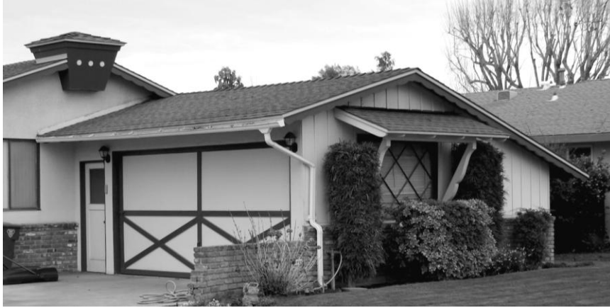
This Rustic Ranch in Bakersfield features x-bracing on the garage door, a diamond-pane window sheltered by a pent roof with shaped brackets, and a prominent (but fake) birdhouse.
