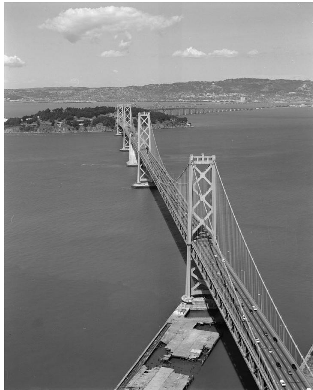
San Francisco – Oakland Bay Bridge, completed in 1936. (Frank Deras, Jr., photographer, 1998, Historic American Engineering Record Collection. Courtesy of the Library of Congress, Prints & Photographs Division.)
