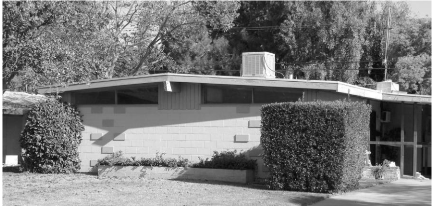
Contemporary style house of concrete block in Fresno, with glazing in the shallow gable.
