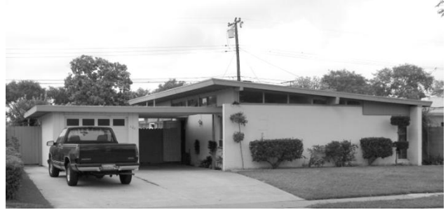
Fullerton Grove tract, Fullerton, Orange County. Built ca. 1953 by Pardee-Phillips Construction. Jones and Emmons, architects.
