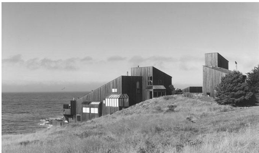
Condominium Building One at Sea Ranch, Sonoma County. Designed by MLTW and built in 1965. (William Turnbull/MLTW Collection, 2000-9. Courtesy of the Environmental Design Archives, University of California-Berkeley.)
