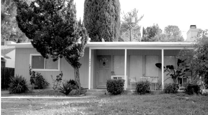
General Panel Corporation house in the San Fernando Valley of Los Angeles. Although the house has been extensively remodeled, the tall, narrow façade windows facing onto the front porch reveal the 40-inch panel width.
