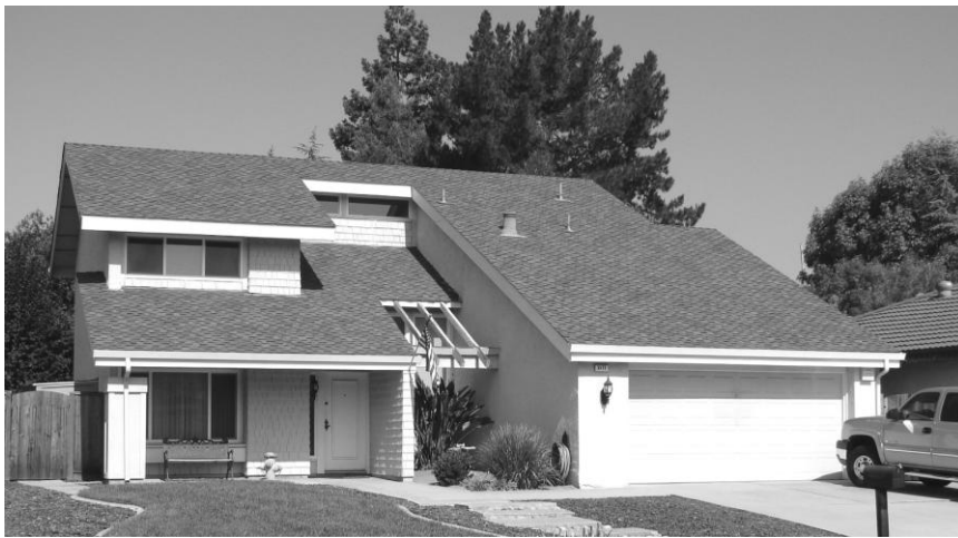
Ponderosa North tract, San Jose. Built ca. 1973 by Ponderosa Homes. With gables at the sides rather than front and rear, the roof is the dominant feature of this house. Note the small roof trellis to the right of the entry.
