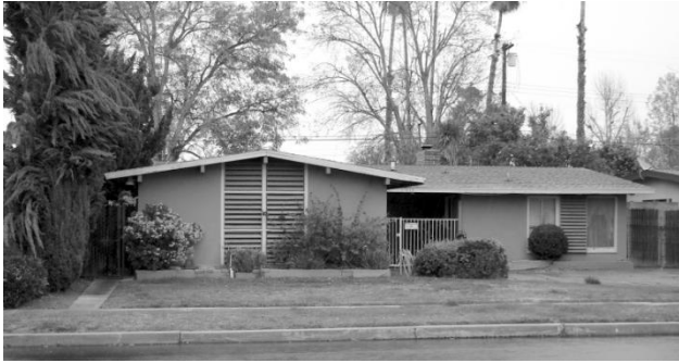
Meadowlark Park tract, Los Angeles. Built ca. 1952 by Ray Hommes. Edward Fickett, architect.
