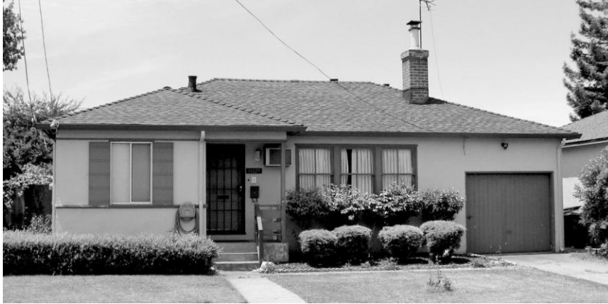
The windows to the right of the front door retain their original double-hung 2/2 wood sash, while the window to the left of the front door is a replacement sliding sash. With only this single alteration, the house could be a contributor to an historic district.
