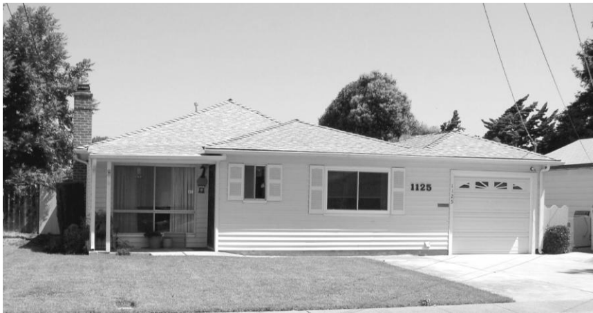
This house, in the same tract as the one shown above, has been extensively altered with a front addition, replacement of the original picture window, new façade windows on the addition, new siding, and a replacement garage door. It would be a non-contributor to an historic district.
