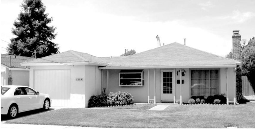
The pop-out window to the left of the front door is not original, but this house is otherwise unaltered and retains sufficient integrity to be a contributor to an historic district.
