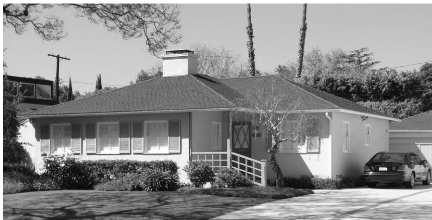
Westdale tract, Los Angeles. The houses in this late-1940s tract have detached garages.
