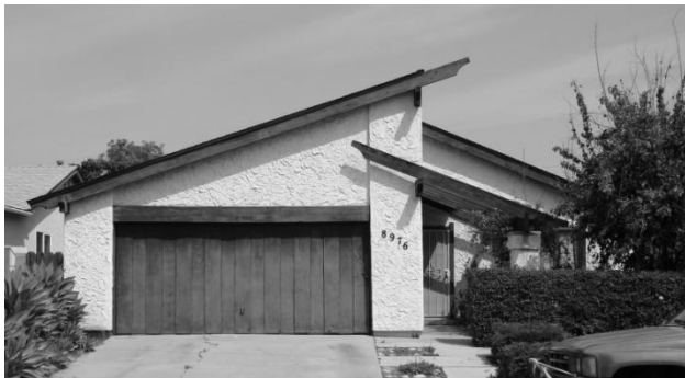
San Diego. Built ca. 1972 by Larwin Construction
