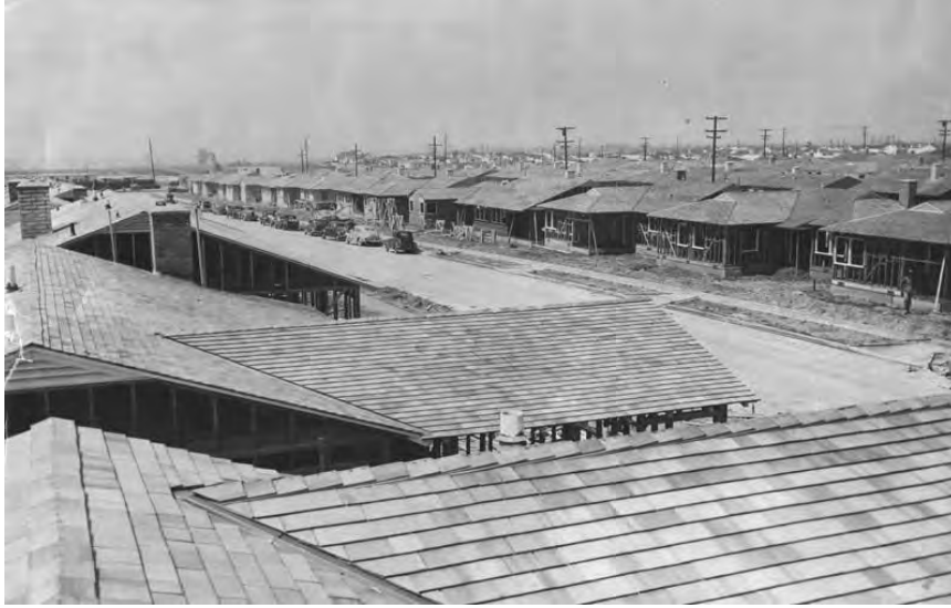
In this view of the Lakewood development in southern Los Angeles County, the street has paving and curbs and the houses have finished roofs, but many do not yet have exterior wall sheathing or finishes. (Lakewood Series, 1950. Courtesy of the Los Angeles Public Library.)
