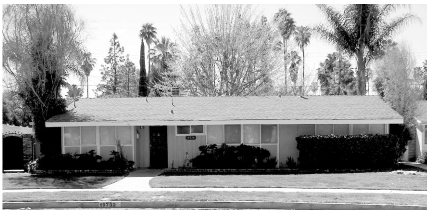
House in the San Fernando Valley of Los Angeles. Edward Fickett, architect.
