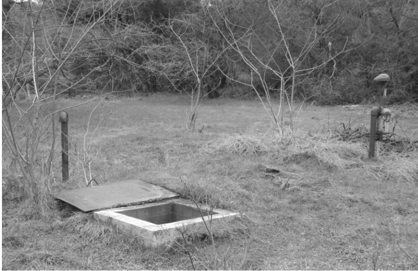
This fallout shelter in Tuolumne County has three features visible above ground: the concrete entrance hatch with a steel door, an exhaust air pipe near the entrance hatch, and a filtered air intake about ten feet away from the entrance hatch. The shelter was determined ineligible for National Register listing, primarily because the associated residence on the property has been demolished.
