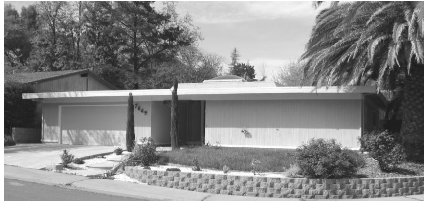
This house in suburban Sacramento is an example of the Streng Brothers' atrium plan, with a plastic dome skylight over the atrium. The exterior walls are raked stucco.
