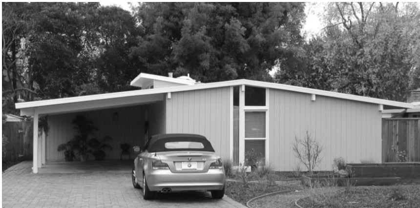
Sunshine Glen tract, Palo Alto, Santa Clara County. Anshen and Allen, architects. Built ca. 1954 by MacKay Homes.
