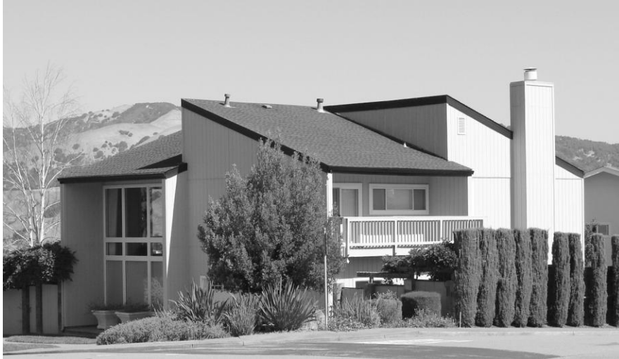
San Rafael, Marin County, ca. 1971. This Sea Ranch style house consists of a cluster of single-pitch roof forms set in a pinwheel pattern.
