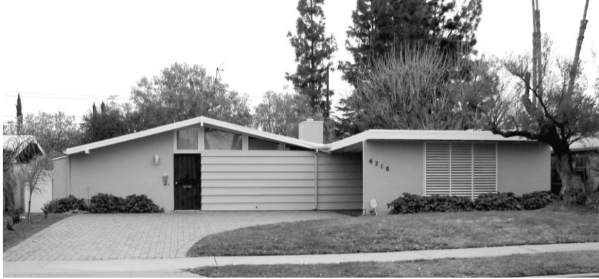
Corbin Palms tract, San Fernando Valley, Los Angeles. Built in 1953 by the Alexander Construction Company.
