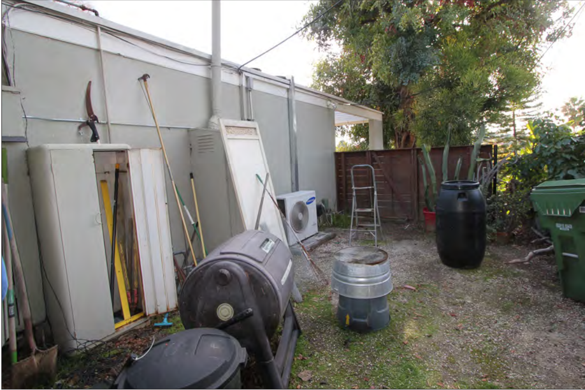
Image 41: Subject property, upper building, west elevation (left), rear yard, view south (Chattel, 2020)
