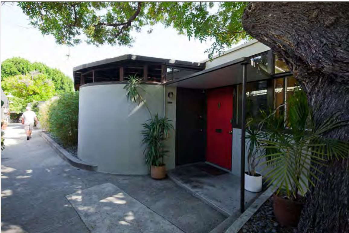
Image 39: Subject property, upper building, north elevation, view south (Kyungsub Shin, 2011)
