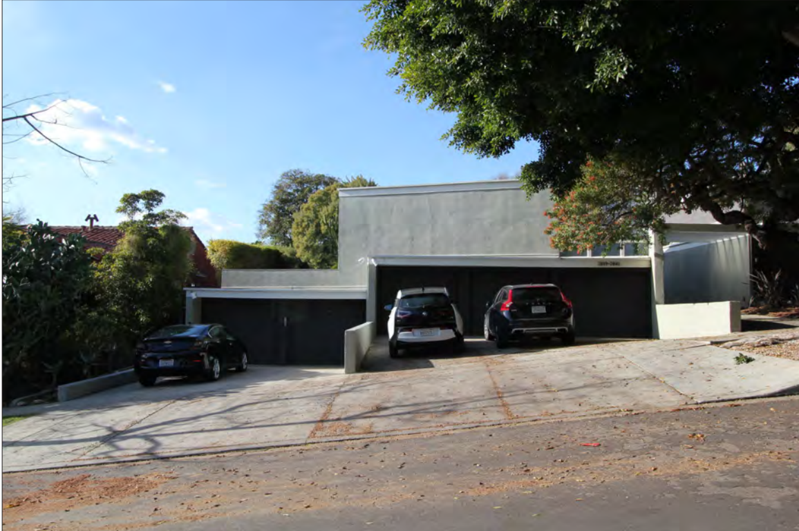
Image 7: Subject property, lower building, east elevation (primary facade), view northwest (Chattel, 2020)
