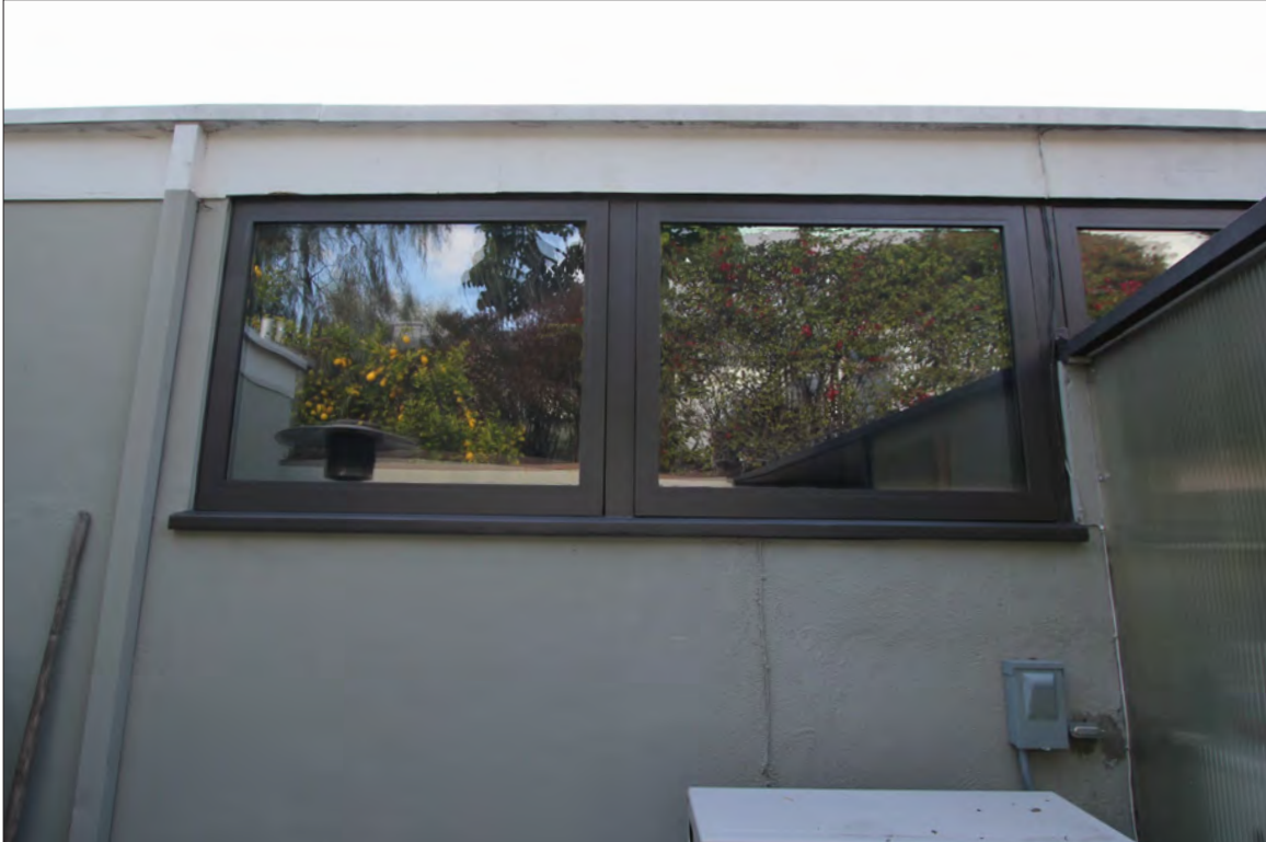
Image 28: Subject property, detail of window at service yard, view southwest (Chattel, 2020)
