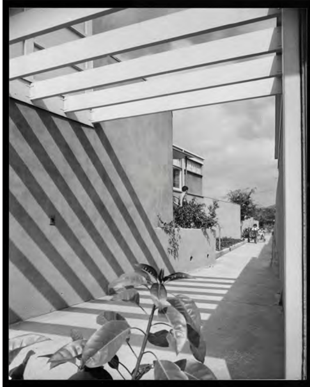
Image 6: Subject property, terraced entrance walkway at north elevation, view west (Julius Shulman Photography Archive, Getty Research Institute Digital Collections, 1949)
