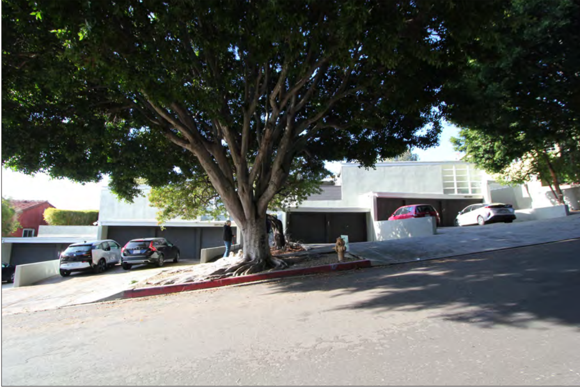
Image 5: Subject property, east elevations (primary facade), view northwest (Chattel, 2020)
