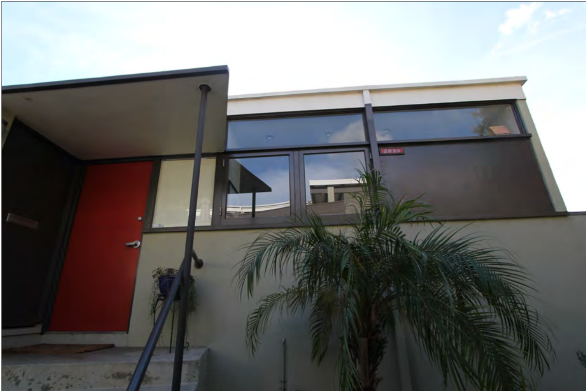
Image 17: Subject property, lower building, north elevation, unit entryway, view southwest (Chattel, 2020)
