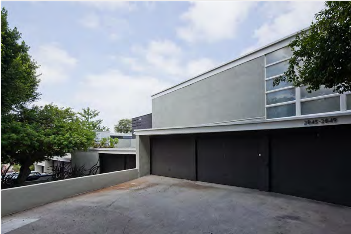
Image 32: Subject property, upper building, east elevation (primary facade), view southwest (Kyungsub Shin, 2011)
