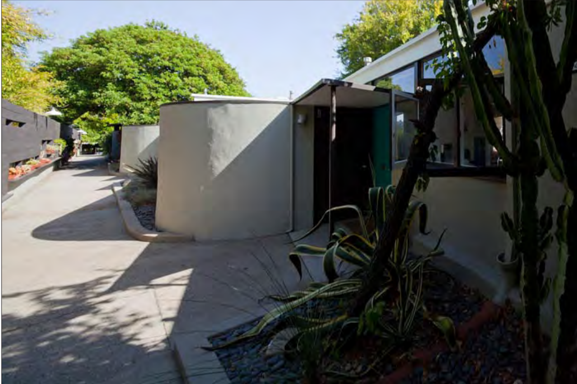
Image 36: Subject property, upper building, north elevation, view southeast (Kyungsub Shin, 2011)
