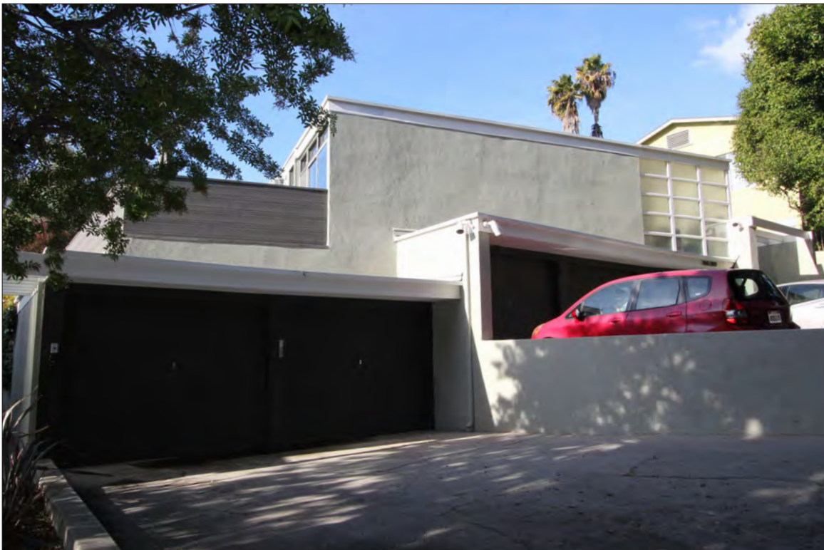
Image 32: Subject property, upper building, east elevation (primary facade), view northwest (Chattel, 2020)
