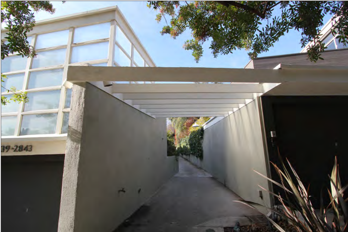
Image 11: Subject property, lower building, terraced entrance walkway at north elevation, (Chattel, 2020)
