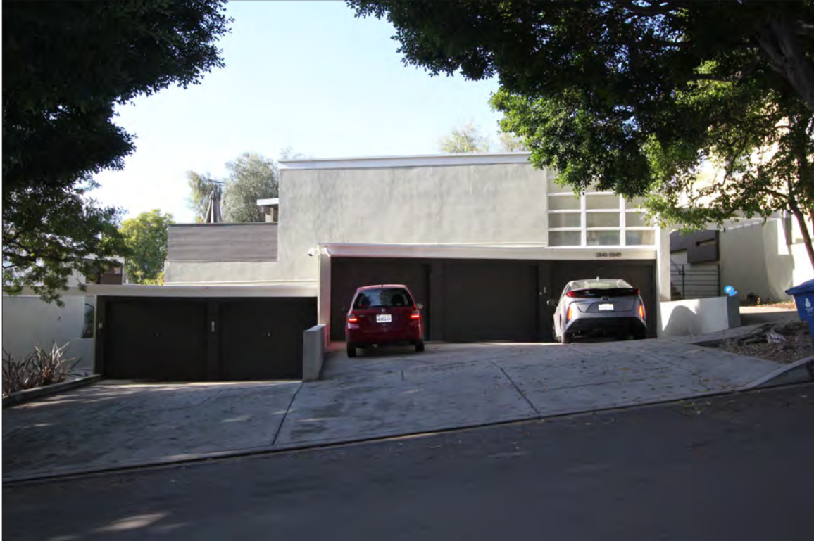
Image 30: Subject property, upper building, east elevation (primary facade), view northwest (Chattel, 2020)
