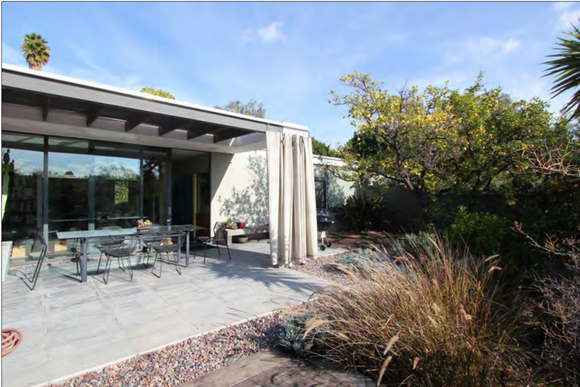
Image 23: Subject property, lower building, south elevation, backyard patio, view east (Chattel, 2020)
