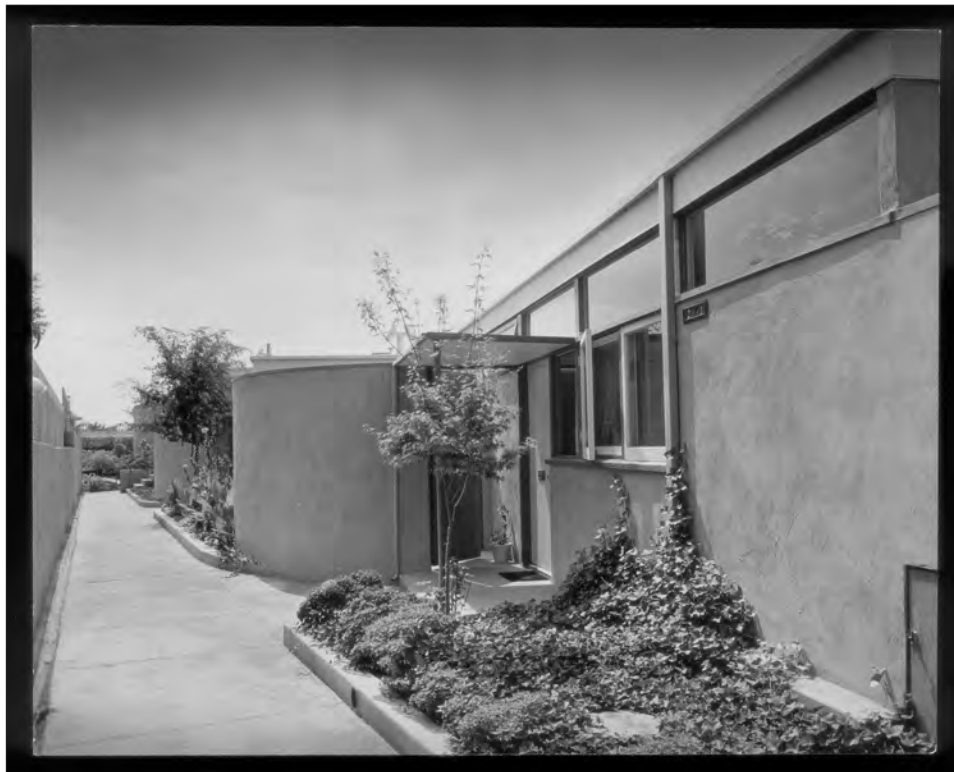
Image 8: Subject property, walkway at north elevation with curved enclosure shielding service yard, view southeast (Julius Shulman Photography Archive, Getty Research Institute Digital Collections, 1949)
