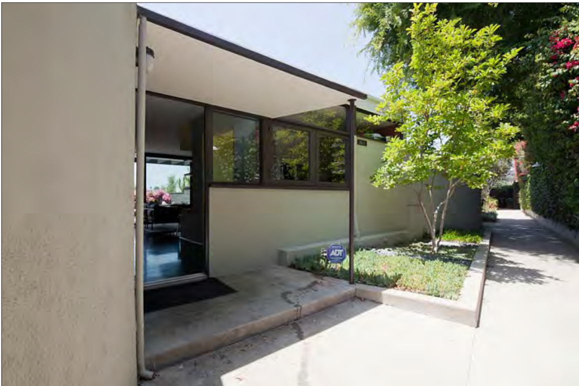
Image 31: Subject property, lower building, north elevation, view west (Kyungsub Shin, 2011)
