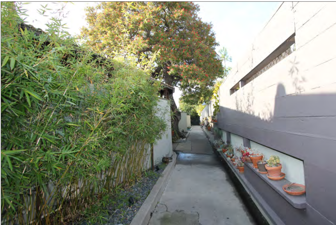
Image 38: Subject property, upper building, north elevation (left), view northwest (Chattel, 2020)
