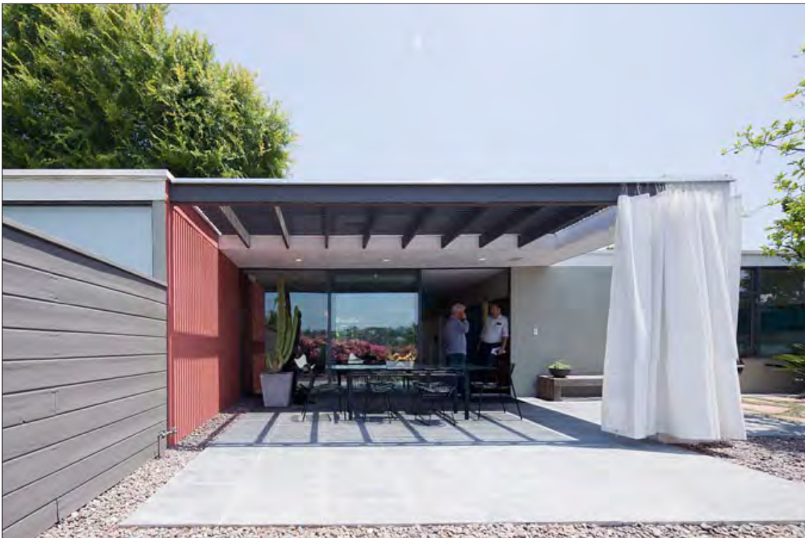
Image 49: Subject property, south elevation, backyard patio, view southwest (Kyungsub Shin, 2011)
