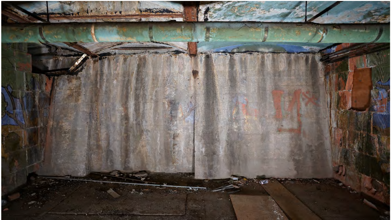
King Edward Hotel Murals in basement of 129-131 E. Fifth Street, facing south Photo taken: Mach 8, 2019
