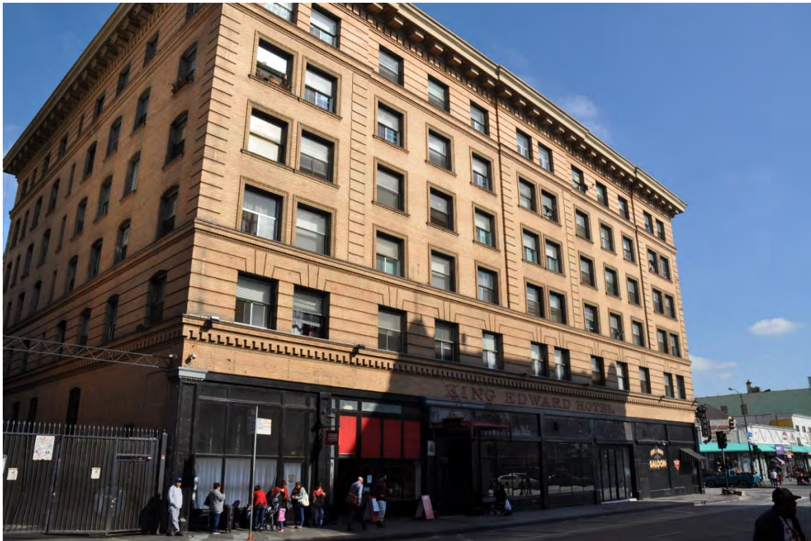
King Edward Hotel South elevation and partial west elevation Photograph taken: December 17, 2018
