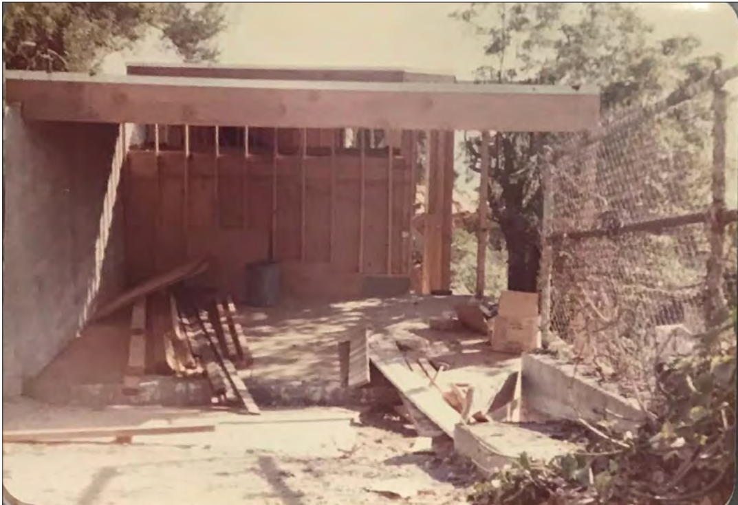
Image 34: 145 Adelaide Drive, construction of studio addition (Huntington Library, 1976)
