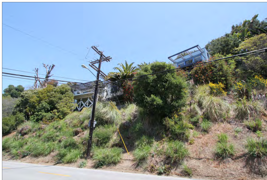
Photo 3: 145 Adelaide Drive, north elevations, view southeast. Note the residence (left) and studio (right) (Chattel, 2018)
