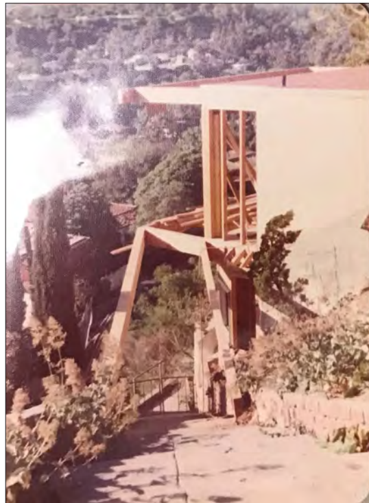
Image 33: 145 Adelaide Drive, construction of studio addition (Huntington Library, 1976)
