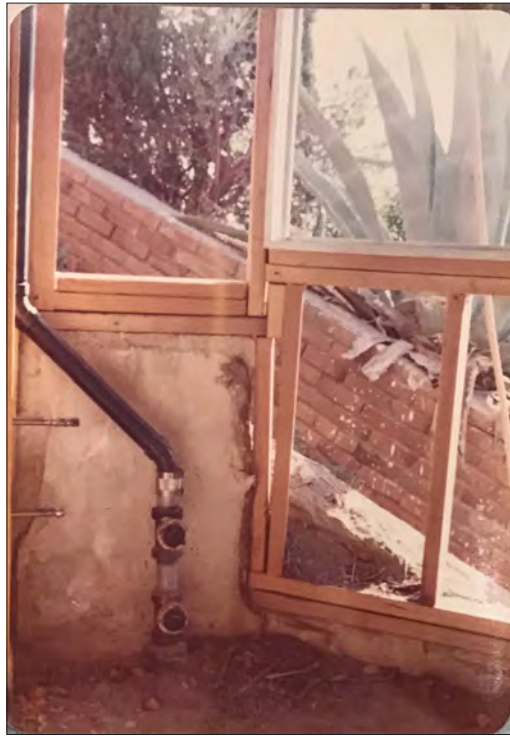
Image 32: 145 Adelaide Drive, construction of studio addition (Huntington Library, 1976)
