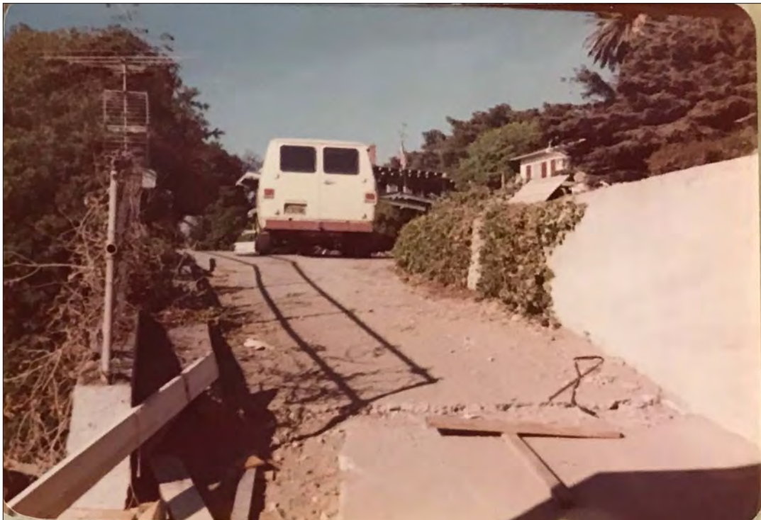
Image 31: 145 Adelaide Drive, construction of studio addition (Huntington Library, 1976)
