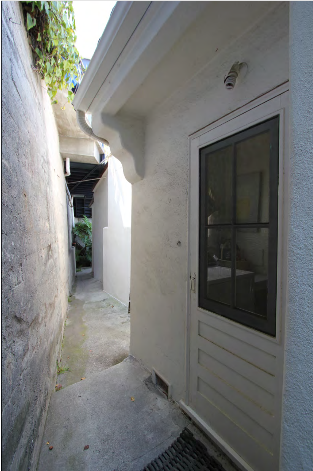
Photo 17: 145 Adelaide Drive, south elevation of residence, view west (Chattel, 2018)
