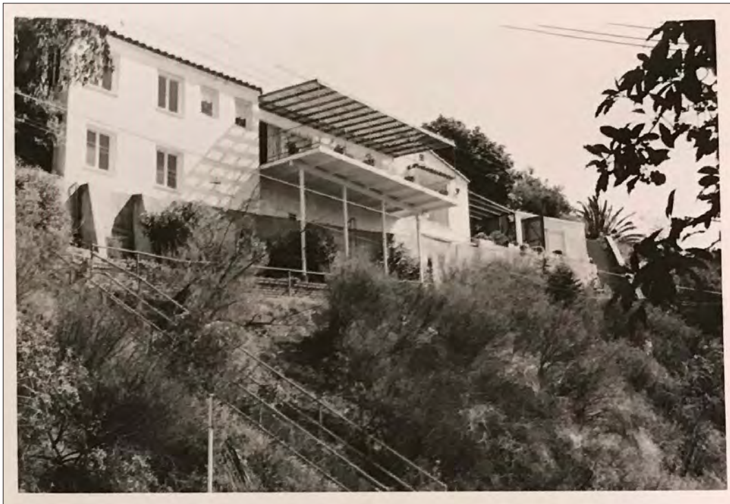
Image 13: 145 Adelaide Drive, residence, view south (Huntington Library, 1963)
