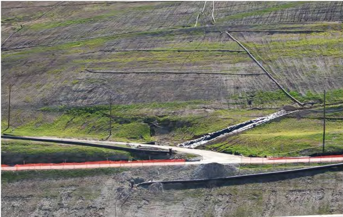
Photo 41: Sloughing at toe of slope above access road at level of Cell CC3
