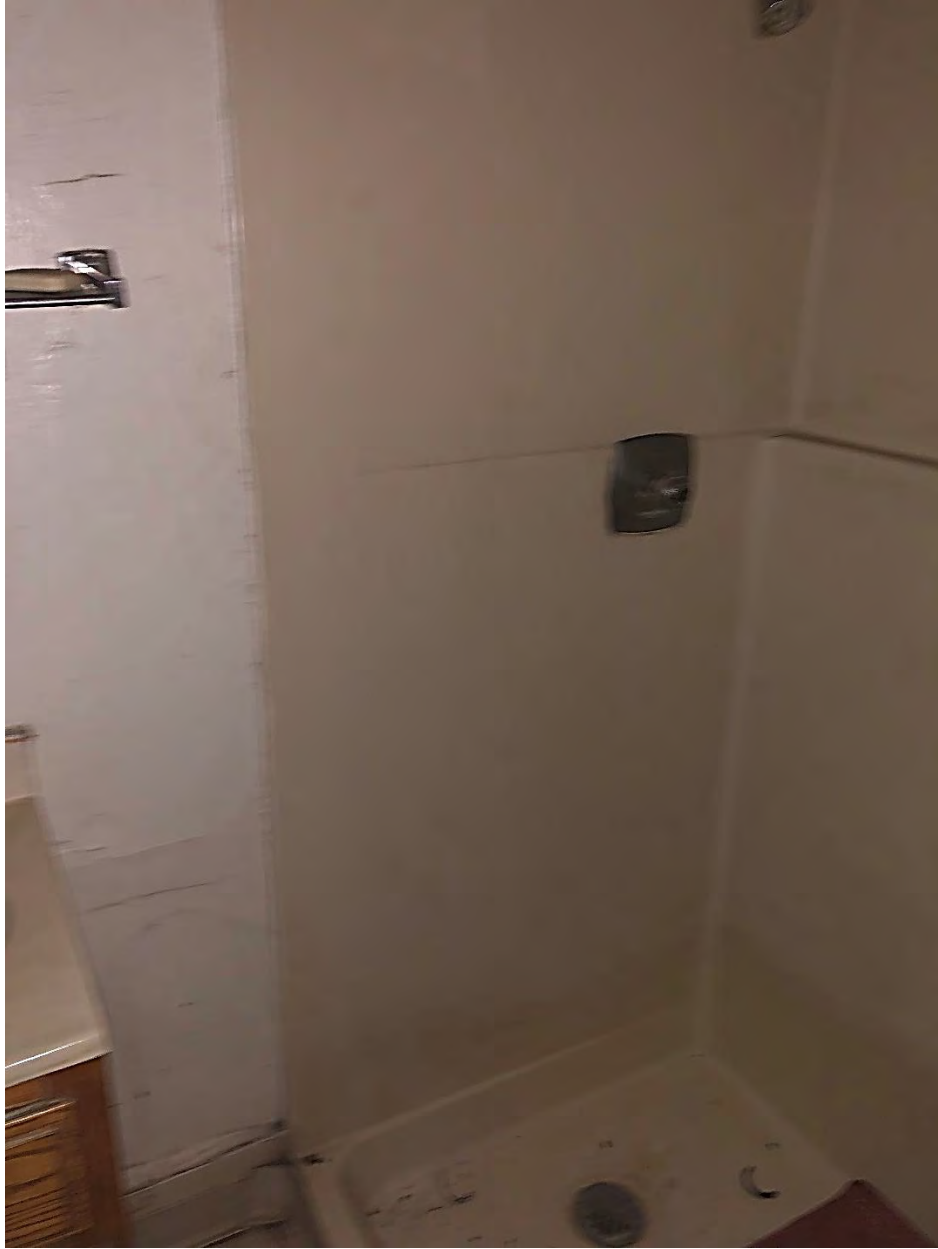
12. 1251-1259 Sunset Boulevard, Manager's Unit, Tub Alteration, June 26, 2020
