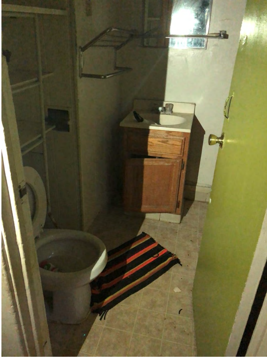
11. 1251-1259 Sunset Boulevard, Manager's Unit, Bathroom Alteration, June 26, 2020
