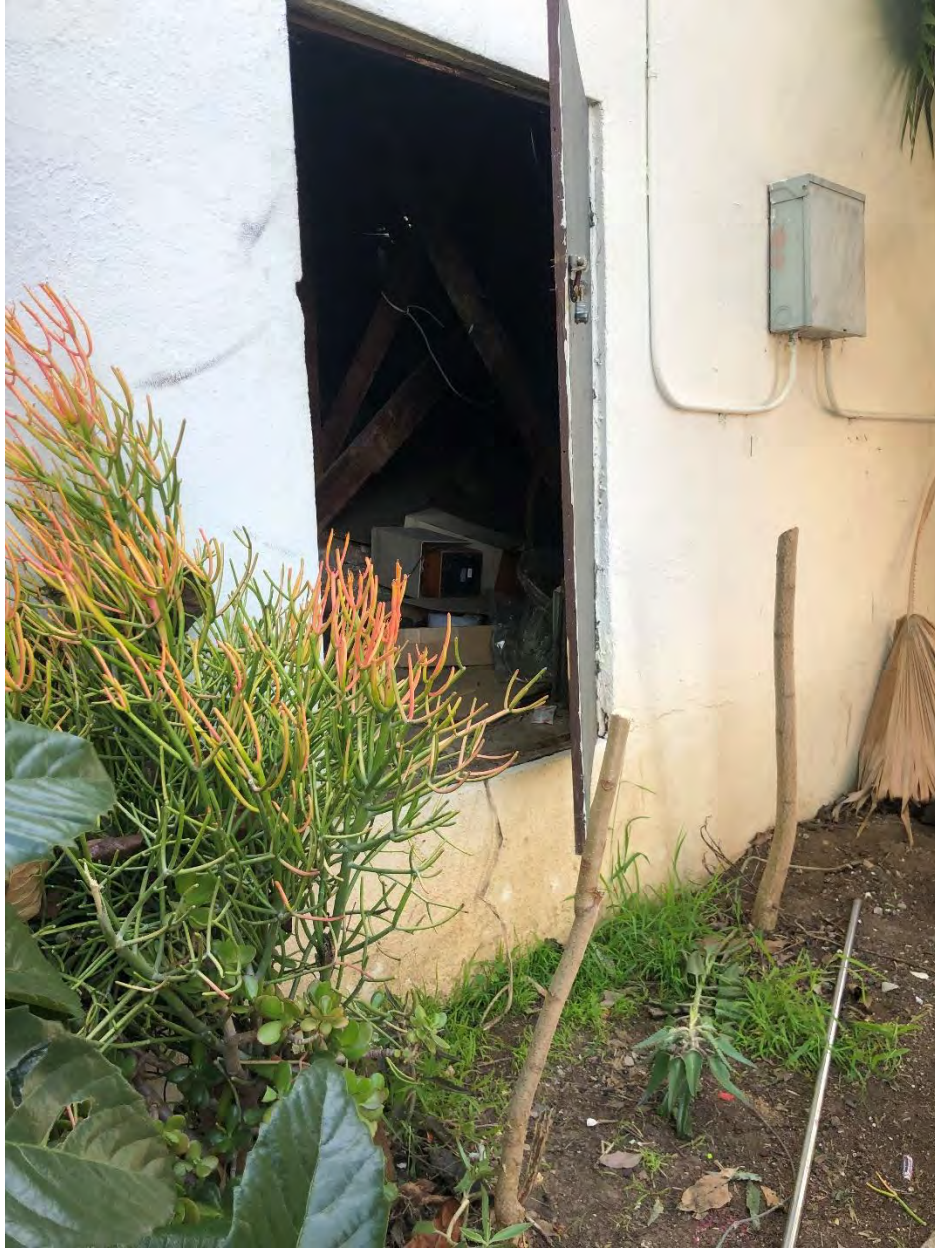
8. 1251–1259 Sunset Boulevard, Crawl Space Below Units; view southeast, April 1, 2020
