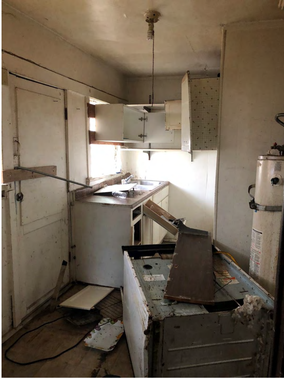
9. 1251-1259 Sunset Boulevard, Manager's Unit, Kitchen Alteration, June 26, 2020
