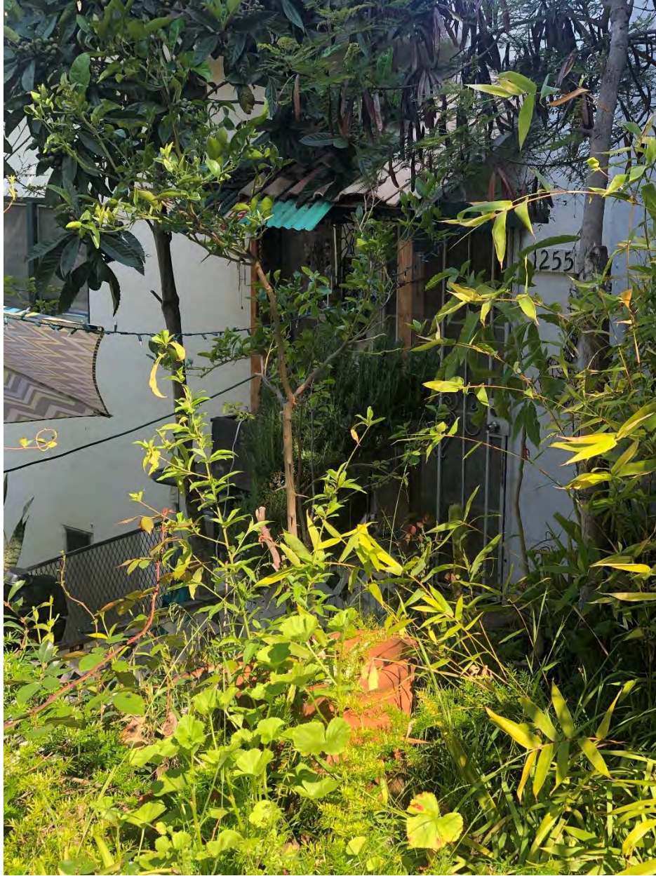
5. 1251–1259 Sunset Boulevard, Individual Bungalow with Corrugated Sheet Metal Awning, view northwest, April 1, 2020
