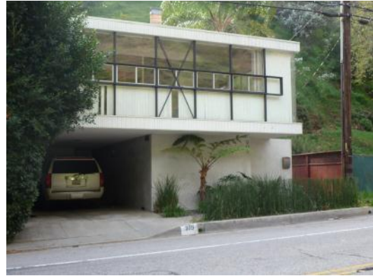
Address: 909 Beverly Glen Boulevard Architect: Craig Elwood Date: 1949
