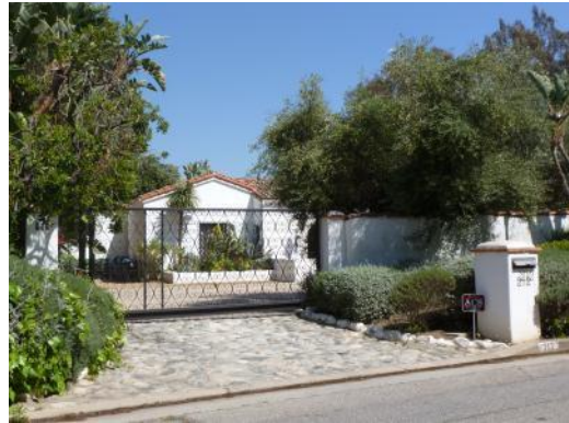
Address: 212 N. Copa de Oro Road Architect: Wallace Neff Date: 1928
