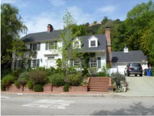
Address: 913 N. Chantilly Road Architect: Carroll Clark Date: 1948
