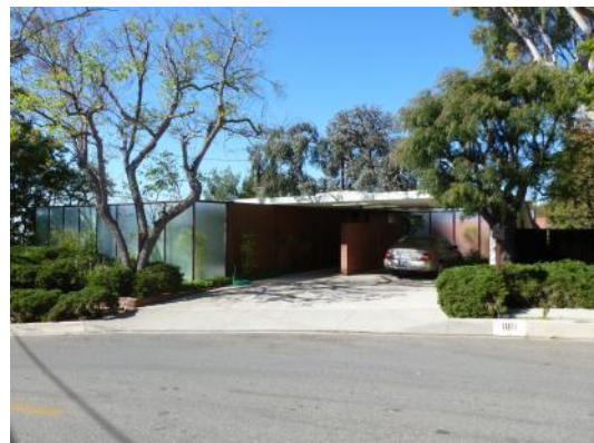
Address: 1811 Bel Air Road Architect: Richard Dorman Date: 1953
