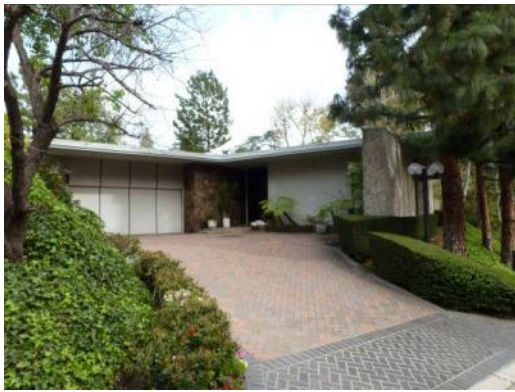
Address: 1044 N. Angelo Drive Architect: Maynard Houston Date: 1960
