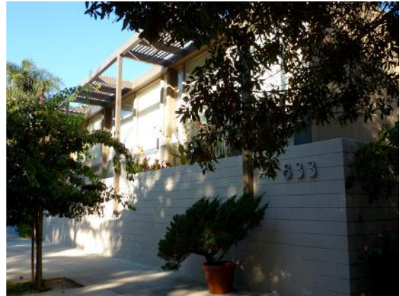
Address: 833 Moraga Drive Name: Moraga Drive Garden Apartment Date: 1963
