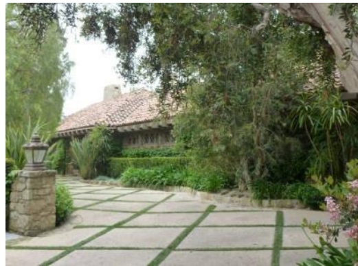
Address: 423 N. Faring Road Architect: Roland Coate Date: 1932
