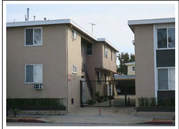
South façade, view northeast (ARG, 2019)
