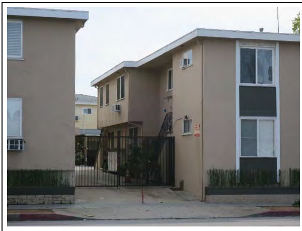
North façade, view southeast (ARG, 2019)
