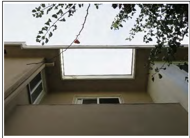
Detail of pierced eave (ARG, 2019)
