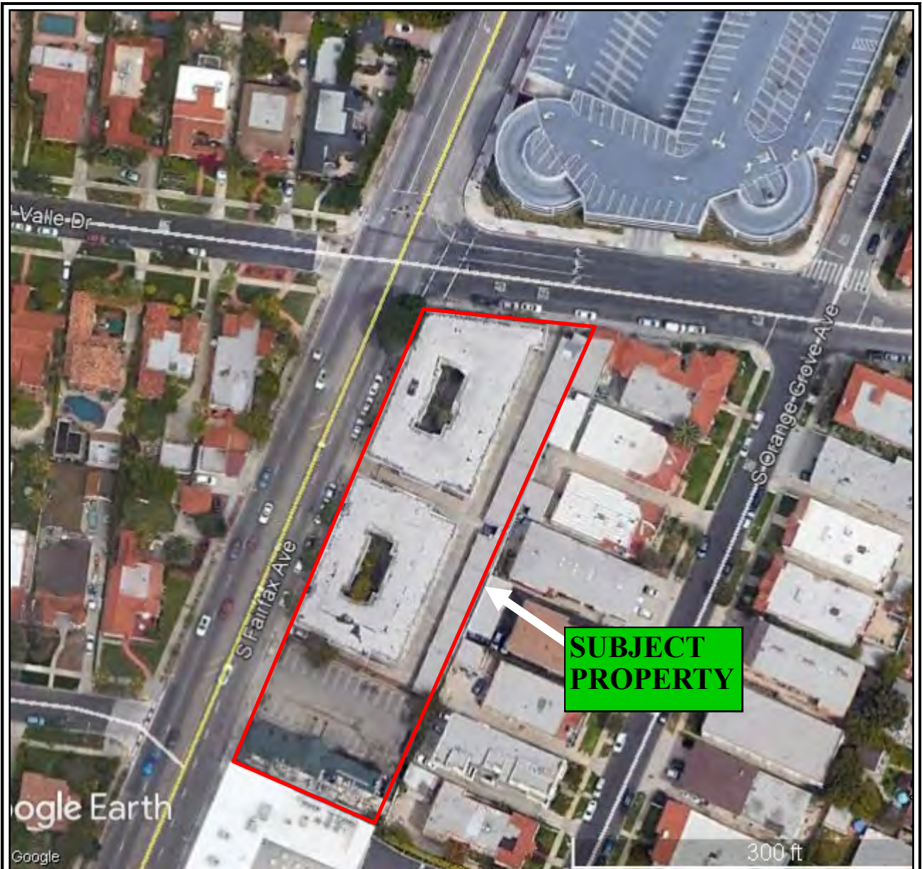
FIGURE 2 SITE LOCATION Subject Property 830 - 840 South Fairfax Avenue Los Angeles, CA
