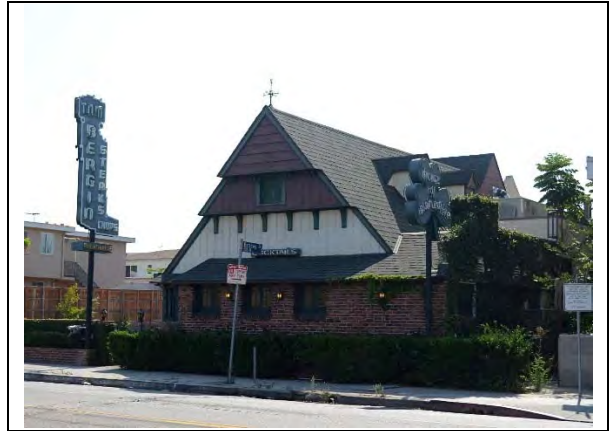
West façade, view northeast (ARG, 2018)
