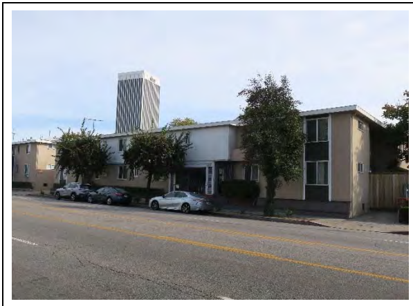
West façade, view northeast (ARG, 2019)
