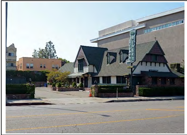
West façade, view southeast (ARG, 2019)
