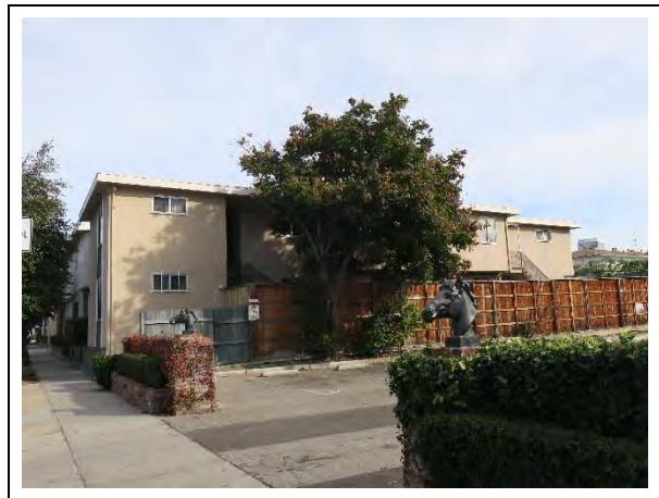
South façade, view northeast (ARG, 2019)
