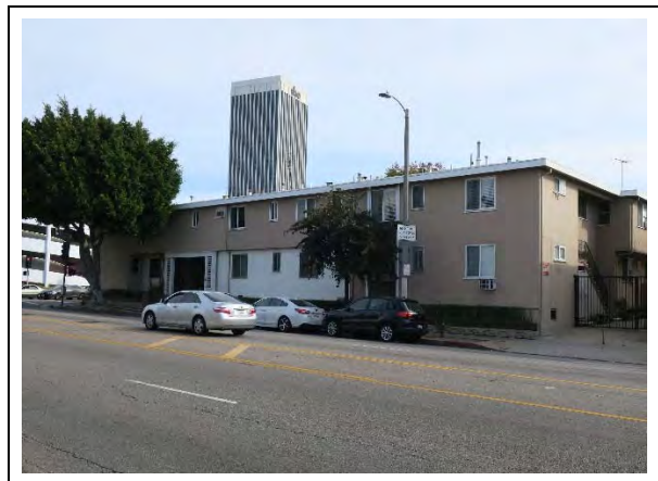
West façade, view northeast (ARG, 2019)
