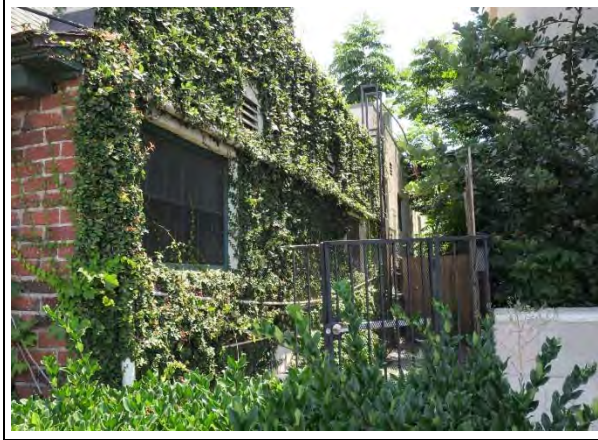
South façade, view northeast (ARG, 2018)
