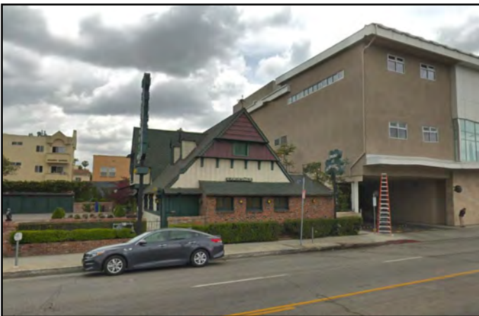
Photo 21. Subject property at 840 Fairfax to the and the adjacent school to the southwest is to the right.
