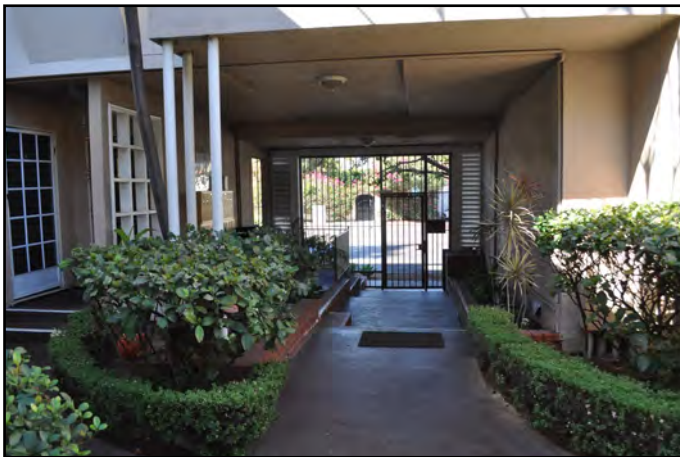
Photo 17. Southern building entrance.
