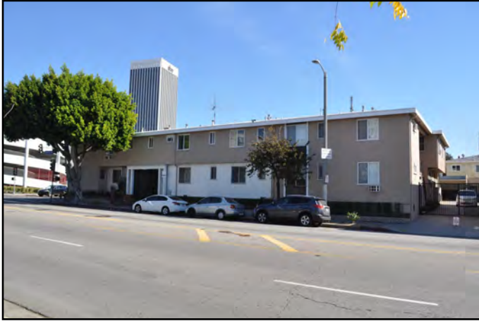
Photo 4. The northern building.
