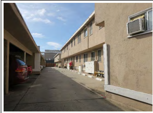
East façade, view southwest. Note detached carport structure at left (ARG, 2019)
