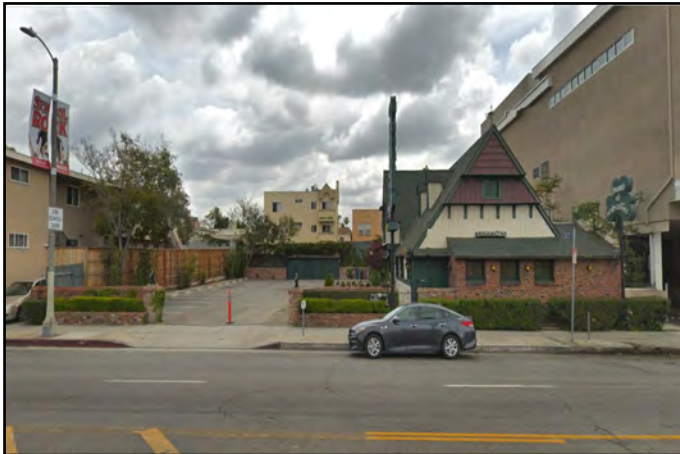
Photo 20. The former restaurant at 840 Fairfax .
