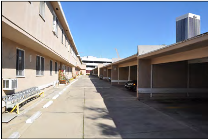
Photo 19. The rear of the property looking north.
