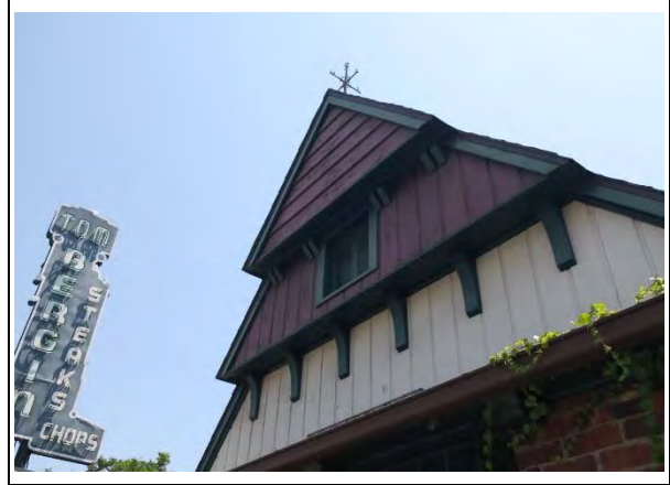
Detail of jettied gable and decorative brackets on west façade (ARG, 2018)
