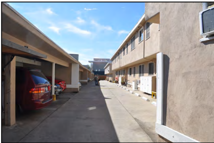
Photo 12. Looking south along the driveway with the apartments to the right and the rear carports to the left.
