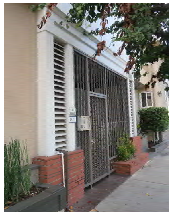
West façade, detail of breezeway entrance, view southeast (ARG, 2019)
