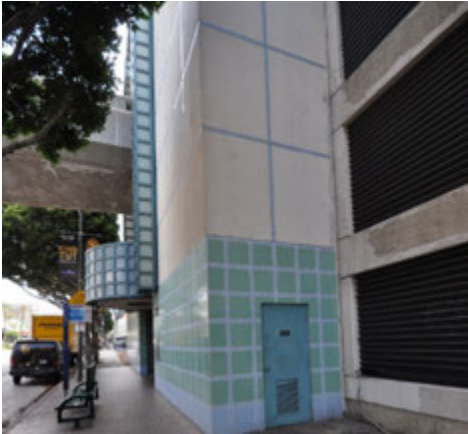
Figure 13: Northwest elevation entrance, view looking northeast (GPA, 2018).
