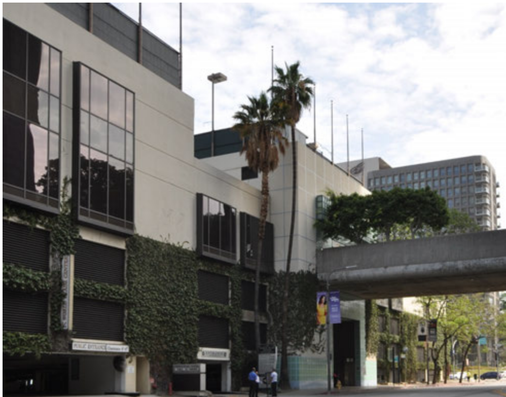
Figure 10: Detail view of southeast elevation, view looking north (GPA, 2018).
