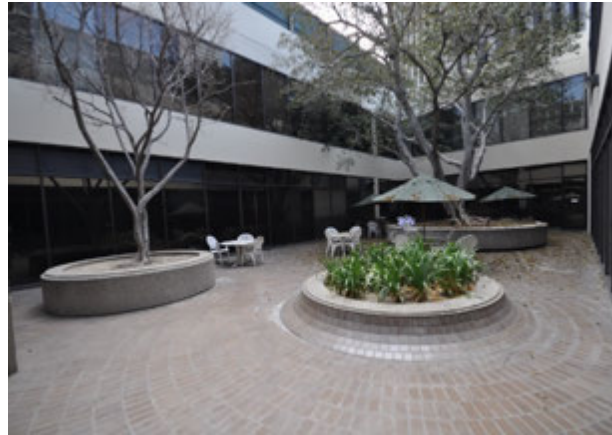
Figure 22: Courtyard between building wings (GPA, 2018).
