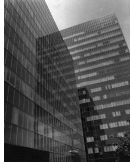
Figure 24: Century City Medical Plaza, Cesar Pelli and Anthony Lumsden for DMJM, 1966-1969, 1972. Source: "Late Modernism, 1965-1986" by Daniel Paul, 2008.
