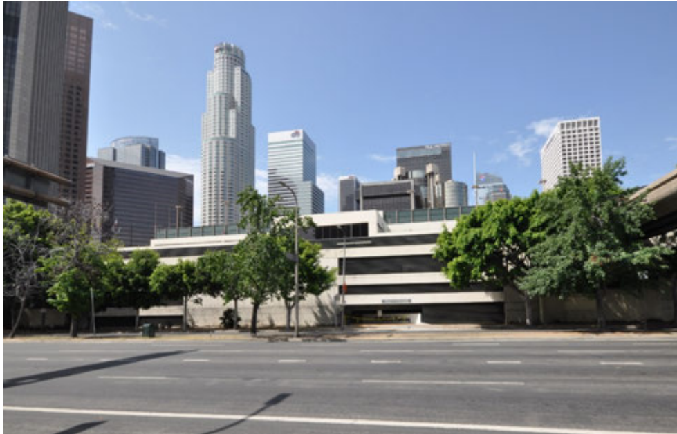
Figure 7: Northeast elevation, view looking south (GPA, 2018).
