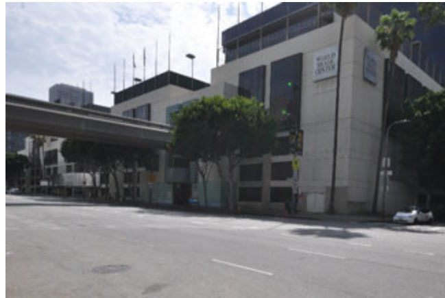
Figure 6: Northwest elevation, view looking southeast (GPA, 2018).
