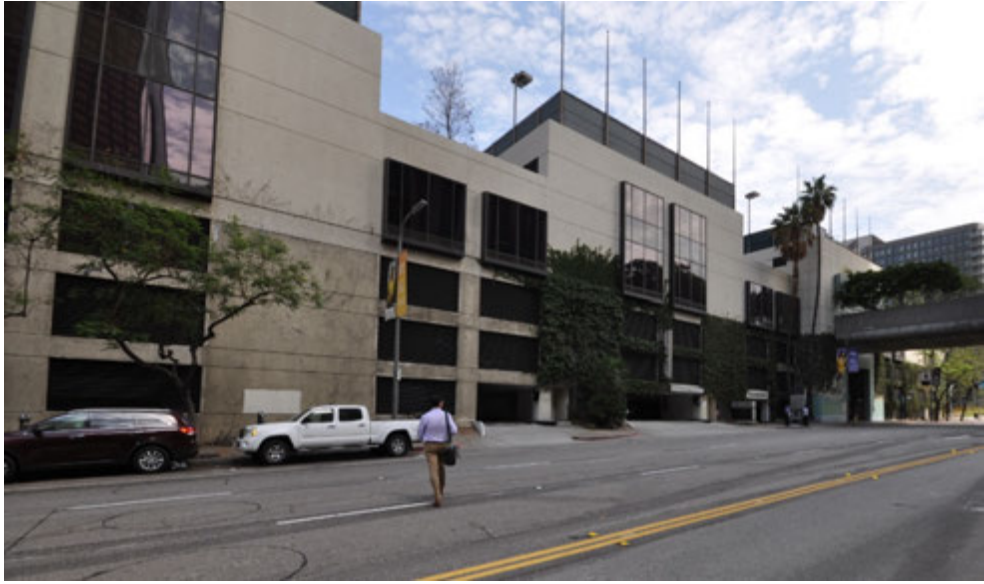
Figure 9: Southeast elevation, view looking northwest (GPA, 2018).
