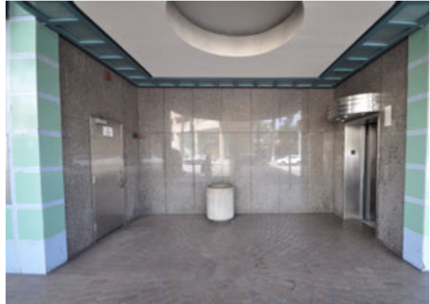
Figure 14: Detail view, ground floor elevator (GPA, 2018).
