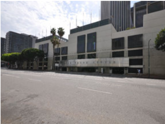
Figure 5: Northeast elevation, view looking east (GPA, 2018).
