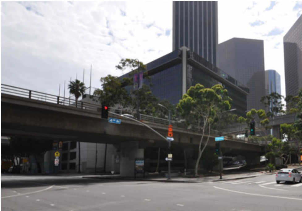
Figure 12: Southwest elevation, view looking east (GPA, 2018).
