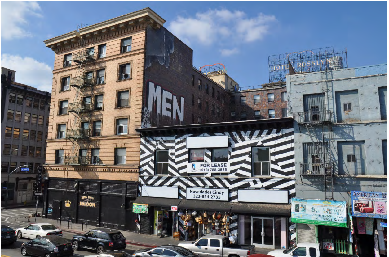
King Edward Hotel East elevation and north elevation Photo taken: December 17, 2018
