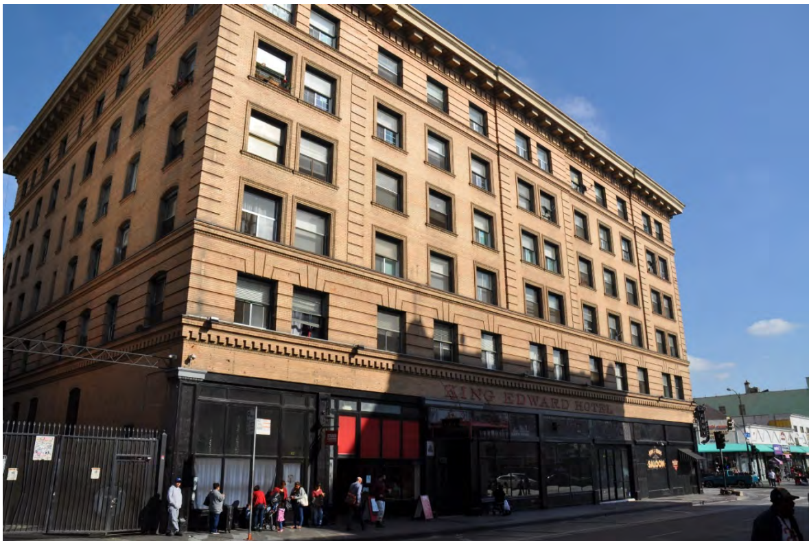
King Edward Hotel South elevation and partial west elevation Photograph taken: December 17, 2018
