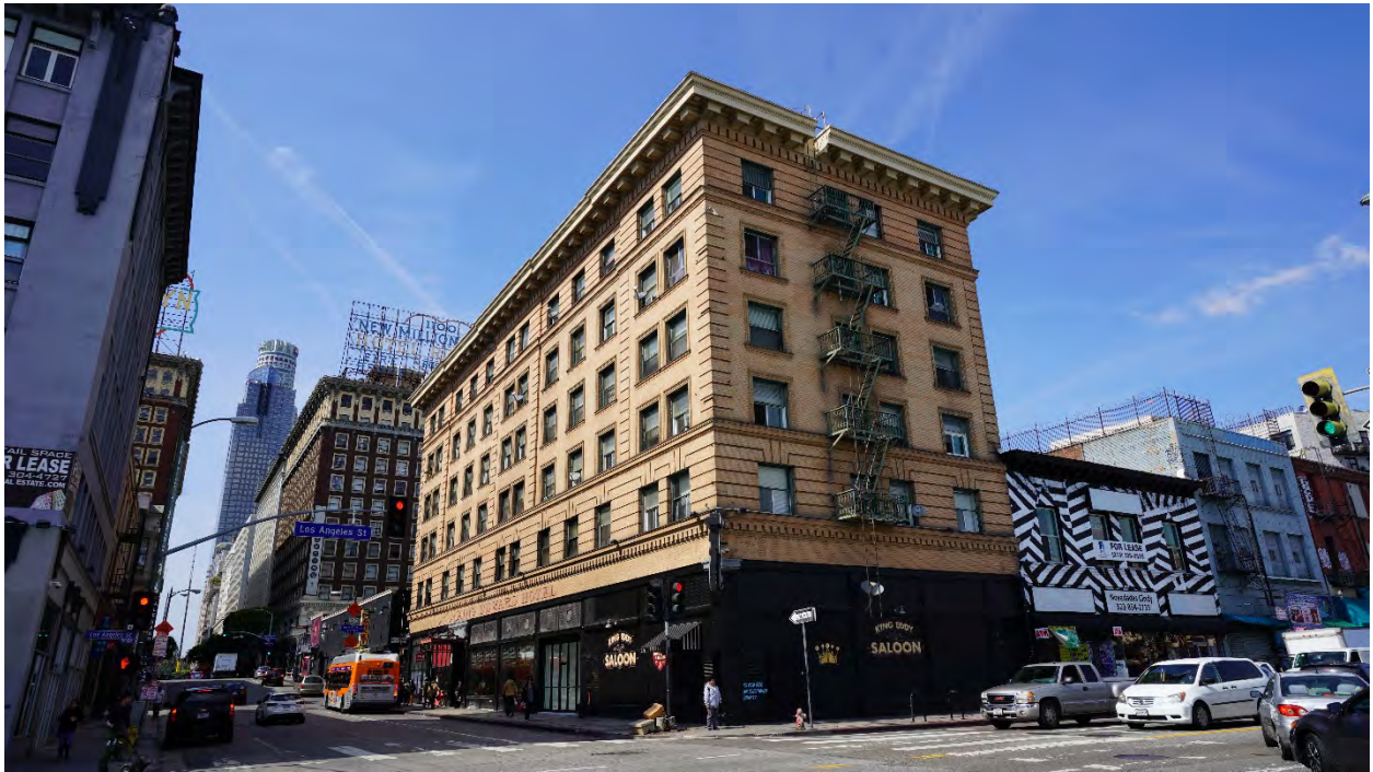
King Edward Hotel South elevation and east elevation Photograph taken: March 29, 2019
