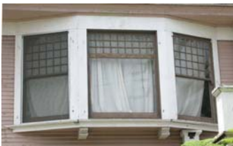
A window bay with decorative multi-light windows is shown.
