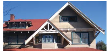
The original windows on this house contribute to its historic integrity.
