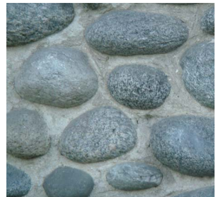
Wood clapboard, concrete and stone are all historically appropriate materials. When replaced, care should be taken to replicate texture, arrangement and dimension.
