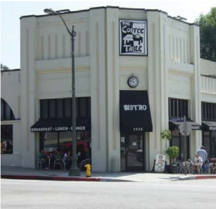
This plaster facade provides vertical ridges.
