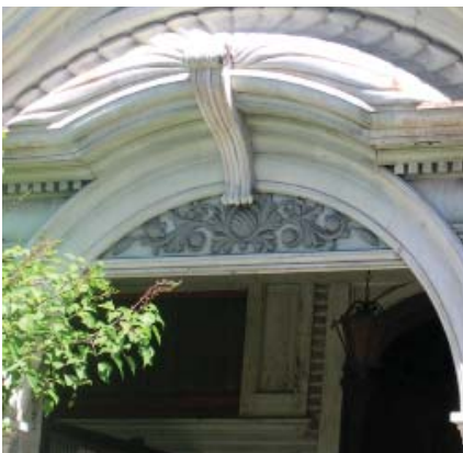
The intricate woodwork on this house requires careful maintenance.
