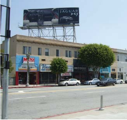
Storefront improvements should be consistent with the overall building facade. This building has been chopped into irreconcilable pieces.
