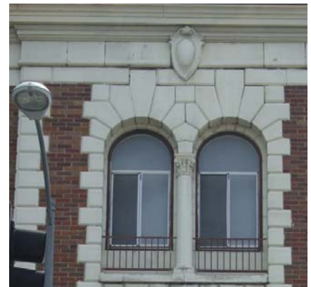
Pilasters, quoins and lentils are used on this building facade.
