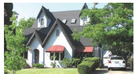
This second-story addition, with its noticeable dormers, calls attention to itself, overwhelming the original cottage.
