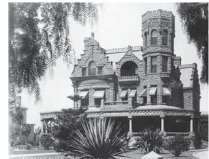
Prominent developer and subdivider, George W. Stimson’s own home just blocks from the Adams-Normandie neighborhood. The Romanesque mansion was built in 1891.
