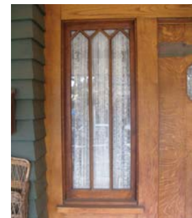
Side lights are the windows that flank one or both sides of a door and are found on many historic doors
