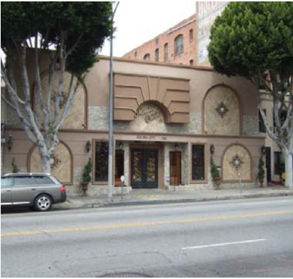
Pre-cast concrete, foam plant-ons and other similar materials are inappropriate on historic buildings.
