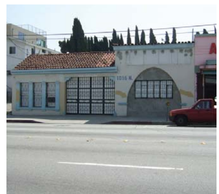
Concrete block is not a material that is original to this Spanish Colonial building.
