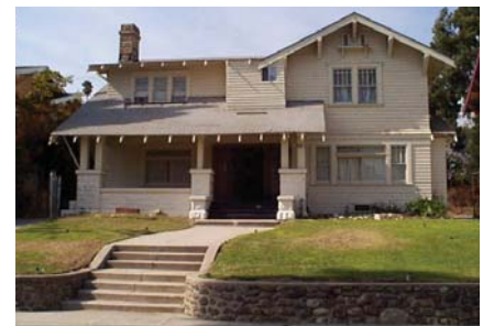
Historic retaining walls often comprised of stone, are an important part of the neighborhood setting.
