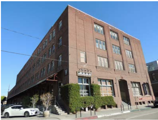
Address: 924 E 2 nd Street Name: Pacific Commercial Warehouse Date: 1910
