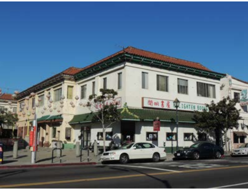
Location: Greater Chinatown Description: Chung King Court Date: 1947
