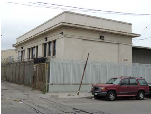
Address: 2417 E Porter Street Name: Edison Electrical Substation Date: 1911
