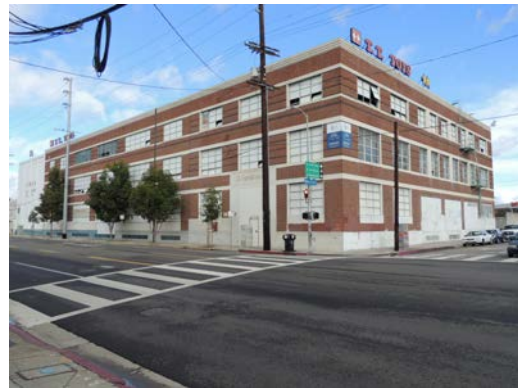
Address: 947 E 4 th Street Name: Coca-Cola Syrup Manufacturing Plant Date: 1915; remodeled 1939
