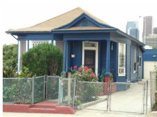
Address: 920 W New Depot Street Date: 1899
