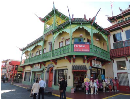
Description: 949 N Sun Mun Way Date: 1940
