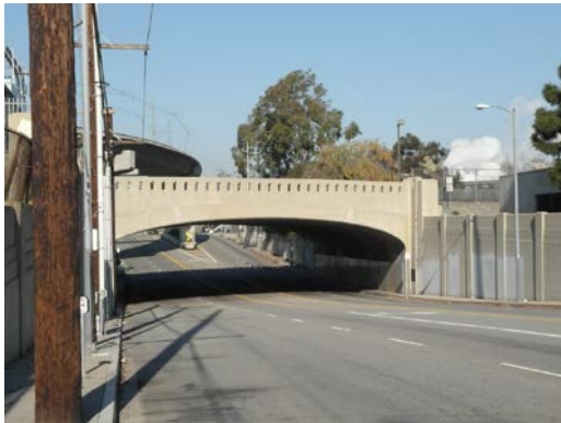
Location: Vignes Street near Bauchet Street Name: Vignes Street Grade Separation Date: 1938
