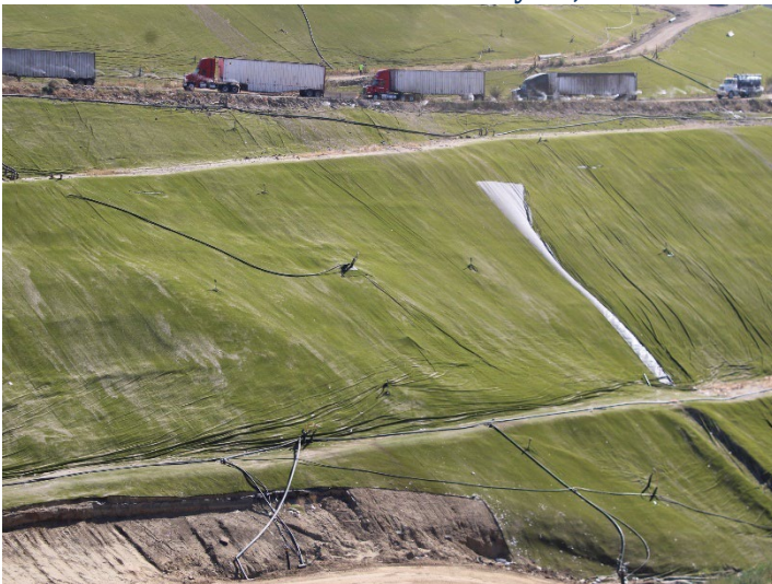
Photo 103: Closure Turf: June 18, 2025
