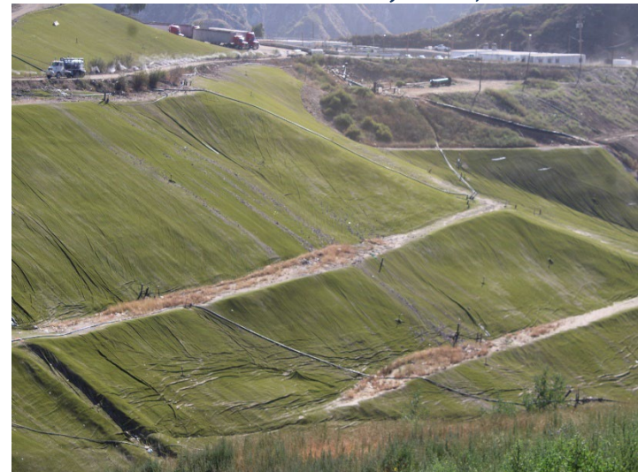
Photo 104: Closure Turf: June 18, 2025
