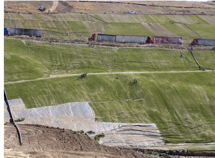
Photo 102: Closure Turf: June 18, 2025
