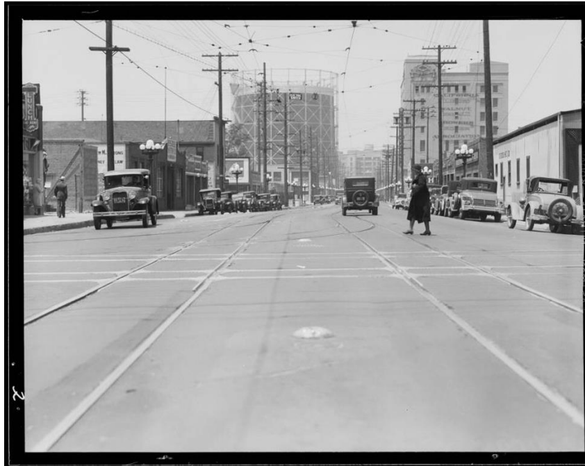
Figure 14. View of 7th Street at Mateo Street, facing west toward Alameda Street, 1933. (Source: USC Libraries Special Collections, Dick Whittington Studio, File DW-1933-05-27-153, Image 2)
