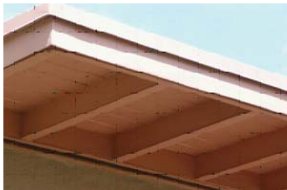
Detail of exposed eave rafters on Beethoven Street.
