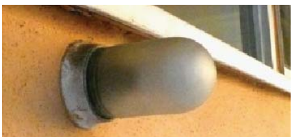
Door detail: Original entrance light.
