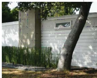
Chimney configuration facing street.
