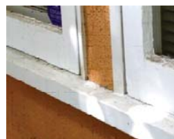
Detail of closed ¾ height windows.
