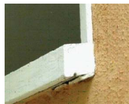
Detail of clerestory window sill.
