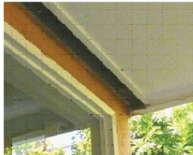
Detail off entrance side roof vents.
