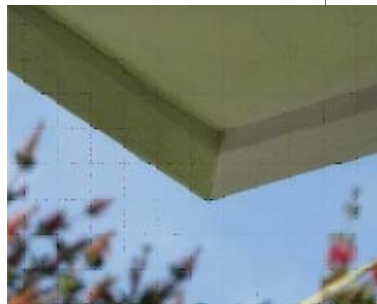
Detail of mitered fascia and beveled drip edge.
