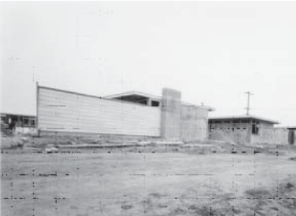
1948 Construction under way on Beethoven Street.
