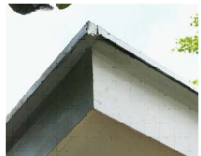
Detail of 1"x1" roof flashing spacing shim.
