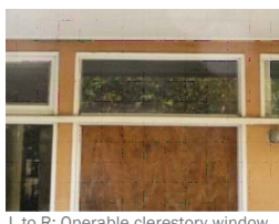
L to R: Operable clerestory window with screen, door transom, and fixed clerestory window .
