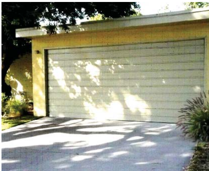
Typical street-facing garage configuration.
