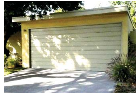
Typical street-facing garage configuration.
