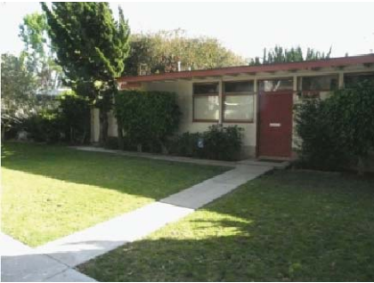
Architectural detail: Front entrance and side entrance concrete walkways.
