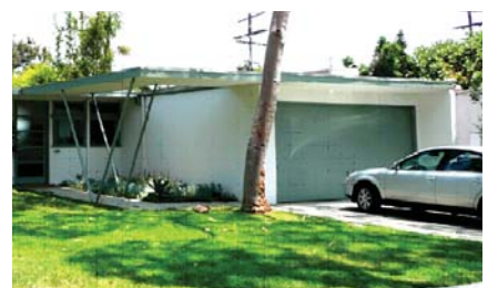
Original garage configuration with sidewall, eave, and “V”-supported canopy.
