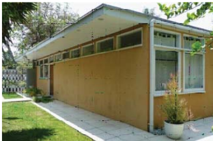
On perpendicular homes, two bedroom windows were placed on the side wall facing the rear to allow privacy between side neighbors. Extra clerestory windows make up for the missing third bedroom window.
