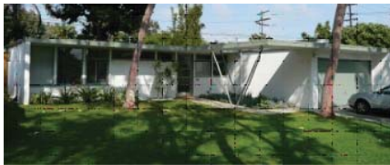
Side walls on homes parallel to the street were left blank with no windows to allow for privacy between neighbors. Notice the extended side privacy wall next to the bedroom windows.
