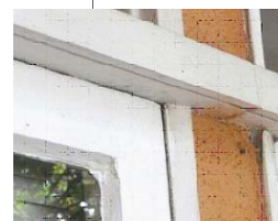
Detail of operable ¾ height windows and clerestory window sill.
