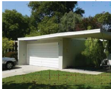
Flat roof extending into entrance walkway canopy.
