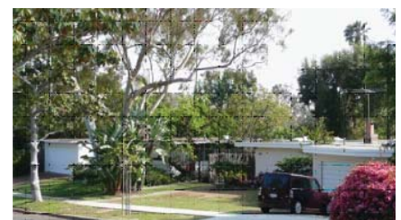
A second-story addition on a single story Mid-Century Modern home in a district comprised of similarly sized single-story Mid-Century Modern homes would be inappropriate
