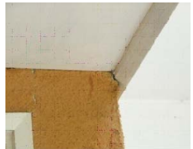
The fascia's beveled drip edge leads any rain water away from the stucco wall.
