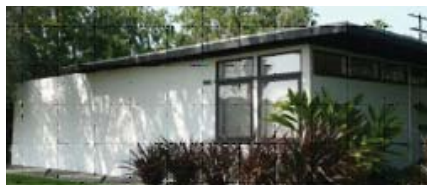
Perpendicularly situated home with double bedroom windows on short wall towards the street. Notice the extended privacy wall left.
