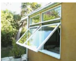
Operable ¾ height windows open outwards and rely on a friction hinge.
