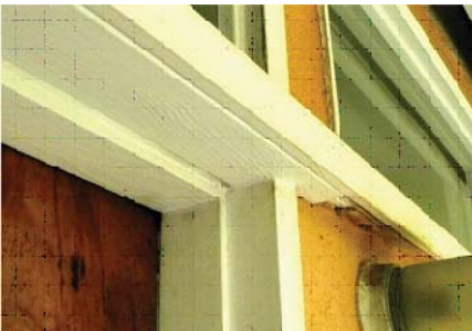
Detail of entrance frame and transom sill.
