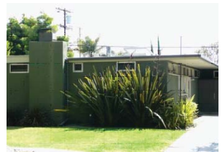
Careful placement of ducting and AC-unit made this installation invisible from the street.
