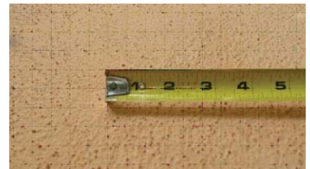
Close-up of appropriate stucco finish.
