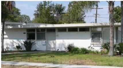
On some homes two of the clerestory windows were omitted to allow for kitchen cabinet storage space up to ceiling height.
