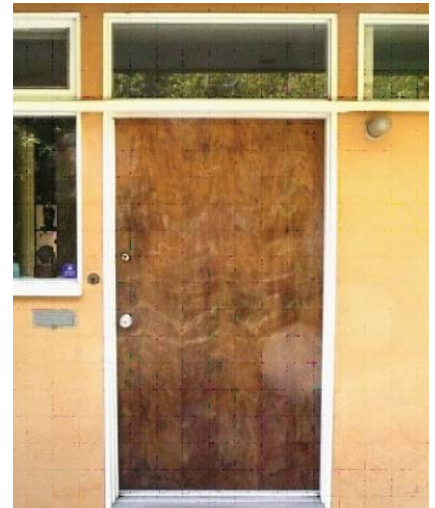
Original entrance door with transom/ clerestory window.
