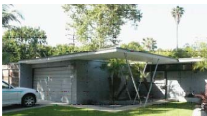
Original zigzag concrete walkway with canopy from garage to entrance.
