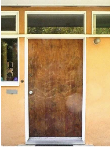
Original veneered entrance door with transom, doorknob, lock, light fixture, door bell and pot metal mail drop.
