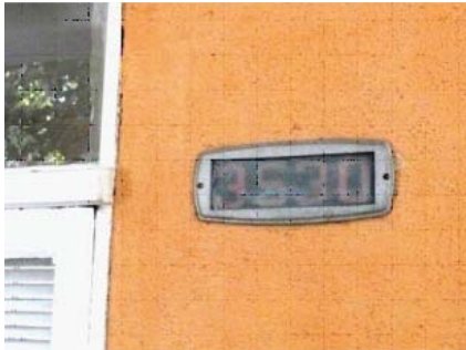
Architectural detail: Illuminated street numbers in "aluminum" pot metal frame.
