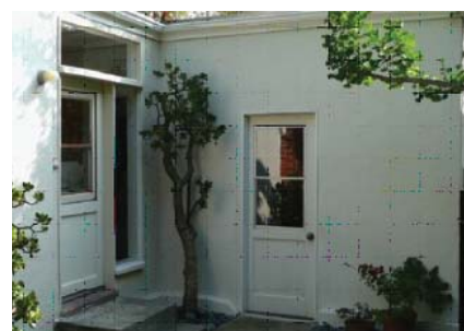
Original kitchen entrance door/window (left) and rear garage entrance (right).
