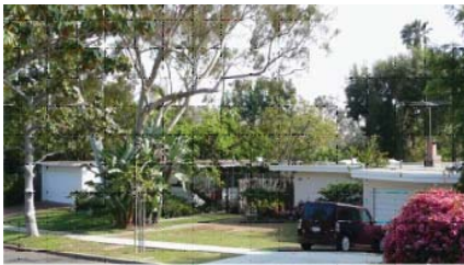
Solar panels should not be placed upon rooftops that are visible to the general public.
