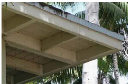
Detail of exposed eave rafters on Moore Street west side.
