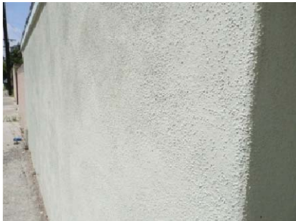
Mar Vista tract stucco finish
