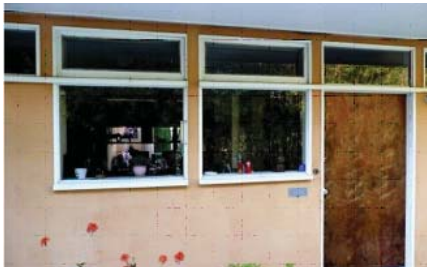
Entrance door and left-side kitchen window configuration.
