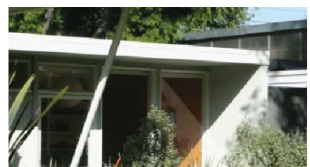
Architectural detail: Front bedroom privacy wall.
