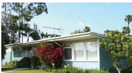
Mar Vista Tract materials and finishes: Stucco wall finish, wood trim and windows, stucco and wood panel privacy walls and fences.
