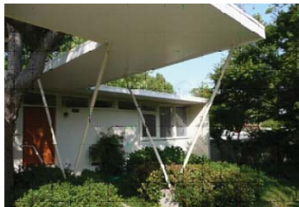
"V"-shaped support stands for the walkway canopy – an important architectural detail.
