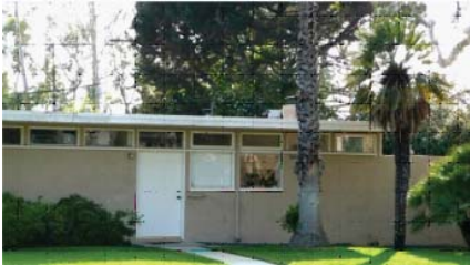
Landscape screening and the use of paint colors to match the surrounding environment should be used if an installation must be placed in public view.
