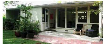
Homes parallel to the street have master bedroom windows facing side privacy walls on each side, and a blank rear wall. The living room window configuration features two ¾ height windows, two full-size floor-to-ceiling windows and a glazed door.
