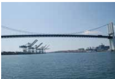
Vincent Thomas Bridge
