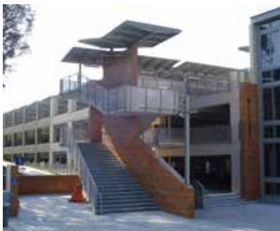
Solar panels on top of parking structure
