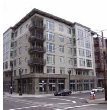
Architectural features on all street frontages
