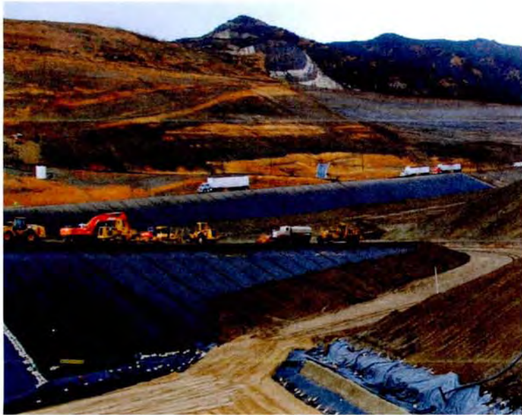
Photo 3: Operation layer over geosynthetics in Cell CC3a Part 1
