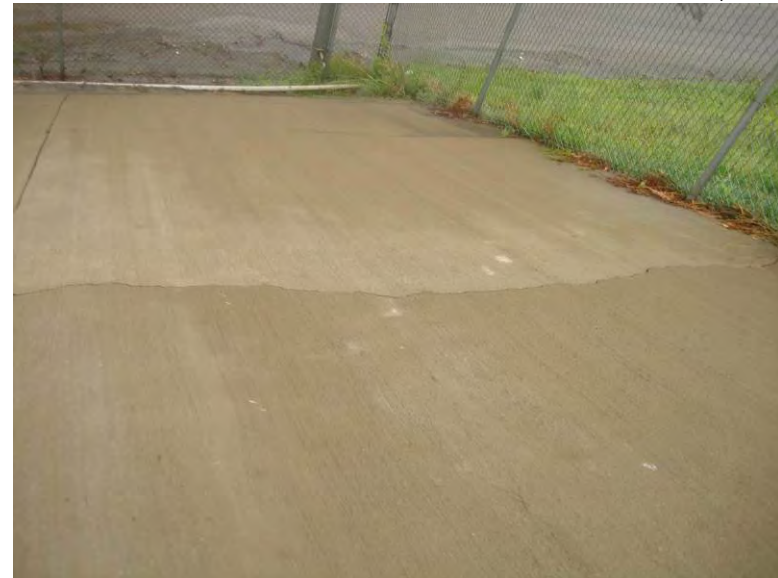
Photo 220: Terminal Basin Exterior Wall Crack: October 9, 2013
