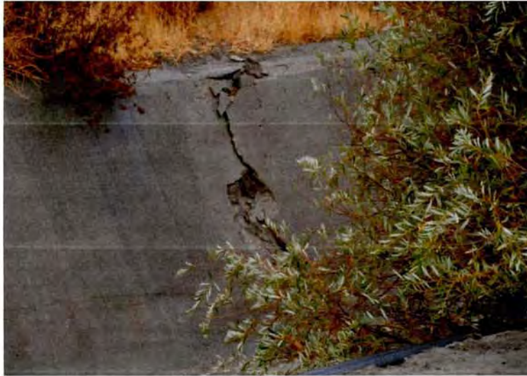
Photo 1: North channel – crack in concrete wall
