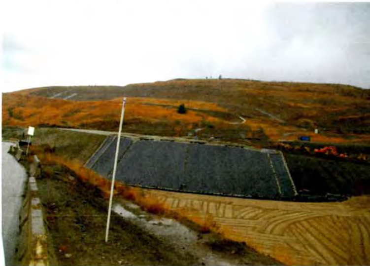
Photo 2: Stability berm in place at Cell CC3a Part 1
