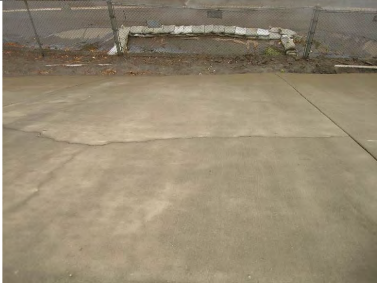
Photo 217: Terminal Basin Exterior Wall Crack: October 9, 2013
