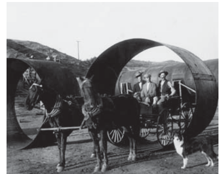
Construction of the Owens Valley Aqueduct. A horse-drawn carriage poses in one of the large pipes used in the construction of the aqueduct.
