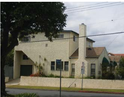
The use of highly textured stucco along with inappropriate window replacement both detract from the look of this structure.
