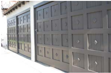
Historic garage doors often included decorative panels and either slid along tracks or swung open. New doors should replicate this look.
