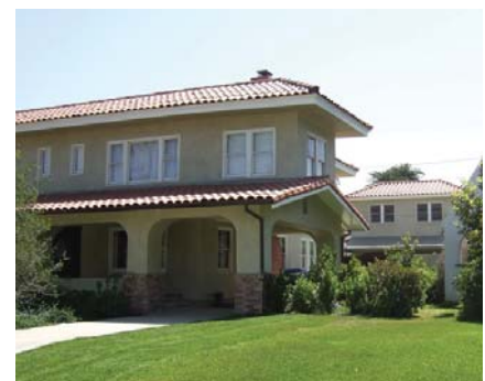
This in-fill accessory structure is diminutive to its primary structure.”
