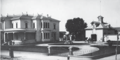
Exterior corner view of the three-story (formerly two-story) home and carriage house of Isaac Newton Van Nuys, located at Spring and 7th Street.
