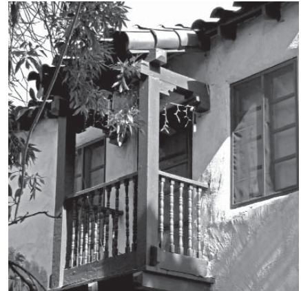
Small balconies with rustic wood spindlework are common on Spanish Colonial Revival houses.
