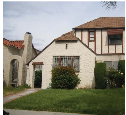
The use of highly textured stucco is a modern look and inappropriate on an historic home. Adding faux historic features, such as the timbering and stone on this front facade, is inappropriate.
