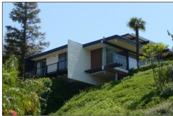
Address: 18918 La Montana Pl. Architect: Dion Neutra Date: 1972
