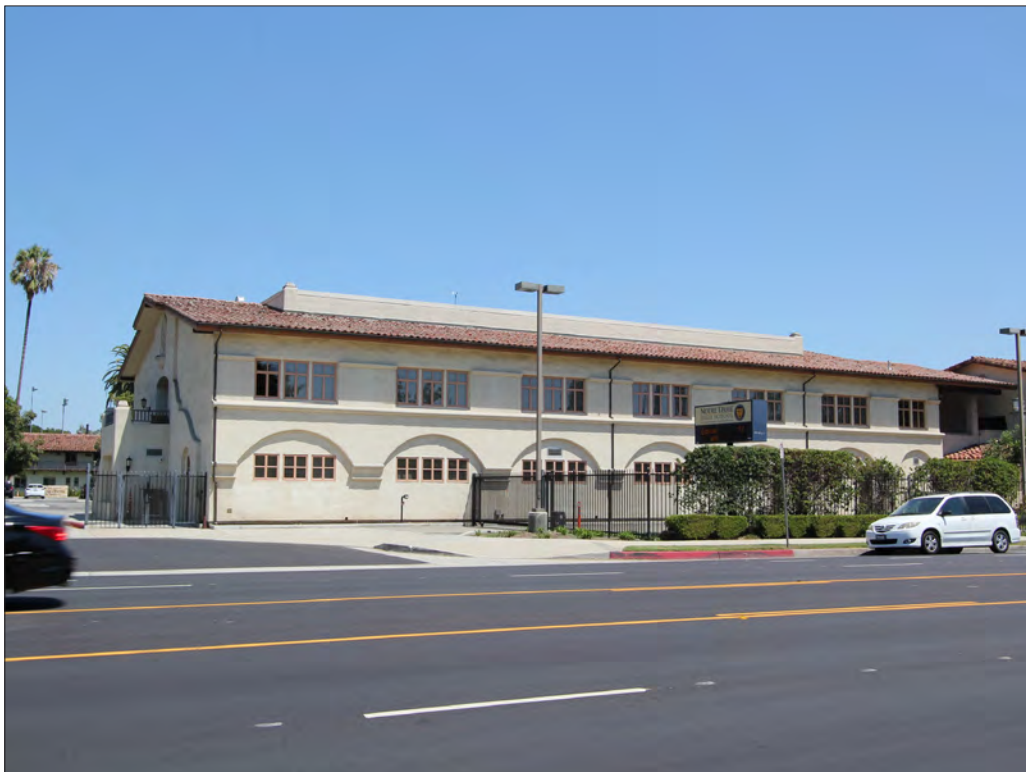
Image 114: Hampton Building, west elevation elevation, view east (Chattel, 2018)
