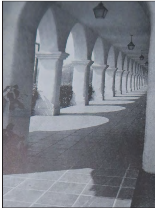
Image 8: Moreau Hall, south elevation arcade, view west (Notre Dame High School Yearbook, 1951)
