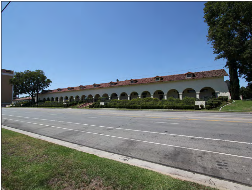
Image 34: Moreau Hall, south elevation, view northwest.(Chattel, 2017)
