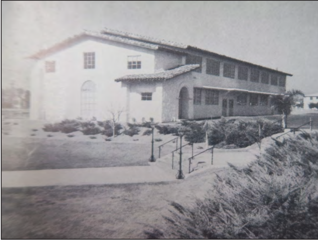
Image 30: St. Andre Bessette Hall, southeast corner, view northwest (Notre Dame High School Yearbook, 1956)
