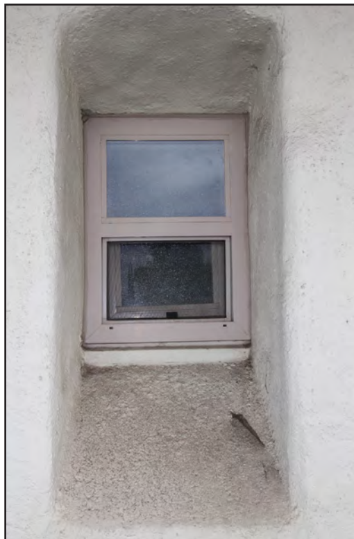
Image 60: Holy Cross Center, west elevation, view east, window detail (Chattel, 2018)
