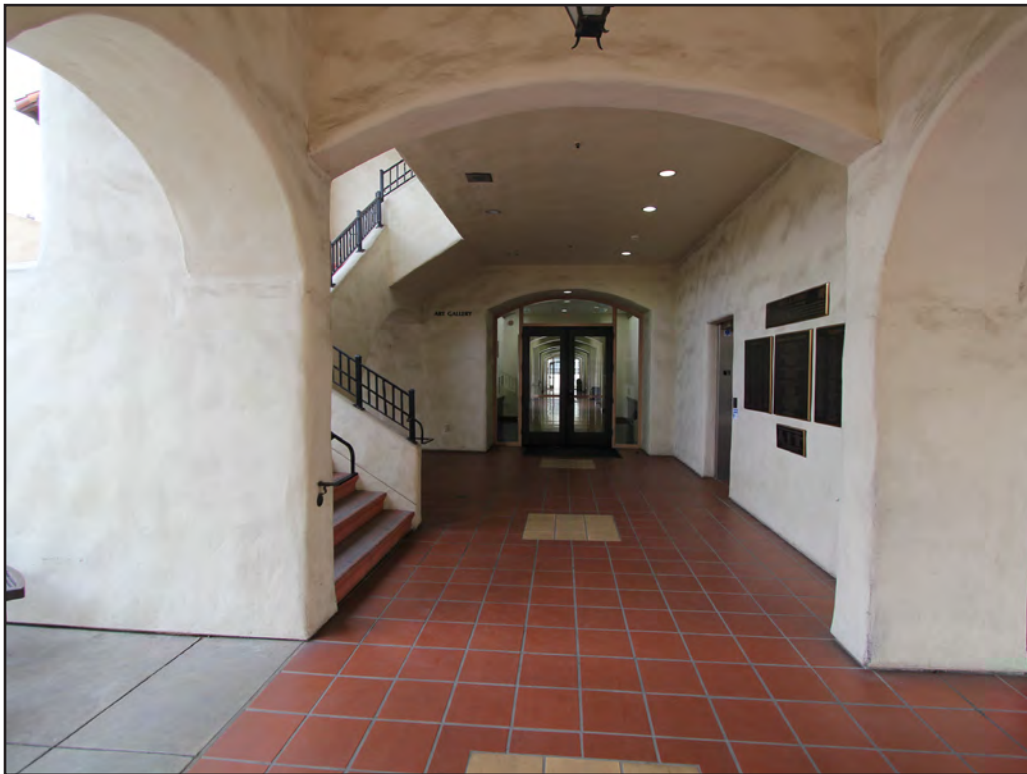
Image 106: Burns Arts & Technology Building, entrance from courtyard, view south (Chattel, 2018)
