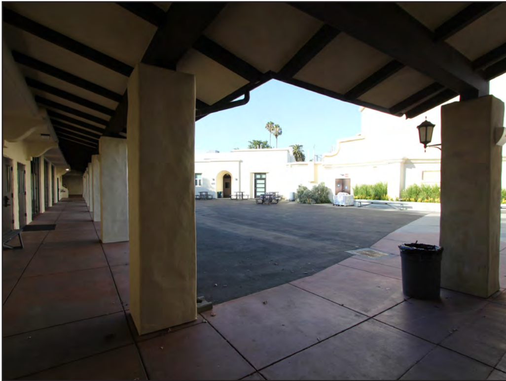
Image 87: St. Andre Bessette Hall, east elevation arcade, view northeast (Chattel,
