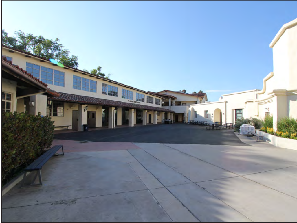
Image 81: St. Andre Bessette Hall, east elevation, view northwest (Chattel, 2018)
