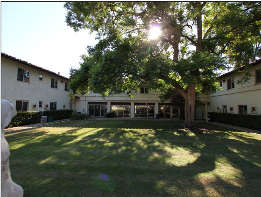
Image 64: Holy Cross Center, portion of east elevation, view west (Chattel, 2018)
