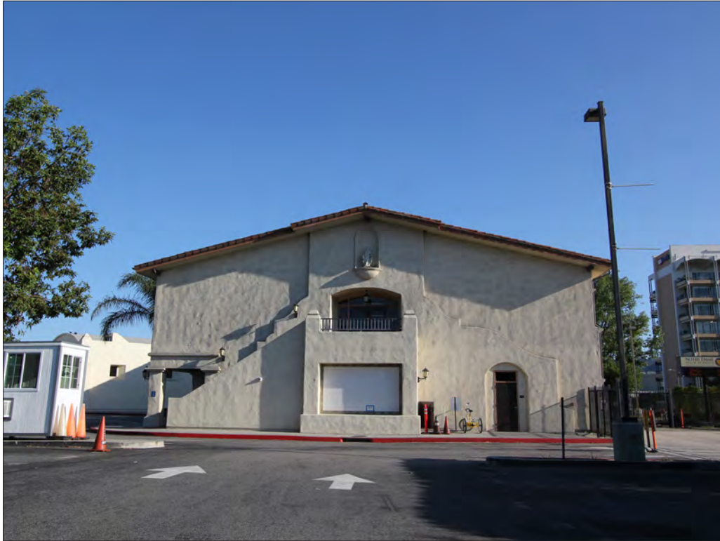
Image 113: Hampton Building, north elevation, view south (Chattel, 2018)
