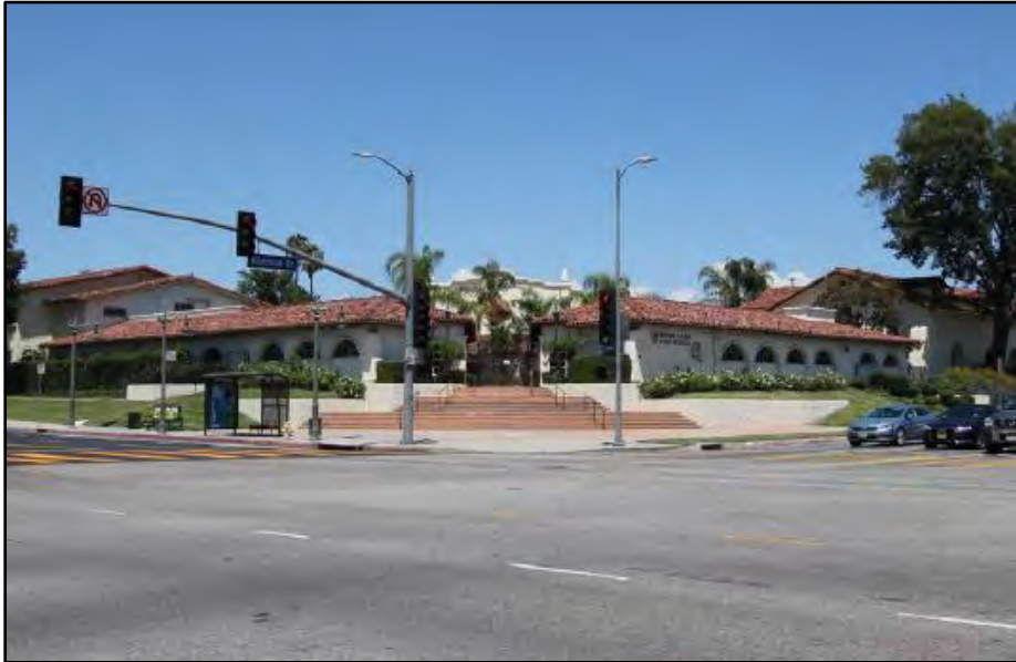
Figure 10. Allegratti Building, southwest corner, view northeast (Chattel, 2018)
