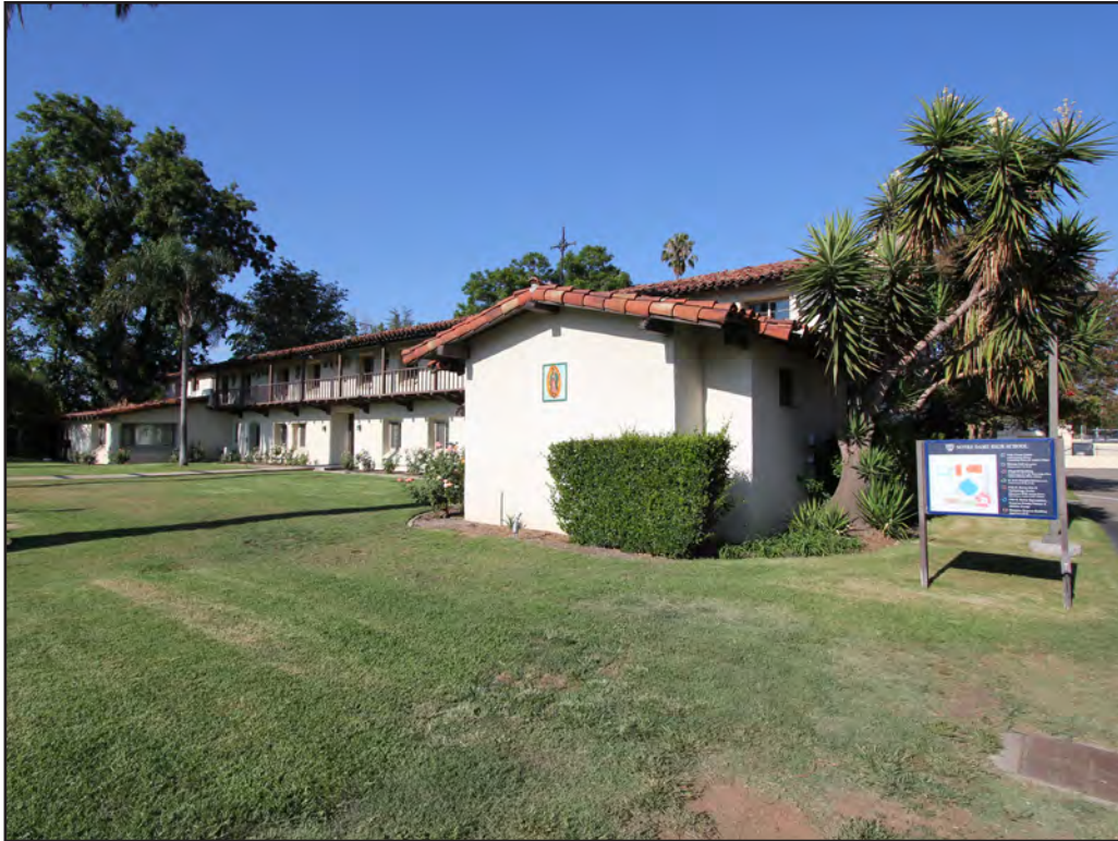
Image 58: Holy Cross Center, west elevation, view east (Chattel, 2017)
