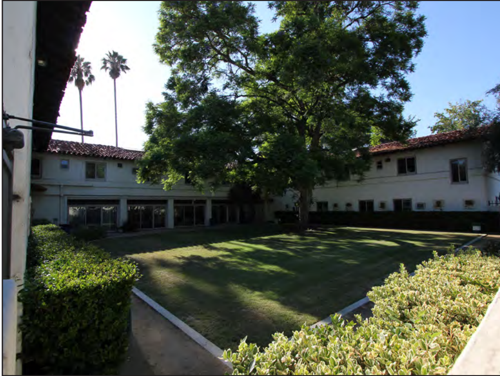
Image 65: Holy Cross Center, portion of east elevation, view northwest (Chattel, 2018)
