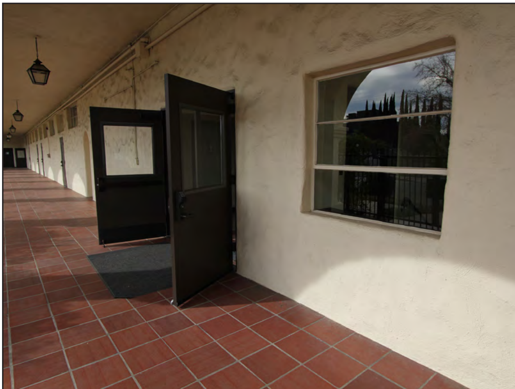
Image 39: Moreau Hall, south elevation, view west (Chattel, 2018)
