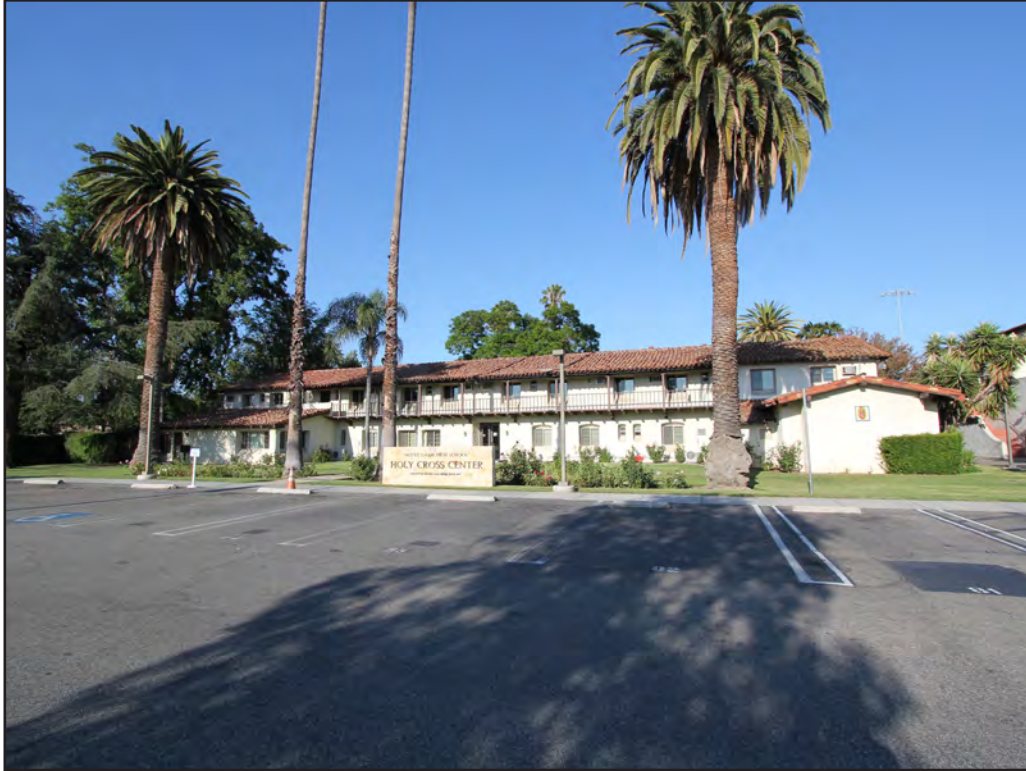
Image 53: Holy Cross Center, west elevation, view east (Chattel, 2017)
