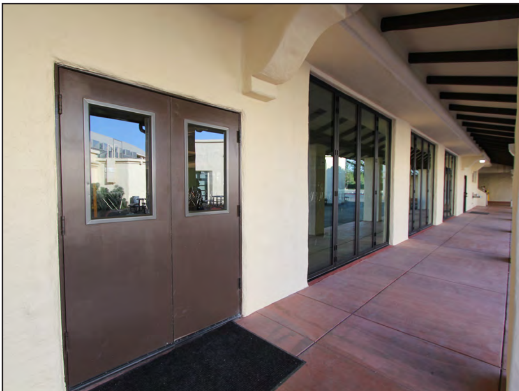
Image 88: St. Andre Bessette Hall, east elevation arcade, view northwest (Chattel, 2018)
