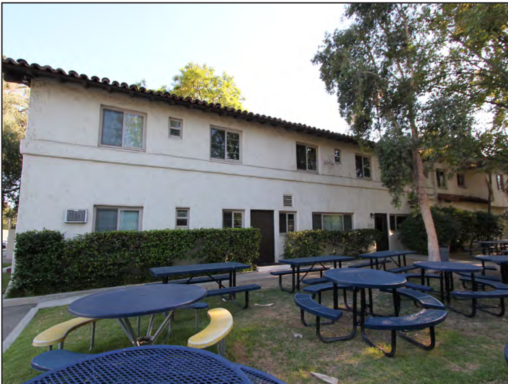
Image 67: Holy Cross Center, north elevation, view southwest (Chattel, 2018)
