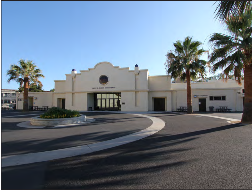
Image 72: Fritz B. Burns Gymnasium, north elevation, view southwest (Chattel, 2018)
