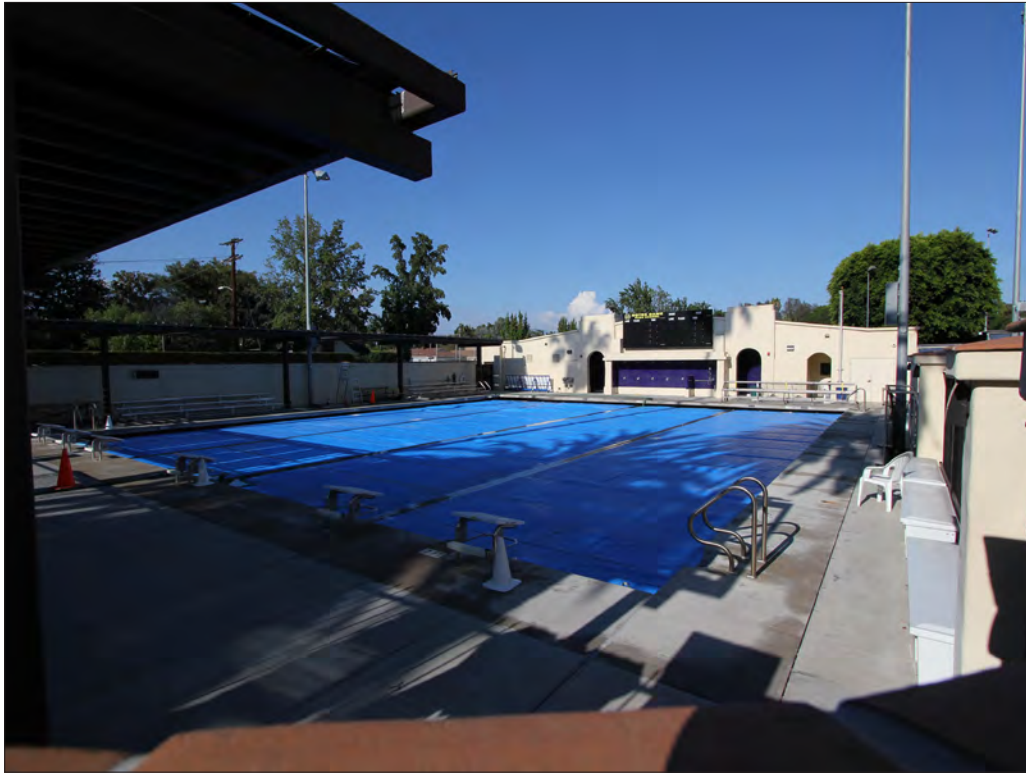
Image 119: Joseph E. Rawlinson Aquatic Center, view northeast (Chattel, 2018)
