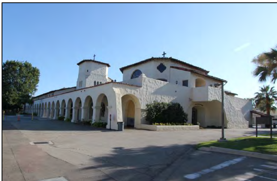
Figure 11. Burns Arts & Technology Building, northeast corner, view southwest (Chattel, 2018)
