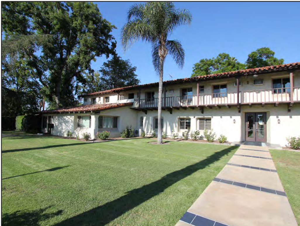
Image 54: Holy Cross Center, portion of west elevation, view northeast (Chattel, 2017)
