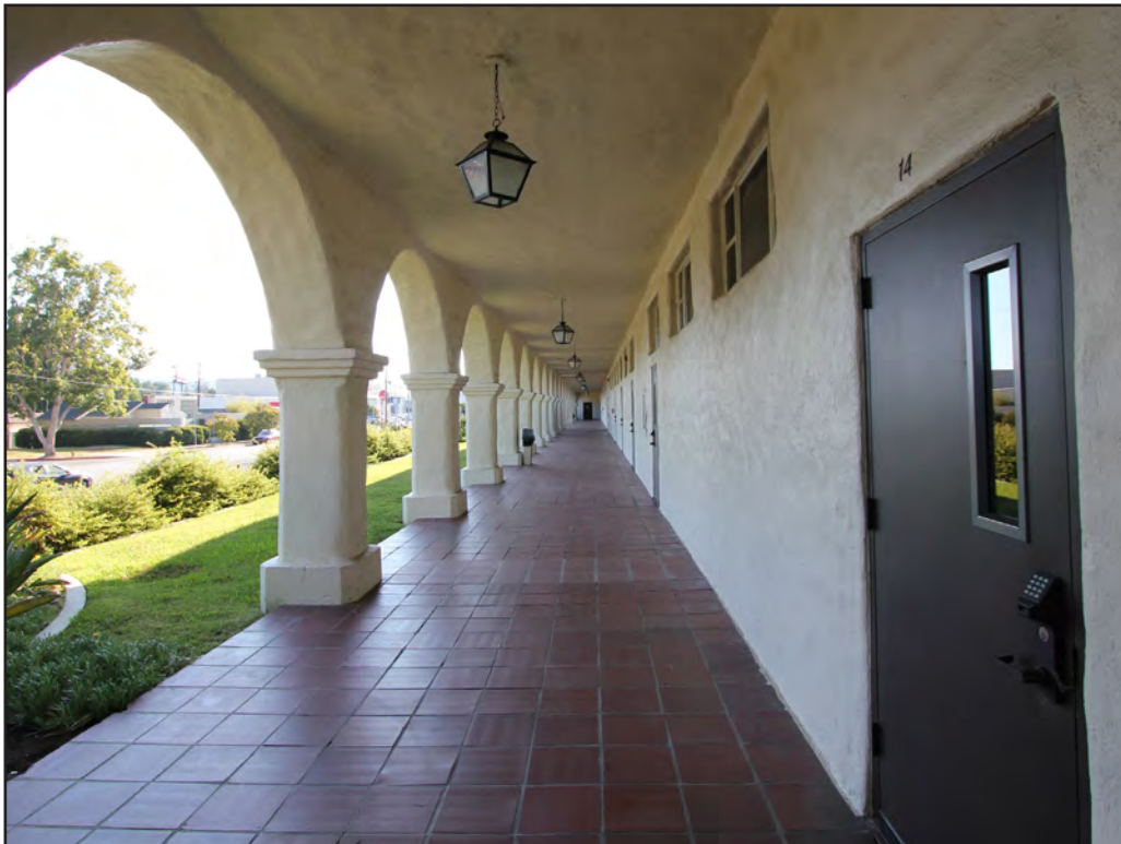
Image 38: Moreau Hall, south elevation arcade, view southwest (Chattel, 2017)
