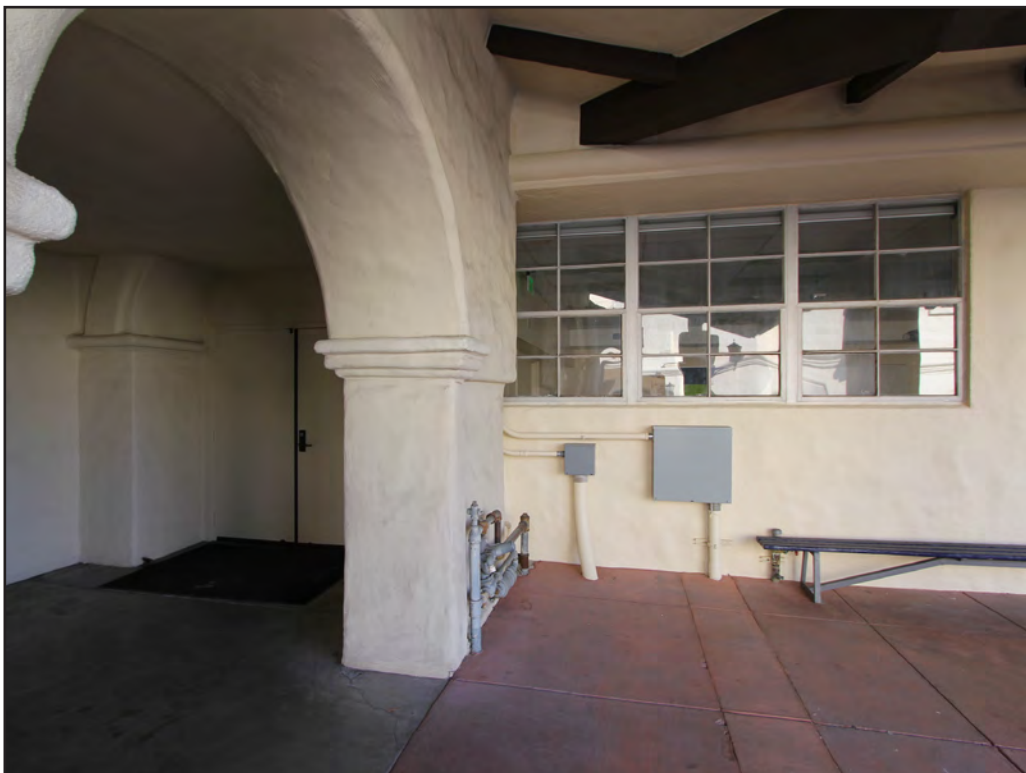
Image 84: St. Andre Bessette Hall, east elevation arcade, view west (Chattel, 2018)
