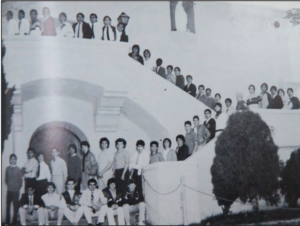
Image 16: Moreau Hall, east elevation, view west (Notre Dame High School Yearbook, 1983)
