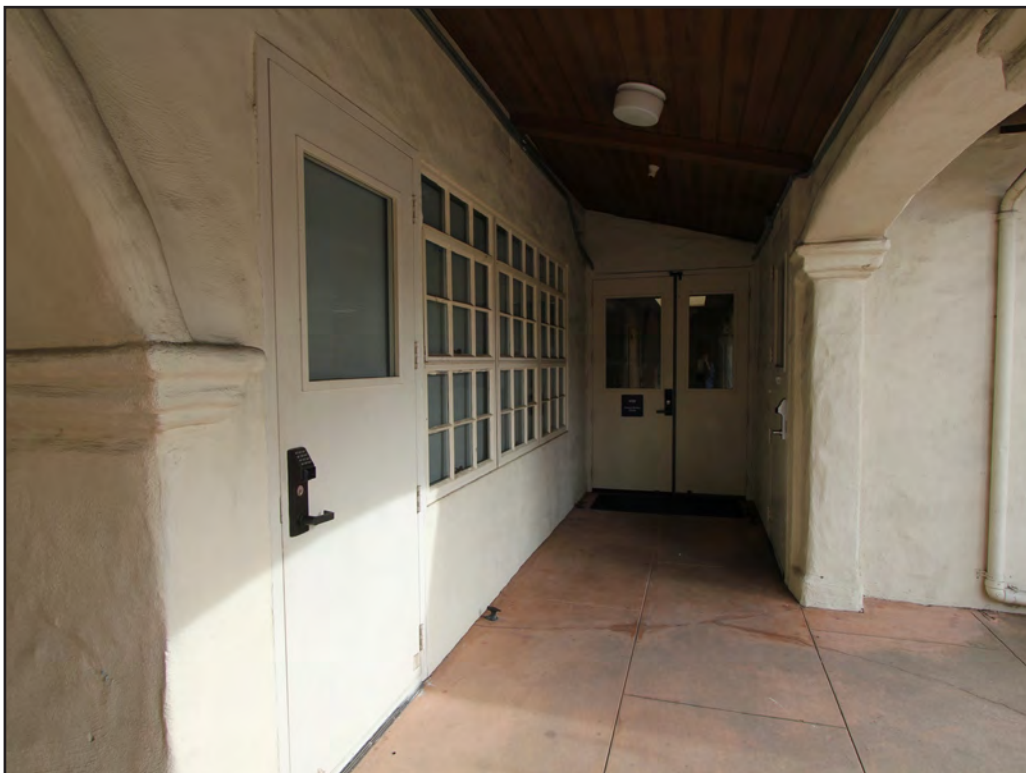
Image 86: St. Andre Bessette Hall, east elevation arcade, view west (Chattel, 2018)
