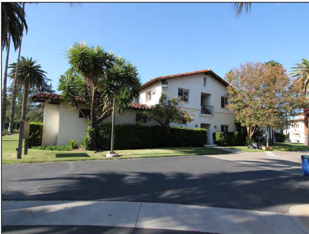
Image 57: Holy Cross Center, south elevation, view north (Chattel, 2017)
