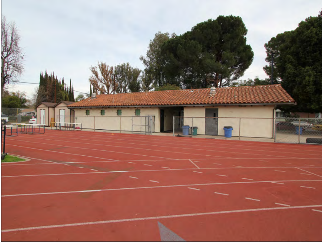
Image 121: Concession stands and restroom, west elevation, view northeast (Chattel, 2018)
