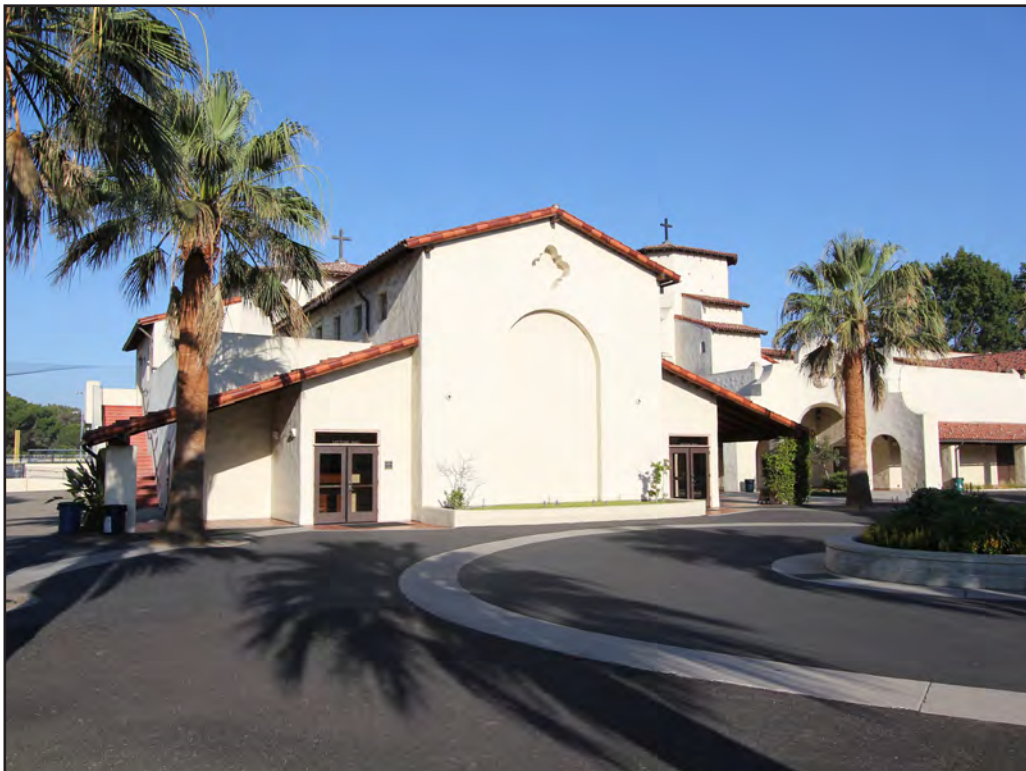
Image 100: Burns Arts & Technology Building, west elevation, view east (Chattel, 2018)
