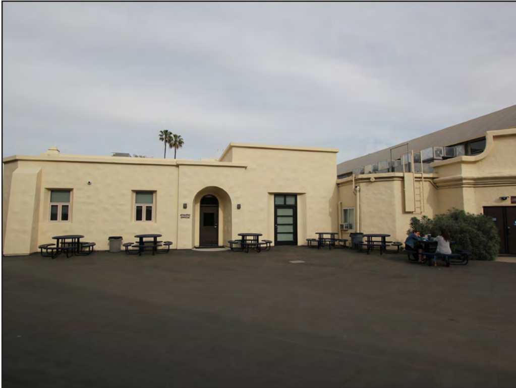
Image 76: Fritz B. Burns Gymnasium, Donahue Fitness Center, west elevation, view southeast (Chattel, 2018)
