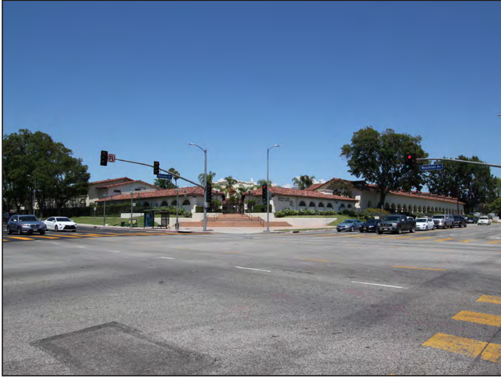
Image 91: Allegretti Building, southwest corner, view northeast (Chattel, 2018)
