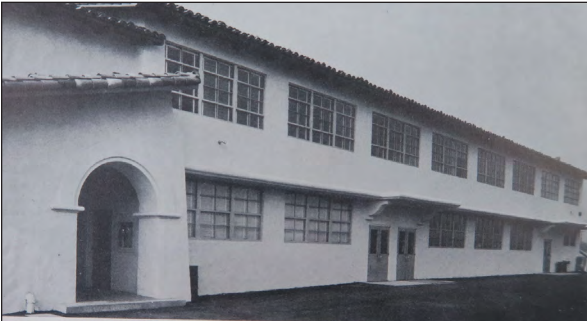
Image 31: St. Andre Bessette Hall, east elevation, view northwest (Notre Dame High School Yearbook, 1956)
