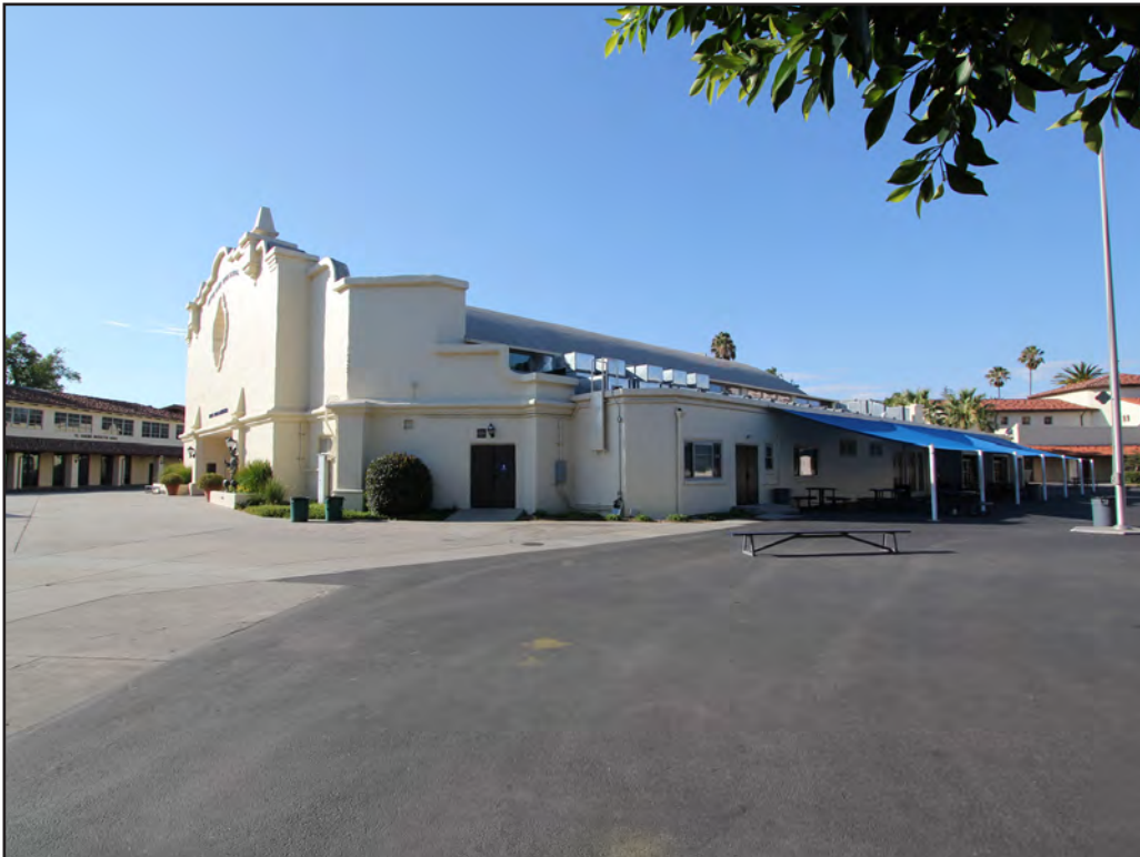
Image 79: Fritz B. Burns Gymnasium, east elevation, view northwest (Chattel, 2018)
