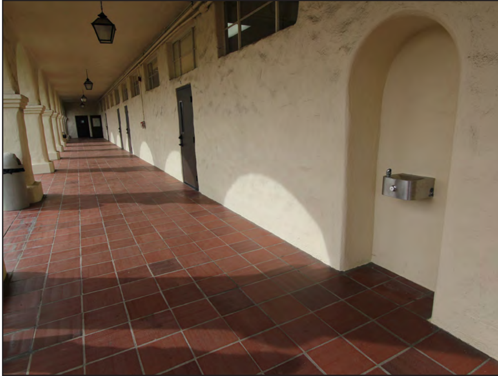
Image 40: Moreau Hall, south elevation windows and entry doors, view southwest (Chattel, 2018)
