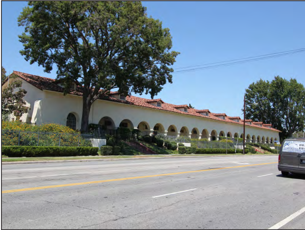
Image 33: Moreau Hall, south elevation, view east (Chattel, 2017)
