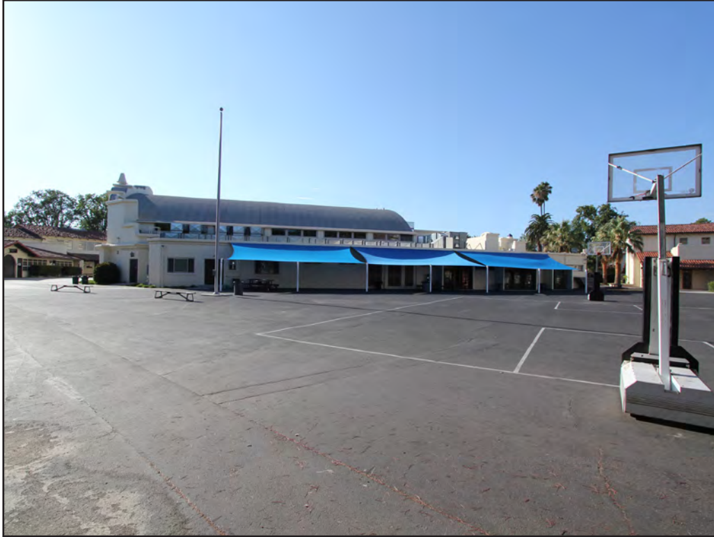
Image 78: Fritz B. Burns Gymnasium, east elevation, view northwest (Chattel, 2018)
