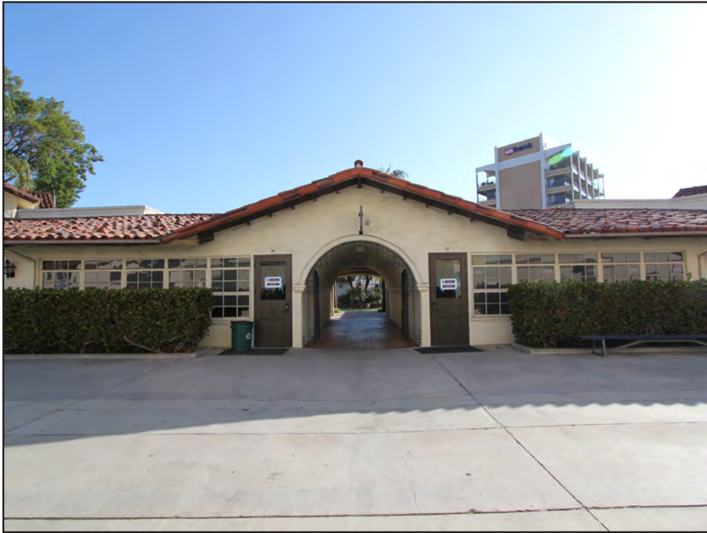
Image 95: Allegratti Building, entrance from northeast corner to courtyard, view southwest (Chattel, 2018)
