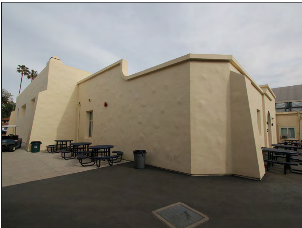
Image 75: Fritz B. Burns Gymnasium, Donahue Fitness Center, west elevation, view northeast (Chattel, 2018)
