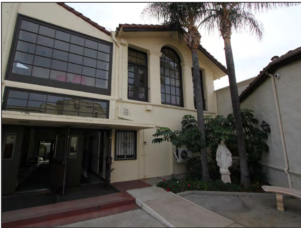
Image 52: Moreau Hall, portion of north elevation, view south (Chattel, 2018)
