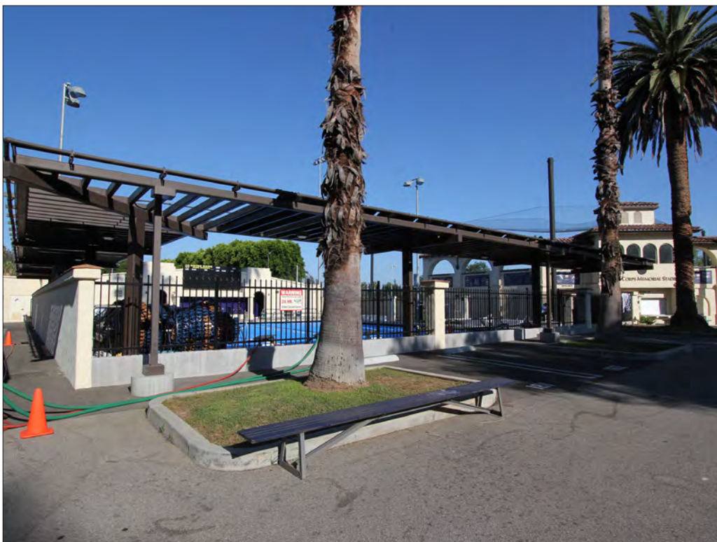
Image 118: Joseph E. Rawlinson Aquatic Center, southwest corner, view northeast (Chattel, 2018)
