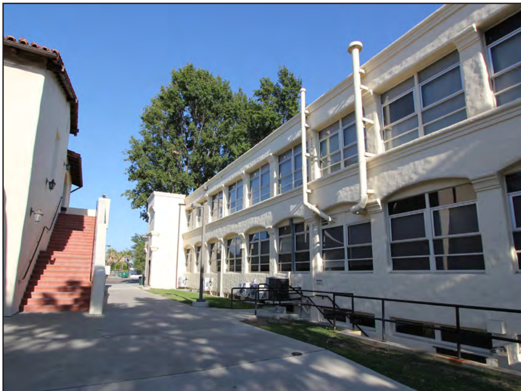
Image 46: Moreau Hall, portion of north elevation, view southeast (Chattel, 2017)
