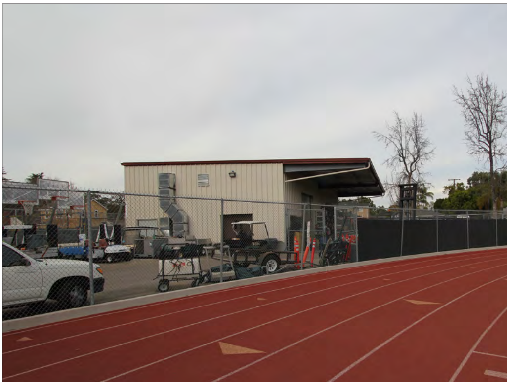
Image 120: Maintenance building, view northwest (Chattel, 2018)
