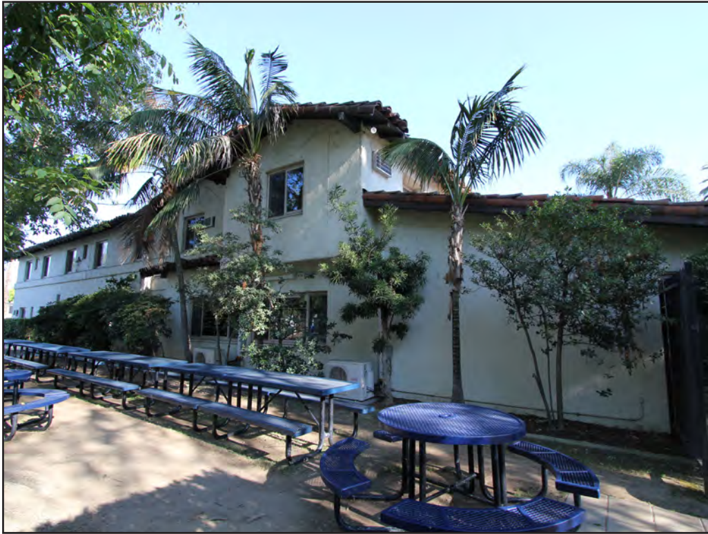
Image 69: Holy Cross Center, north elevation, view southwest (Chattel, 2018)
