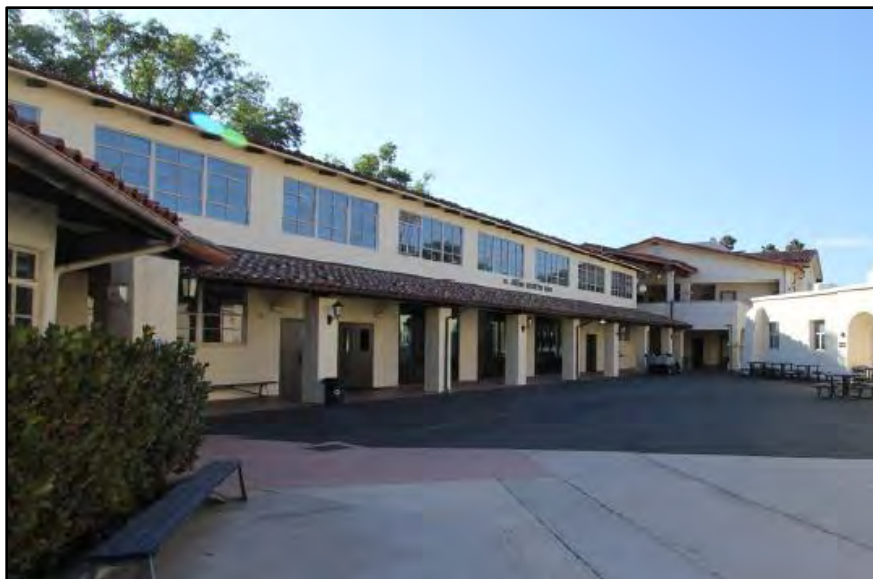
Figure 9. St. Andre Bessette Hall, east elevation, view northwest (Chattel, 2018)
