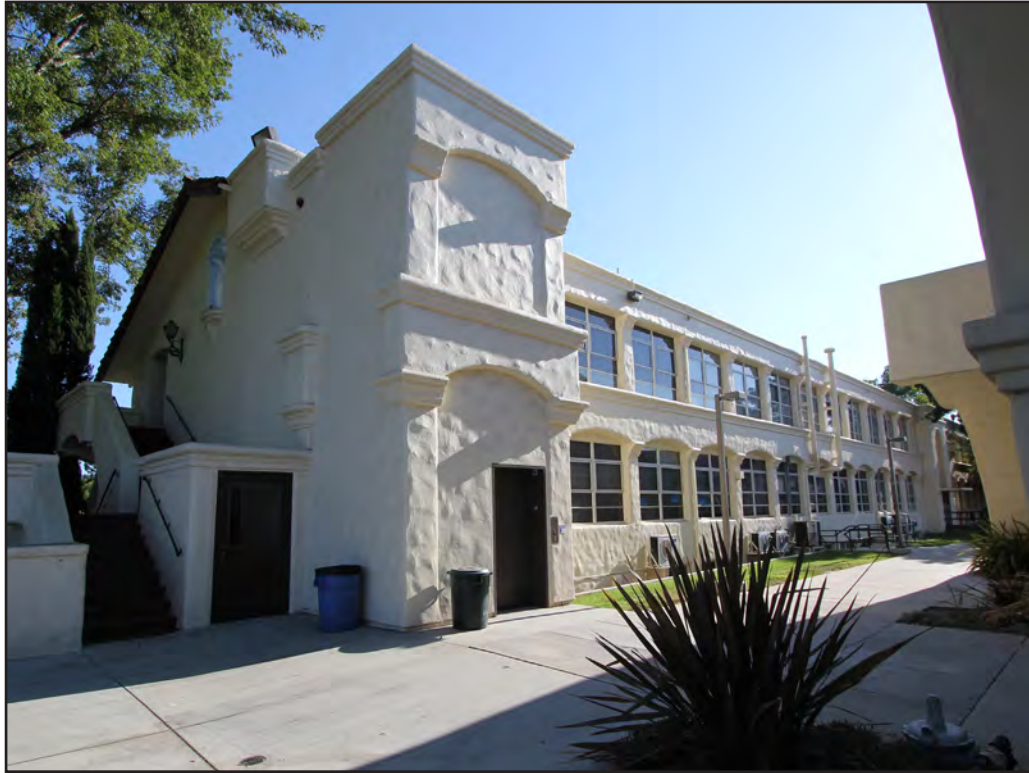
Image 45: Moreau Hall, northeast corner, view southwest (Chattel, 2017)
