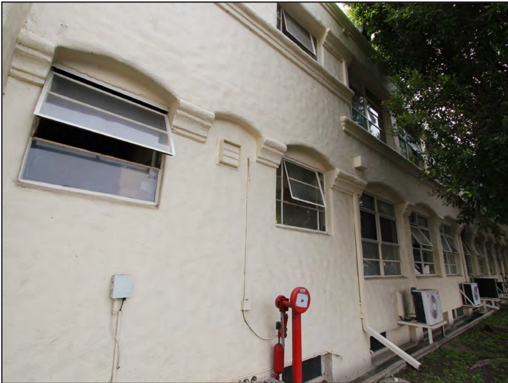
Image 47: Moreau Hall, portion of north elevation, view southwest (Chattel, 2018)
