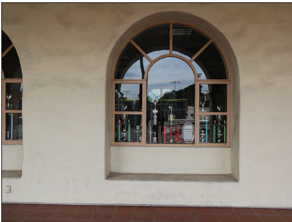
Image 108: Burns Arts & Technology Building, east elevation window detail, view west (Chattel, 2018)
