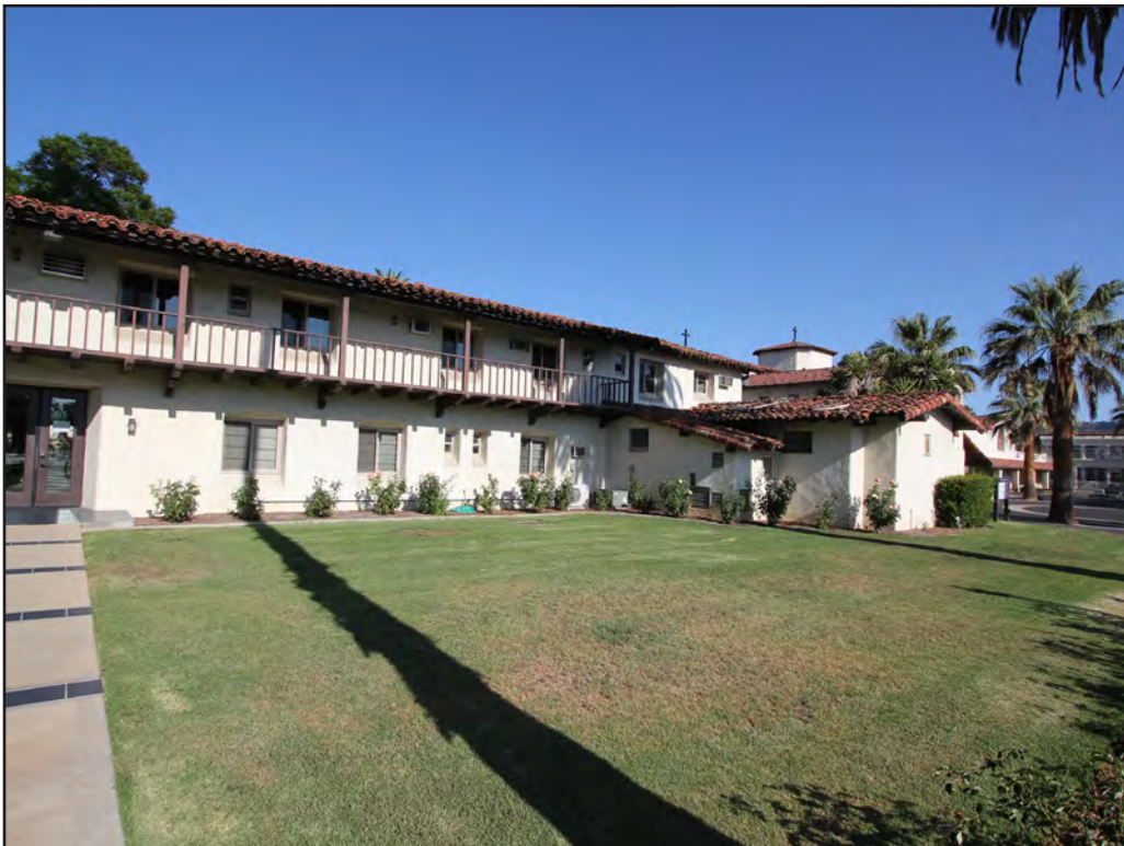
Image 56: Holy Cross Center, west elevation addition, view northeast (Chattel, 2017)
