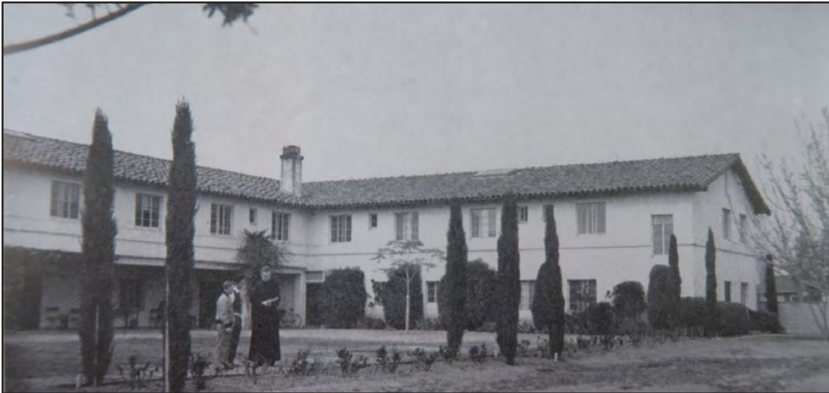
Image 23: Holy Cross Center, east elevation, view northwest (Notre Dame High School Yearbook, 1955)
