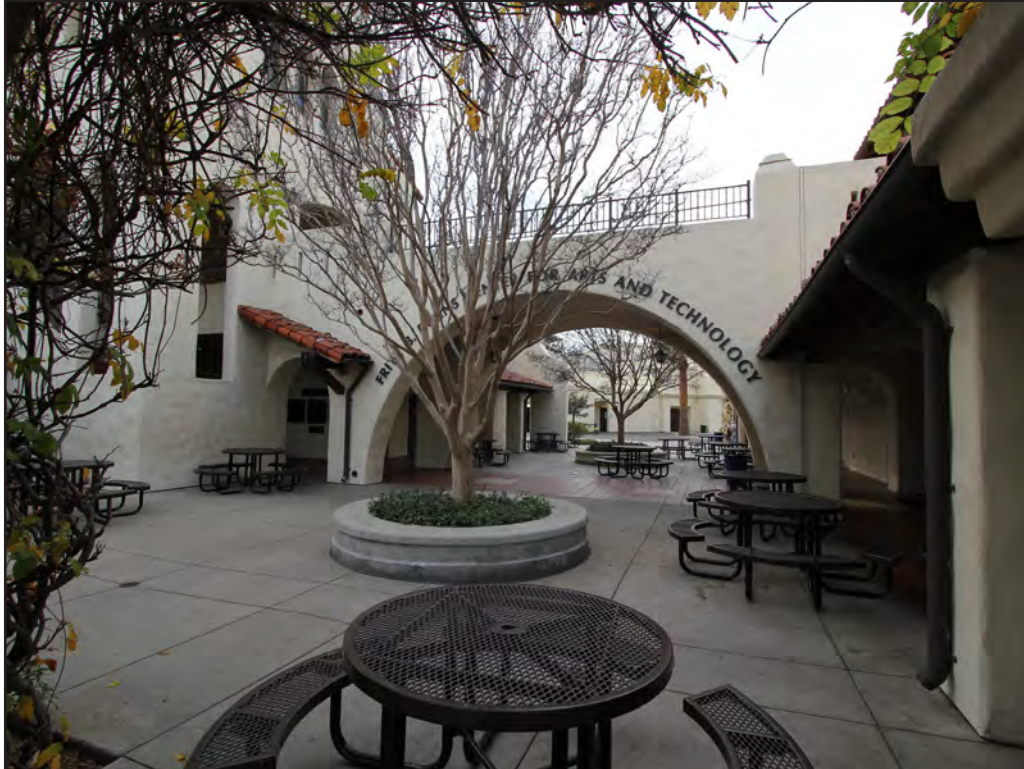
Image 103: Burns Arts & Technology Building, courtyard, view northeast (Chattel, 2018)
