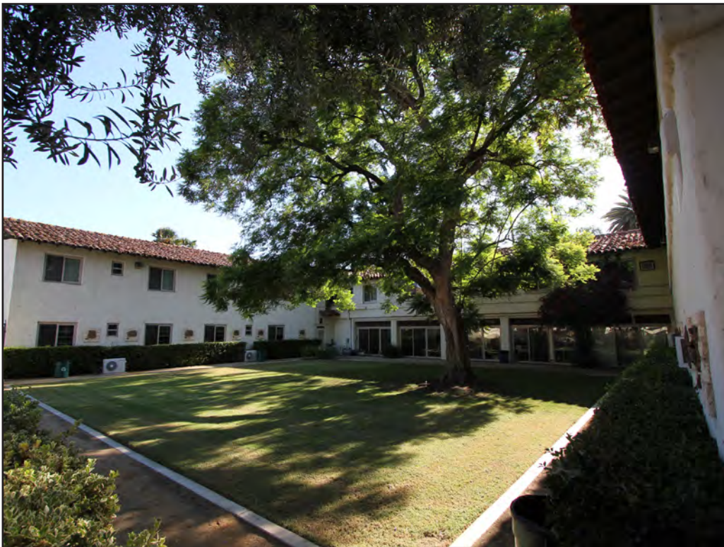
Image 66: Holy Cross Center, portion of east elevation, view southwest (Chattel, 2018)
