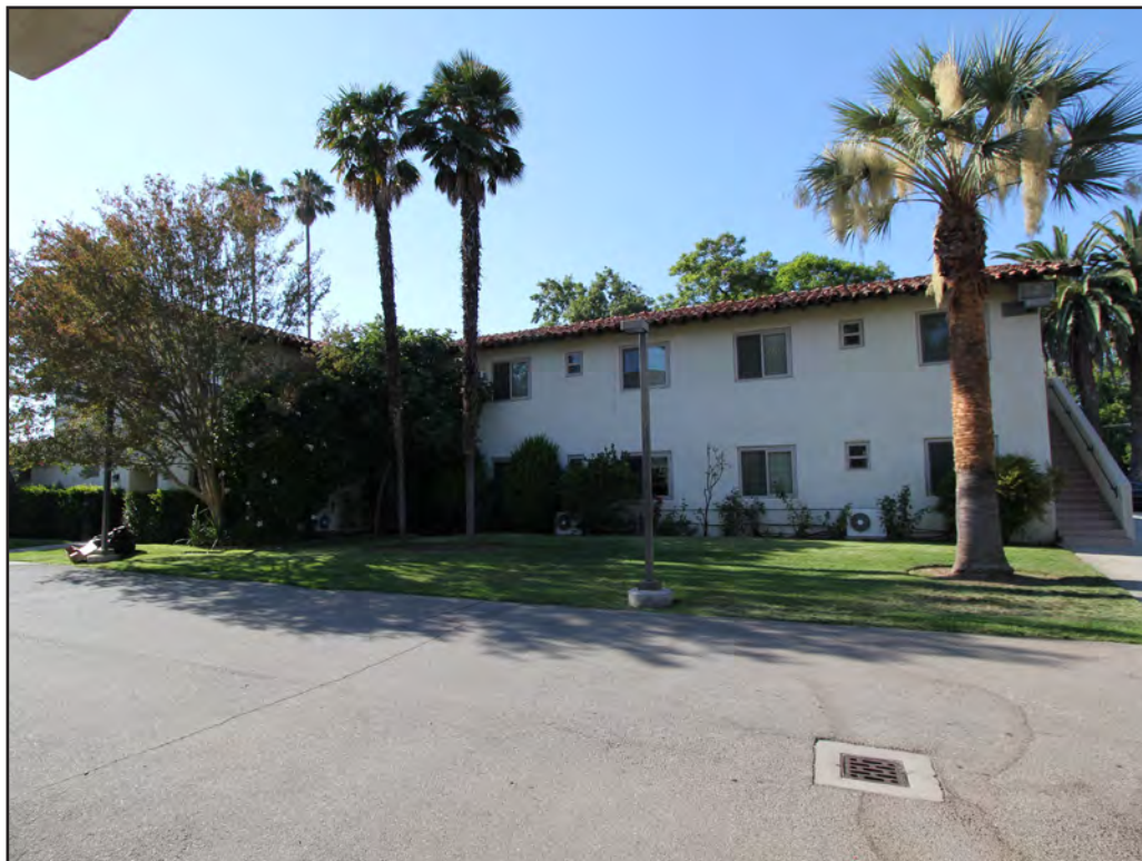
Image 62: Holy Cross Center, south elevation, view north (Chattel, 2018)
