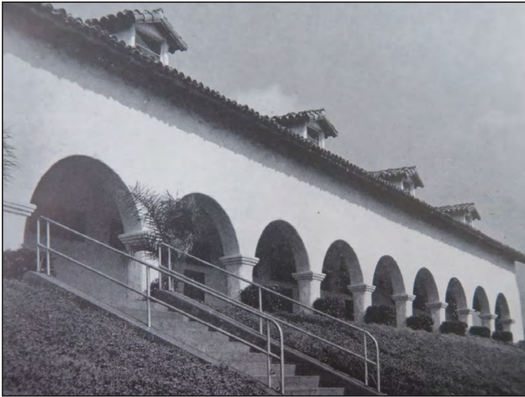
Image 12: Moreau Hall, south elevation, view northeast (Notre Dame High School Yearbook, 1952)
