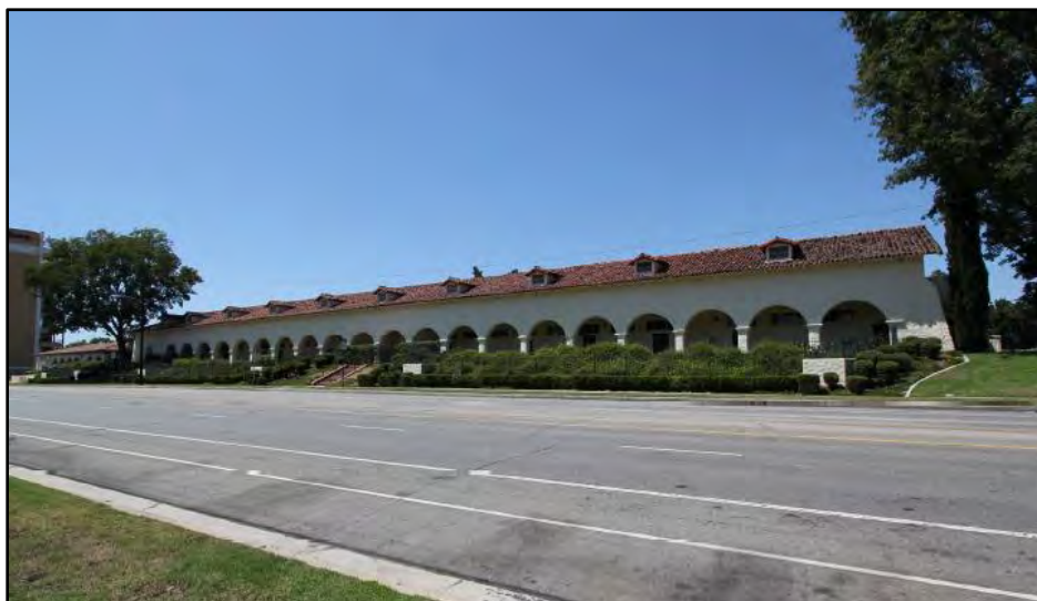
Figure 6. Moreau Hall, south elevation, view northwest (Chattel, 2017)
