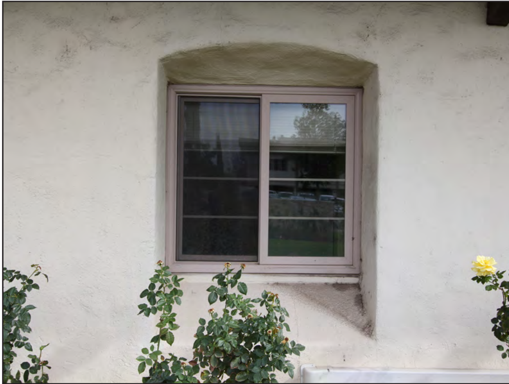
Image 59: Holy Cross Center, west elevation, view east, window detail (Chattel, 2018)
