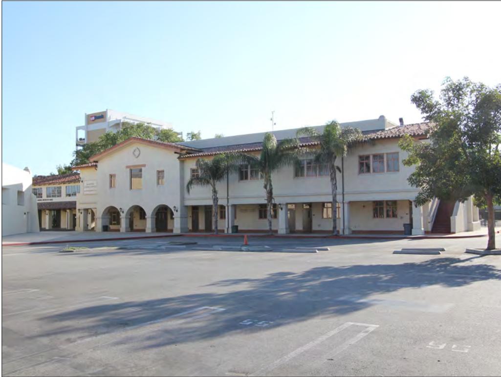
Image 109: Hampton Building, east elevation, view southwest (Chattel, 2018)
