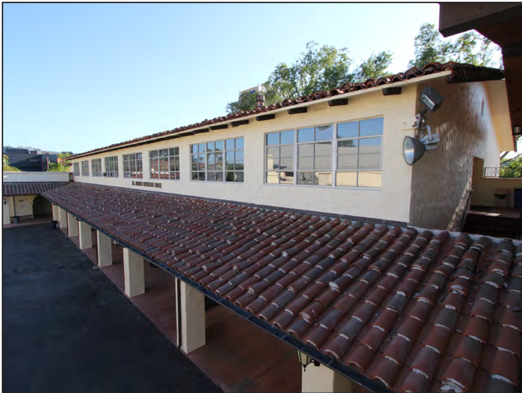
Image 82: St. Andre Bessette Hall, east elevation, view southwest (Chattel, 2018)
