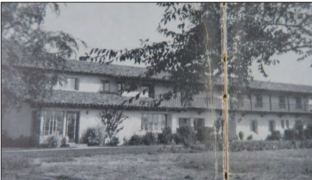
Image 18: Holy Cross Center, west elevation, view southeast (Notre Dame High School Yearbook, 1951)
