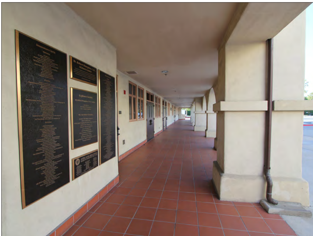
Image 112: Hampton Building, east elevation arcade, view north (Chattel, 2018)
