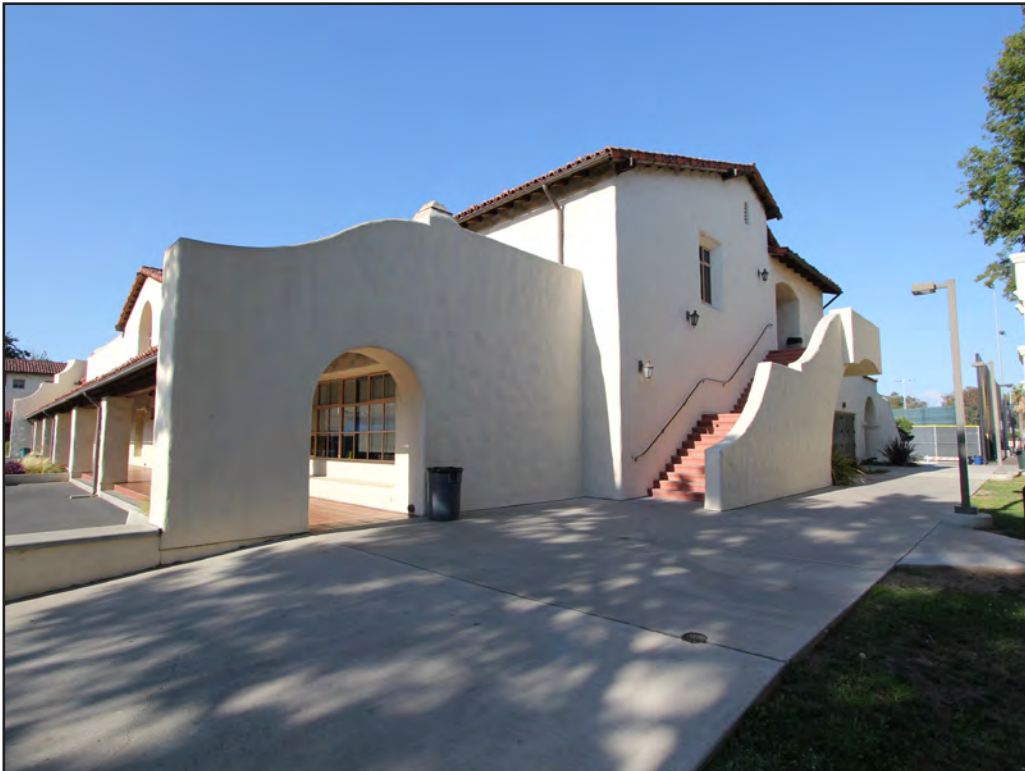
Image 102: Burns Arts & Technology Building, southwest corner, view northeast (Chattel, 2018)
