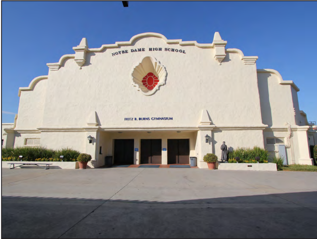
Image 80: Fritz B. Burns Gymnasium, south elevation, view northeast (Chattel, 2018)
