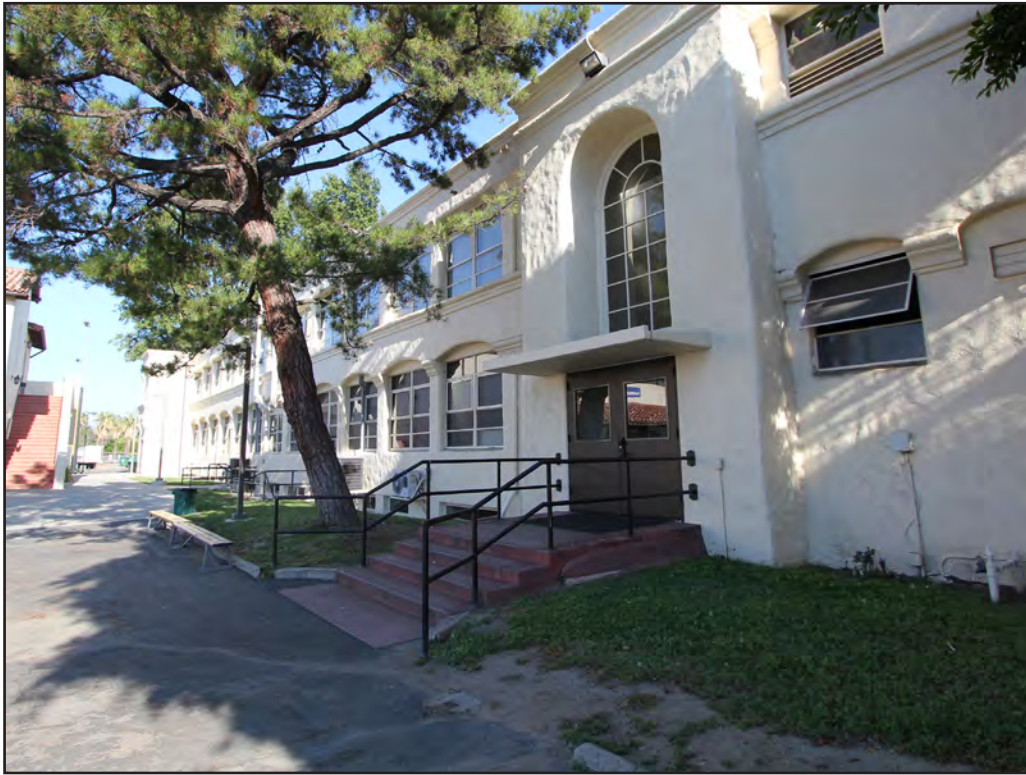
Image 48: Moreau Hall, portion of north elevation, view southeast (Chattel, 2017)
