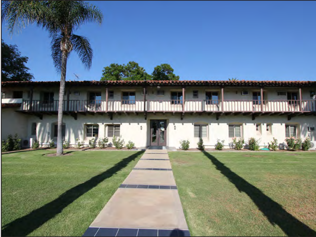
Image 55: Holy Cross Center, portion of west elevation, view east (Chattel, 2017)
