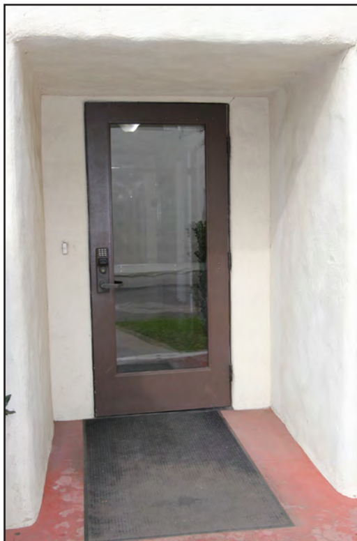
Image 61: Holy Cross Center, east elevation, view northwest (Chattel, 2018)
