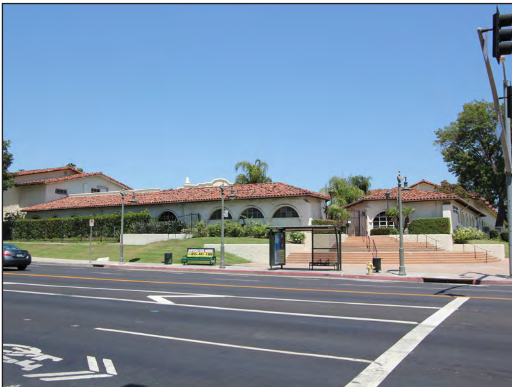
Image 92: Allegretti Building, west elevation, view northeast (Chattel, 2018)
