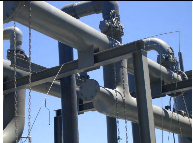
Photo 294: Flare 1 Piping Supports: May 29, 2013
