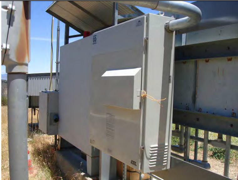
Photo 305: Flare 3 Generator Hookup Panel: May 29, 2013
