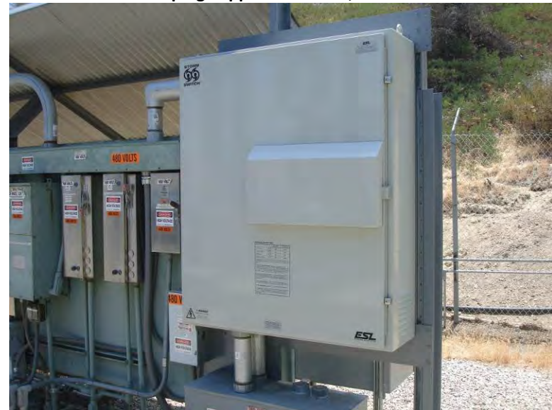
Photo 300: Flare 1 Piping Supports Emergency Generator Hookup Panel: June 12, 2013
