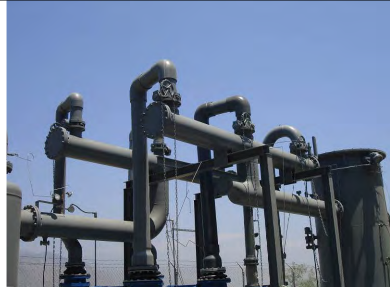
Photo 298: Flare 1 Piping Supports: June 12, 2013
