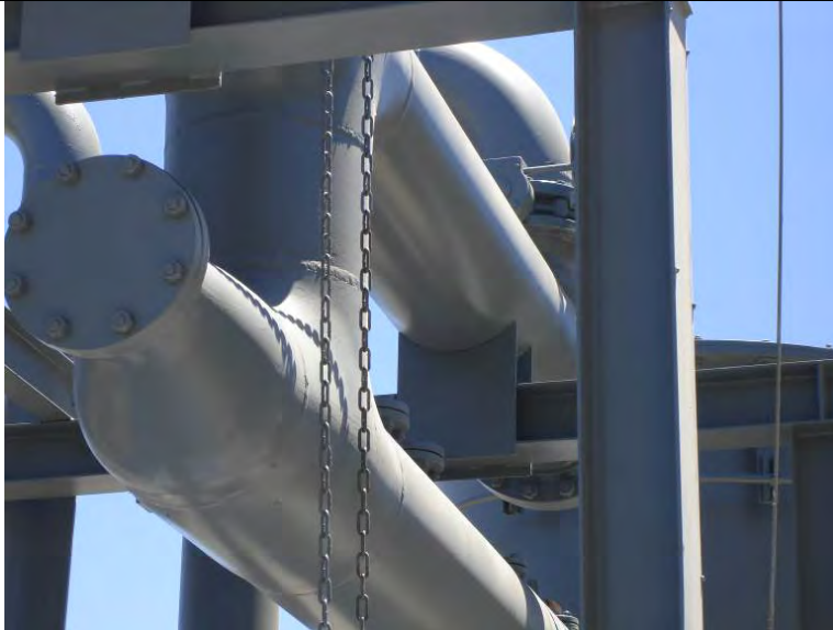
Photo 297: Flare 1 Piping Supports: May 29, 2013
