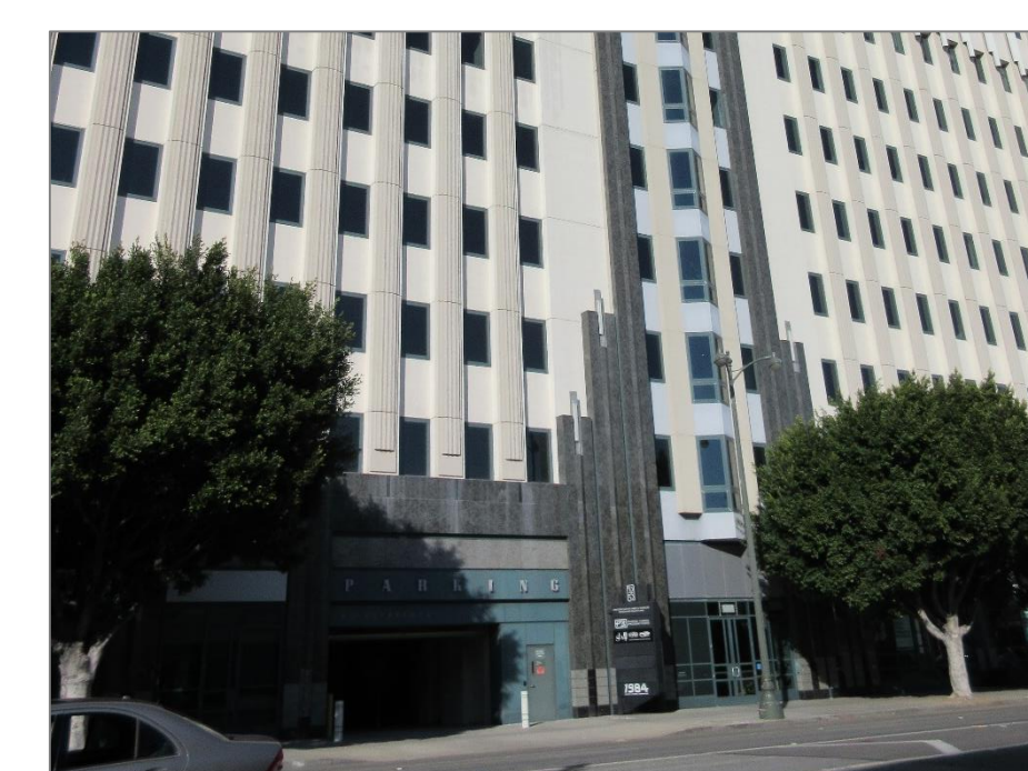
Central entrance, lower visibility
