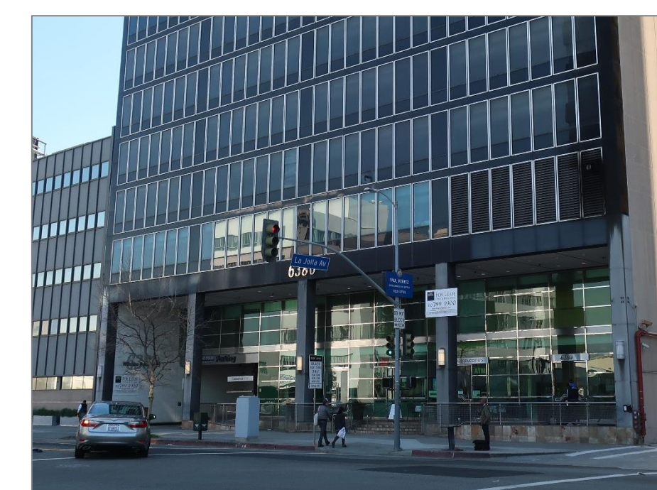
Underground with visible driveway
