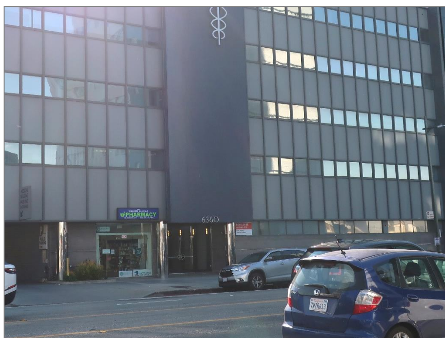
Central entrance, lower visibility
