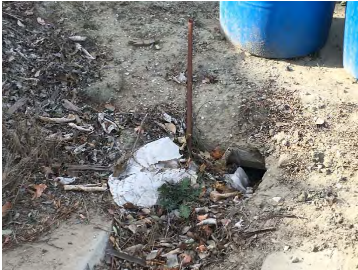
Photo 237: Drain Clogged at Leachate Facility: December 9, 2015
