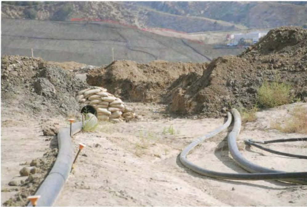
Figure 3: Channel out of Basin A Partially Blocked
