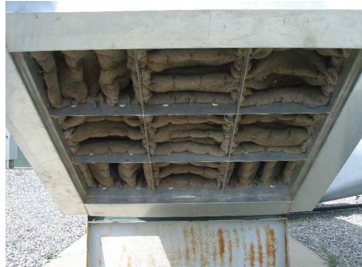
Photo 104: Old Flare 10 Air Blower Filter: October 14, 2015
