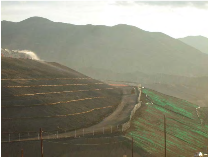
Photo 253: City Slope Erosion Control: October 14, 2015
