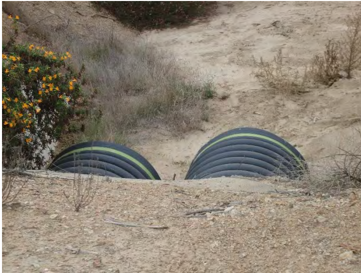
Photo 269: Native Slope Drainage to Bench Above Offices: October 28, 2015
