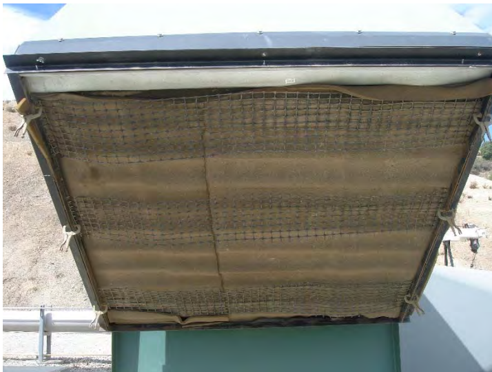
Photo 103: New Flare 9 Air Blower Filter October 14, 2015
