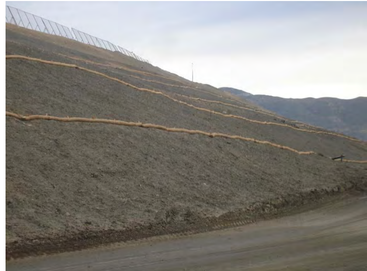
Photo 262: City Slope Erosion Control: October 28, 2015
