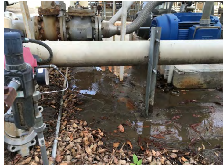
Photo 234: Water Pipe Leak at Treatment Plant: December 9, 2015
