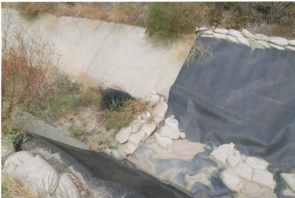
Photo 6: Geomembrane liner at beginning of lined portion between Basin D and Flare 9-10 access road
