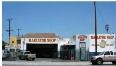
Repair and Maintenance Facilities
