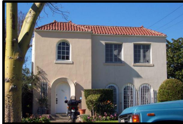
39- 5012 W BEVERLY BLVD; 253 N IRVING BLVD Contributor 1923- Spanish Colonial Revival Lot Coverage: 32% Setback: 36' # of Stories: 2 Approx. Height: 23'
