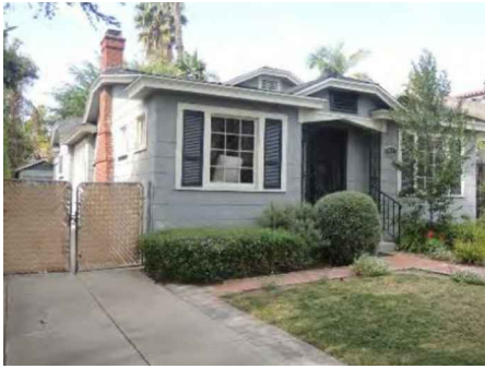
1629 N. Stanley Ave. American Colonial Revival Lot Coverage: 42% Setback: 23.25' Stories: 1.5 Non Contributor Approx. Ht: 21'-0"
