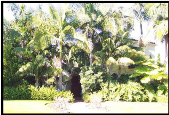
38- 101 N WINDSOR BLVD – Contributor 1927- Spanish Colonial Revival Lot Coverage: 35% Setback: 32' # of Stories: 2 Approx. Height: 21' * Second story addition under construction
