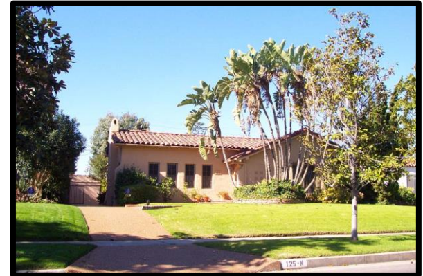
35- 125 N WINDSOR BLVD – Contributor 1922- Spanish Colonial Revival Lot Coverage: 34% Setback: 33' # of Stories: 1 Approx. Height: 16' * Second story addition approved
