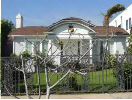
1605 N. Stanley Ave. American Colonial Revival Lot Coverage: 45% Setback: 24.00' Stories: 1.5 Altered Contributor Approx. Ht: 21'-0"
