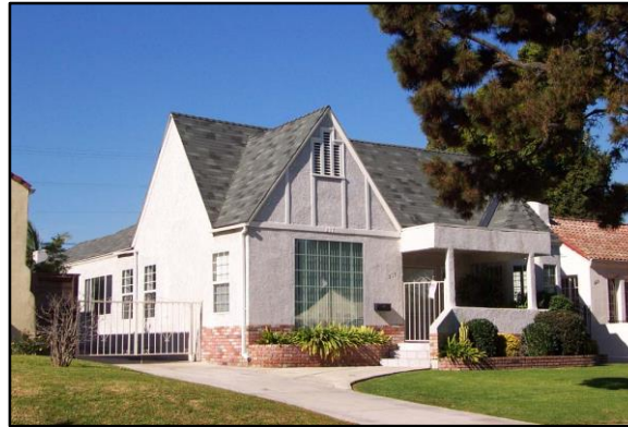
26- 217 N WINDSOR BLVD – Non Contributor 1923- Spanish Colonial Revival Lot Coverage: 49% Setback: 29' # of Stories: 1 Approx. Height: 14' * New 2-story under construction currently
