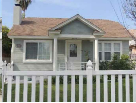
1619 N. Stanley Ave. American Colonial Revival Lot Coverage: 58% Setback: 24.00' Stories: 1.5 Altered Contributor Approx. Ht: 21'-0"
