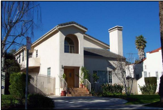
53- 137 N IRVING BLVD– Non Contributor 1923/90- Post Modern Remodel Lot Coverage: 43% Setback: 30' # of Stories: 2 Approx. Height: 23'
