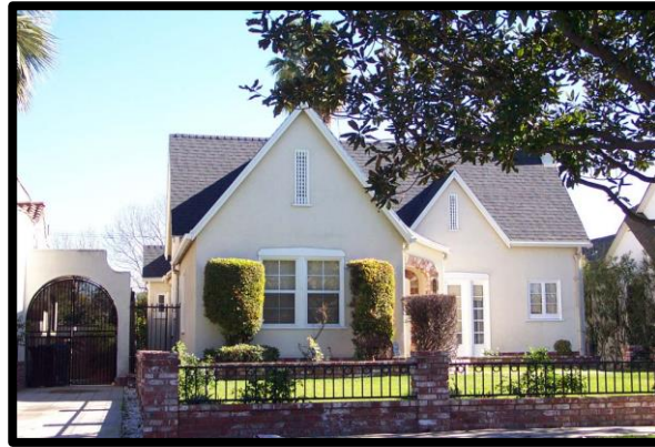
11- 146 N WINDSOR BLVD –Contributor 1923- English Revival Lot Coverage: 32% Setback: 30' # of Stories: 2 Approx. Height: 19'
