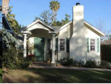
1632 N. Stanley Ave. American Colonial Revival Lot Coverage: 35% Setback: 25.00' Stories: 1 Non Contributor Approx. Ht: 15'-0"
