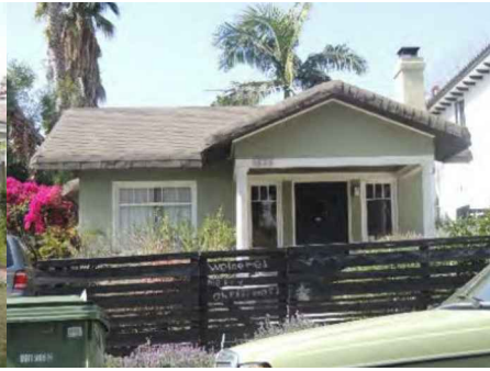
1633 N. Stanley Ave. American Colonial Revival Lot Coverage: 38% Setback: 21.50' Stories: 1 Non Contributor Approx. Ht: 21'-0"
