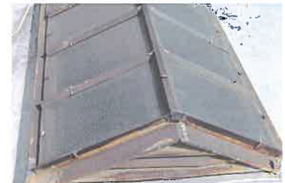
TYPICAL RUSTED SKYLIGHT
