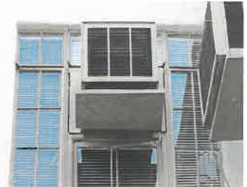
STEEL CASEMENT WINDOW WITH AIR CONDITIONERS
