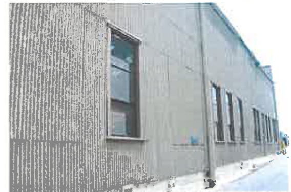
CORRUGATED METAL SIDING INDICATING PATCHING - AVENUE 12
