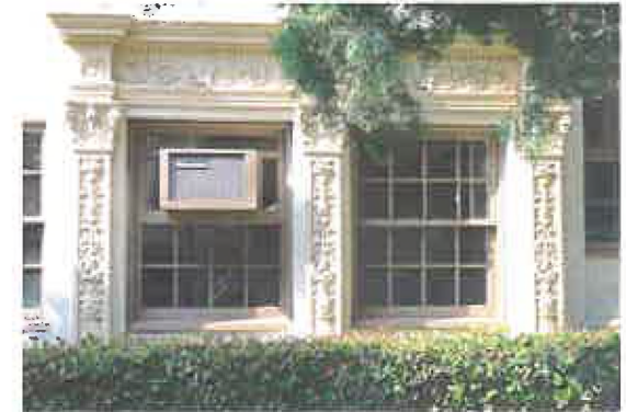
WOOD DOUBLE HUNG WINDOW IN CAST SURROUND
