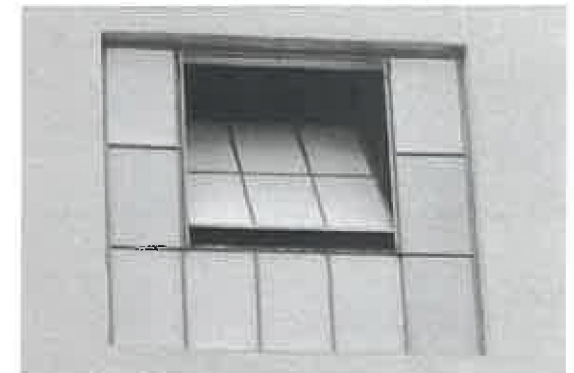
STEEL PIVOT WINDOW WITH BACK PAINTED GLASS
