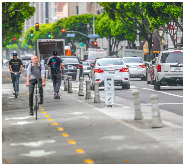
Figure 12. Main & Spring Street Forward protected two-way bike lanes Photo by LADOT Livable Streets
