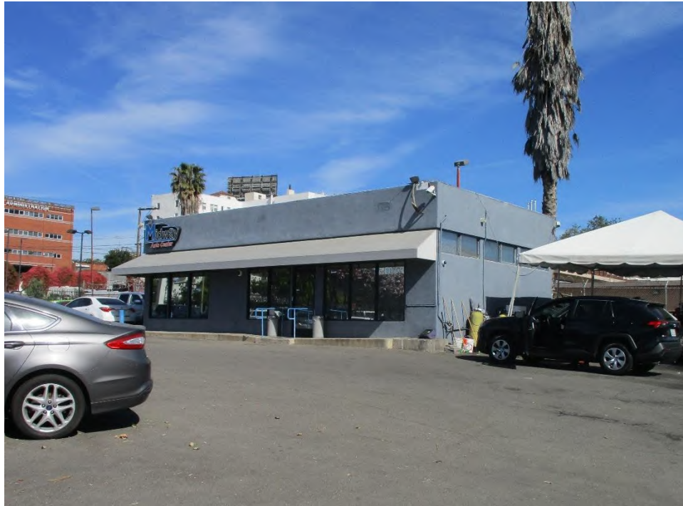
Figure 17. 3725 Beverly Boulevard main (south) and west elevations (IMG_2546)
