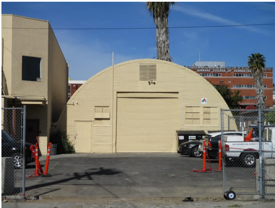
Figure 1. 307 N. Madison Ave main (north) elevation (IMG_2551)
