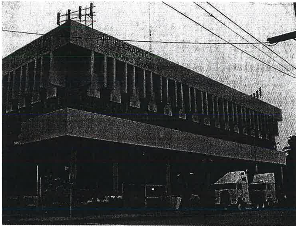
AT&T Wireless Services previously mounted several antennas to the roof of the building. View to the southeast.
