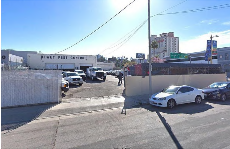
Figure 4. 306 N. Madison Avenue, Service Garage, west elevation of the building and parking area (Photo courtesy of Google Earth, 2018)
