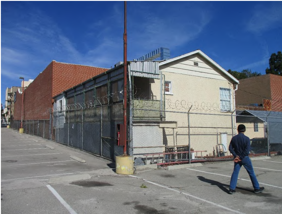
Figure 3. Two-story Garage south (rear) and east elevations (IMG_2508)
