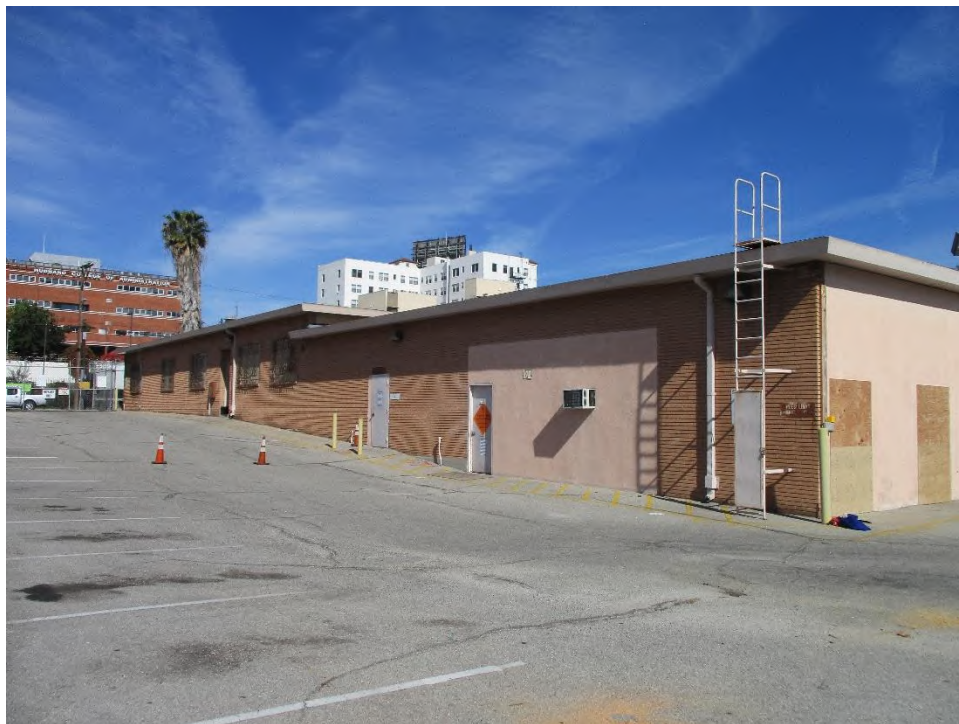
Figure 14. South and east elevation of the Plant Operating Center, looking northwest (IMG_2526)
