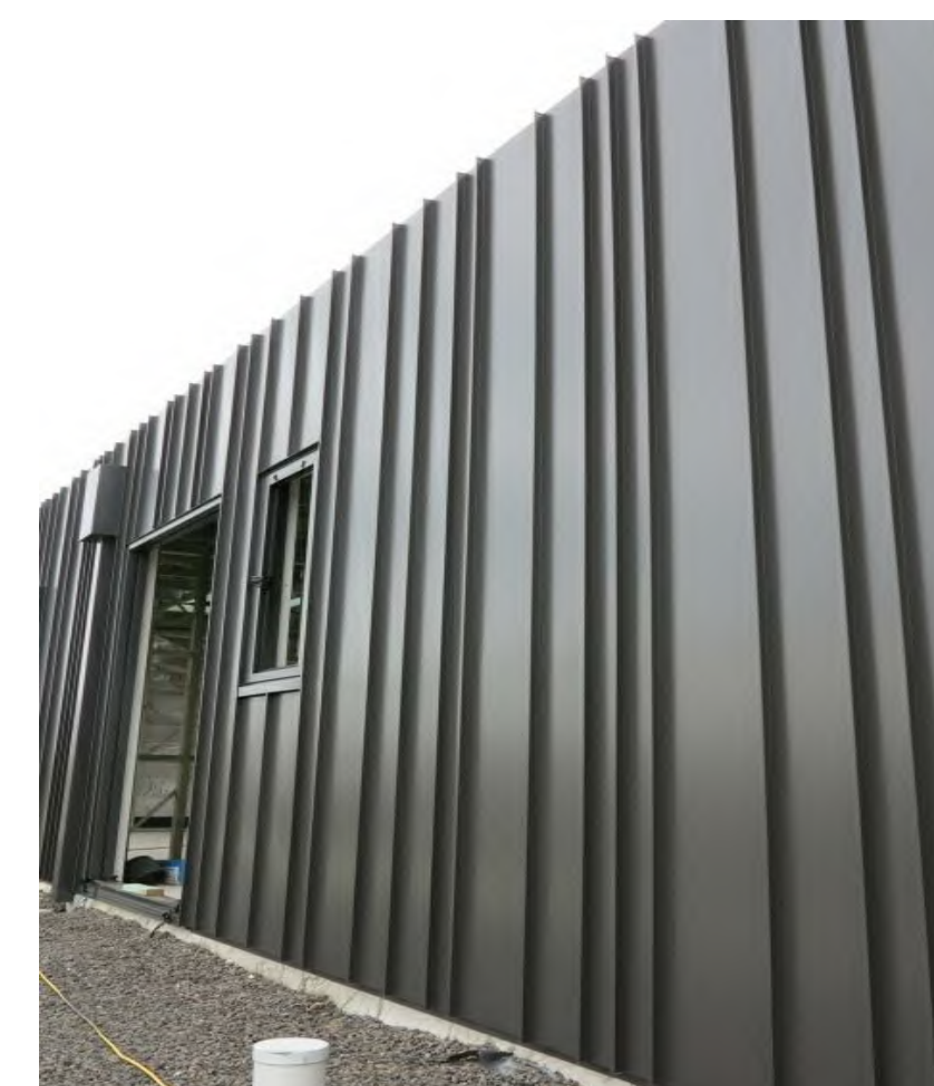
STAGGERED STANDING SEAM EXAMPLE COLOR: DARK GREY SUBSTITUTE MATERIAL - STUCCO W/ STAGGERED REVEALS
