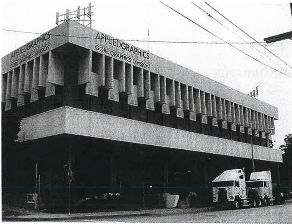
AT&T Wireless Services previously mounted several antennas to the roof of the building. View to the southeast.
