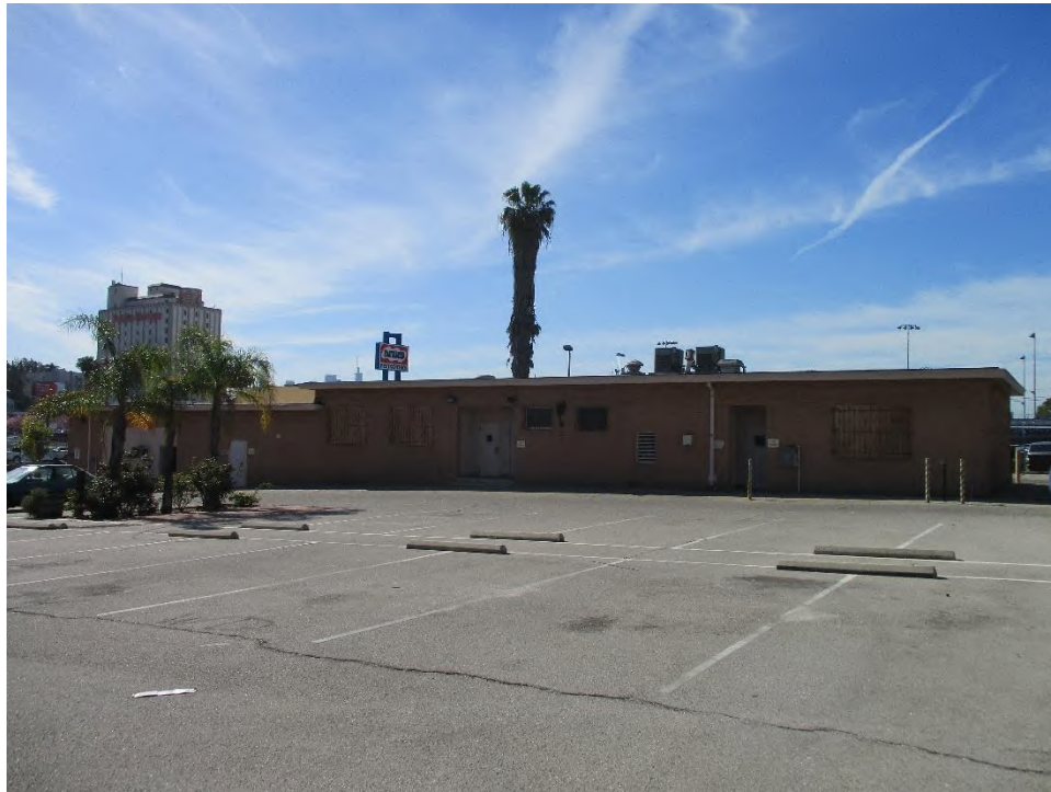
Figure 13. North elevation of the Plant Operating Center, looking southeast (IMG_2502)
