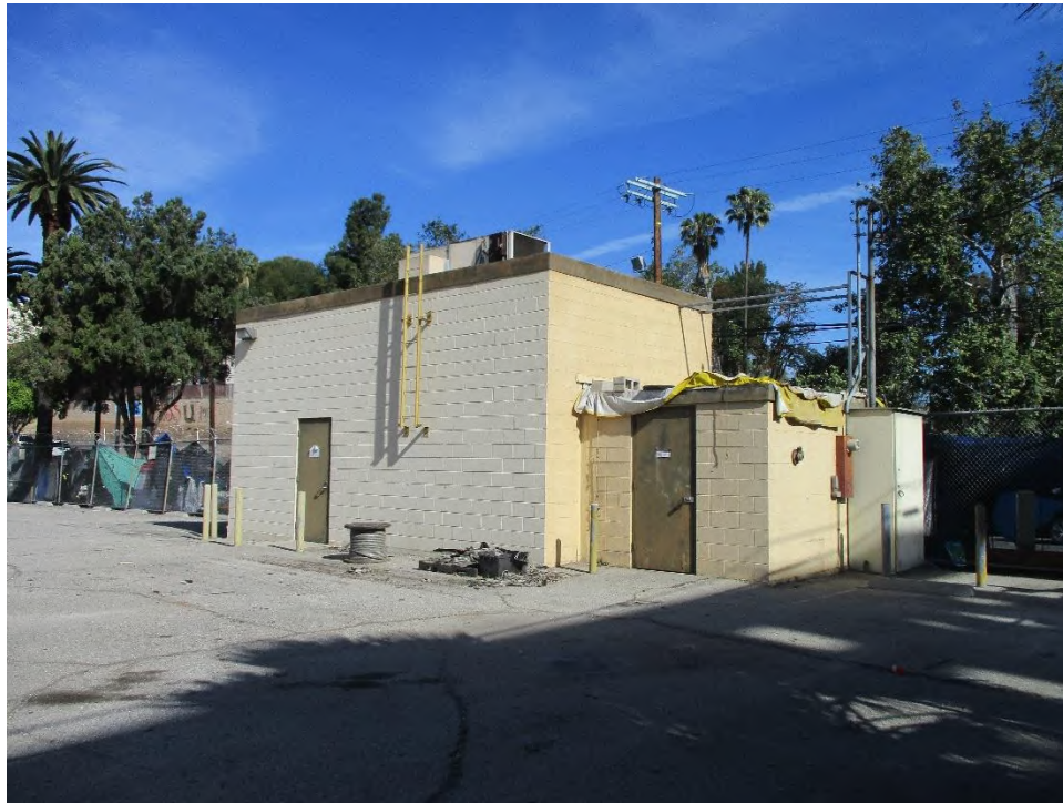
Figure 16. Equipment Storage Building main (south) and east elevations (IMG_2466)
