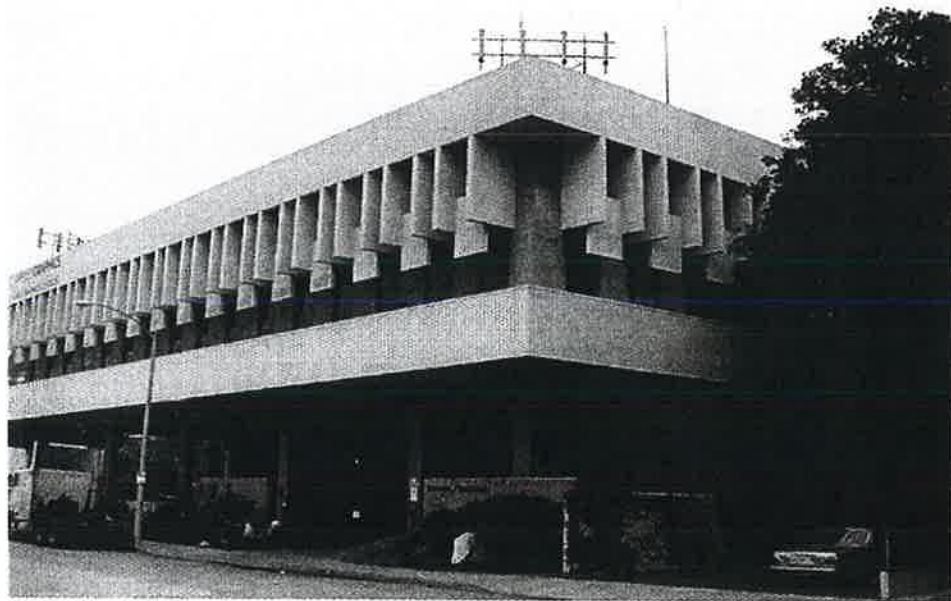
AT&T Fixed Wireless Services proposes to place a new equipment shelter on the roof of the building. Four new antennas will be mounted to this equipment shelter. View to the northeast.
