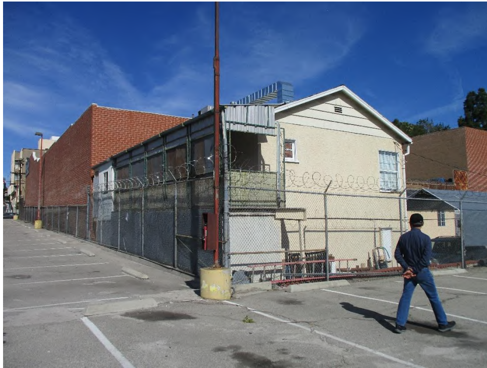
Figure 11. Two-story Garage south (rear) and east elevations (IMG_2508)
