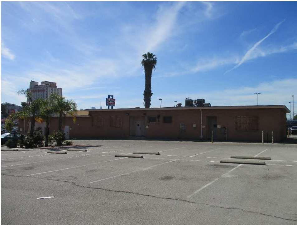
Figure 1. North elevation of the Plant Operating Center, looking southeast (IMG_2502)
