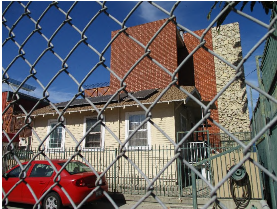
Figure 9. 3812 Oakwood Avenue Building A main (west) and south elevations (IMG_2517)
