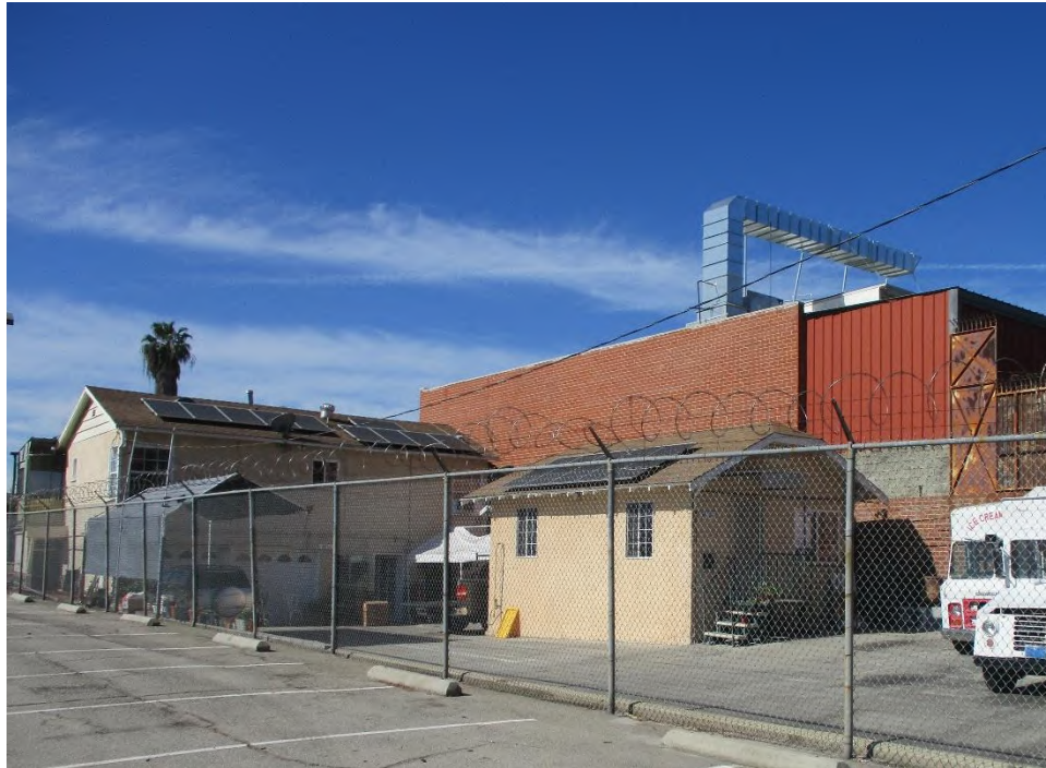
Figure 10. Building B north (main) and east elevation, with two-story garage in background, looking southwest (IMG_2519)
