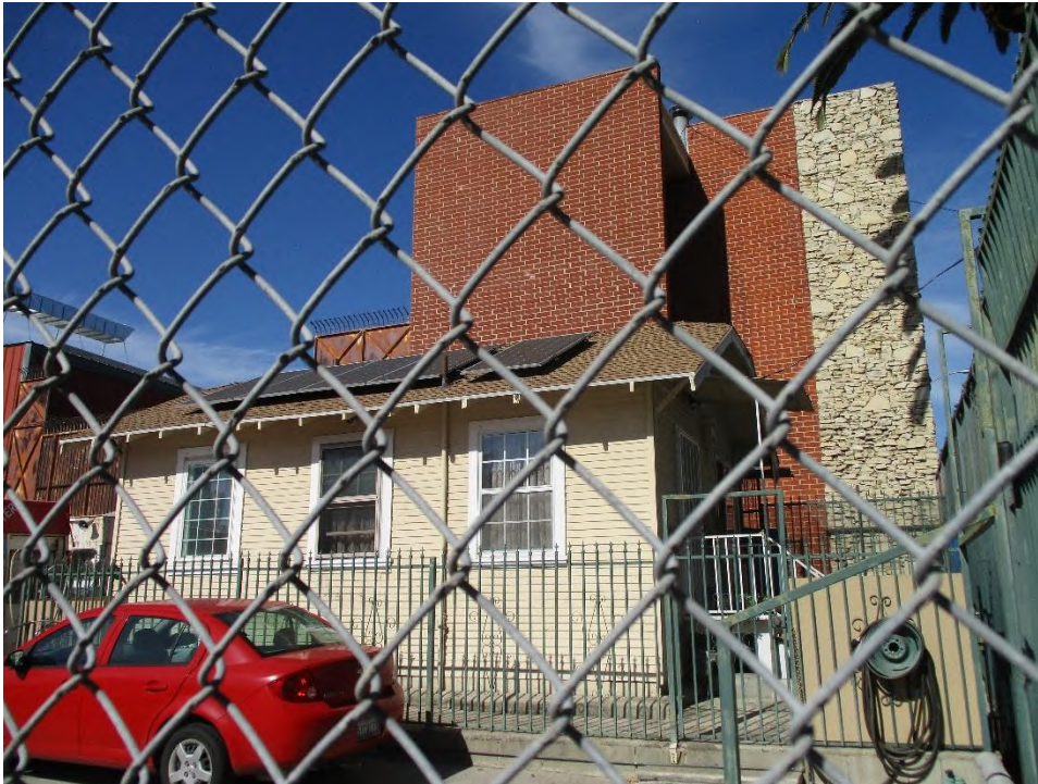
Figure 1. 3812 Oakwood Avenue Building A main (west) and south elevations (IMG_2517)
