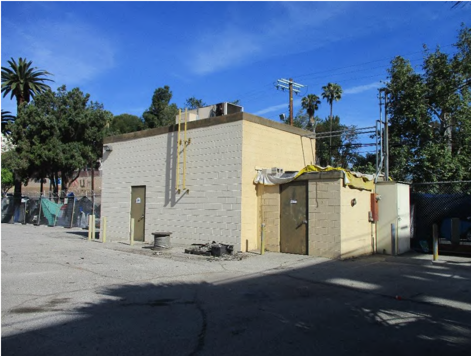
Figure 4. Equipment Storage Building main (south) and east elevations (IMG_2466)
