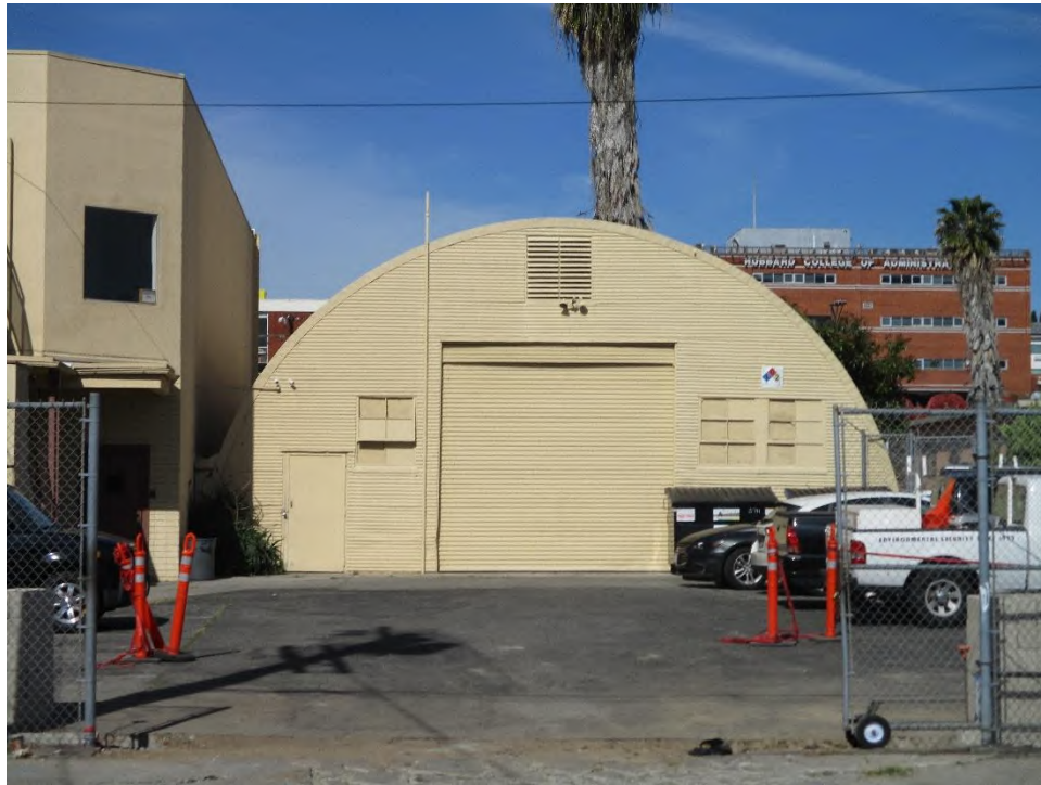
Figure 18. 307 N. Madison Ave main (north) elevation (IMG_2551)
