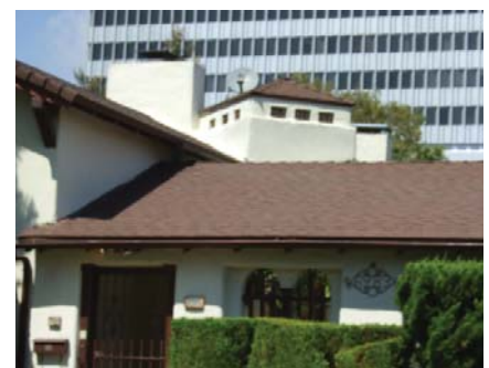
Asphalt shingle is not an appropriate material for Spanish and Mediterranean style roofs.
