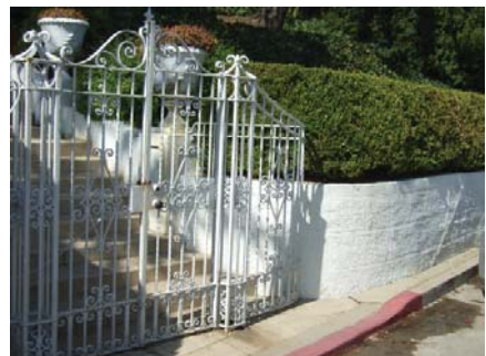
Walls and gates are often the most visible parts of the HPOZ. Historic materials should always be retained.
