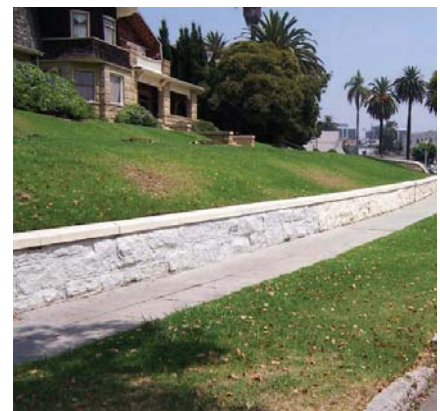
This retaining wall is a significant part of the neighborhood's historic fabric.
