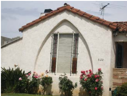
When new windows must be installed they should match the originals. Poorly placed windows, such as the one above, can dramatically impact the character of the district.
