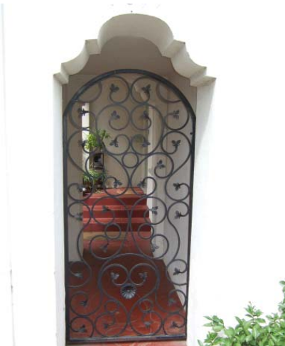
Arcades should always read as open voids. When grilles are appropriate they should be transparent and architecturally compatible.
