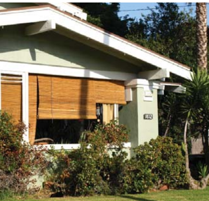
Non-permanent devices such as this bamboo screen may effectively screen a porch without altering the home and disrupting the streetscape.
