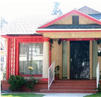
This doorway has been altered with a metal gate and plate glass sidelights.
