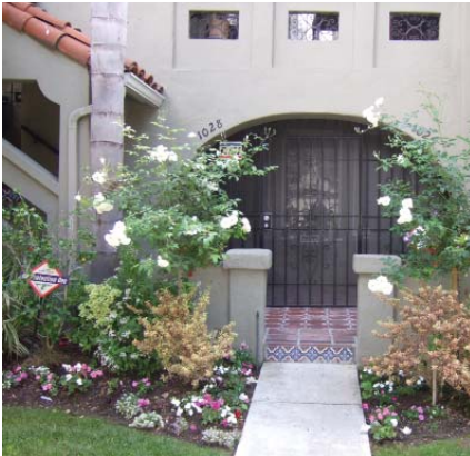
Enclosing a front porch disrupts the porch's intended purpose as an outdoor room.
