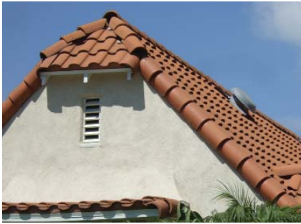
Clay tile is an inappropriate material for this English Cottage style home.
