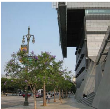
IMAGE A: Example of building overhang that does not interfere with street tree growth.
