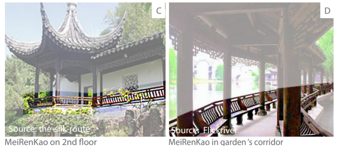
Figure C & D show different ways of applying Mei Ren Kao, a kind of bench, in traditional Chinese architecture. In some cases, the benches can also combine with a low retaining wall.
