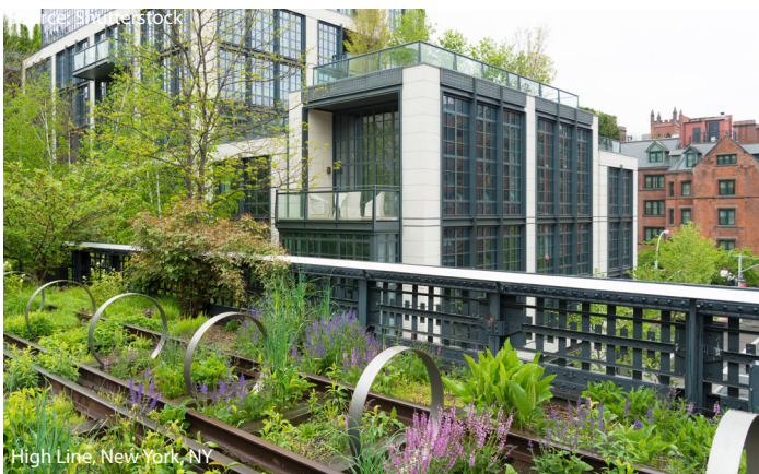
These images illustrate how historic rail features can be incorporated into the design of both active and passive spaces. These features can serve many functions such as wayfinding or public art.
