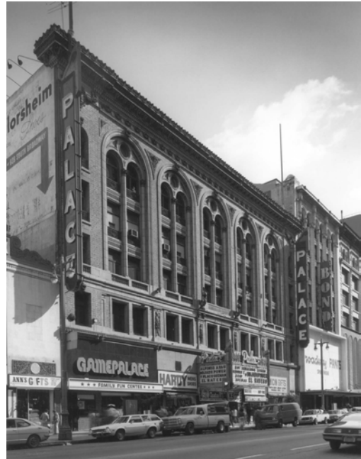
Palace Theater, 634 S. Broadway, 1911 (Office of Historic Resources)
