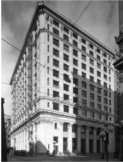
Pacific Southwest Trust & Savings Bank, National Register, Spring Street Financial District, 215 W 6 th Street, 1920 (Los Angeles Public Library)
