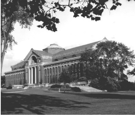
Roosevelt Hall, Washington D.C., 1972 National Register of Historic Places Nomination
