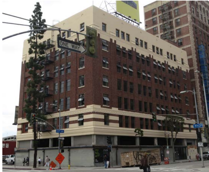
Harris Building, 1923 110 W 11th Street (SurveyLA)
