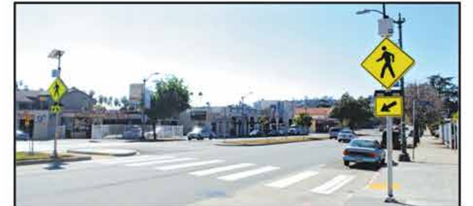
This picture shows a midblock crossing with a pedestrian refuge area. Potential locations for midblock crossings are at Crenshaw/Florence Avenue or at Crenshaw/73rd Street.
