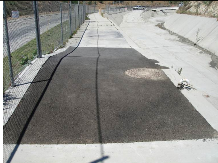
Photo 66: Terminal Basin Manhole Repair (June 5, 2012)
