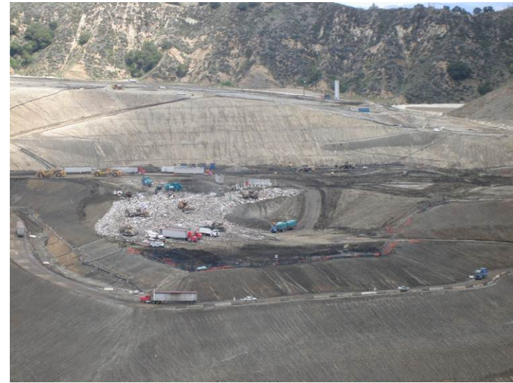
Photo 68: Working Face Active Fill Area (April 12, 2012)
