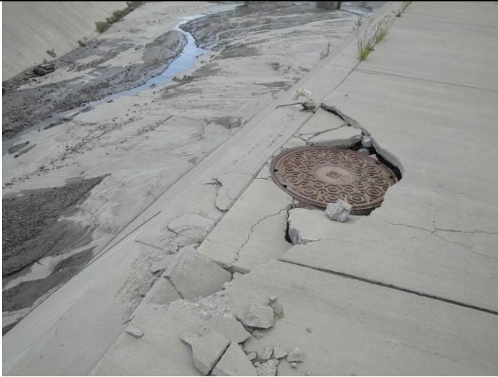
Photo 65: Terminal Basin (Cracks in slab on top of embankment) (April 12, 2012)
