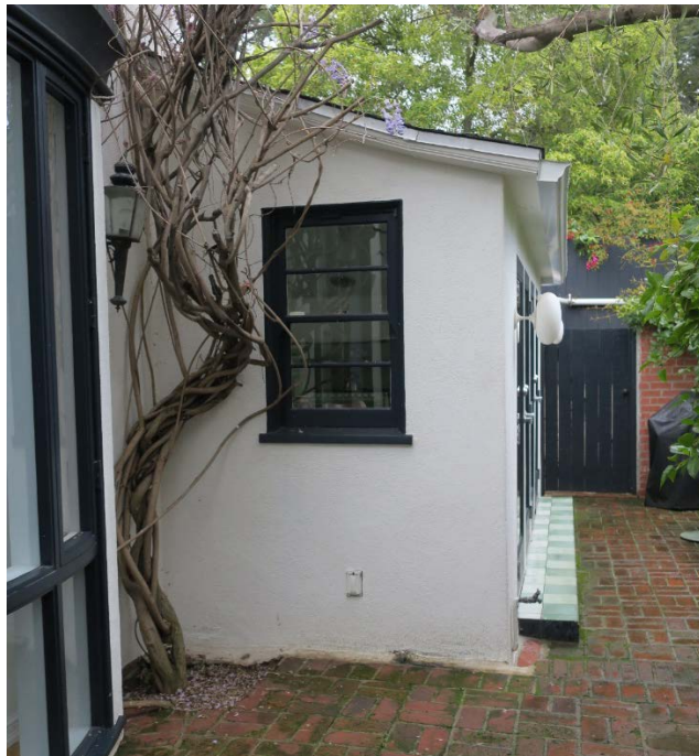
Seiter Residence, view west of the north façade, 1939-42 volume (ARG, 2020).
