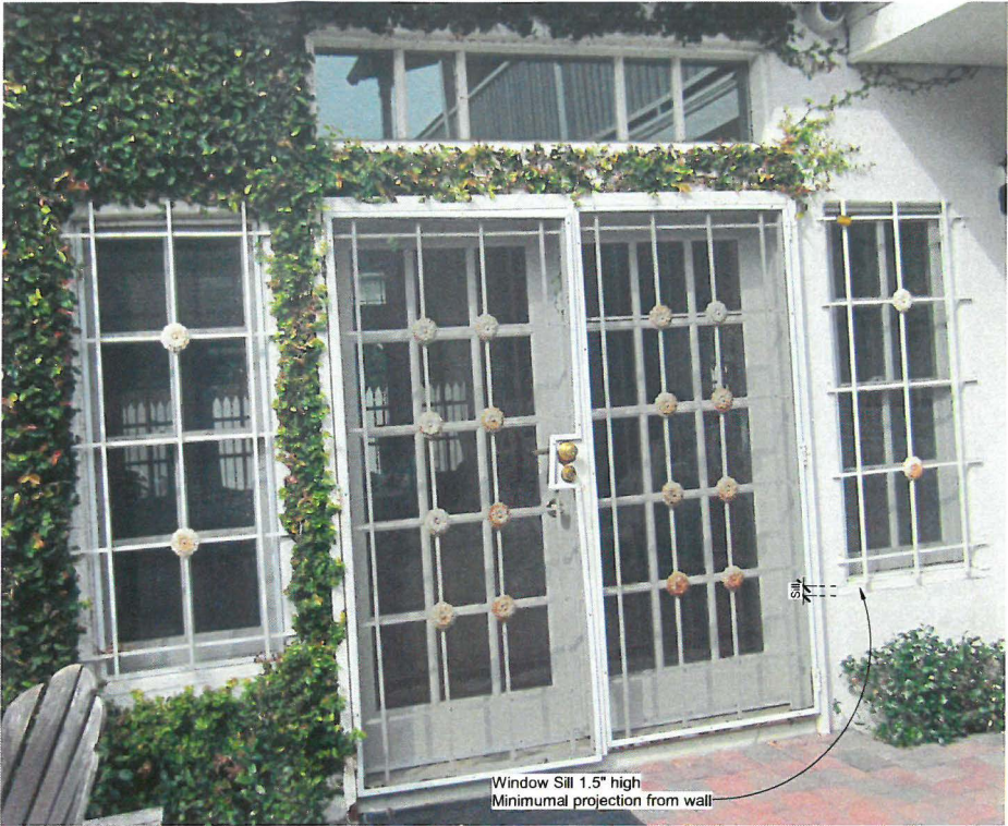
Existing Windows and Doors do not have exterior casings, minimal window sill projection and about 1.5\"/>
