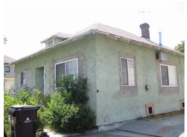
The original window openings have been altered and the accompanying sashes and sills have been removed resulting in a house with out of scale fenestration that is inconsistent with the neighborhood.
