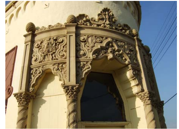
Architectural features such as the decorative plaster work surrounding this building entrance should be preserved.
