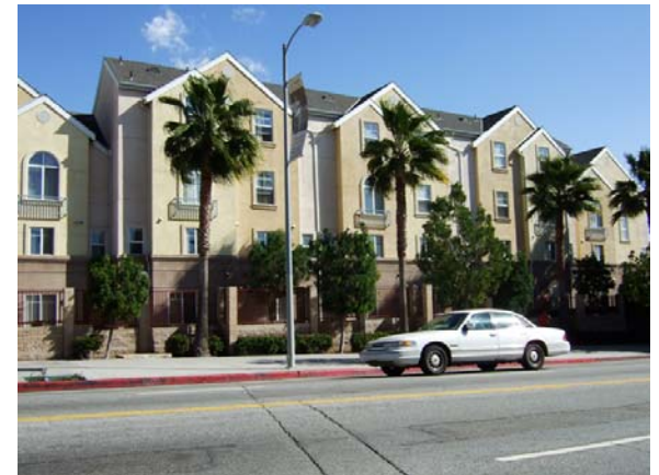
The apartment building show here articulates the façade through plane changes, different building materials and decorative window sills. The roof is articulated through a cross-gable design that makes the building appear less massive.
