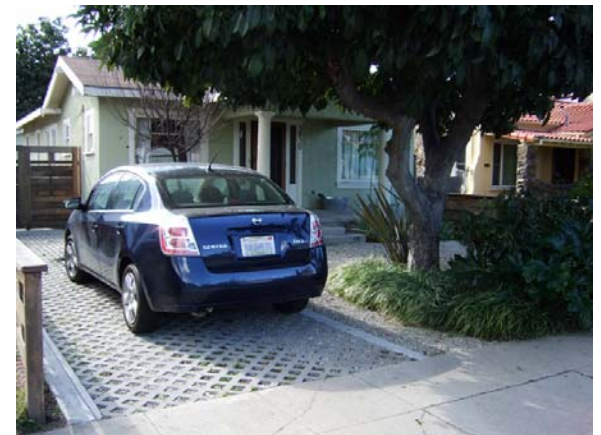
This driveway utilizes grass-crete which increases rain water permeability and adds an attractive landscape feature to the front yard.
