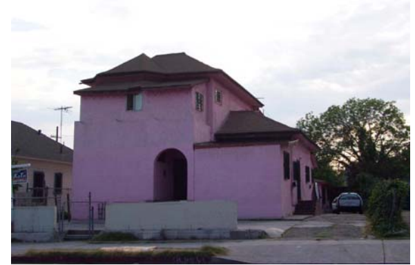
This home has been stripped of most of its original architectural features resulting in a blighting effect on the surrounding neighborhood.
