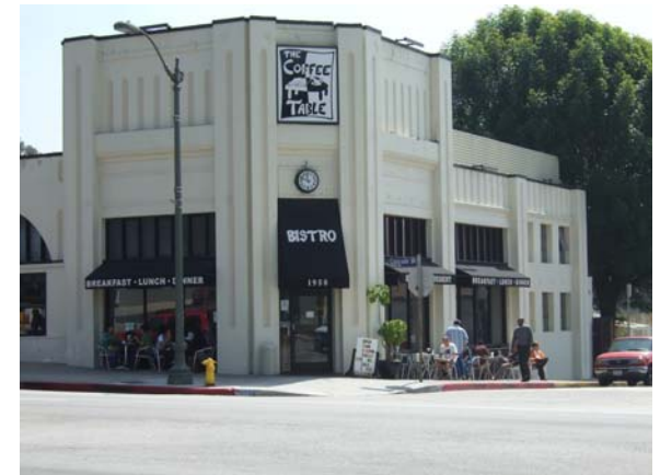
Signage that is simple and complementary to building architecture effectively communicates a professional look that is beneficial to the business and the District.
