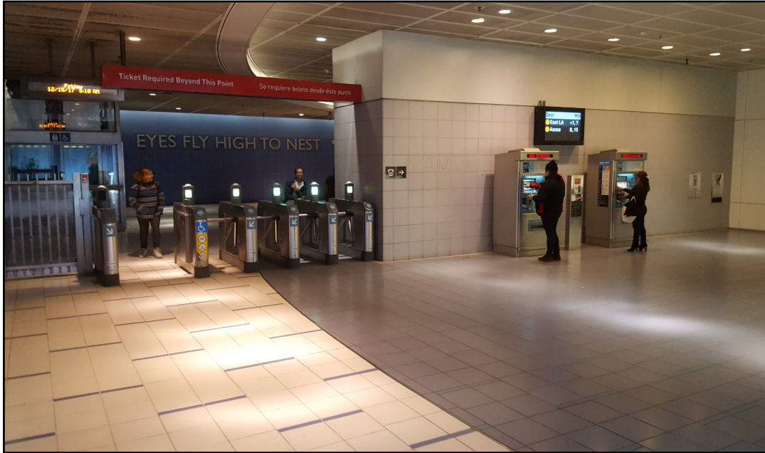
Photo 7— Interior of subsurface subway station (Soto Station) beneath the E. 1st Street parcels.
