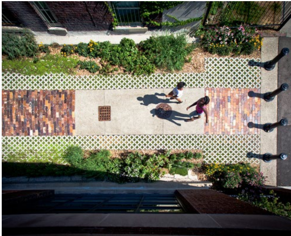
Green Alley with Turf Block Paving
