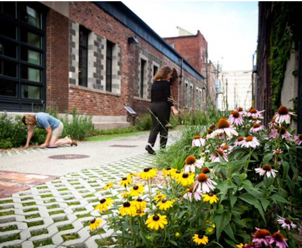
Green Alley with Turf Block Paving
