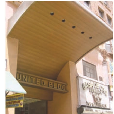
United Building shown as example of rehabilitated lighting fixtures.
