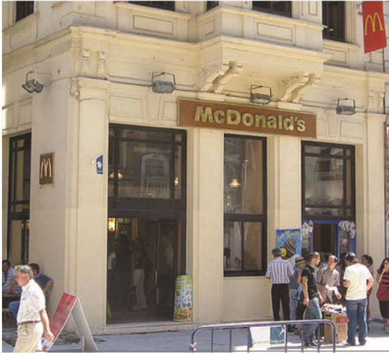
Corporate establishments should be designed to comply fully with the design guidelines and development standards.
