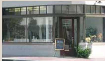
The window sash located above a door. Also called transom light.
