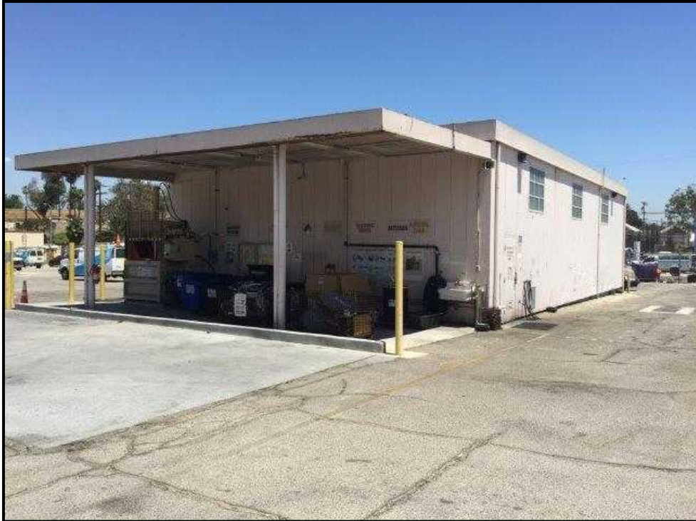
5. Maintenance building near the center of the Subject Property.
