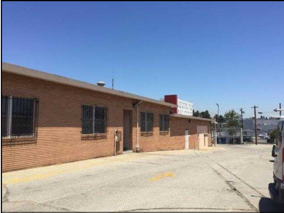
1. Southwest side of the main building on the Subject Property.
