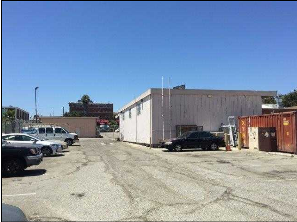
7. East side of the maintenance building.
