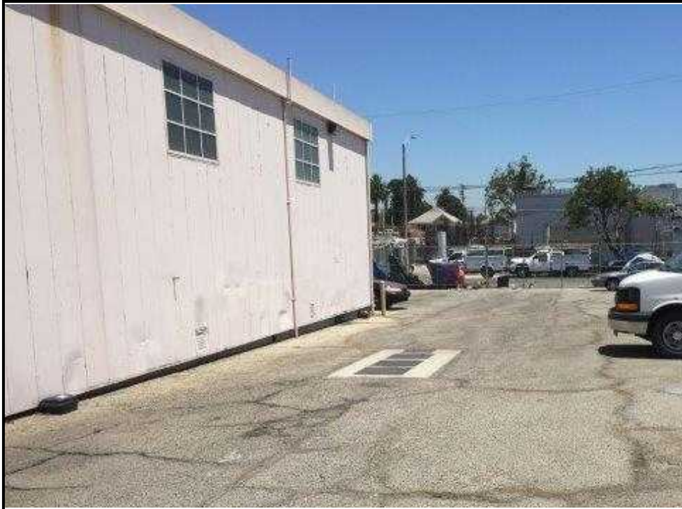
11. Oil/water separator south of the maintenance building.
