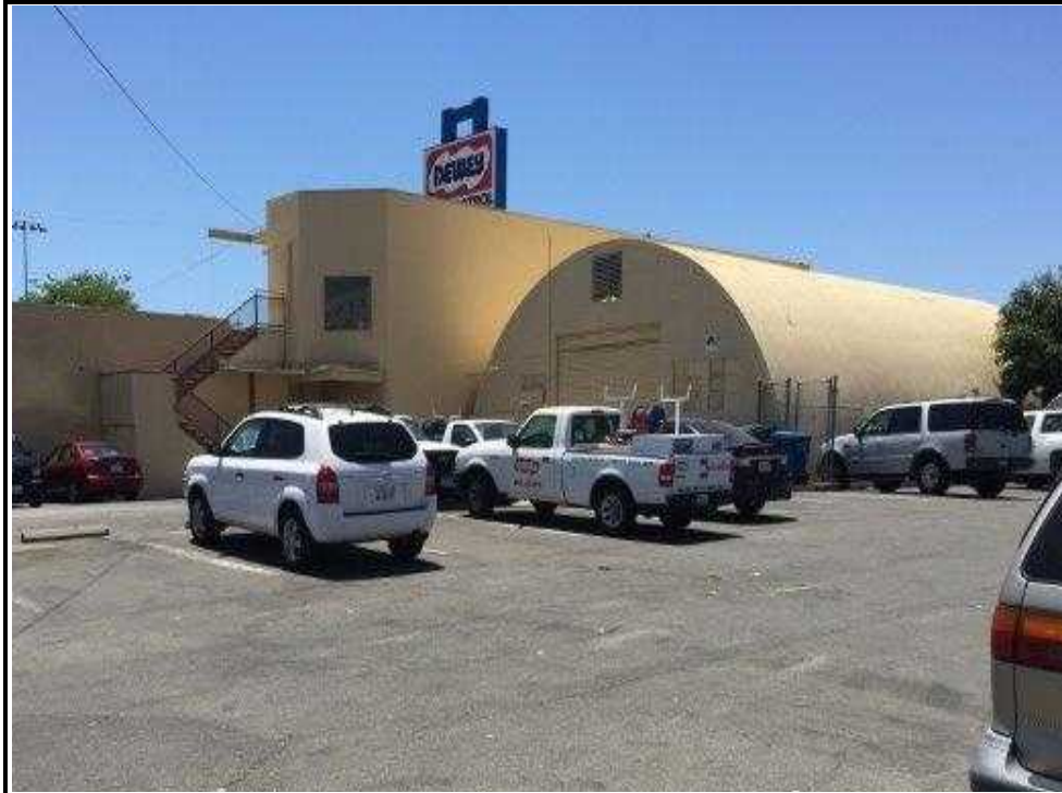
27. Dewey Pest Control south of the Subject Property.
