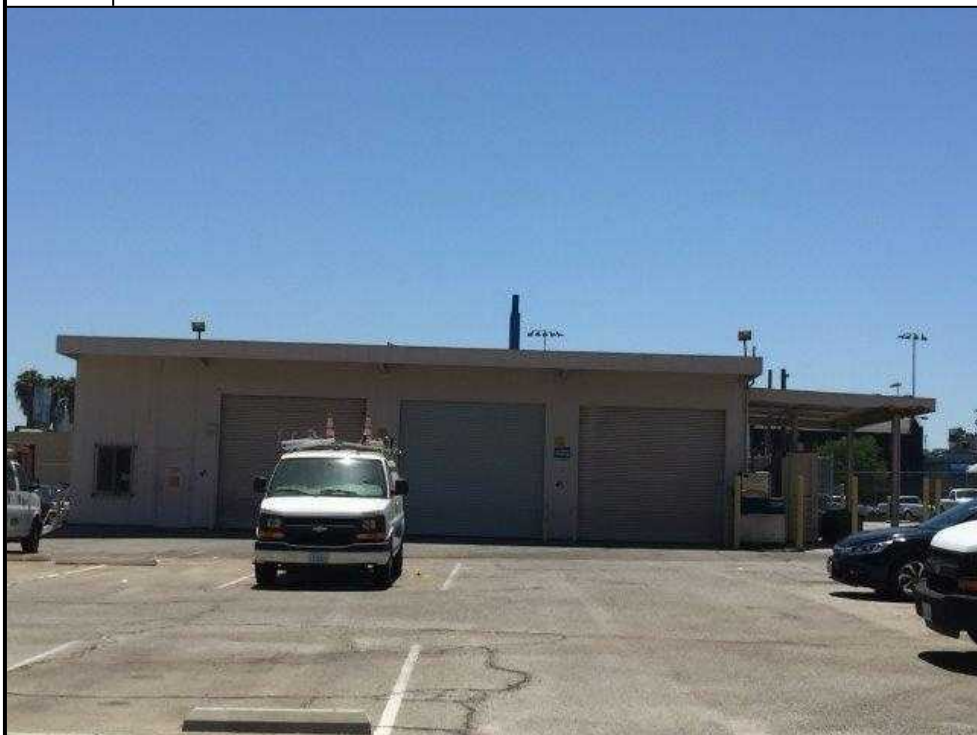
6. North side of the maintenance building.
