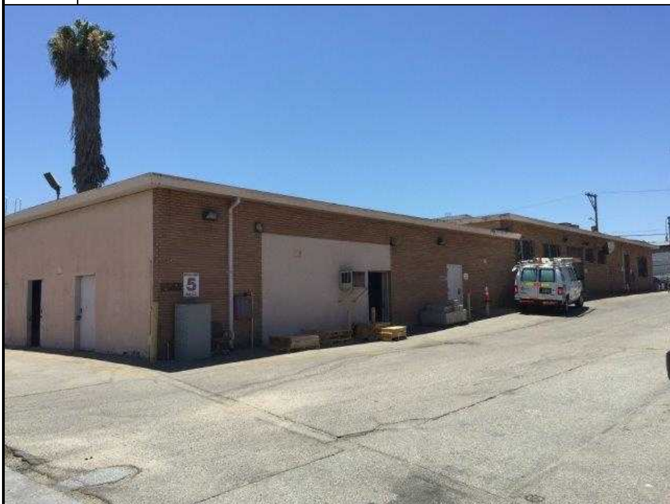
4. East side of the main building.,
