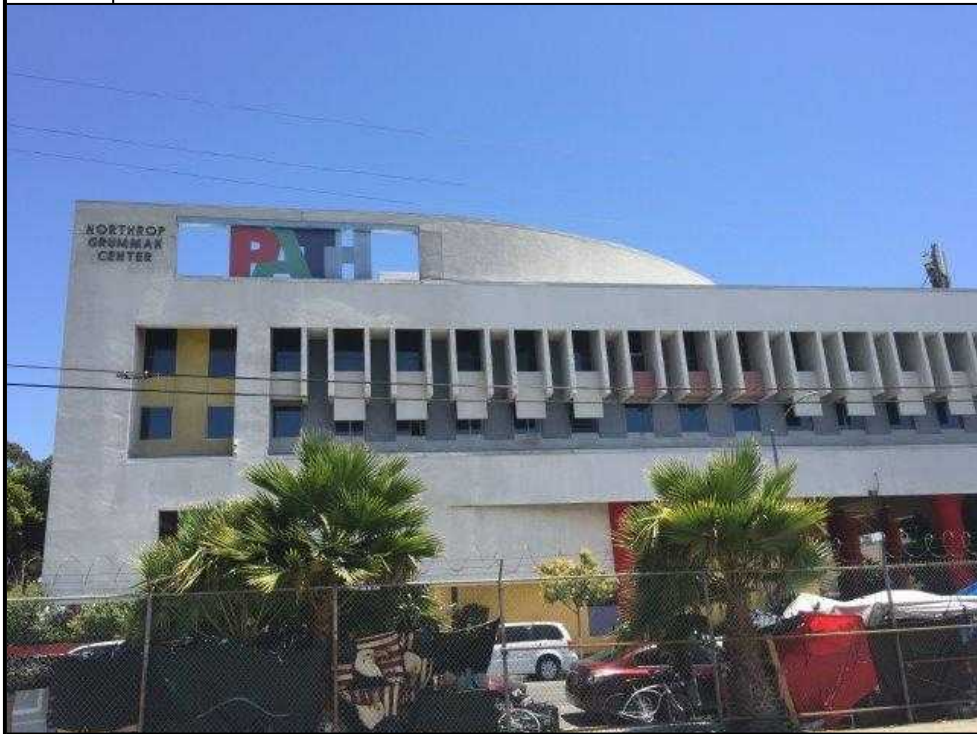
34. Northrup Grumman Center beyond homeless encampment to the east.
