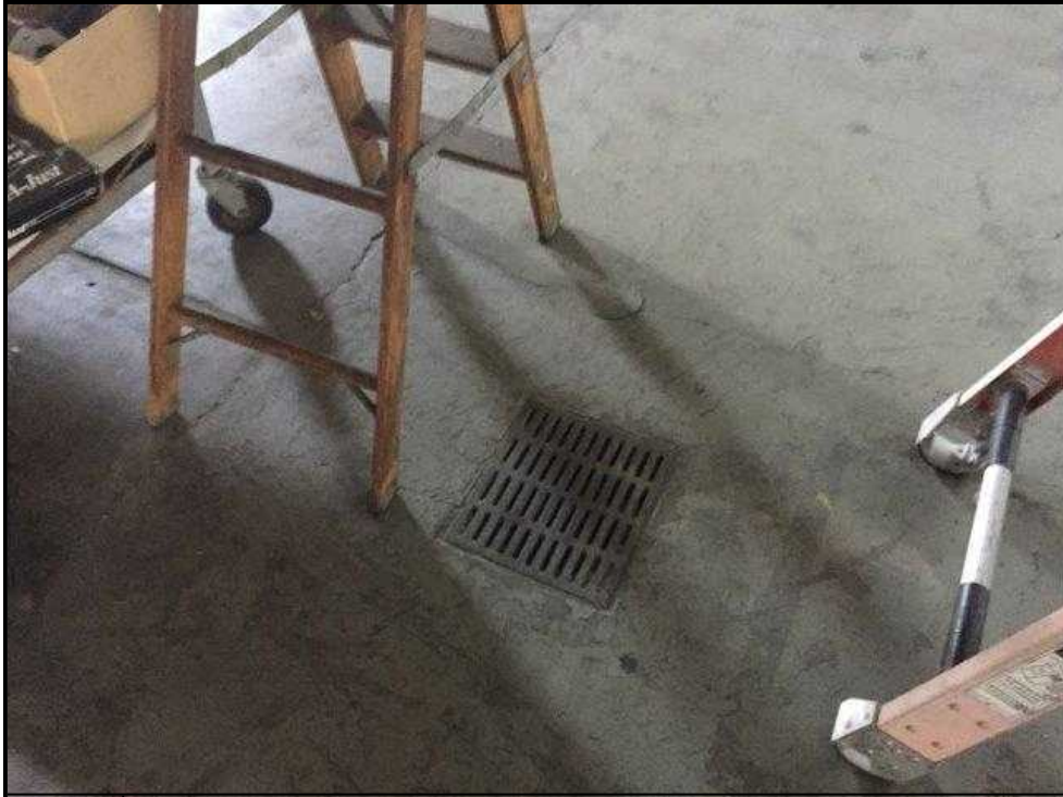
19. Floor drain inside maintenance building.
