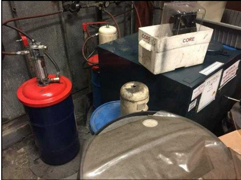
17. Product oil AST and small drums of oil inside maintenance building.
