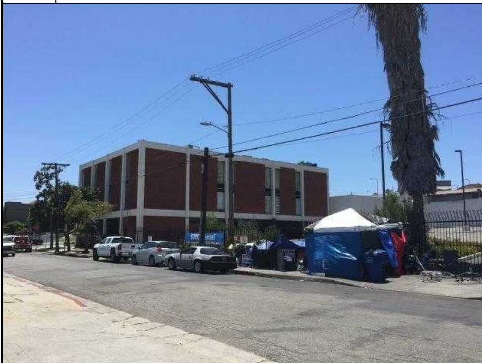
32. Parking lot associated with office building to the west.
