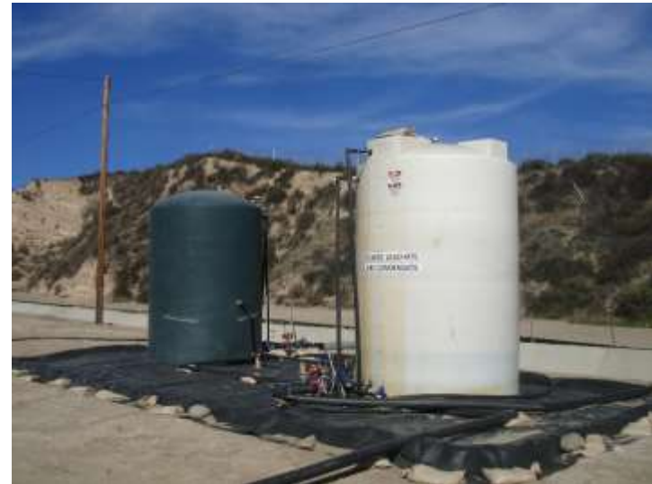
Photo 150: Old City North Treated Leachate and Condensate Holding Tanks: January 7, 2015
