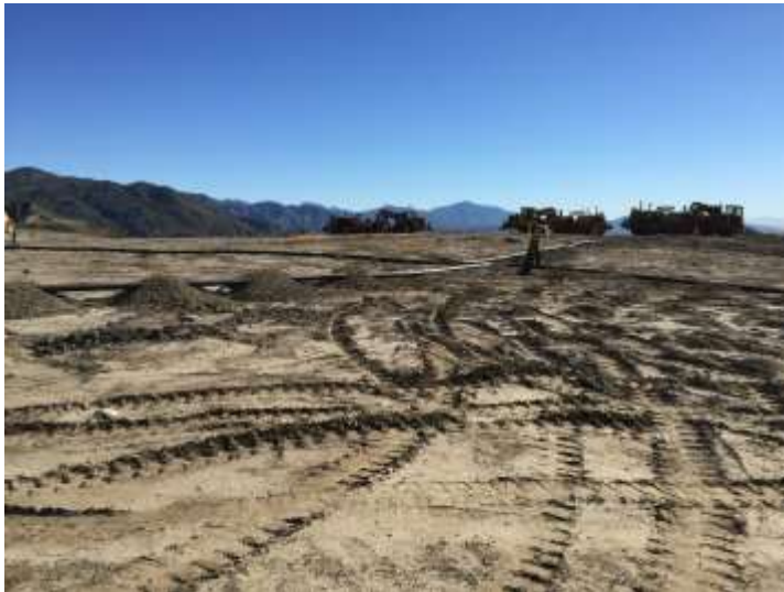
Photo 105: Parked Equipment with No Oil Drip Pans: February 13, 2015
