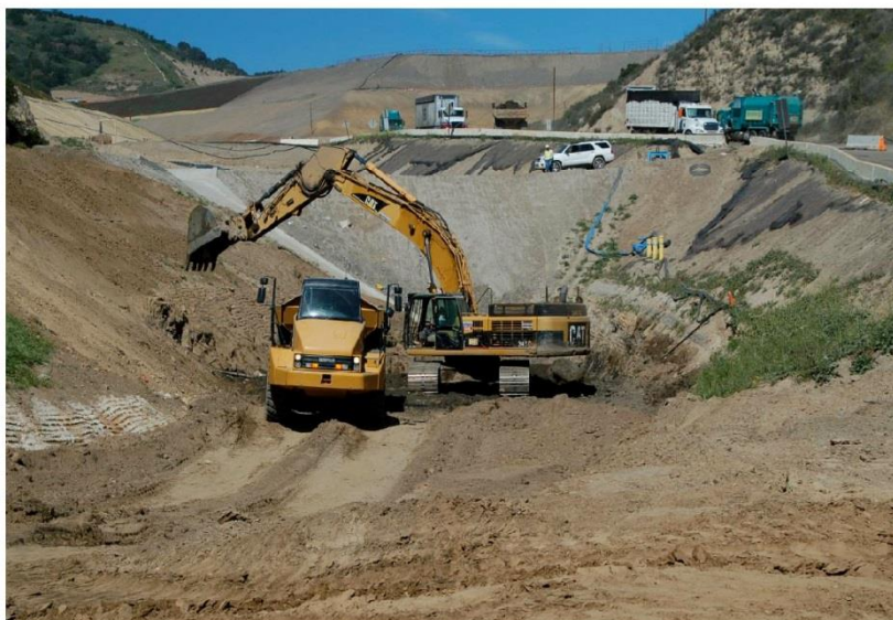
Photo 2: Cleaning of alluvial material
