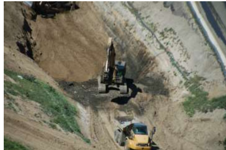
Photo 208: Alluvial Soils Removal Near Temporary Basins: March 24, 2015
