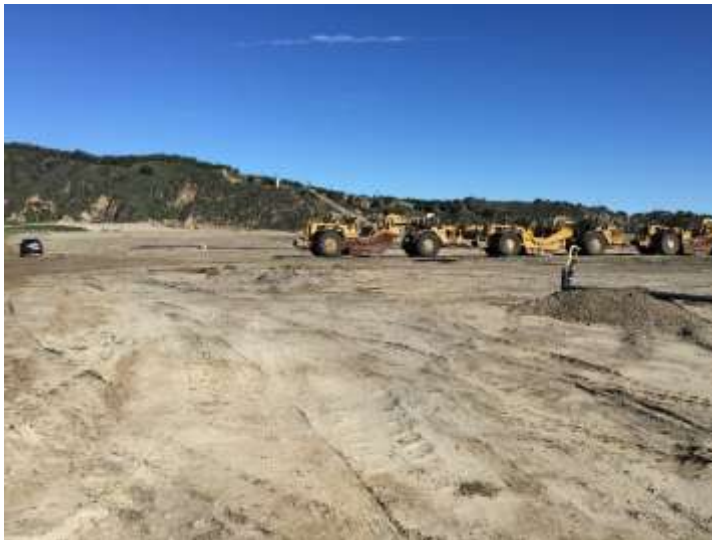
Photo 103: Parked Equipment with No Oil Drip Pans: February 13, 2015
