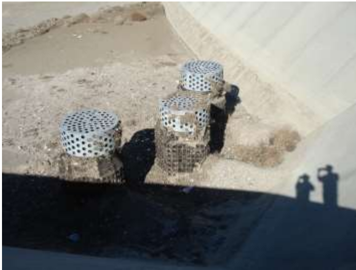
Photo 141: Terminal Basin Outlet Risers: January 7, 2015
