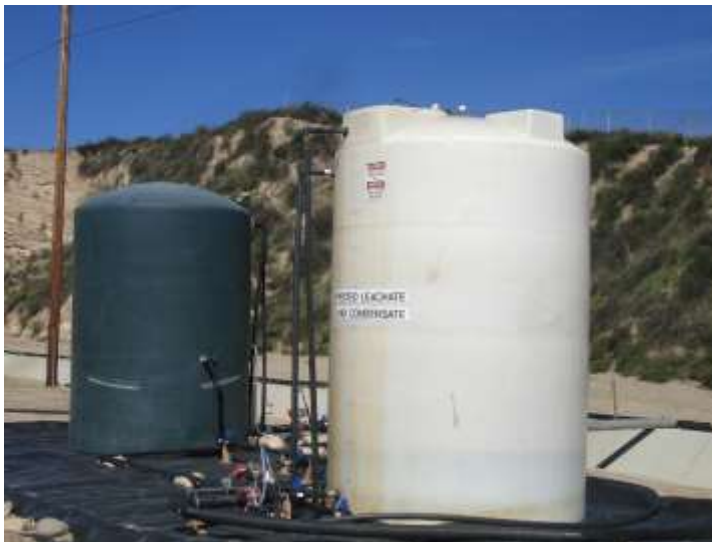
Photo 151: Old City North Treated Leachate and Condensate Holding Tanks: February 13, 2015
