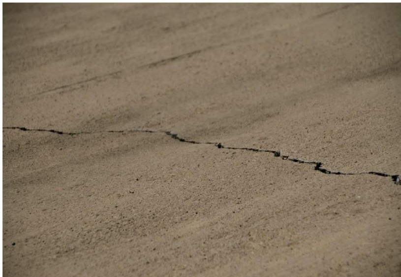
Photo 4: Crack on outside face of terminal basin
