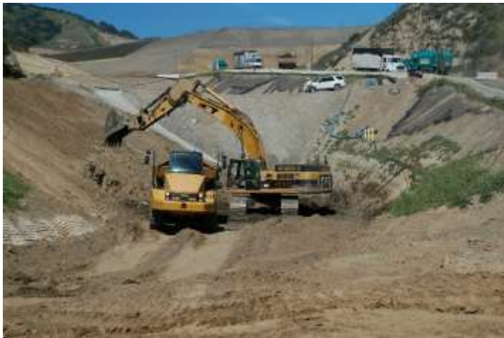
Photo 207: Alluvial Soils Removal Near Temporary Basins: March 24, 2015
