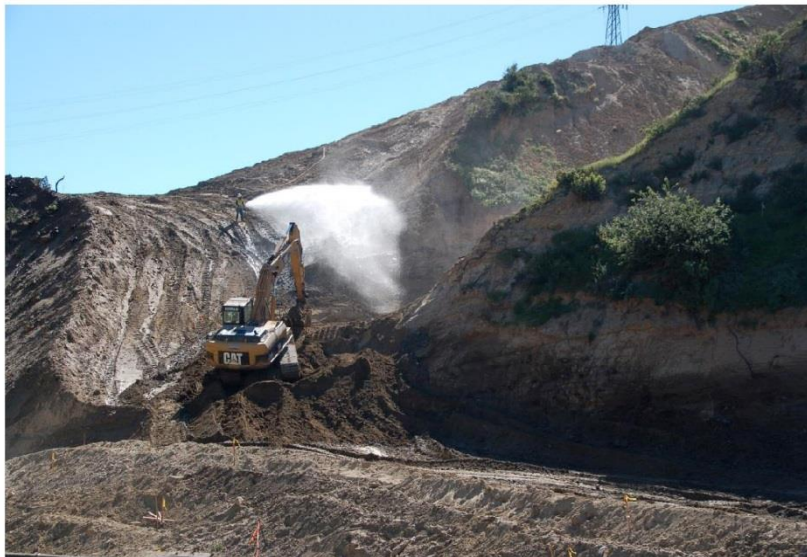
Photo 1: Use of water to moisture condition soil and control dust
