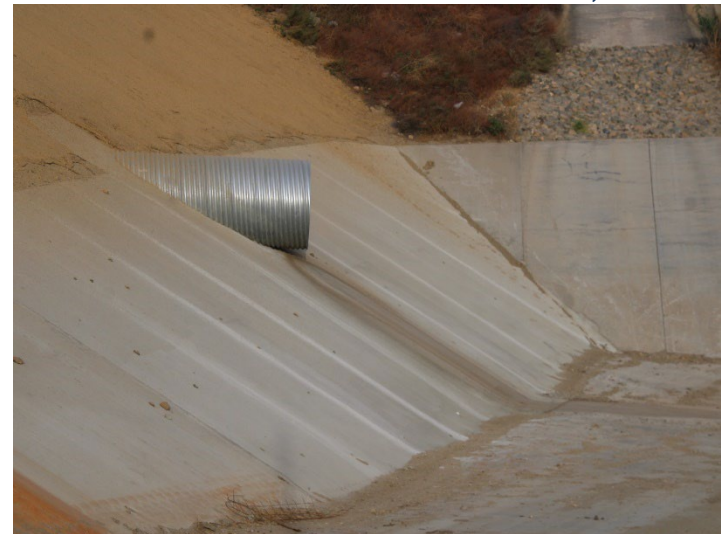
Photo 340: Terminal Basin: December 11, 2024
