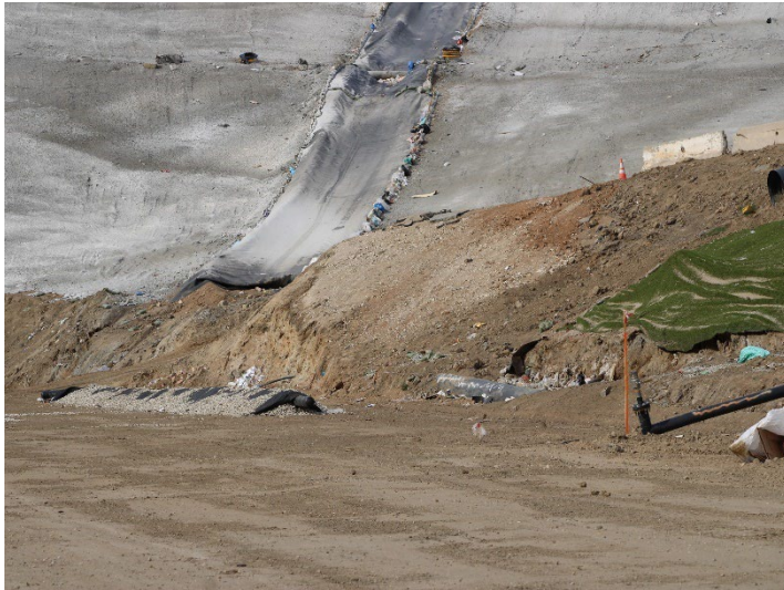
Photo 525: General Site: December 11, 2024
