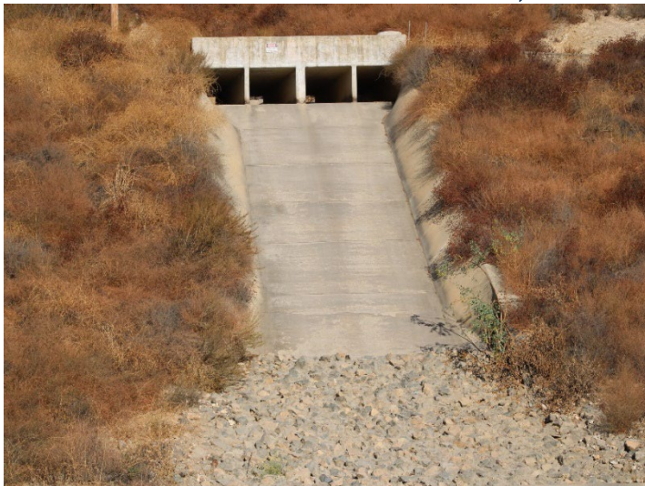
Photo 299: Terminal Basin: October 31, 2024
