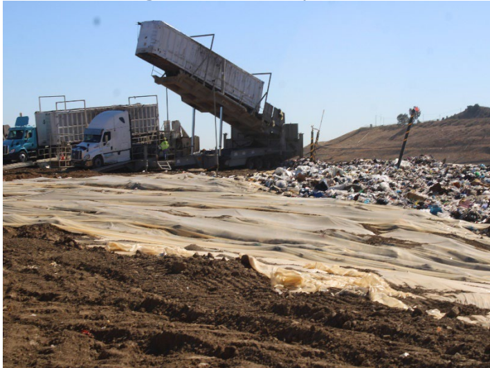
Photo 63: Working Area, CC4 Part 1/2: November 20, 2024
