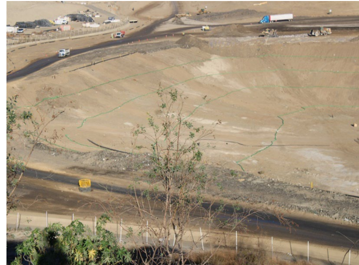
Photo 146: Working Area, CC4 Part 4/5: October 31, 2024
