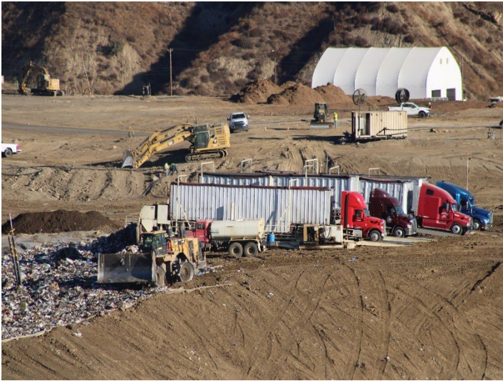
Photo 125: Working Area, CC4 Part 3: October 31, 2024
