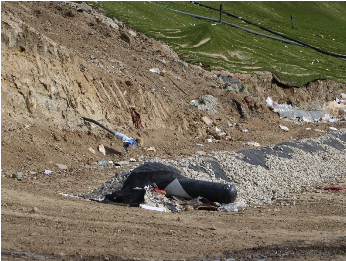
Photo 537: General Site: December 11, 2024
