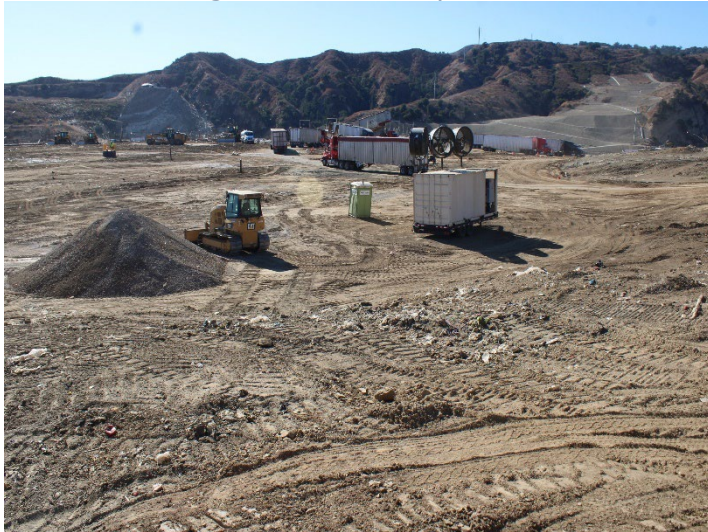
Photo 31: Working Area, CC4 Part 1/2: November 20, 2024
