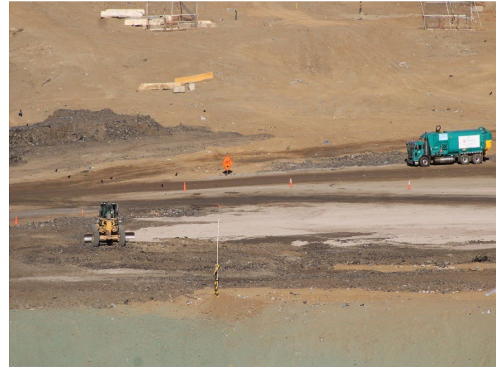
Photo 182: Working Area, CC4 Part 4/5: November 20, 2024
