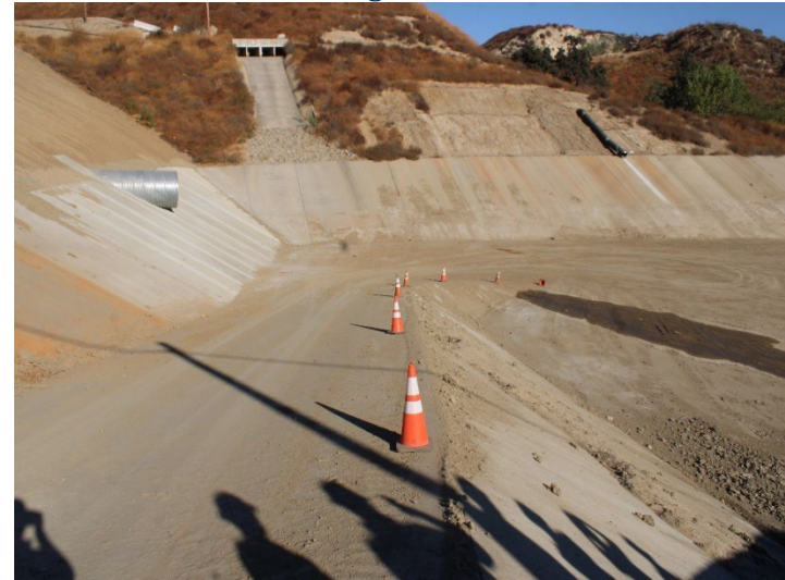
Photo 292: Terminal Basin: October 31, 2024
