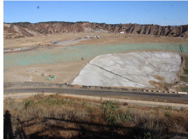
Photo 162: Working Area, CC4 Part 4/5: November 20, 2024
