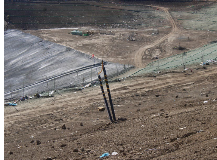
Photo 60: Working Area, CC4 Part 1/2: November 20, 2024
