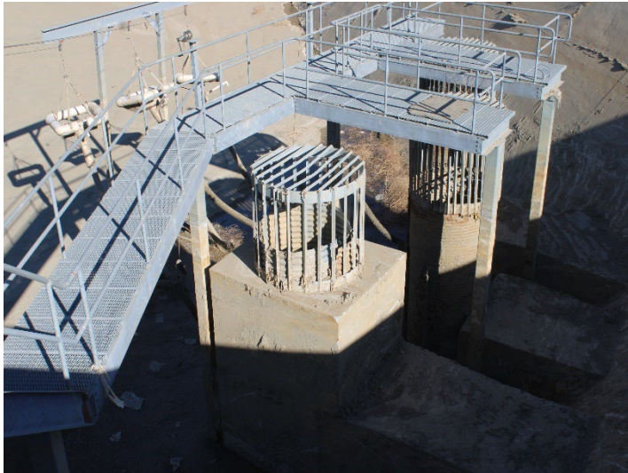
Photo 321: Terminal Basin: November 20, 2024
