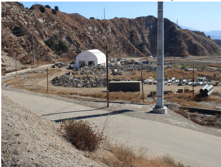
Photo 403: General Site: October 31, 2024
