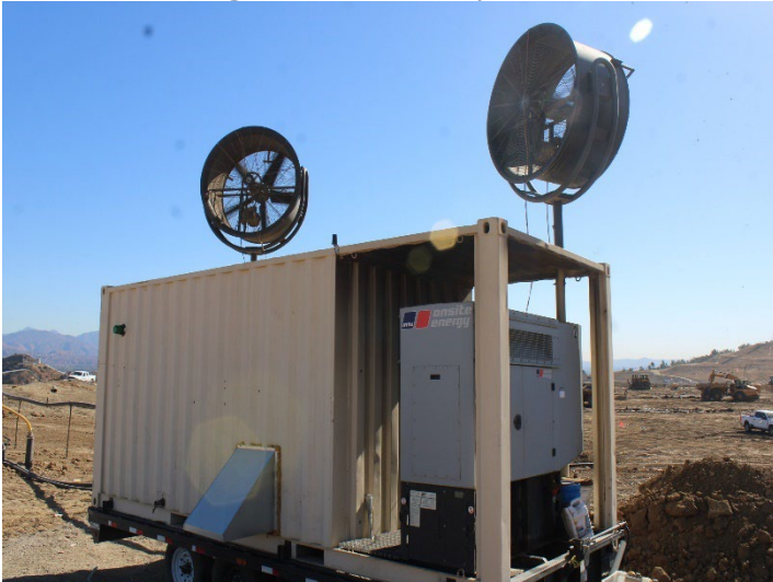
Photo 27: Working Area, CC4 Part 1/2: November 20, 2024
