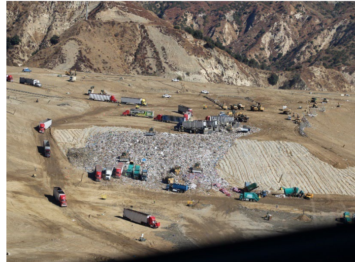
Photo 74: Working Area, CC4 Part 1/2: November 20, 2024
