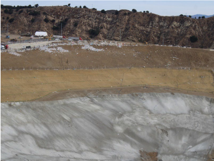
Photo 193: Working Area, CC4 Part 4/5: December 11, 2024
