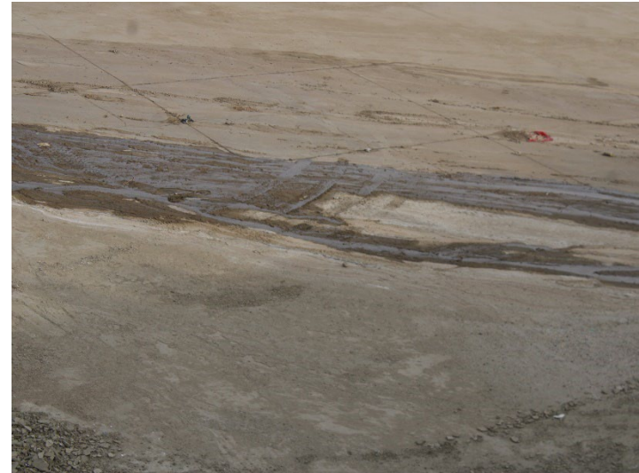
Photo 342: Terminal Basin: December 11, 2024
