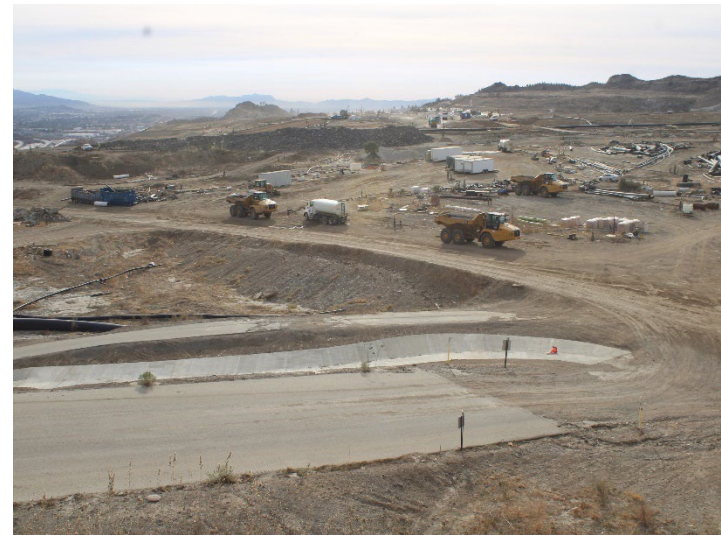
Photo 506: General Site: December 11, 2024
