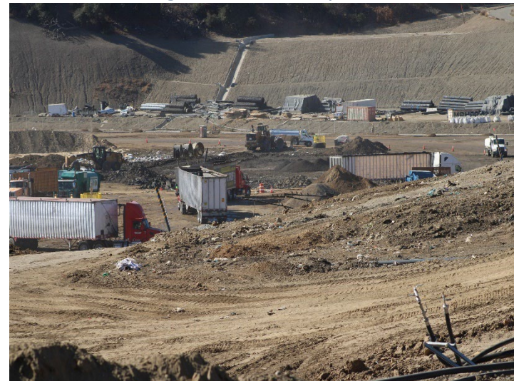
Photo 12: Working Area, CC4 Part 1/2: October 31, 2024
