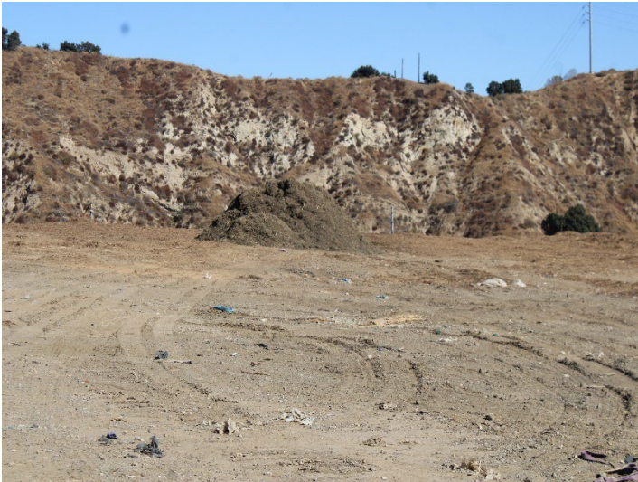
Photo 25: Working Area, CC4 Part 1/2: November 20, 2024
