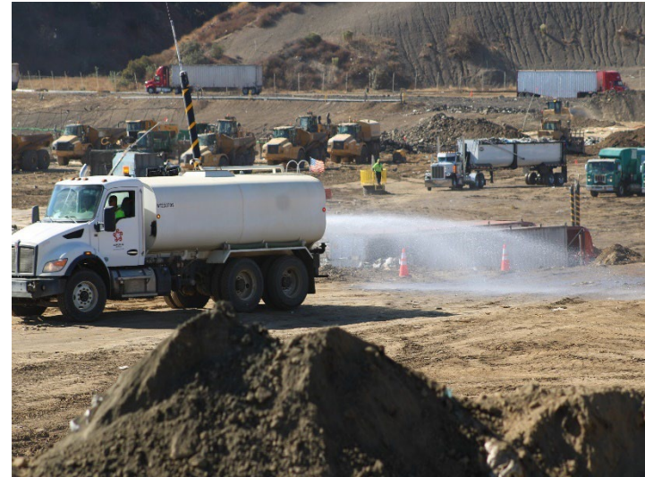
Photo 14: Working Area, CC4 Part 1/2: October 31, 2024
