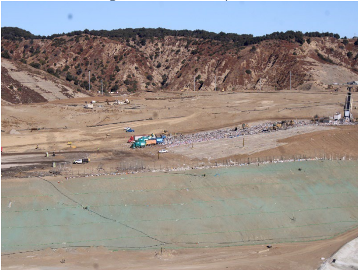
Photo 167: Working Area, CC4 Part 4/5: November 20, 2024
