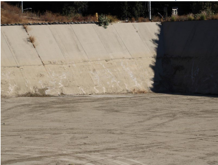
Photo 295: Terminal Basin: October 31, 2024
