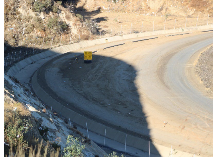
Photo 170: Working Area, CC4 Part 4/5: November 20, 2024
