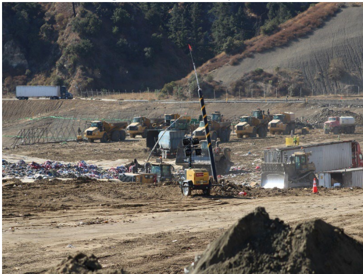
Photo 11: Working Area, CC4 Part 1/2: October 31, 2024
