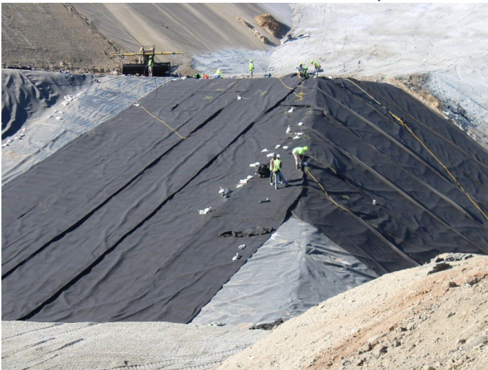
Photo 379: General Site: October 31, 2024
