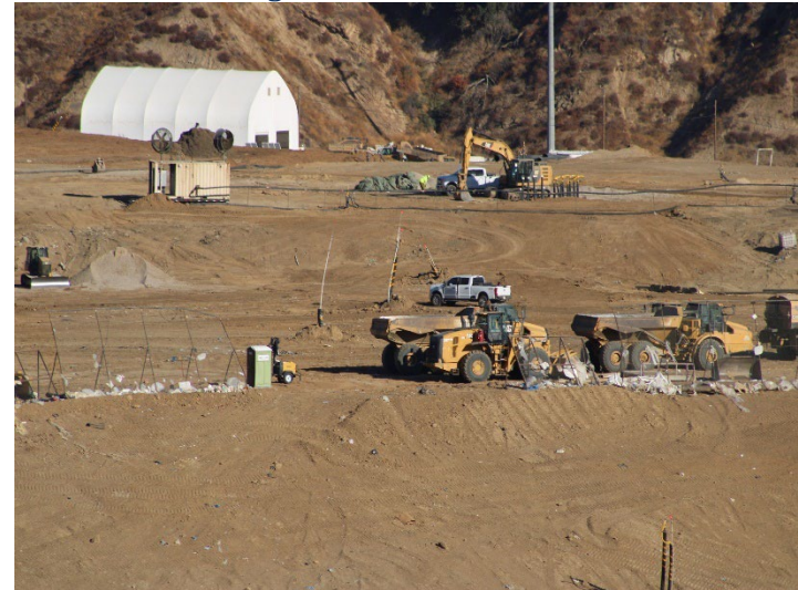
Photo 136: Working Area, CC4 Part 3: November 20, 2024
