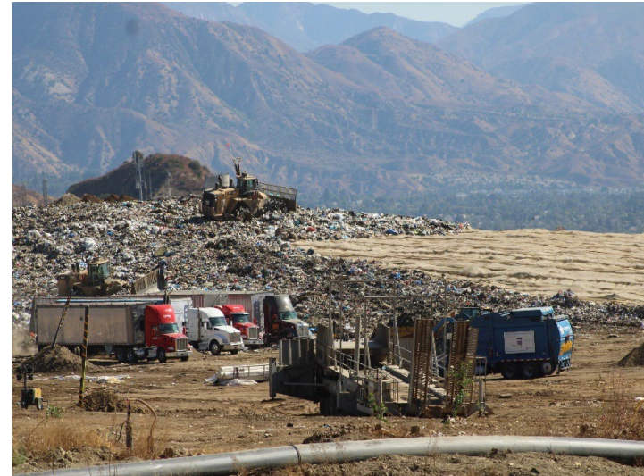
Photo 18: Working Area, CC4 Part 1/2: October 31, 2024
