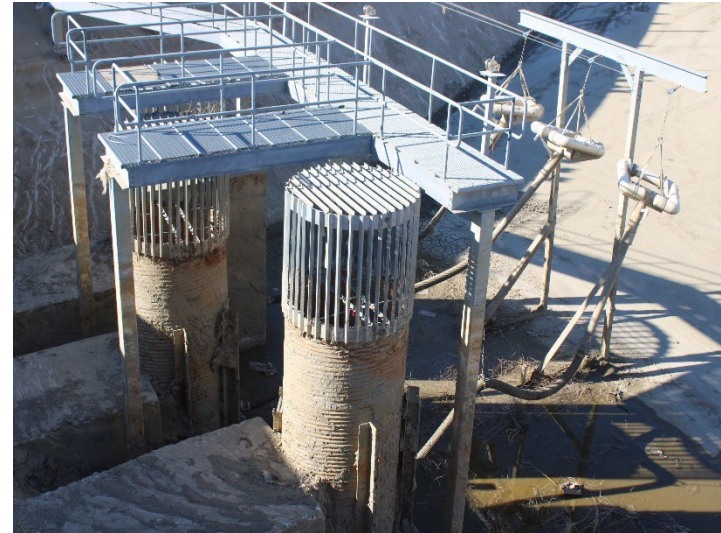
Photo 322: Terminal Basin: November 20, 2024
