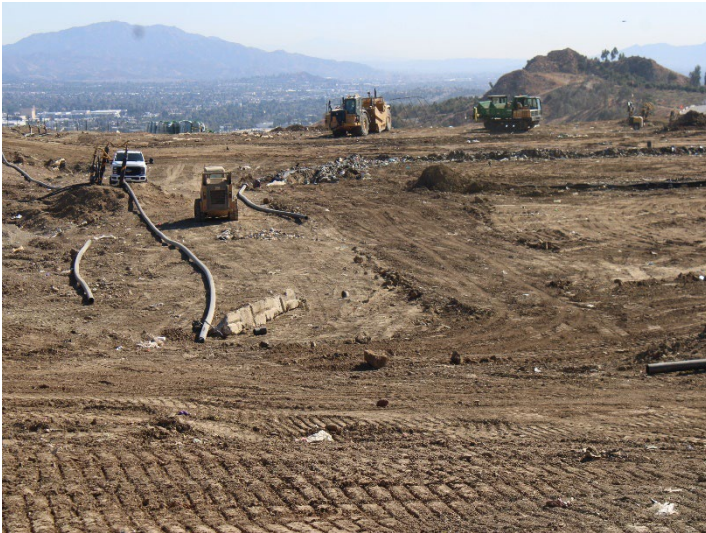
Photo 33: Working Area, CC4 Part 1/2: November 20, 2024
