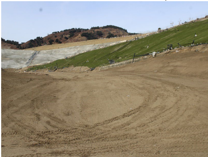
Photo 519: General Site: December 11, 2024
