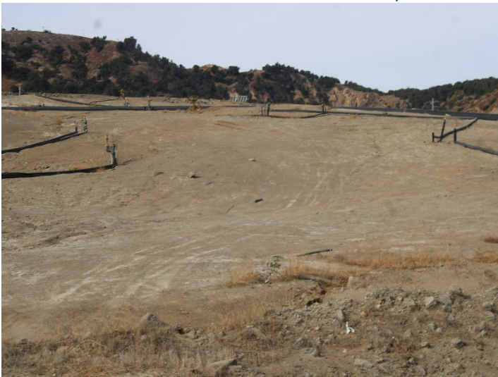
Photo 503: General Site: December 11, 2024
