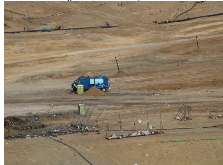
Photo 76: Working Area, CC4 Part 1/2: December 11, 2024
