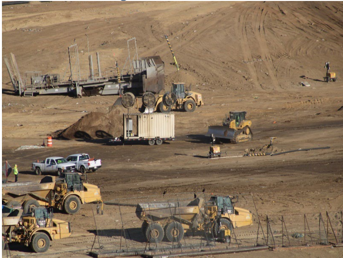
Photo 119: Working Area, CC4 Part 3: October 31, 2024
