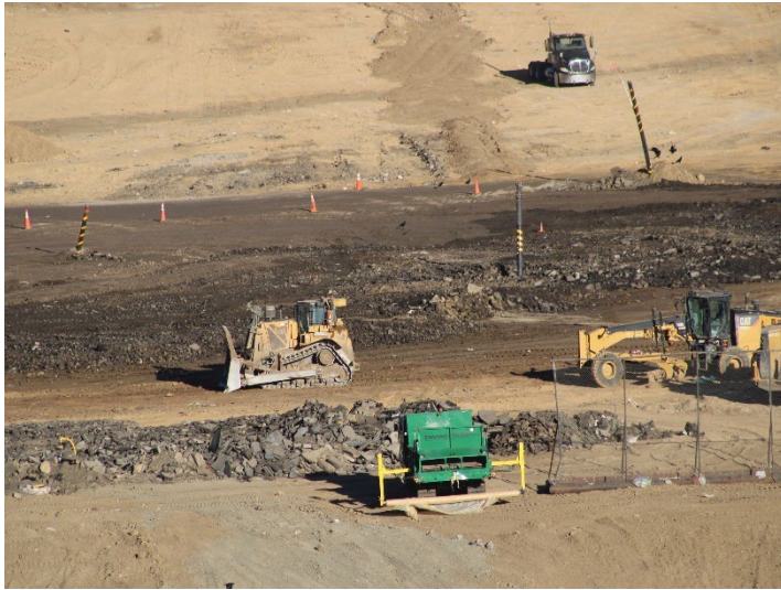
Photo 117: Working Area, CC4 Part 3: October 31, 2024
