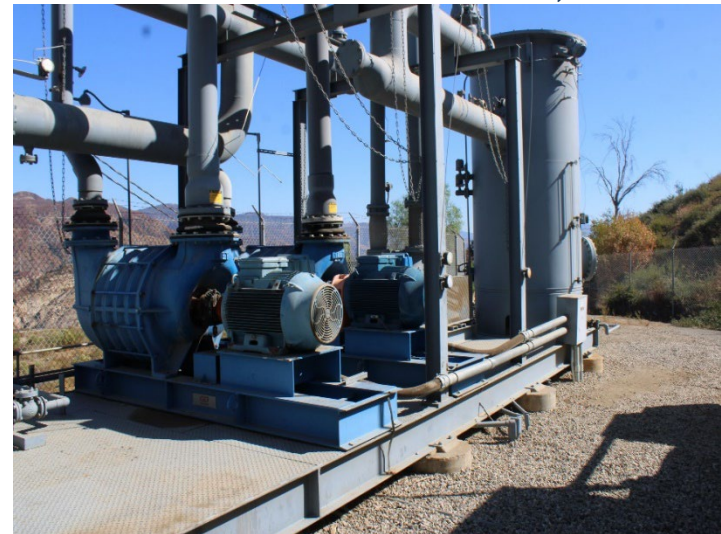
Photo 420: General Site: October 31, 2024
