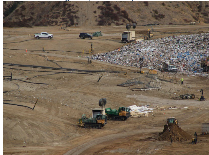
Photo 112: Working Area, CC4 Part 1/2: December 11, 2024
