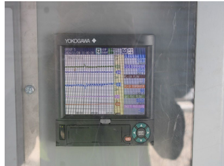
Photo 242: Flares 9, 10, 11 and Gas-to-Energy Facility: November 20, 2024
