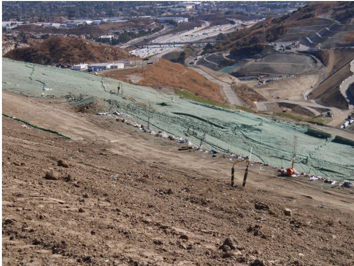
Photo 57: Working Area, CC4 Part 1/2: November 20, 2024
