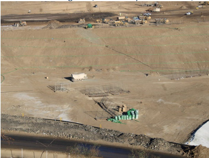
Photo 147: Working Area, CC4 Part 4/5: October 31, 2024
