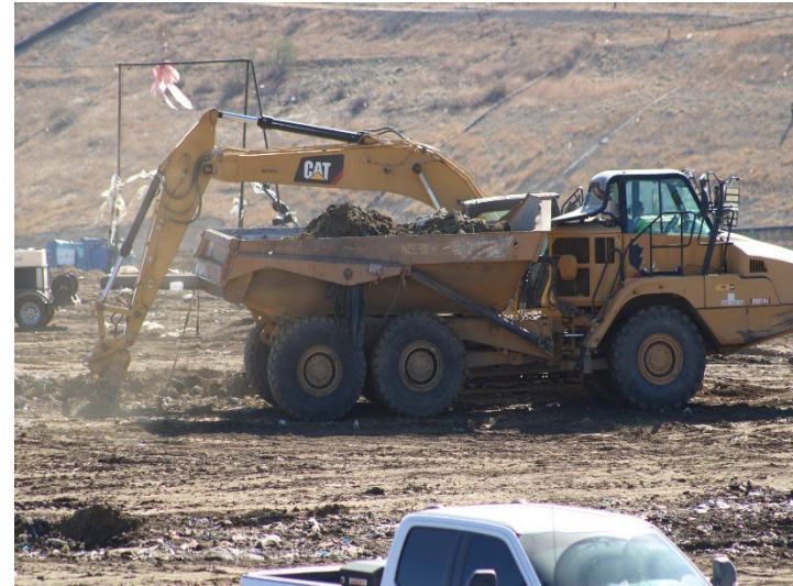
Photo 46: Working Area, CC4 Part 1/2: November 20, 2024
