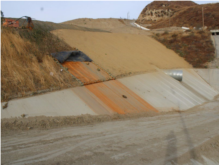
Photo 335: Terminal Basin: December 11, 2024
