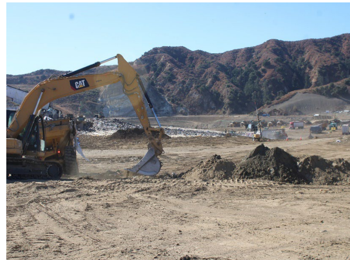
Photo 8: Working Area, CC4 Part 1/2: October 31, 2024
