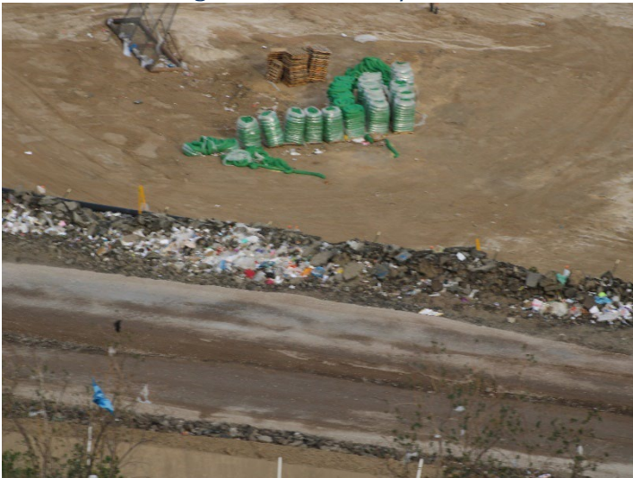
Photo 195: Working Area, CC4 Part 4/5: December 11, 2024
