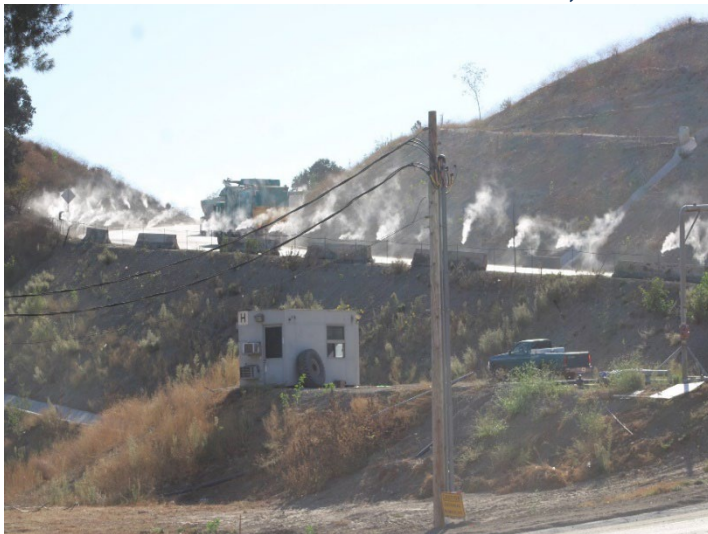
Photo 303: Terminal Basin: October 31, 2024
