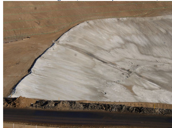
Photo 148: Working Area, CC4 Part 4/5: October 31, 2024
