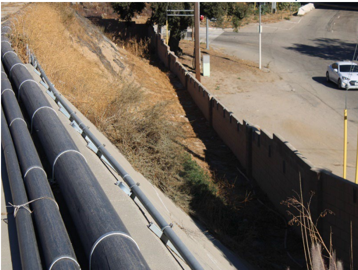
Photo 327: Terminal Basin: November 20, 2024
