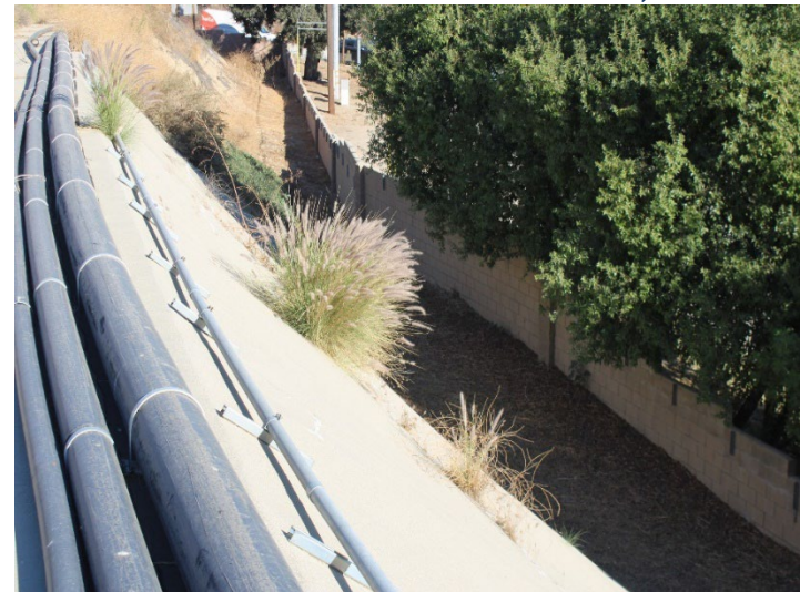
Photo 308: Terminal Basin: October 31, 2024
