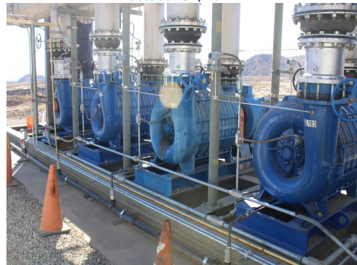
Photo 228: Flares 9, 10, 11 and Gas-to-Energy Facility: October 31, 2024
