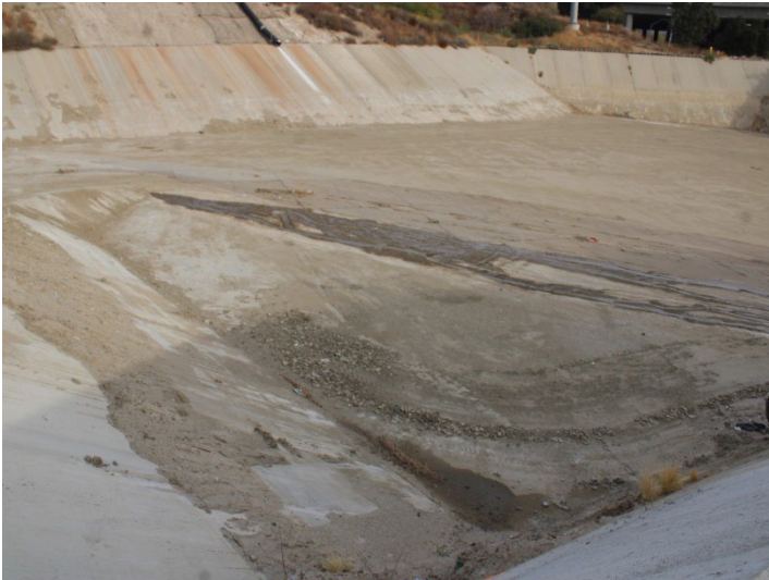
Photo 337: Terminal Basin: December 11, 2024
