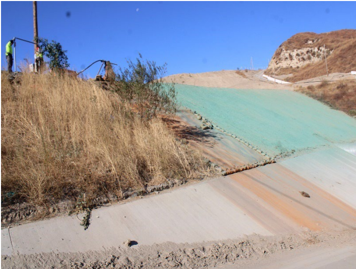
Photo 313: Terminal Basin: November 20, 2024
