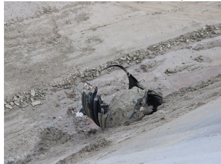
Photo 344: Terminal Basin: December 11, 2024
