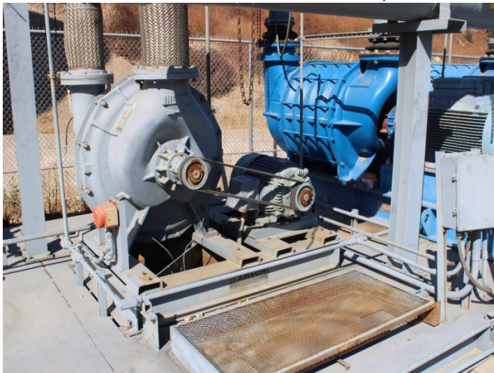
Photo 415: General Site: October 31, 2024
