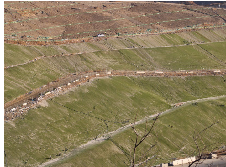
Photo 202: Closure Turf: October 31, 2024
