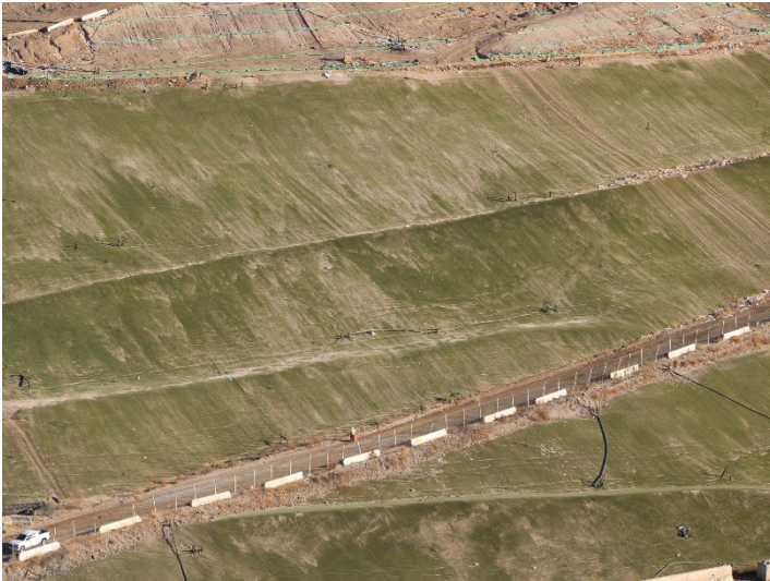
Photo 201: Closure Turf: October 31, 2024
