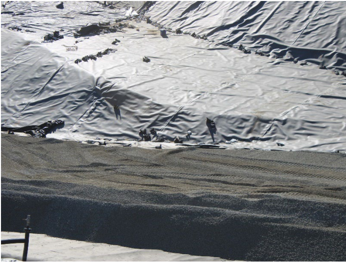
Photo 377: General Site: October 31, 2024
