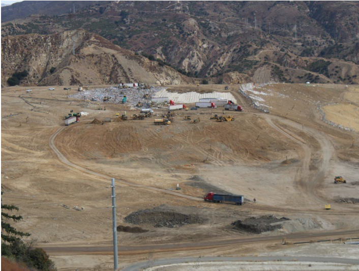
Photo 557: General Site: December 11, 2024
