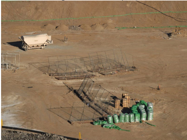
Photo 151: Working Area, CC4 Part 4/5: October 31, 2024
