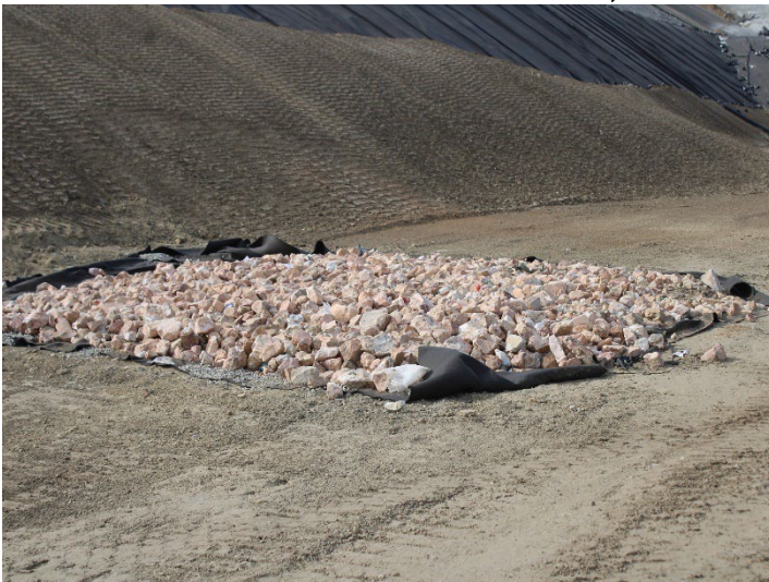
Photo 523: General Site: December 11, 2024
