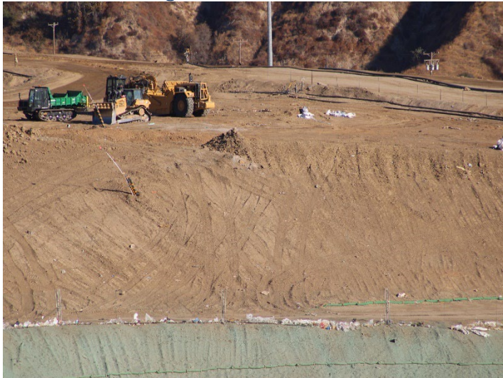
Photo 139: Working Area, CC4 Part 3: November 20, 2024
