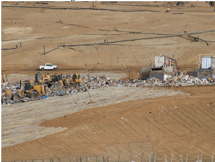
Photo 131: Working Area, CC4 Part 3: November 20, 2024
