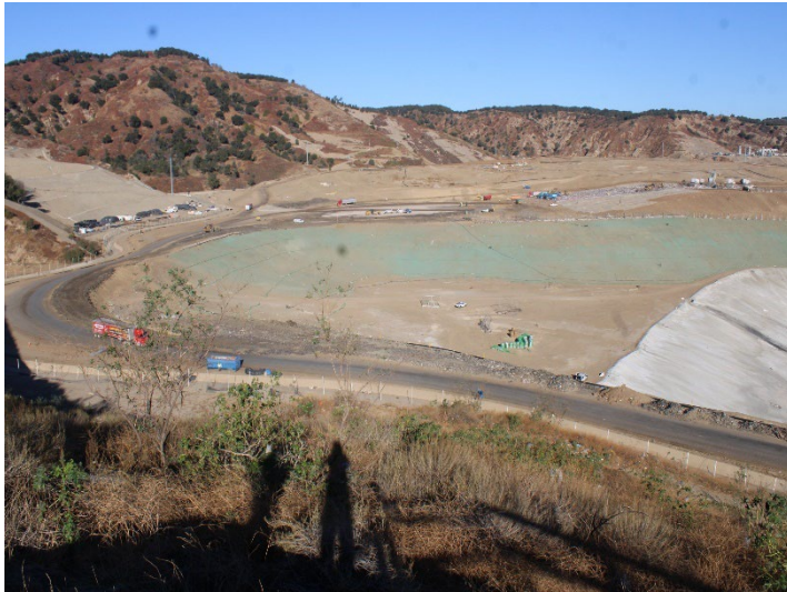
Photo 161: Working Area, CC4 Part 4/5: November 20, 2024
