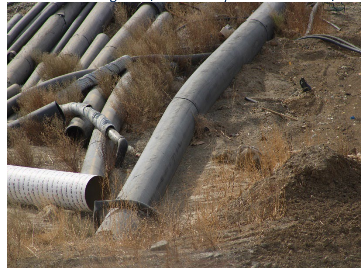
Photo 92: Working Area, CC4 Part 1/2: December 11, 2024
