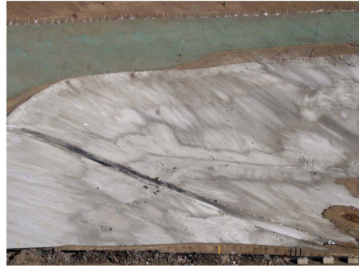
Photo 166: Working Area, CC4 Part 4/5: November 20, 2024
