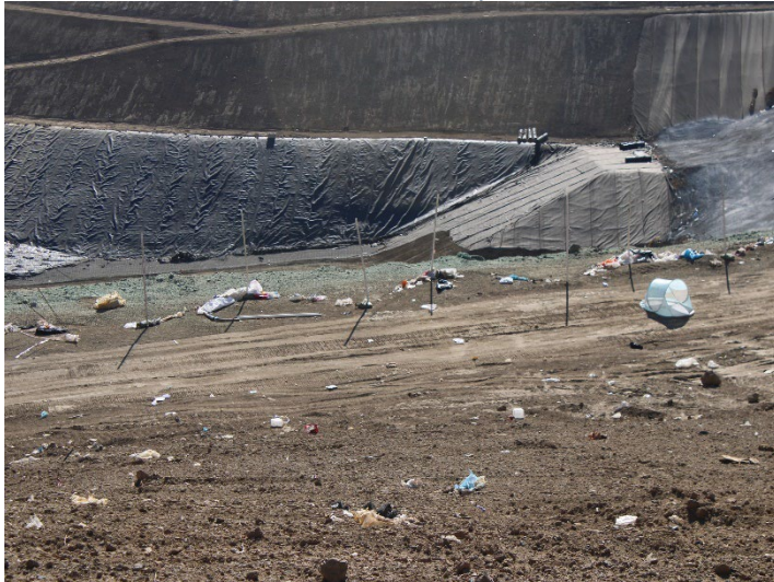
Photo 59: Working Area, CC4 Part 1/2: November 20, 2024
