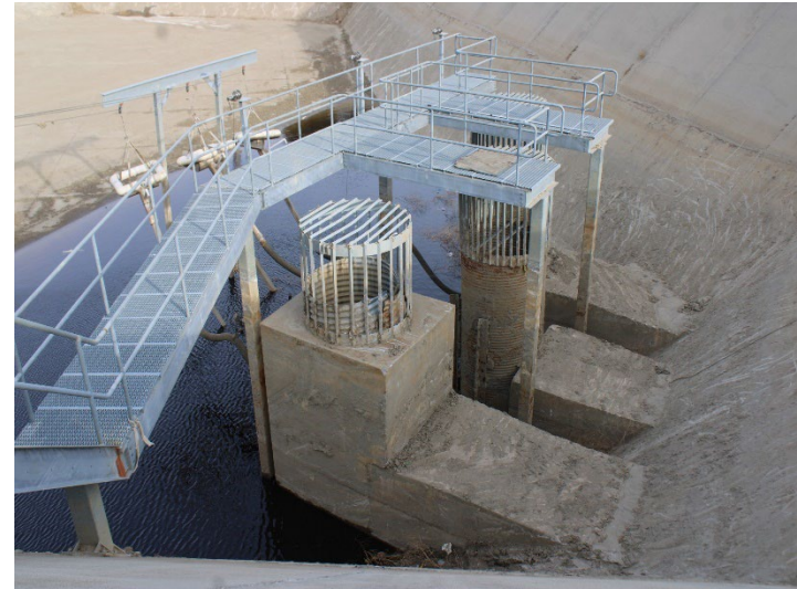
Photo 346: Terminal Basin: December 11, 2024
