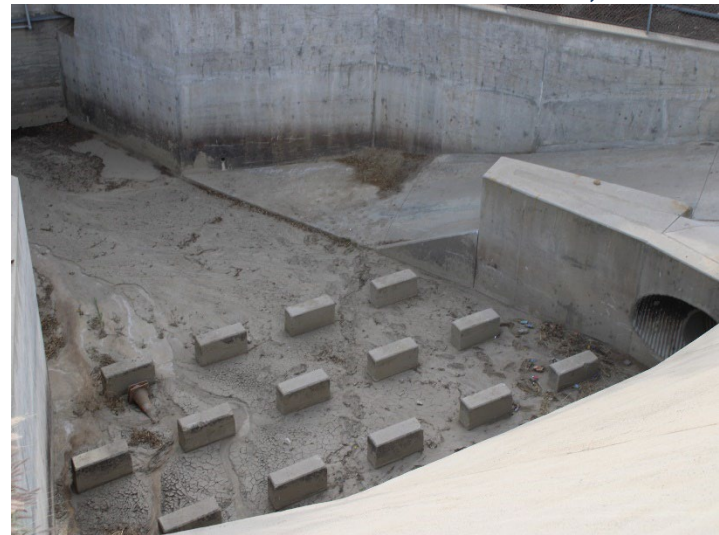
Photo 352: Terminal Basin: December 11, 2024
