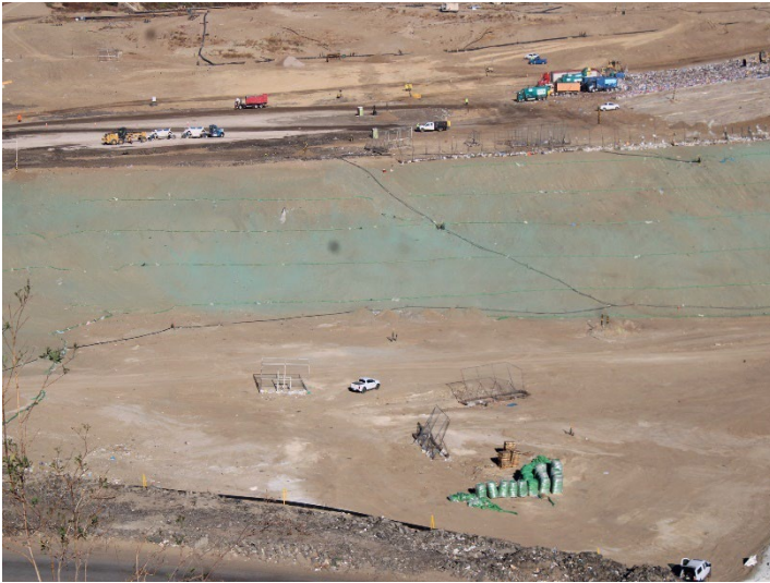
Photo 165: Working Area, CC4 Part 4/5: November 20, 2024
