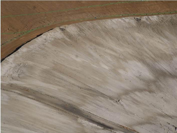
Photo 153: Working Area, CC4 Part 4/5: October 31, 2024
