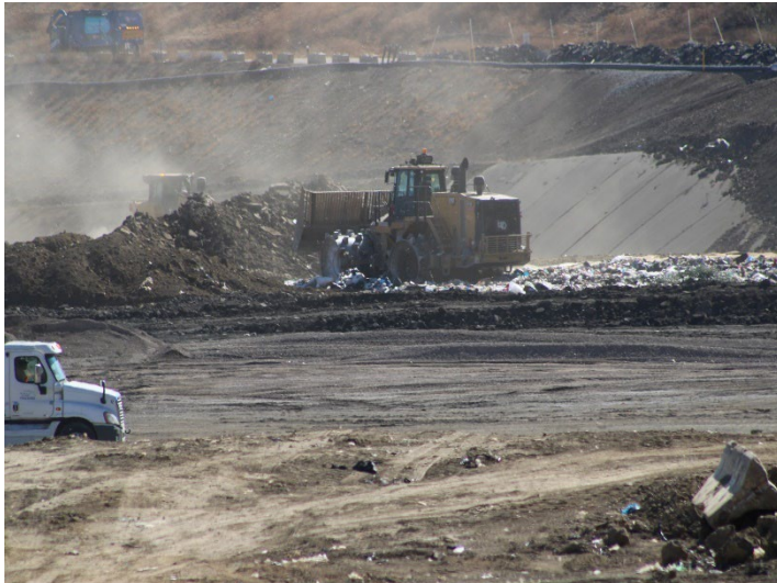
Photo 21: Working Area, CC4 Part 1/2: October 31, 2024
