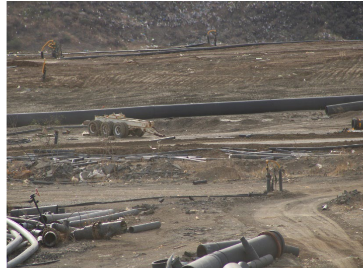
Photo 90: Working Area, CC4 Part 1/2: December 11, 2024
