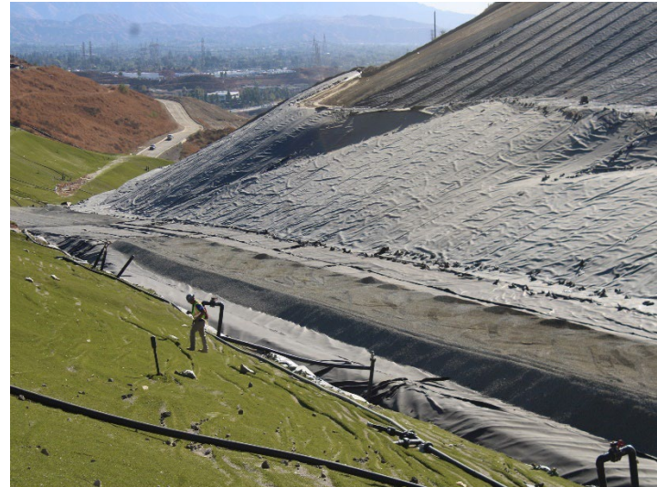
Photo 376: General Site: October 31, 2024
