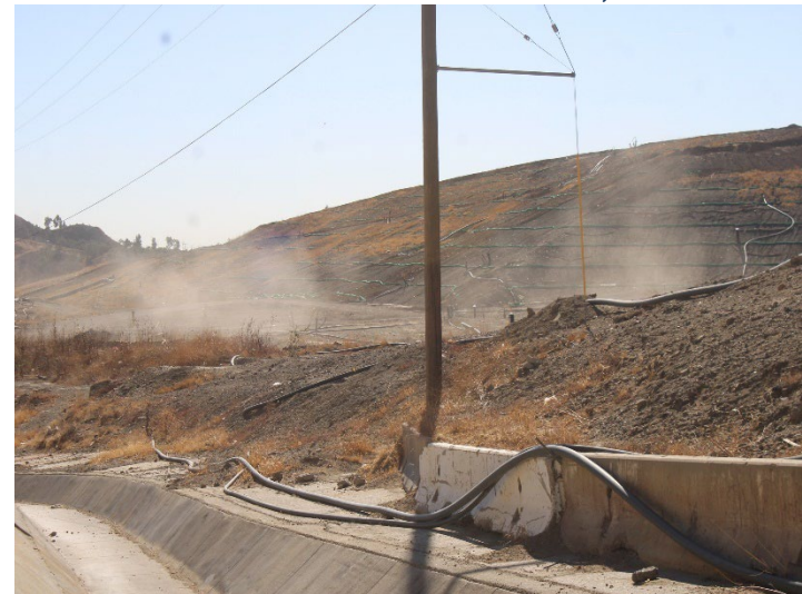
Photo 288: Eastside Drainage Channel: November 20, 2024
