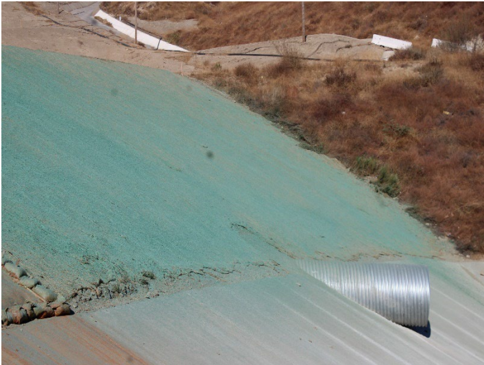
Photo 317: Terminal Basin: November 20, 2024
