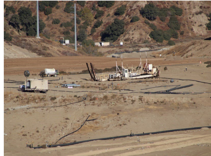
Photo 140: Working Area, CC4 Part 3: November 20, 2024
