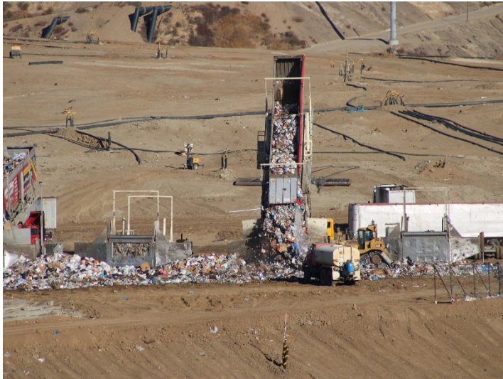
Photo 141: Working Area, CC4 Part 3: November 20, 2024
