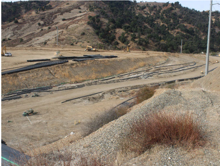
Photo 509: General Site: December 11, 2024
