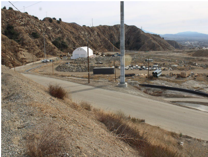
Photo 505: General Site: December 11, 2024
