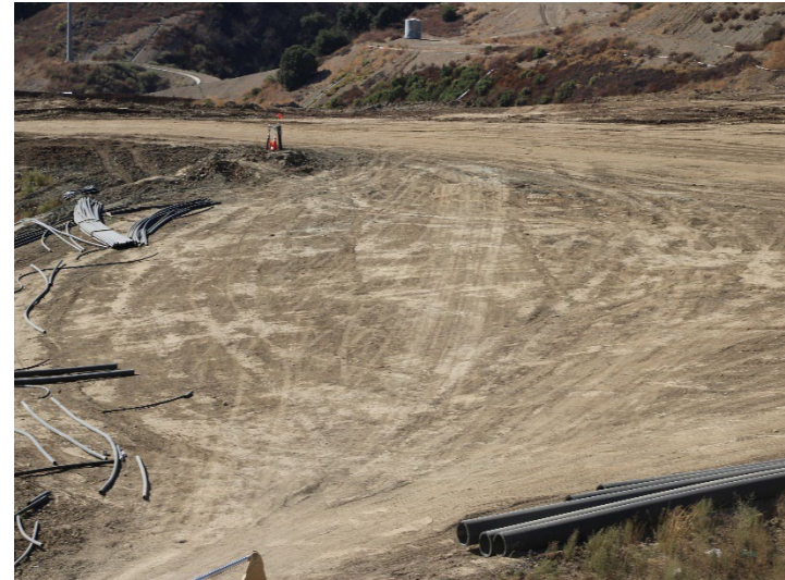
Photo 262: County Top Deck: October 31, 2024
