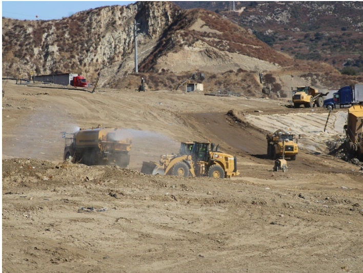
Photo 69: Working Area, CC4 Part 1/2: November 20, 2024
