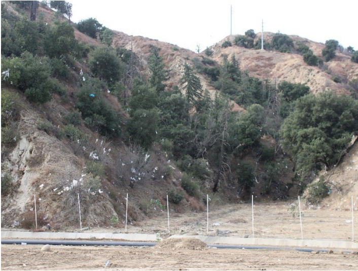
Photo 549: General Site: December 11, 2024
