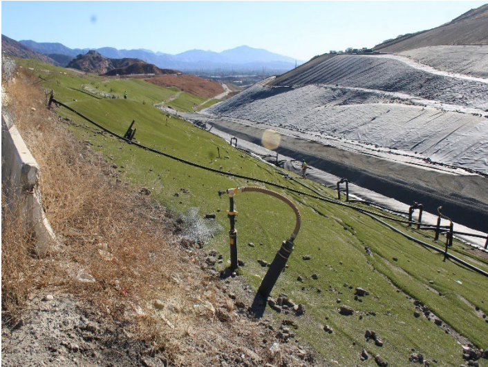
Photo 373: General Site: October 31, 2024
