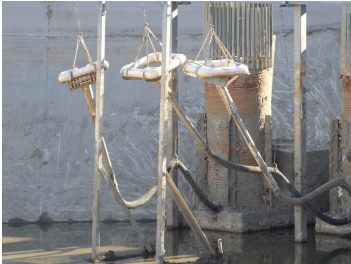
Photo 297: Terminal Basin: October 31, 2024
