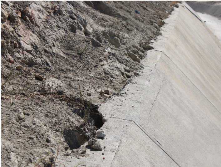
Photo 289: Eastside Drainage Channel: November 20, 2024
