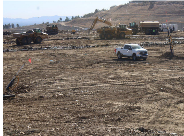
Photo 34: Working Area, CC4 Part 1/2: November 20, 2024
