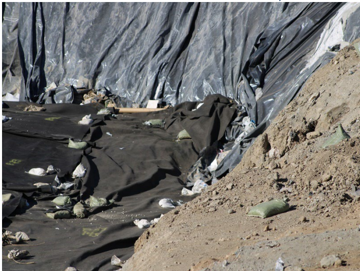
Photo 395: General Site: October 31, 2024
