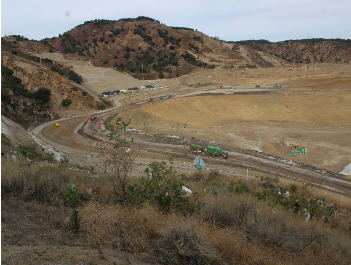
Photo 183: Working Area, CC4 Part 4/5: December 11, 2024
