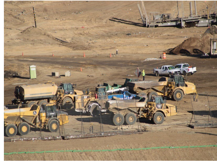
Photo 118: Working Area, CC4 Part 3: October 31, 2024
