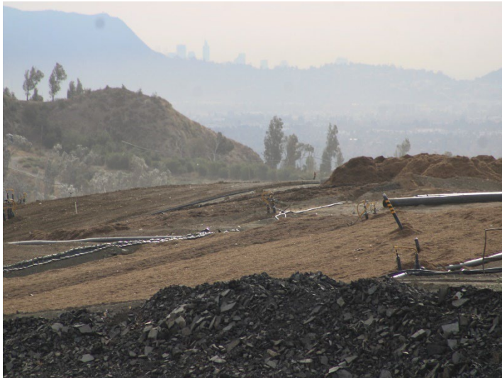
Photo 85: Working Area, CC4 Part 1/2: December 11, 2024
