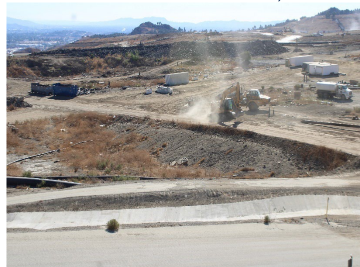
Photo 404: General Site: October 31, 2024
