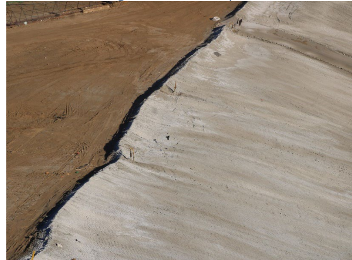
Photo 152: Working Area, CC4 Part 4/5: October 31, 2024
