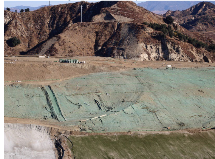
Photo 180: Working Area, CC4 Part 4/5: November 20, 2024
