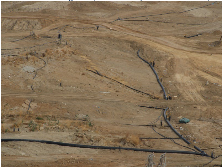
Photo 111: Working Area, CC4 Part 1/2: December 11, 2024
