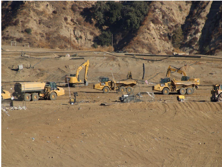
Photo 137: Working Area, CC4 Part 3: November 20, 2024
