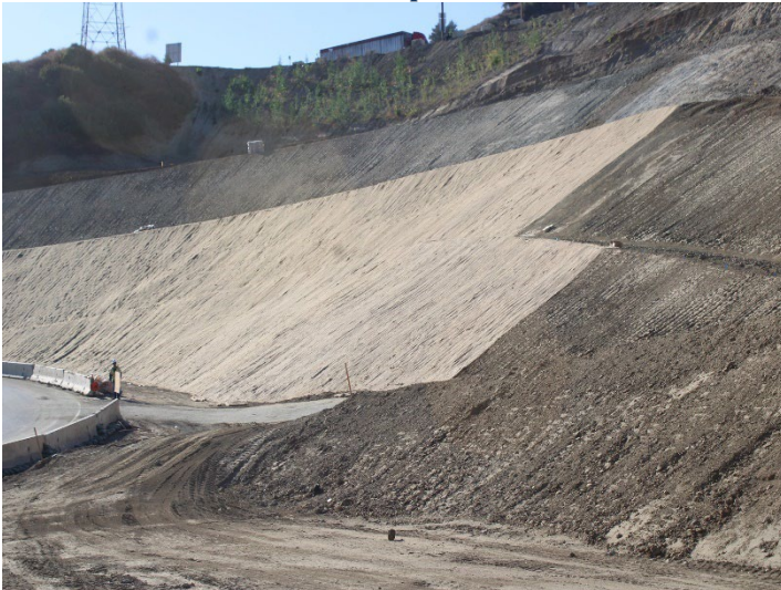
Photo 371: General Site: October 31, 2024
