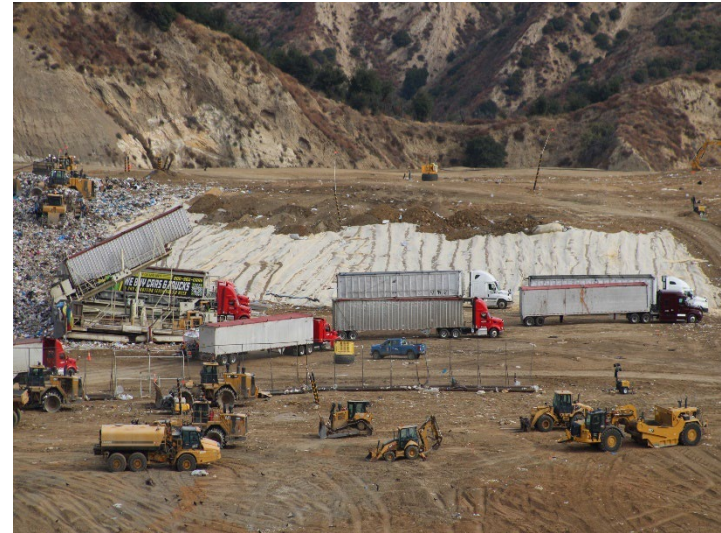
Photo 114: Working Area, CC4 Part 1/2: December 11, 2024
