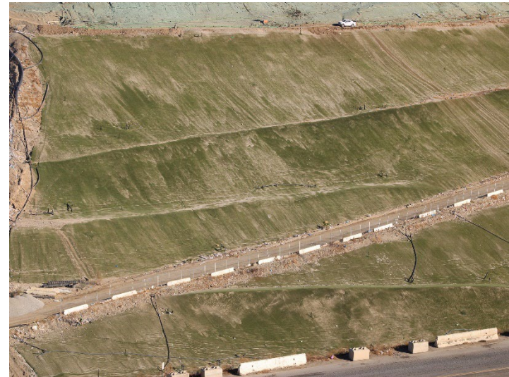
Photo 204: Closure Turf: November 20, 2024
