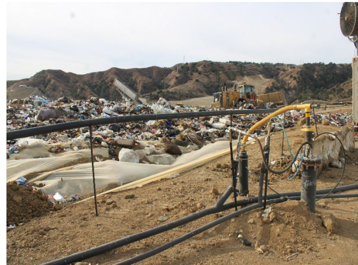
Photo 98: Working Area, CC4 Part 1/2: December 11, 2024
