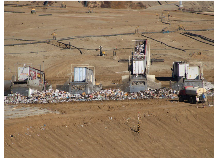
Photo 134: Working Area, CC4 Part 3: November 20, 2024
