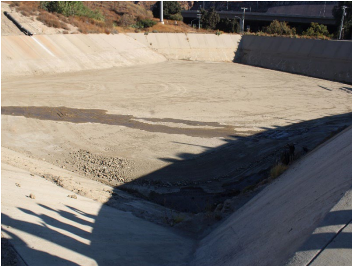
Photo 293: Terminal Basin: October 31, 2024
