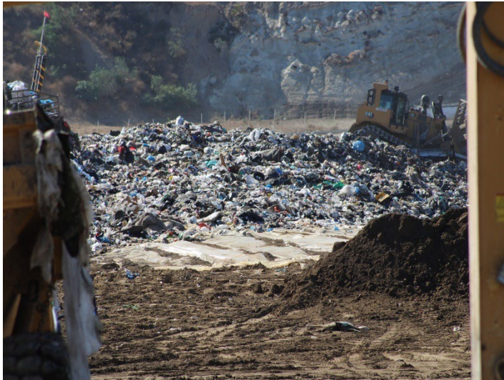
Photo 9: Working Area, CC4 Part 1/2: October 31, 2024
