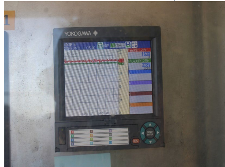
Photo 416: General Site: October 31, 2024
