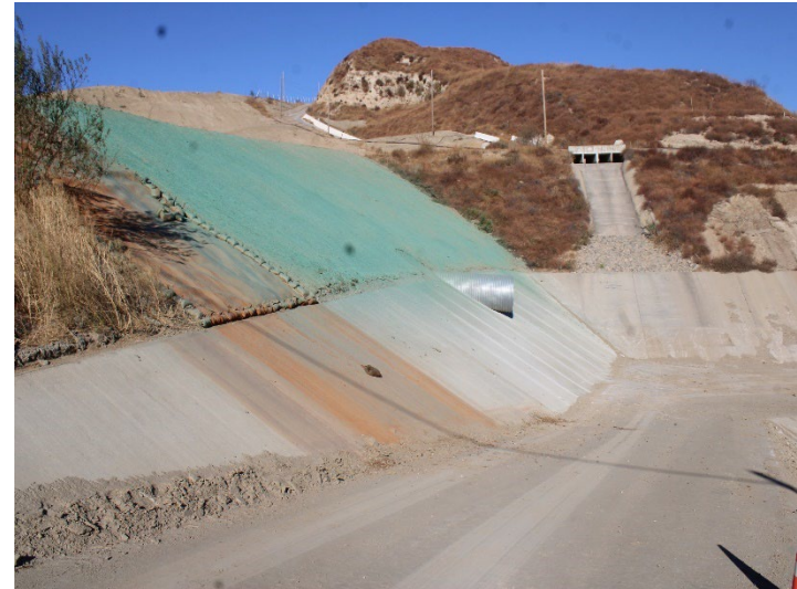
Photo 314: Terminal Basin: November 20, 2024
