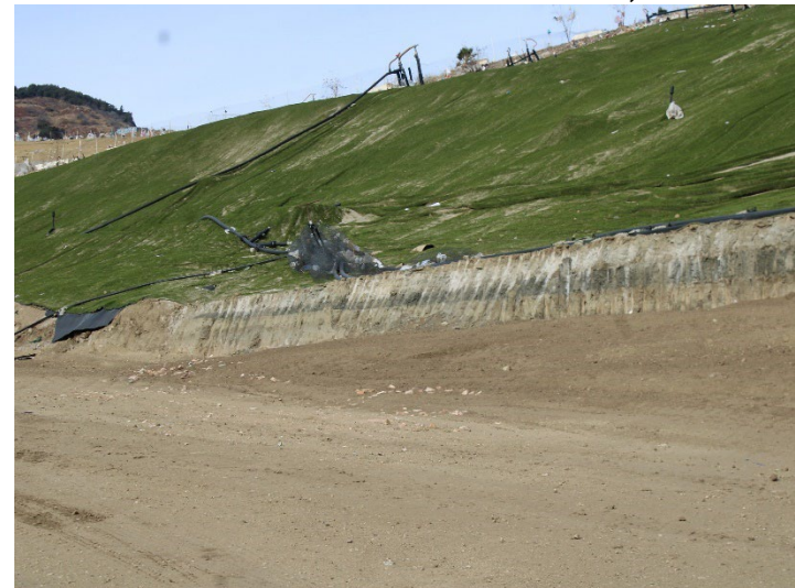
Photo 520: General Site: December 11, 2024
