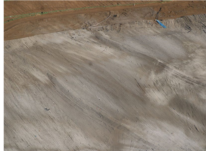
Photo 154: Working Area, CC4 Part 4/5: October 31, 2024
