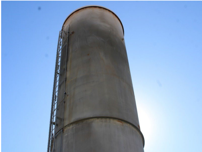
Photo 249: Flares 9, 10, 11 and Gas-to-Energy Facility: November 20, 2024
