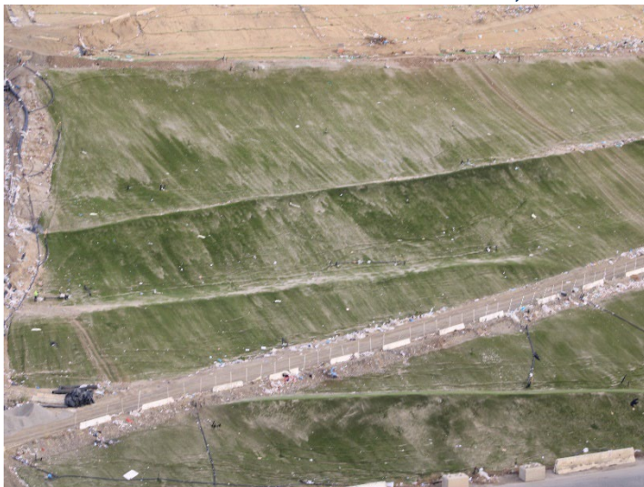
Photo 207: Closure Turf: December 11, 2024
