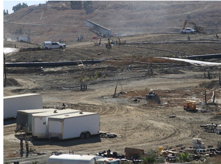
Photo 410: General Site: October 31, 2024
