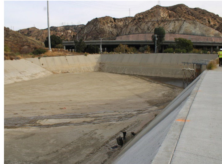
Photo 338: Terminal Basin: December 11, 2024
