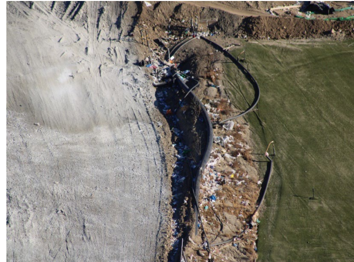
Photo 158: Working Area, CC4 Part 4/5: October 31, 2024
