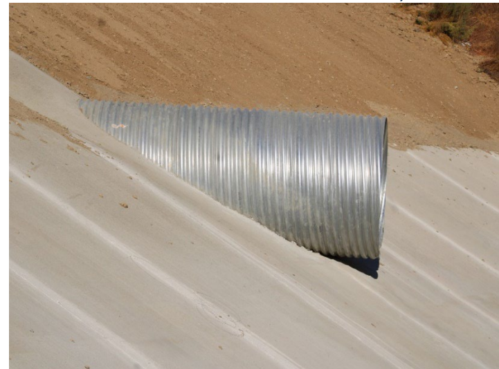
Photo 300: Terminal Basin: October 31, 2024
