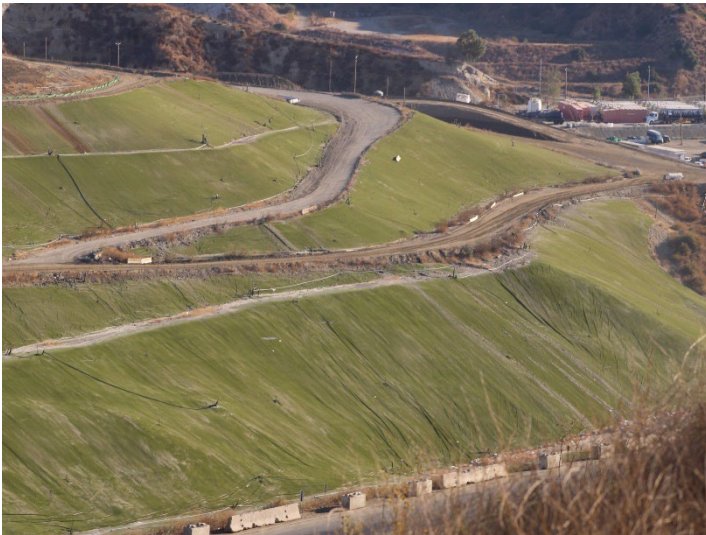
Photo 203: Closure Turf: October 31, 2024
