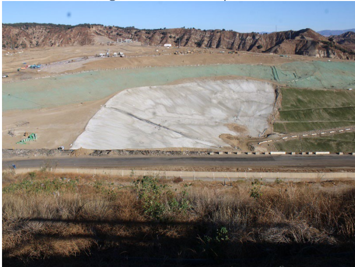
Photo 163: Working Area, CC4 Part 4/5: November 20, 2024
