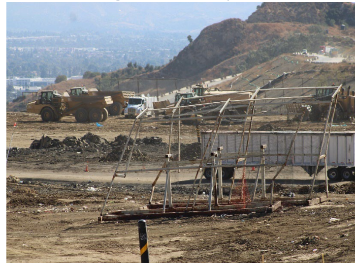
Photo 20: Working Area, CC4 Part 1/2: October 31, 2024
