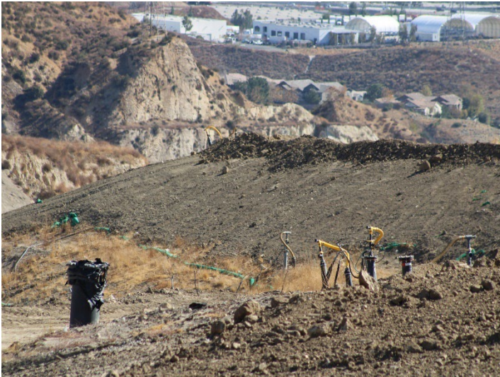
Photo 49: Working Area, CC4 Part 1/2: November 20, 2024
