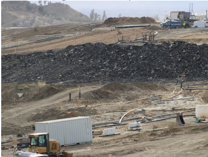
Photo 83: Working Area, CC4 Part 1/2: December 11, 2024
