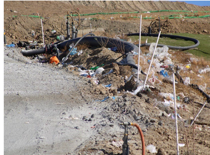
Photo 398: General Site: October 31, 2024
