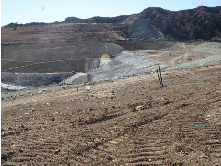
Photo 55: Working Area, CC4 Part 1/2: November 20, 2024
