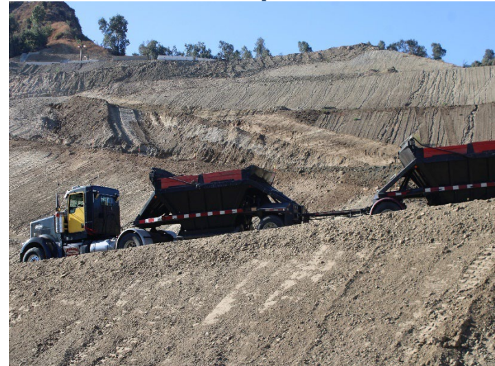
Photo 372: General Site: October 31, 2024
