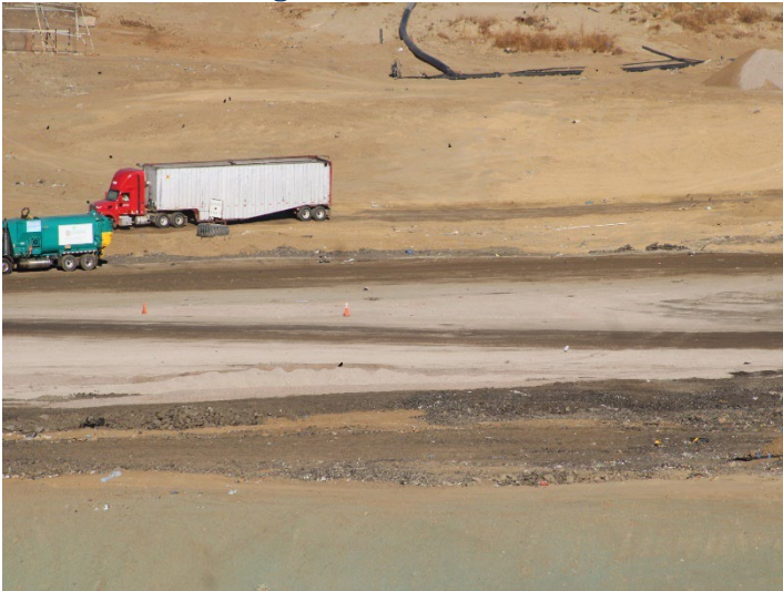
Photo 127: Working Area, CC4 Part 3: November 20, 2024
