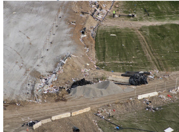
Photo 200: Working Area, CC4 Part 4/5: December 11, 2024
