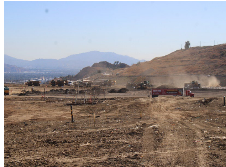
Photo 16: Working Area, CC4 Part 1/2: October 31, 2024
