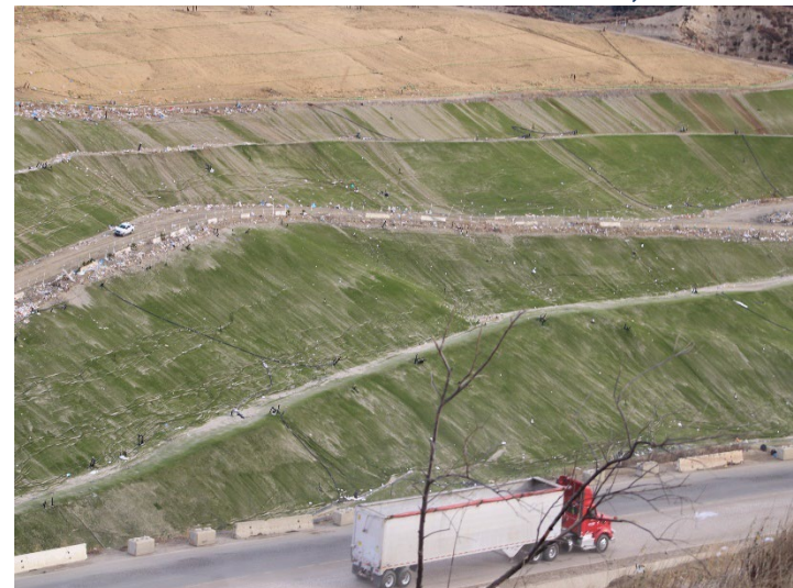
Photo 208: Closure Turf: December 11, 2024
