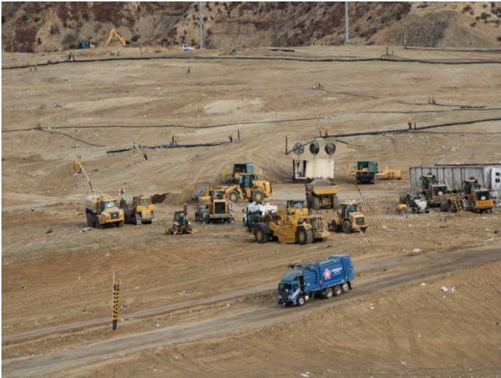
Photo 77: Working Area, CC4 Part 1/2: December 11, 2024
