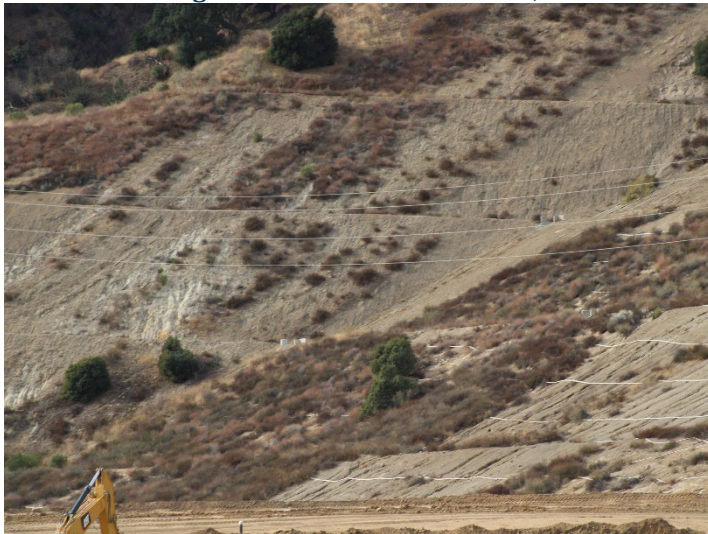
Photo 219: County Sage Mitigation Area and Westside Drainage Channels: December 11, 2024
