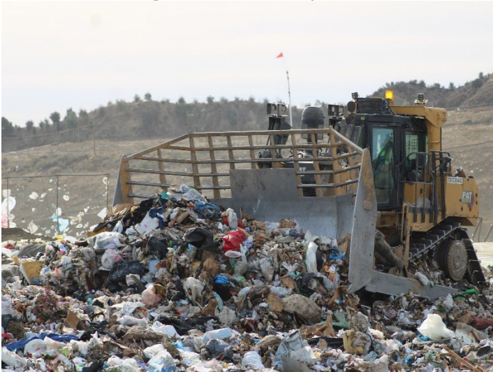
Photo 103: Working Area, CC4 Part 1/2: December 11, 2024
