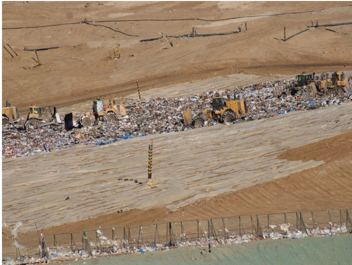
Photo 133: Working Area, CC4 Part 3: November 20, 2024
