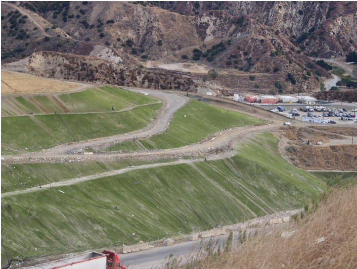
Photo 209: Closure Turf: December 11, 2024
