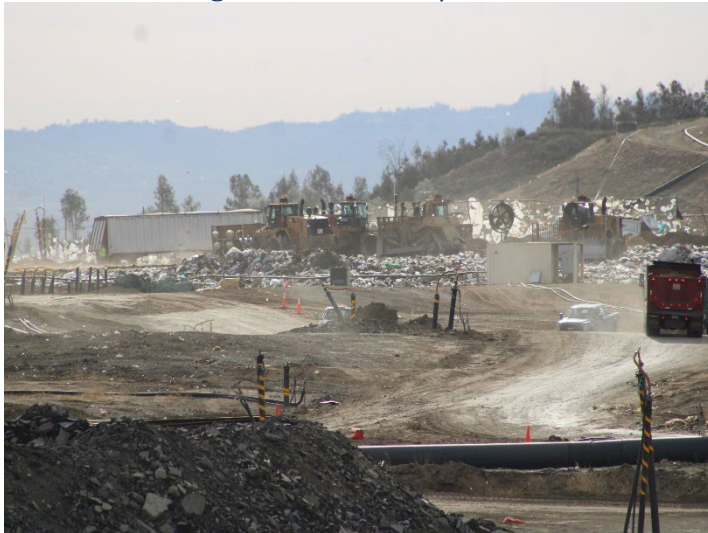
Photo 87: Working Area, CC4 Part 1/2: December 11, 2024
