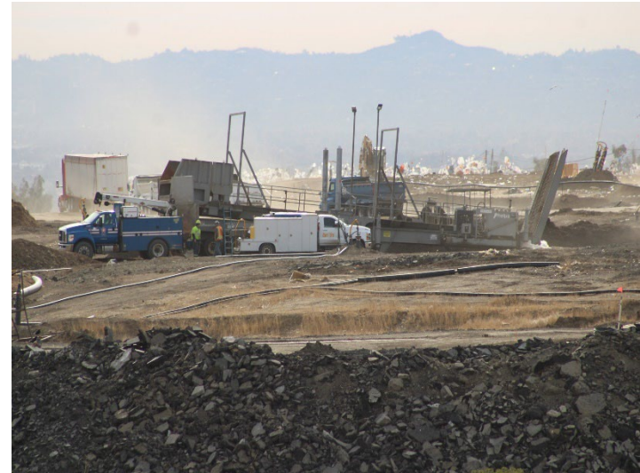
Photo 86: Working Area, CC4 Part 1/2: December 11, 2024
