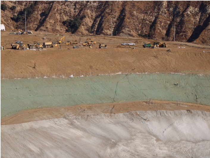
Photo 179: Working Area, CC4 Part 4/5: November 20, 2024
