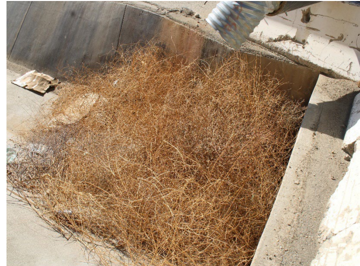
Photo 290: Eastside Drainage Channel: November 20, 2024
