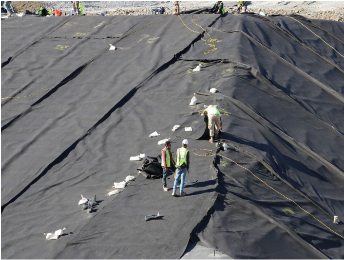
Photo 385: General Site: October 31, 2024
