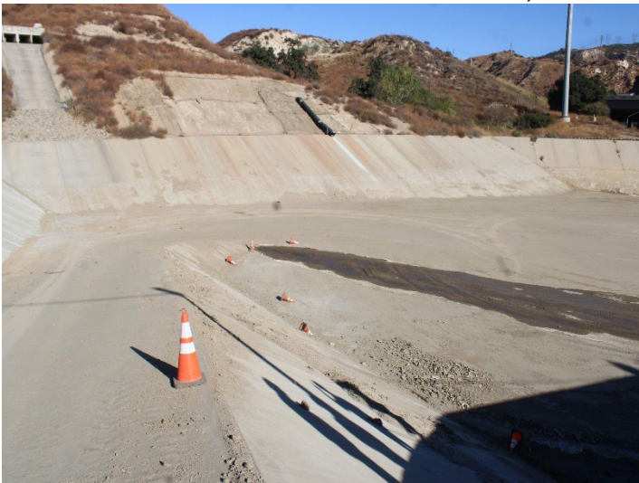
Photo 315: Terminal Basin: November 20, 2024
