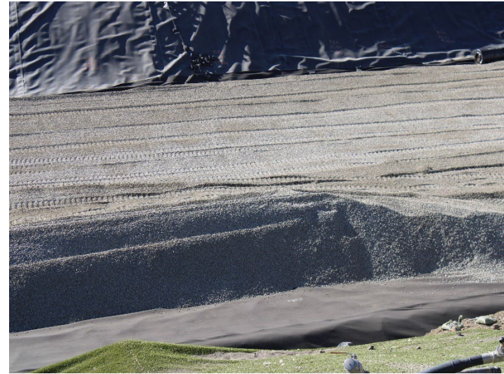
Photo 378: General Site: October 31, 2024
