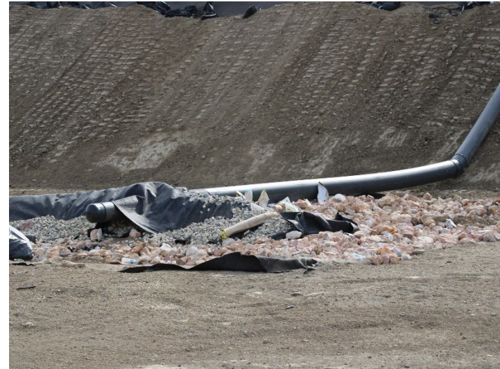
Photo 538: General Site: December 11, 2024
