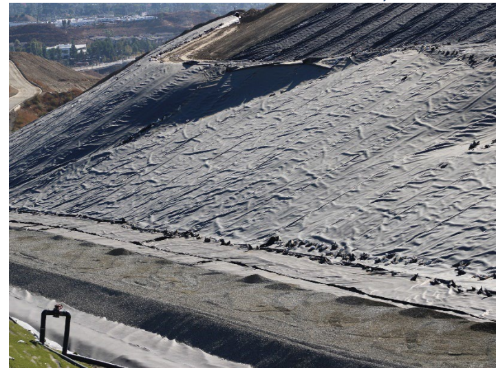
Photo 380: General Site: October 31, 2024
