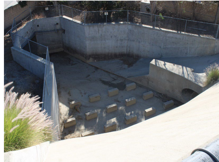
Photo 330: Terminal Basin: November 20, 2024
