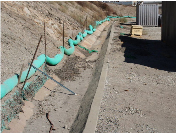
Photo 235: Flares 9, 10, 11 and Gas-to-Energy Facility: October 31, 2024
