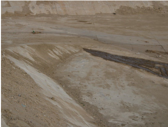
Photo 341: Terminal Basin: December 11, 2024
