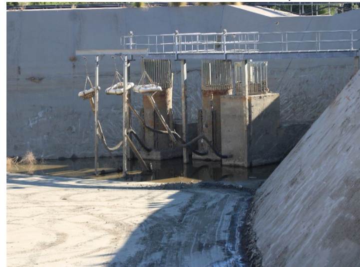
Photo 296: Terminal Basin: October 31, 2024
