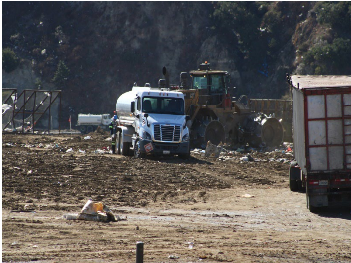
Photo 41: Working Area, CC4 Part 1/2: November 20, 2024
