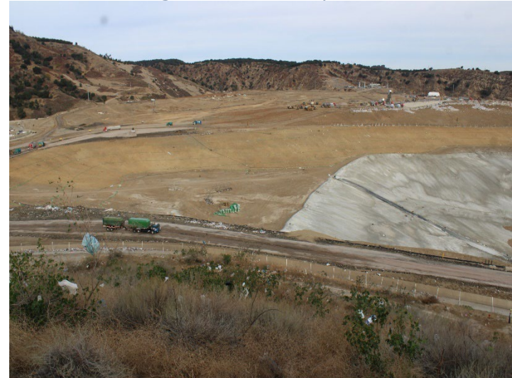
Photo 184: Working Area, CC4 Part 4/5: December 11, 2024
