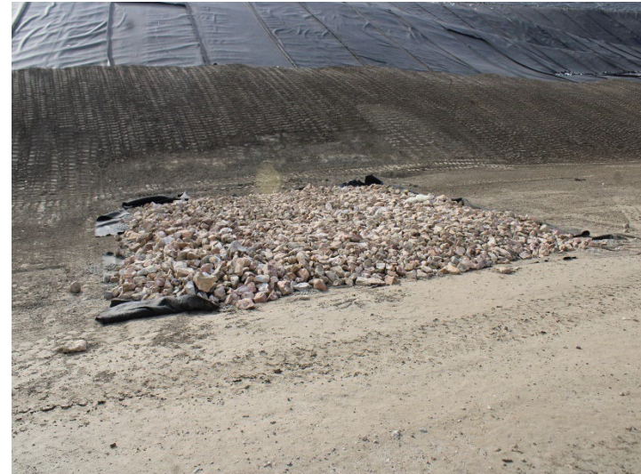
Photo 522: General Site: December 11, 2024
