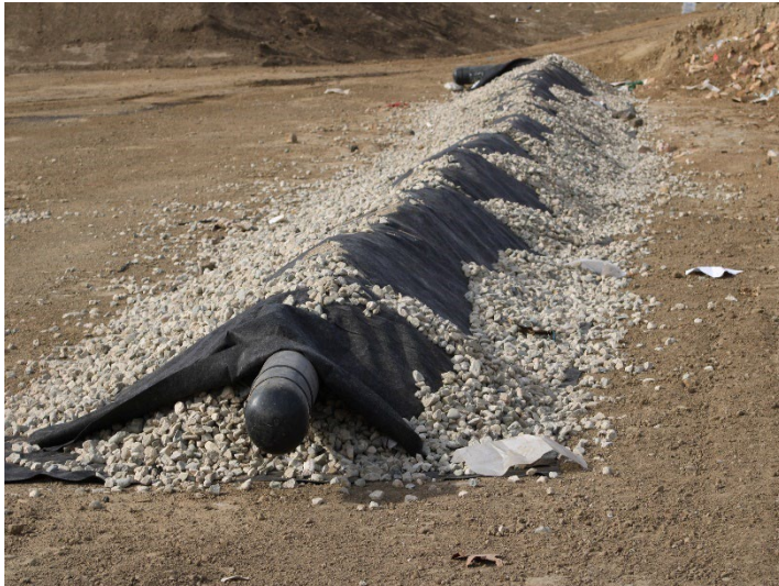
Photo 533: General Site: December 11, 2024
