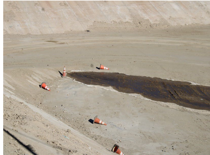
Photo 318: Terminal Basin: November 20, 2024
