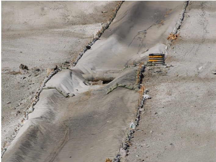
Photo 397: General Site: October 31, 2024
