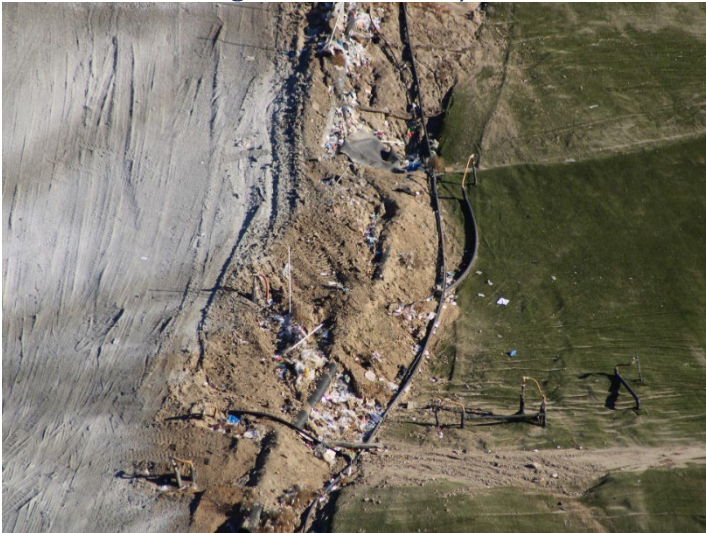
Photo 159: Working Area, CC4 Part 4/5: October 31, 2024
