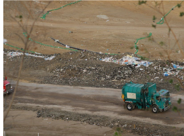
Photo 194: Working Area, CC4 Part 4/5: December 11, 2024
