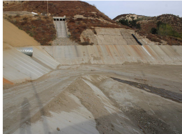
Photo 336: Terminal Basin: December 11, 2024
