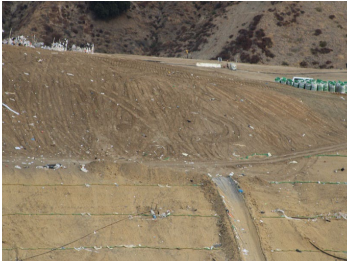
Photo 81: Working Area, CC4 Part 1/2: December 11, 2024
