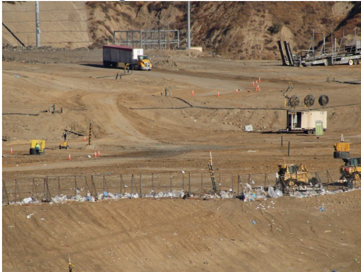
Photo 135: Working Area, CC4 Part 3: November 20, 2024
