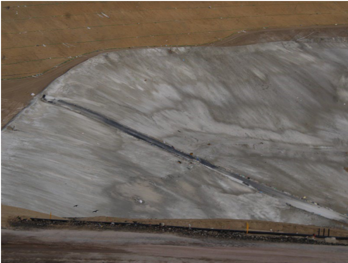
Photo 189: Working Area, CC4 Part 4/5: December 11, 2024
