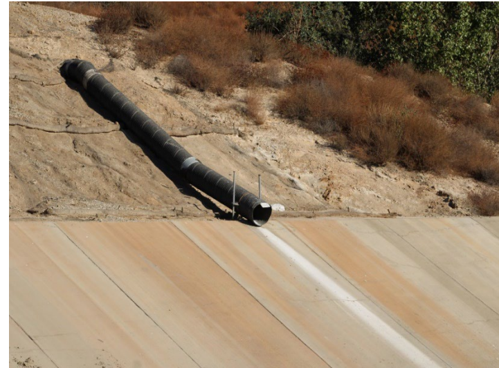
Photo 302: Terminal Basin: October 31, 2024
