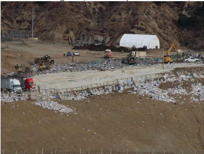
Photo 79: Working Area, CC4 Part 1/2: December 11, 2024
