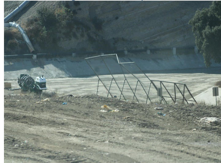
Photo 24: Working Area, CC4 Part 1/2: October 31, 2024
