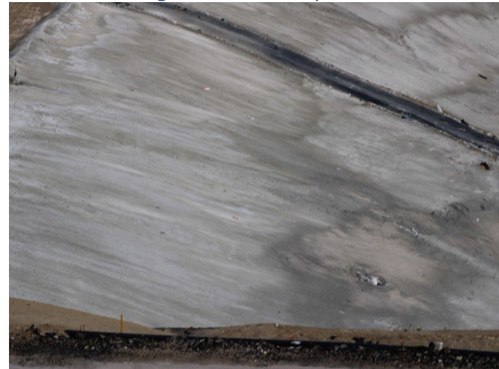
Photo 196: Working Area, CC4 Part 4/5: December 11, 2024
