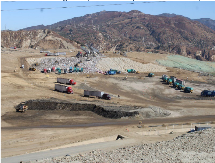
Photo 75: Working Area, CC4 Part 1/2: November 20, 2024
