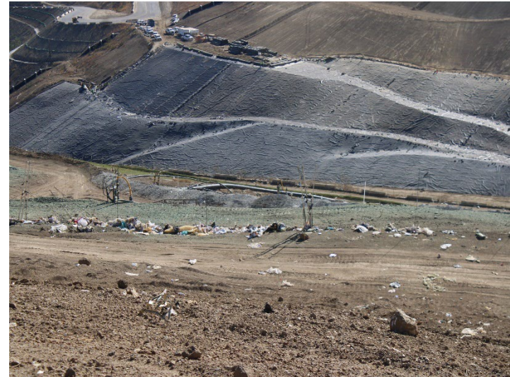
Photo 58: Working Area, CC4 Part 1/2: November 20, 2024
