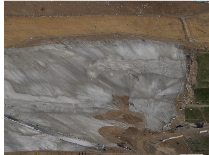
Photo 190: Working Area, CC4 Part 4/5: December 11, 2024
