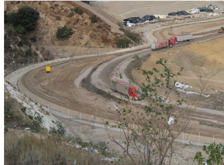
Photo 186: Working Area, CC4 Part 4/5: December 11, 2024
