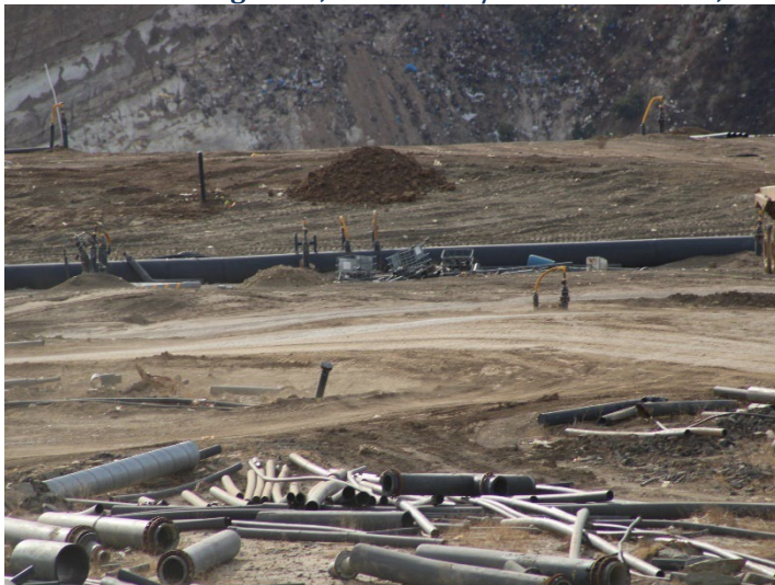
Photo 91: Working Area, CC4 Part 1/2: December 11, 2024
