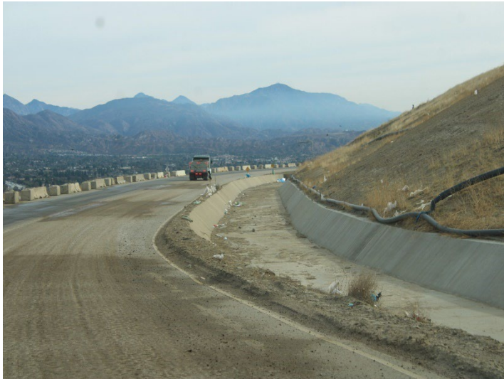
Photo 221: County Sage Mitigation Area and Westside Drainage Channels: December 11, 2024
