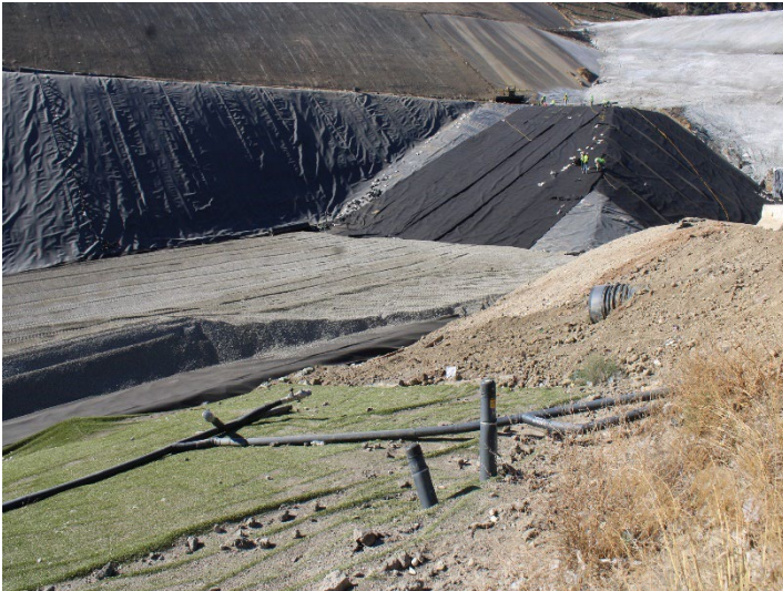
Photo 375: General Site: October 31, 2024
