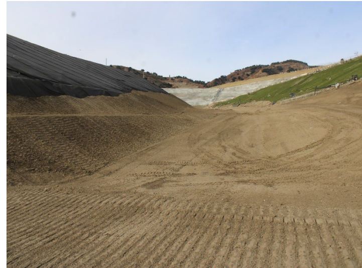
Photo 518: General Site: December 11, 2024
