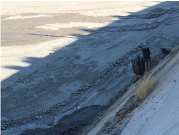
Photo 319: Terminal Basin: November 20, 2024
