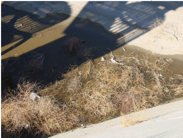
Photo 323: Terminal Basin: November 20, 2024
