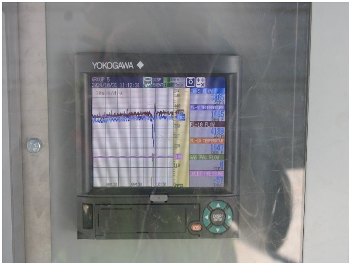
Photo 229: Flares 9, 10, 11 and Gas-to-Energy Facility: October 31, 2024
