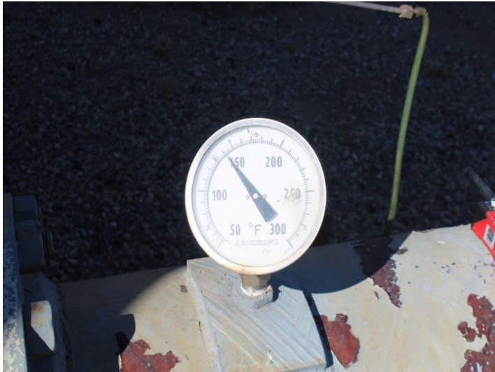
Photo 413: General Site: October 31, 2024
