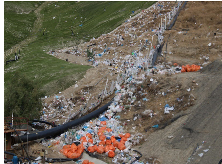
Photo 568: General Site: December 11, 2024
