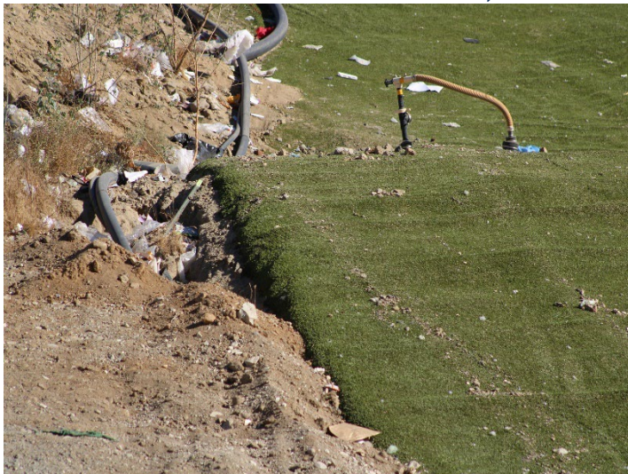
Photo 399: General Site: October 31, 2024
