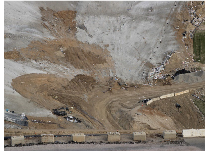
Photo 198: Working Area, CC4 Part 4/5: December 11, 2024
