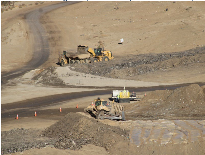
Photo 115: Working Area, CC4 Part 3: October 31, 2024
