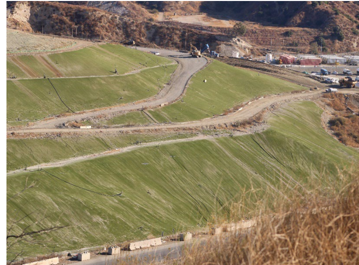
Photo 206: Closure Turf: November 20, 2024
