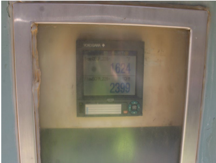
Photo 421: General Site: October 31, 2024
