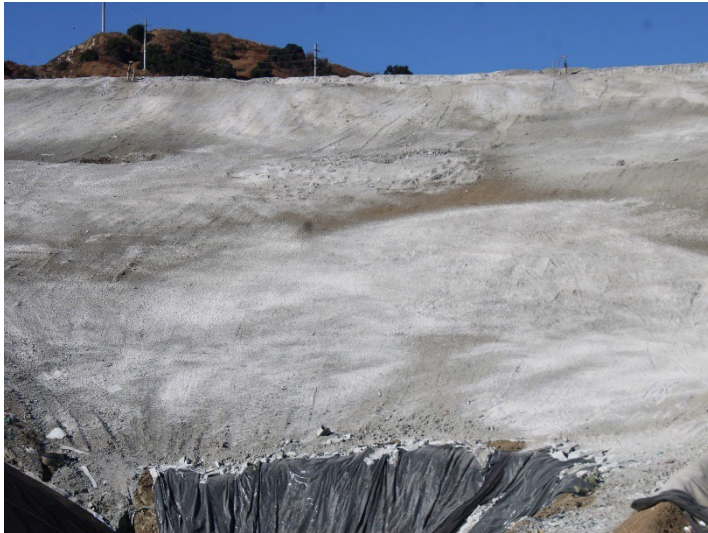
Photo 389: General Site: October 31, 2024
