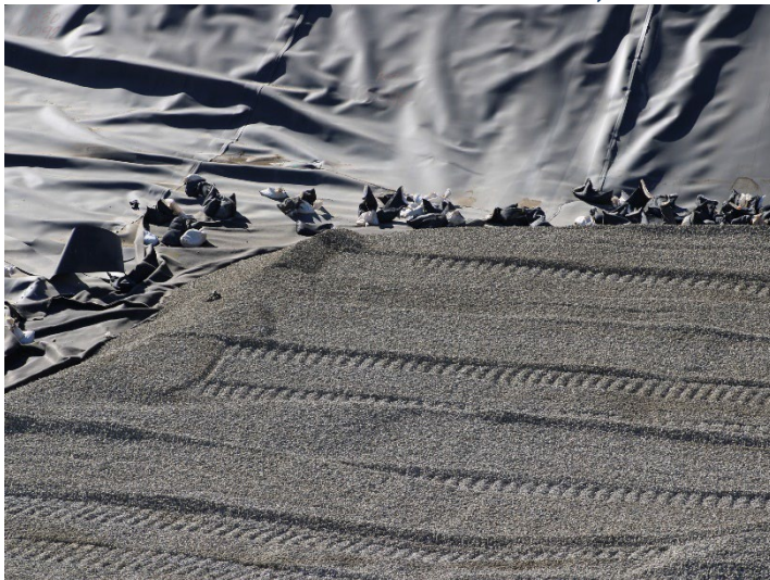
Photo 383: General Site: October 31, 2024
