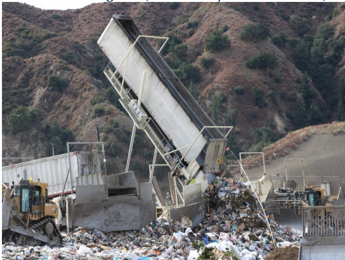
Photo 107: Working Area, CC4 Part 1/2: December 11, 2024
