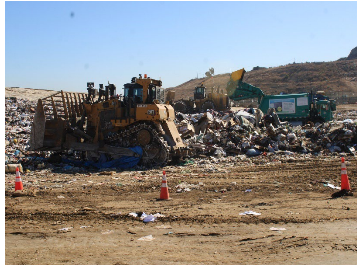
Photo 66: Working Area, CC4 Part 1/2: November 20, 2024
