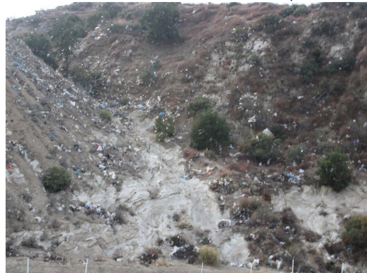
Photo 548: General Site: December 11, 2024
