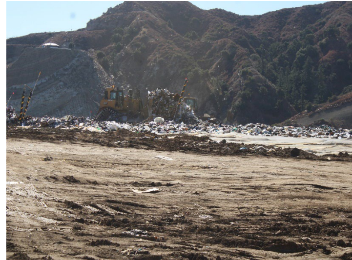
Photo 62: Working Area, CC4 Part 1/2: November 20, 2024
