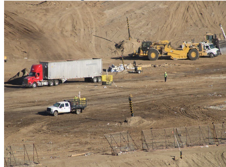
Photo 120: Working Area, CC4 Part 3: October 31, 2024
