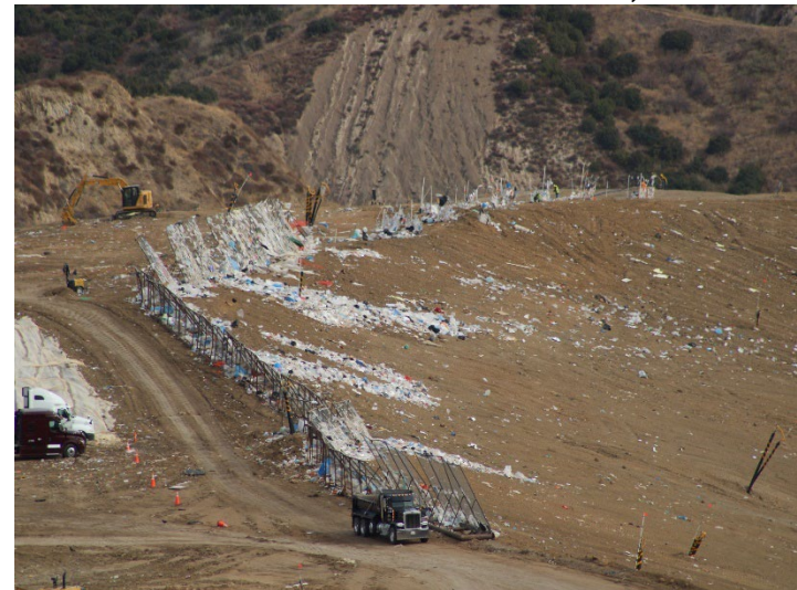
Photo 564: General Site: December 11, 2024
