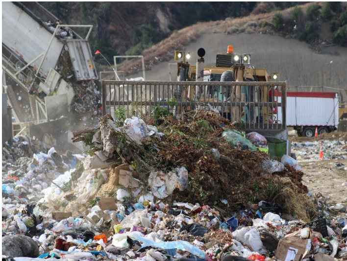
Photo 105: Working Area, CC4 Part 1/2: December 11, 2024
