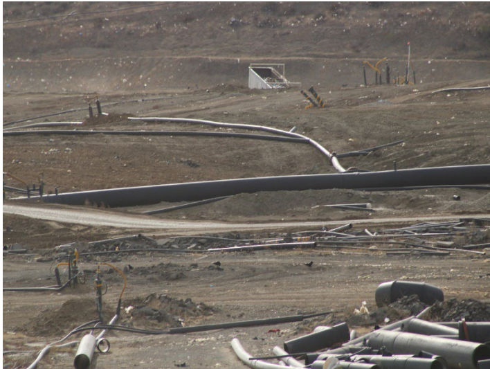
Photo 89: Working Area, CC4 Part 1/2: December 11, 2024
