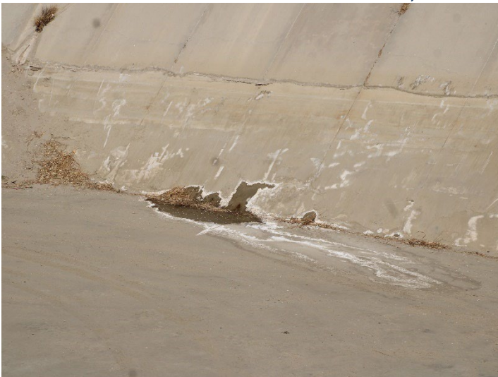
Photo 331: Terminal Basin: November 20, 2024
