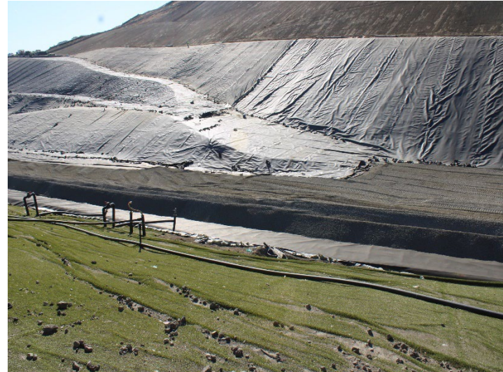
Photo 374: General Site: October 31, 2024
