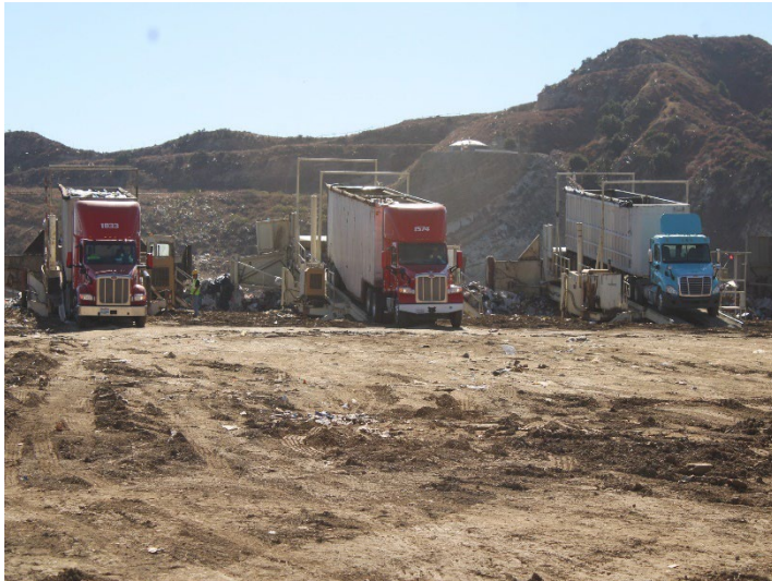
Photo 61: Working Area, CC4 Part 1/2: November 20, 2024
