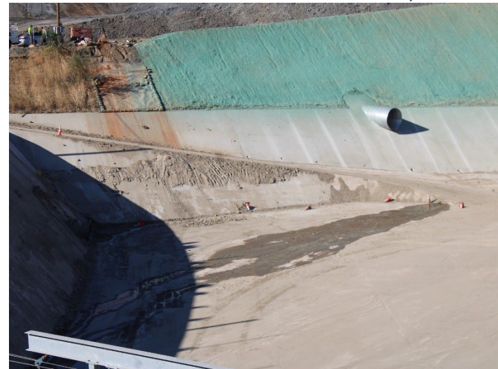
Photo 324: Terminal Basin: November 20, 2024
