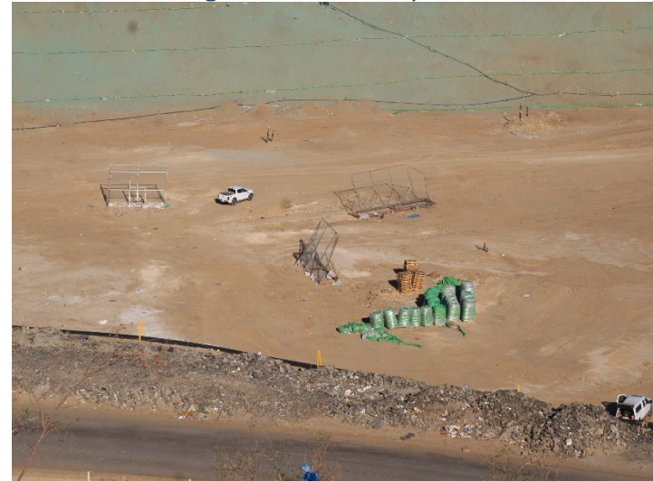
Photo 172: Working Area, CC4 Part 4/5: November 20, 2024
