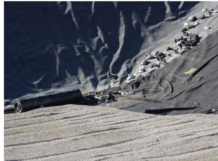
Photo 384: General Site: October 31, 2024
