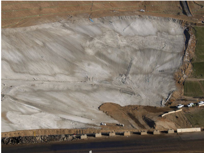
Photo 149: Working Area, CC4 Part 4/5: October 31, 2024
