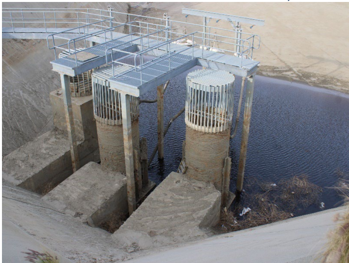
Photo 347: Terminal Basin: December 11, 2024
