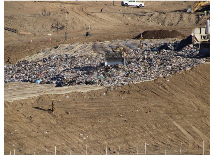
Photo 124: Working Area, CC4 Part 3: October 31, 2024
