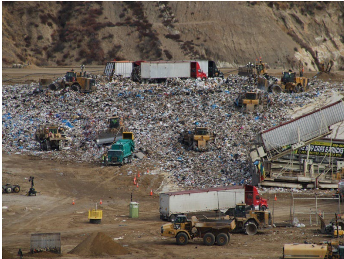
Photo 113: Working Area, CC4 Part 1/2: December 11, 2024
