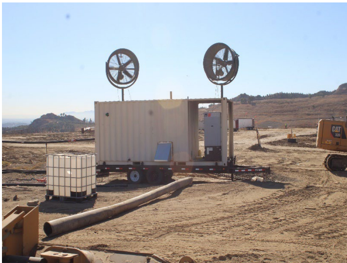
Photo 7: Working Area, CC4 Part 1/2: October 31, 2024
