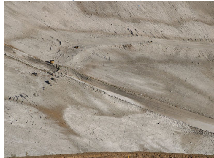
Photo 156: Working Area, CC4 Part 4/5: October 31, 2024
