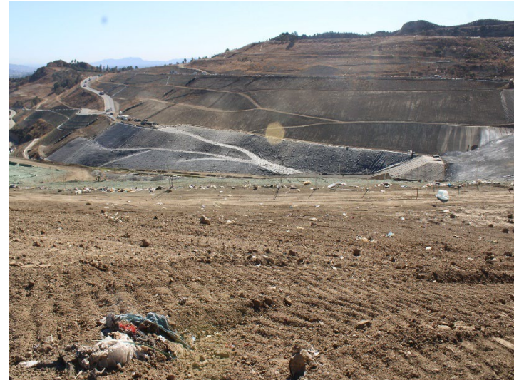
Photo 54: Working Area, CC4 Part 1/2: November 20, 2024
