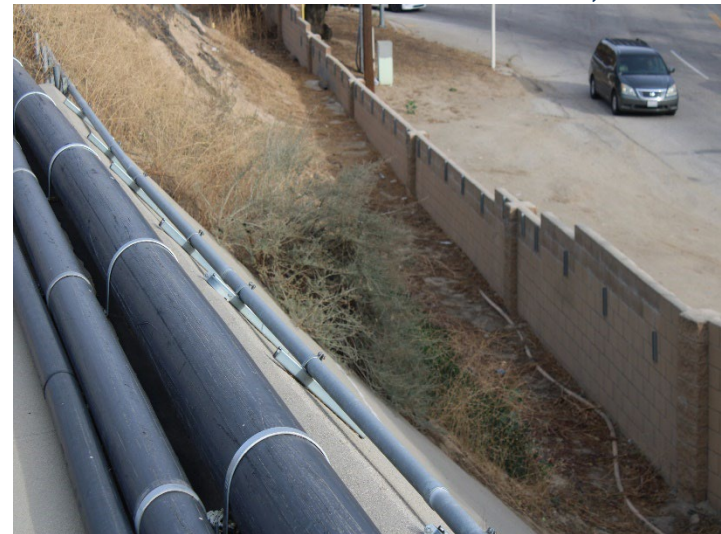
Photo 348: Terminal Basin: December 11, 2024
