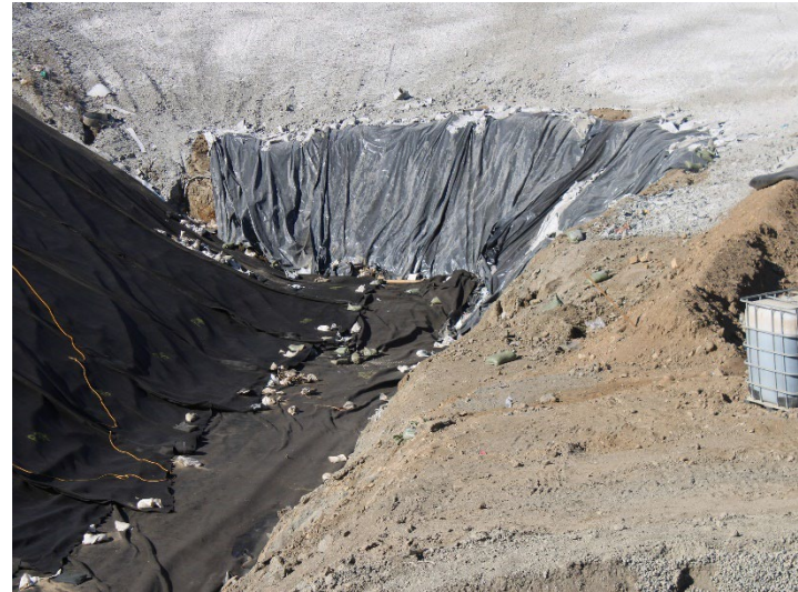
Photo 388: General Site: October 31, 2024
