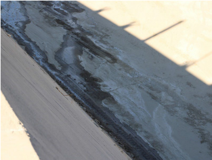
Photo 333: Terminal Basin: November 20, 2024
