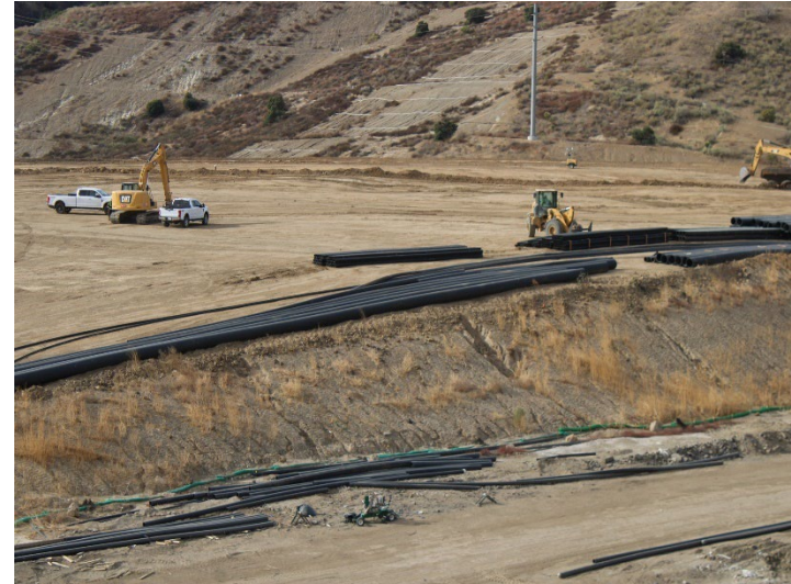
Photo 270: County Top Deck: December 11, 2024
