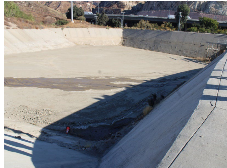
Photo 316: Terminal Basin: November 20, 2024
