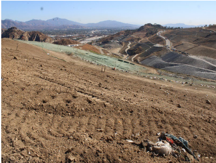
Photo 53: Working Area, CC4 Part 1/2: November 20, 2024
