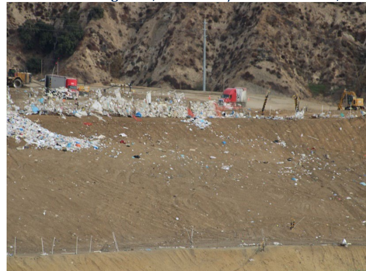
Photo 80: Working Area, CC4 Part 1/2: December 11, 2024
