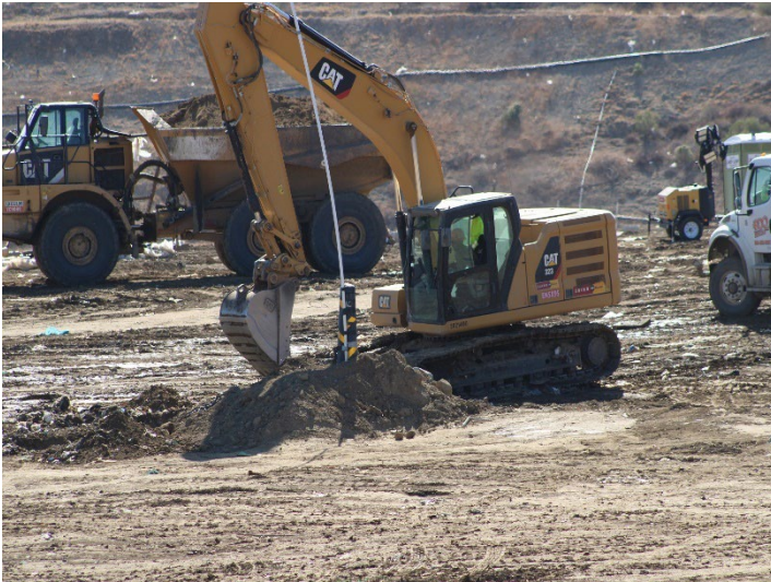
Photo 45: Working Area, CC4 Part 1/2: November 20, 2024
