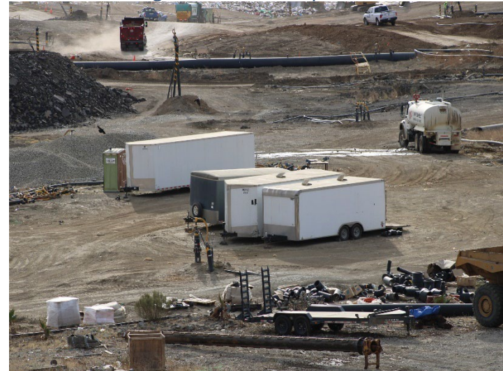
Photo 84: Working Area, CC4 Part 1/2: December 11, 2024
