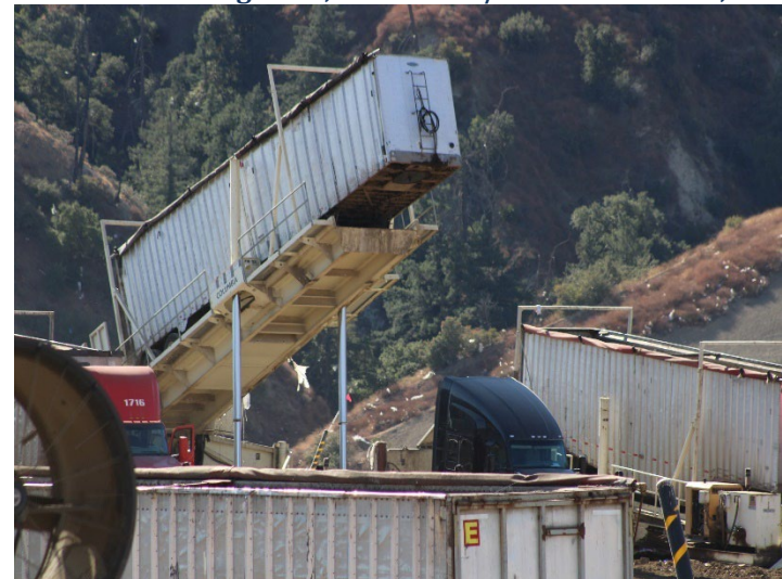
Photo 48: Working Area, CC4 Part 1/2: November 20, 2024
