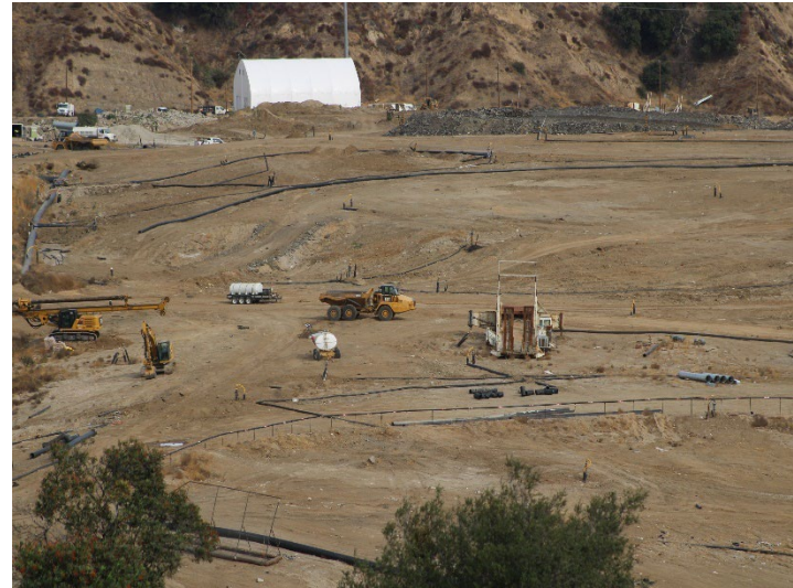
Photo 110: Working Area, CC4 Part 1/2: December 11, 2024
