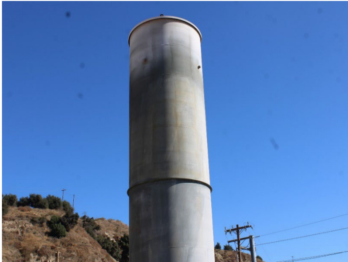
Photo 237: Flares 9, 10, 11 and Gas-to-Energy Facility: November 20, 2024
