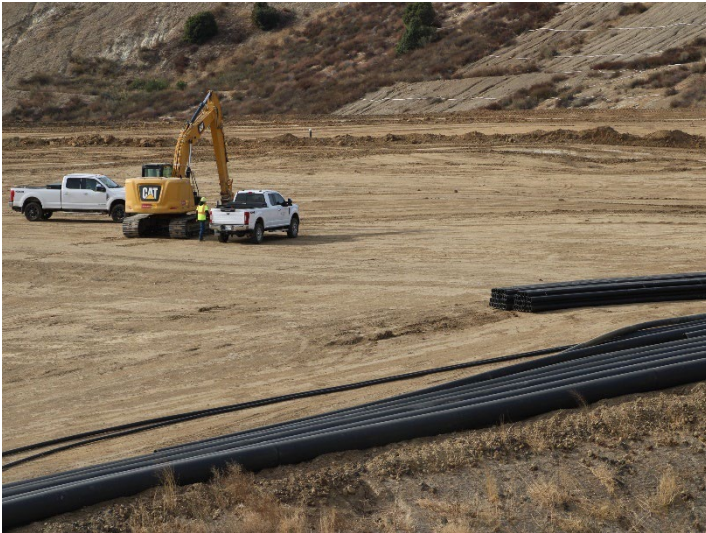
Photo 273: County Top Deck: December 11, 2024
