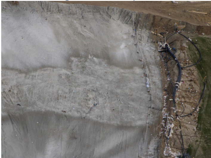
Photo 199: Working Area, CC4 Part 4/5: December 11, 2024
