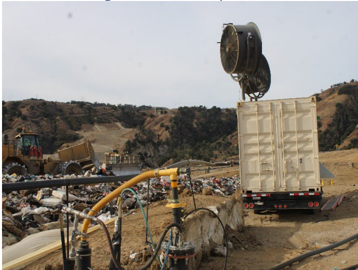
Photo 99: Working Area, CC4 Part 1/2: December 11, 2024
