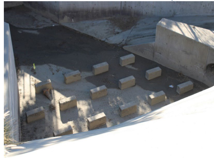
Photo 312: Terminal Basin: October 31, 2024
