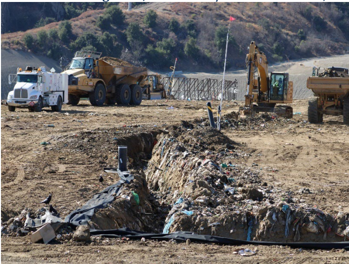
Photo 51: Working Area, CC4 Part 1/2: November 20, 2024
