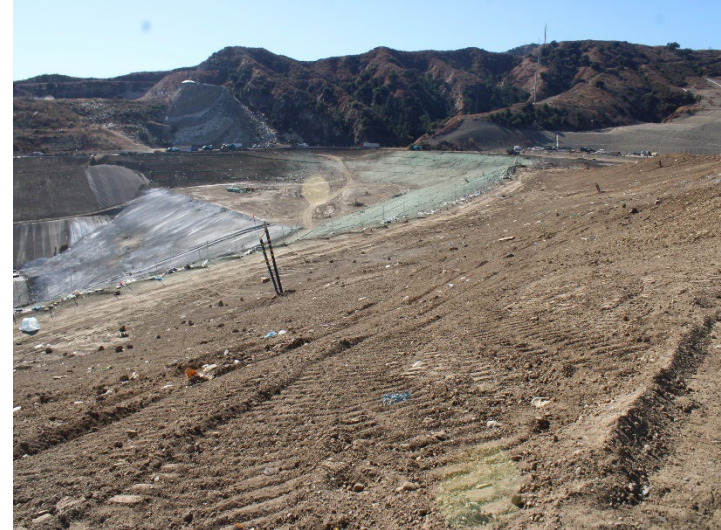
Photo 56: Working Area, CC4 Part 1/2: November 20, 2024
