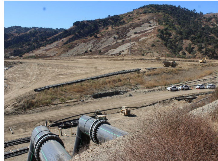
Photo 406: General Site: October 31, 2024
