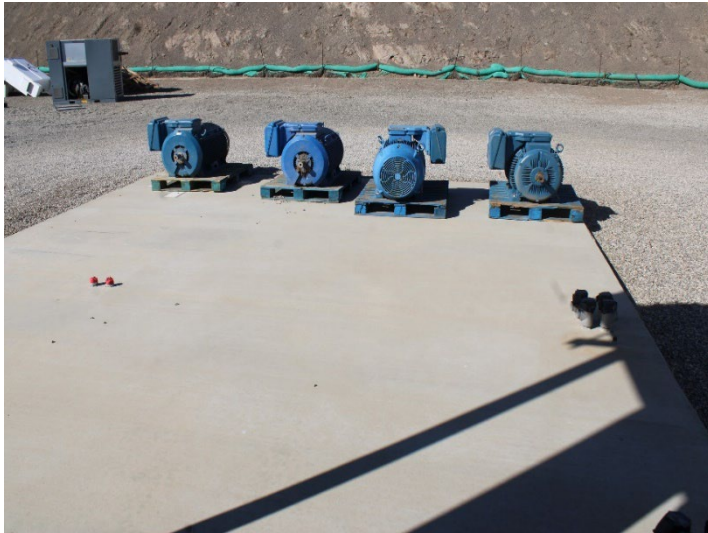
Photo 245: Flares 9, 10, 11 and Gas-to-Energy Facility: November 20, 2024
