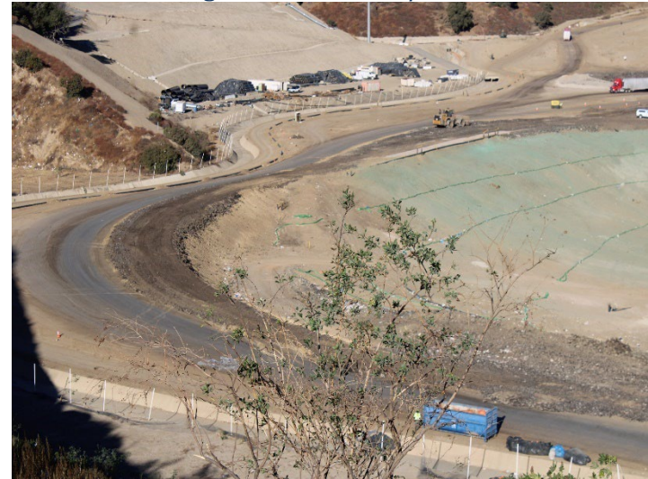
Photo 164: Working Area, CC4 Part 4/5: November 20, 2024
