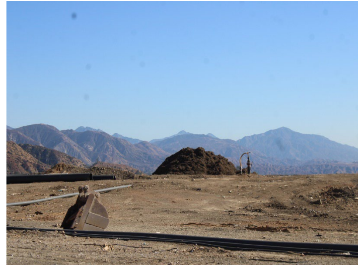
Photo 26: Working Area, CC4 Part 1/2: November 20, 2024
