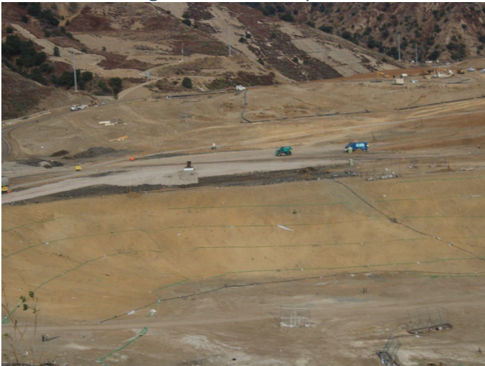
Photo 191: Working Area, CC4 Part 4/5: December 11, 2024
