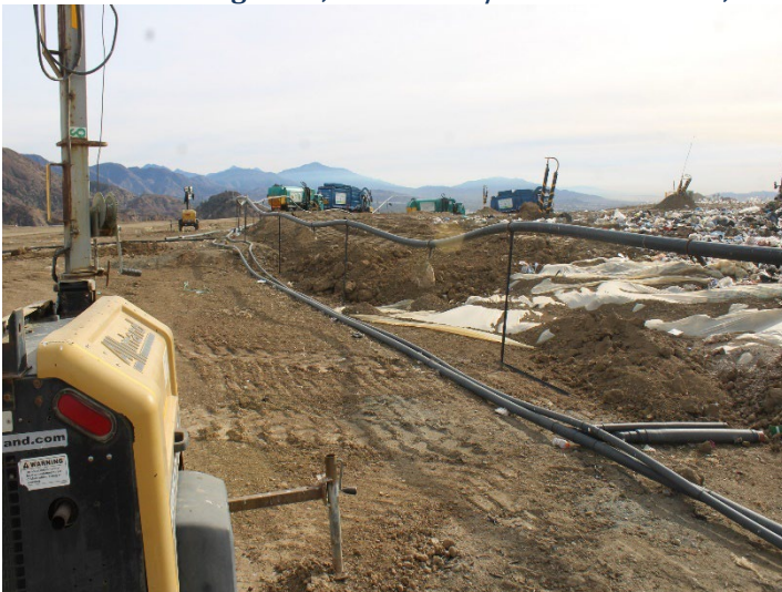
Photo 95: Working Area, CC4 Part 1/2: December 11, 2024
