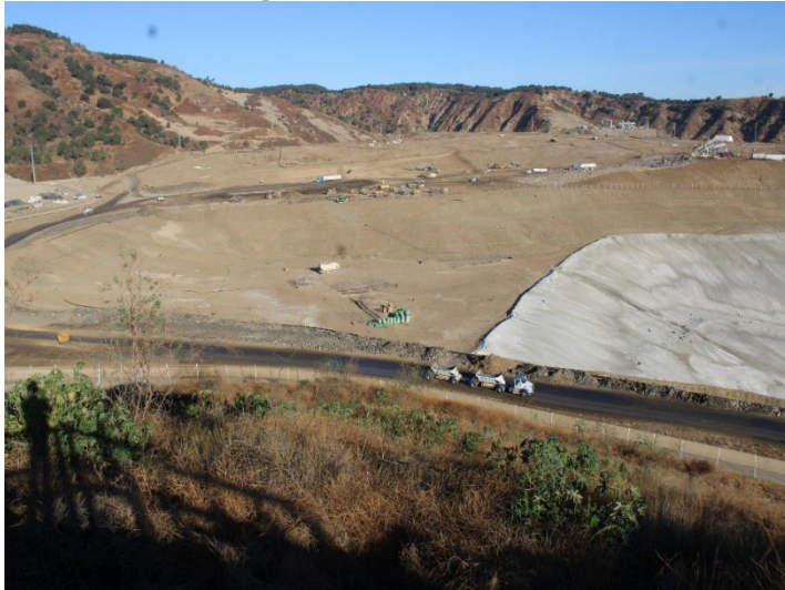
Photo 143: Working Area, CC4 Part 4/5: October 31, 2024
