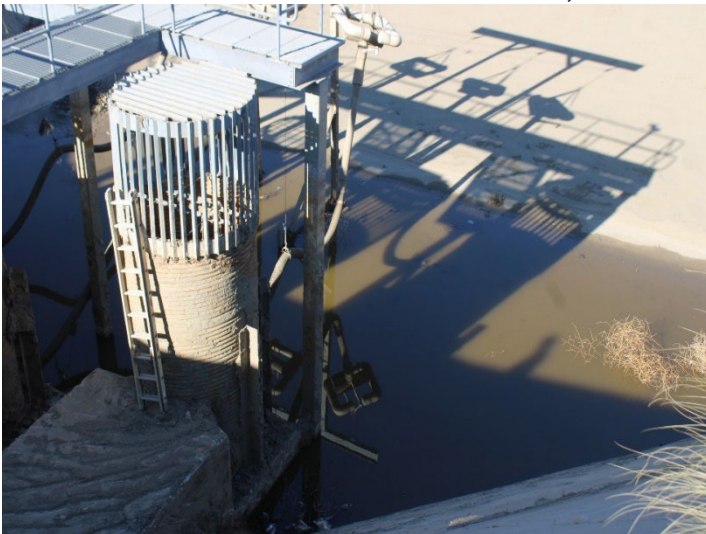
Photo 311: Terminal Basin: October 31, 2024
