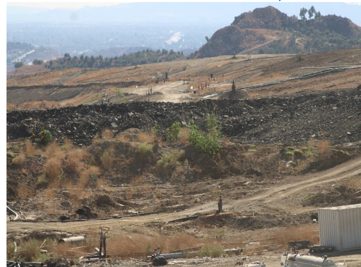
Photo 408: General Site: October 31, 2024
