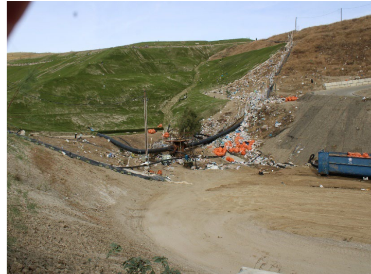
Photo 566: General Site: December 11, 2024
