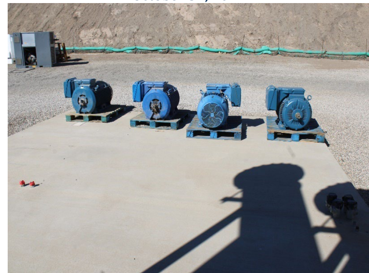
Photo 232: Flares 9, 10, 11 and Gas-to-Energy Facility: October 31, 2024
