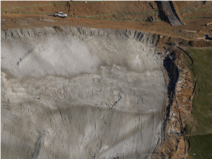
Photo 155: Working Area, CC4 Part 4/5: October 31, 2024
