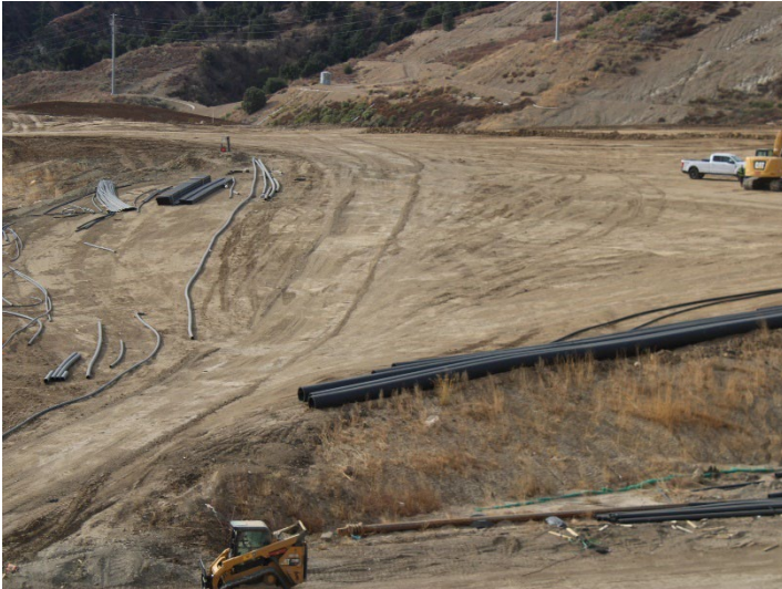
Photo 269: County Top Deck: December 11, 2024
