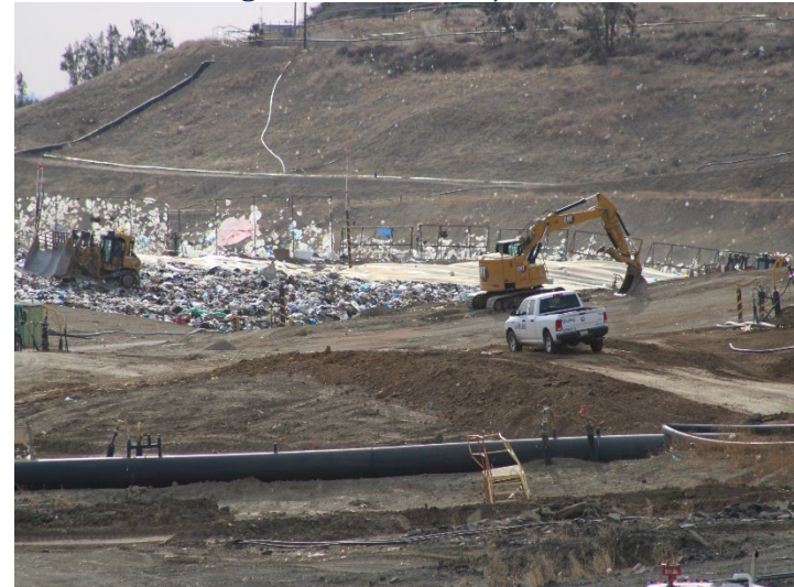
Photo 88: Working Area, CC4 Part 1/2: December 11, 2024
