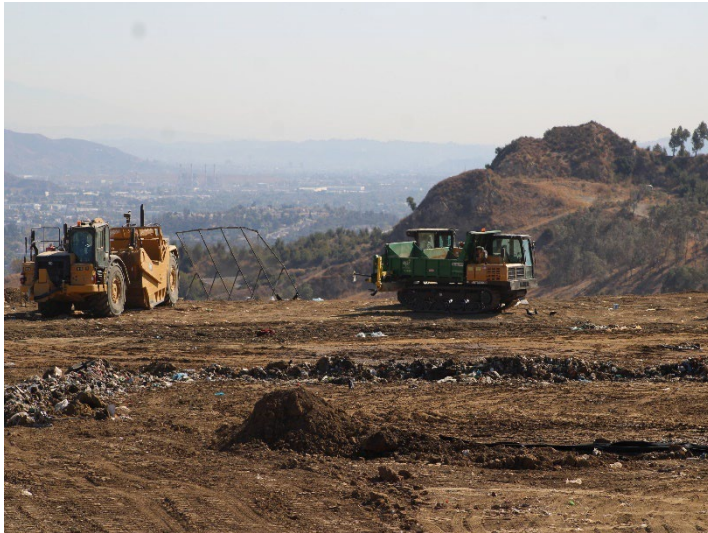
Photo 37: Working Area, CC4 Part 1/2: November 20, 2024
