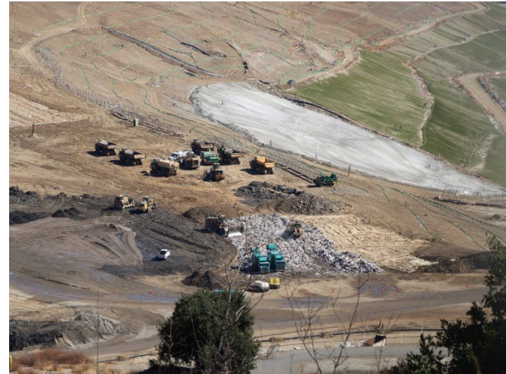
Photo 418: General Site: October 31, 2024
