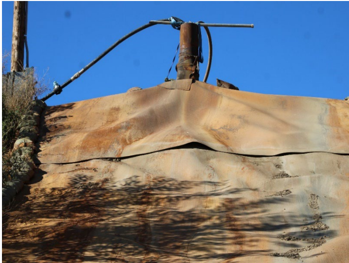
Photo 301: Terminal Basin: October 31, 2024
