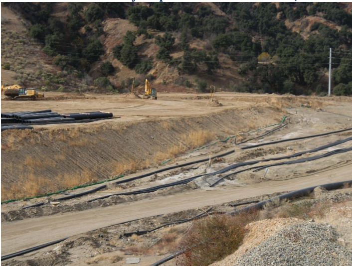
Photo 271: County Top Deck: December 11, 2024
