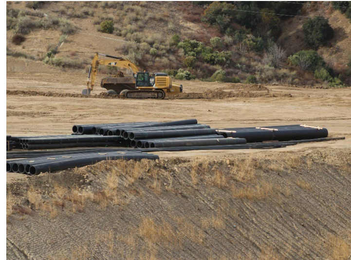
Photo 274: County Top Deck: December 11, 2024
