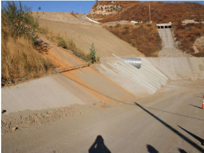
Photo 291: Terminal Basin: October 31, 2024
