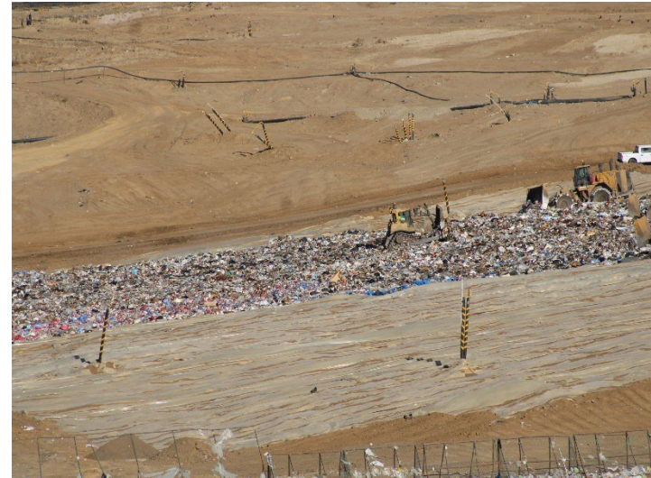
Photo 130: Working Area, CC4 Part 3: November 20, 2024
