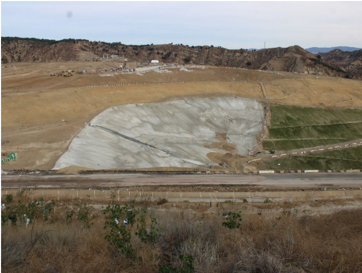
Photo 185: Working Area, CC4 Part 4/5: December 11, 2024
