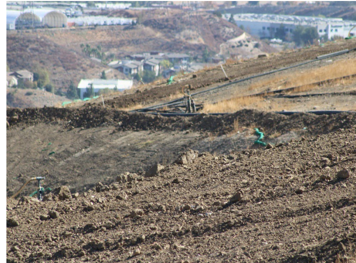
Photo 50: Working Area, CC4 Part 1/2: November 20, 2024
