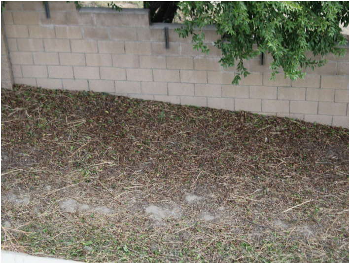
Photo 349: Terminal Basin: December 11, 2024
