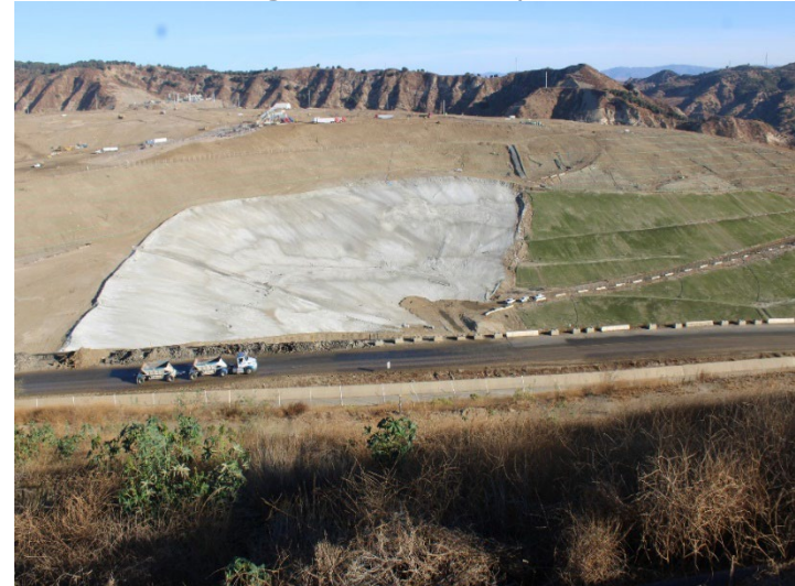
Photo 144: Working Area, CC4 Part 4/5: October 31, 2024
