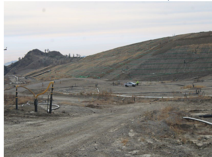
Photo 500: General Site: December 11, 2024
