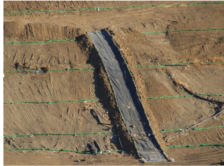
Photo 126: Working Area, CC4 Part 3: October 31, 2024
