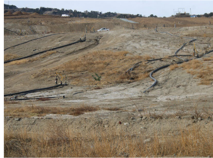
Photo 502: General Site: December 11, 2024
