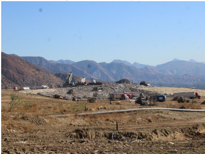
Photo 15: Working Area, CC4 Part 1/2: October 31, 2024
