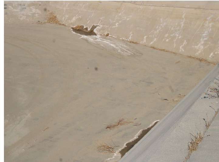
Photo 326: Terminal Basin: November 20, 2024
