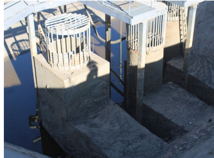
Photo 306: Terminal Basin: October 31, 2024
