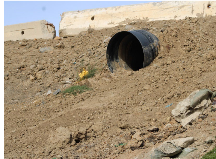
Photo 534: General Site: December 11, 2024
