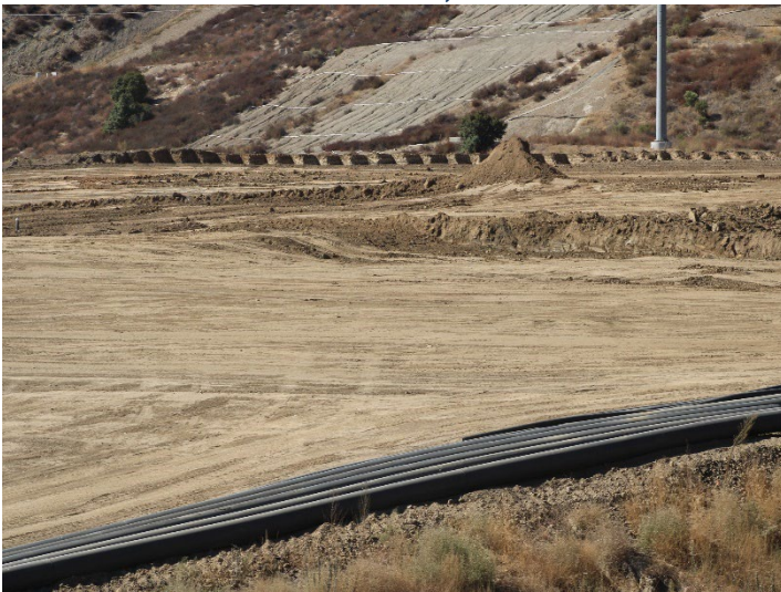
Photo 263: County Top Deck: October 31, 2024
