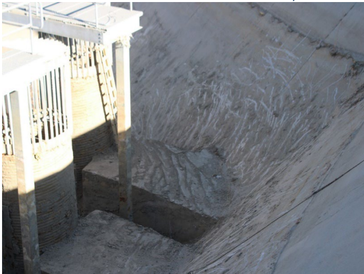
Photo 307: Terminal Basin: October 31, 2024
