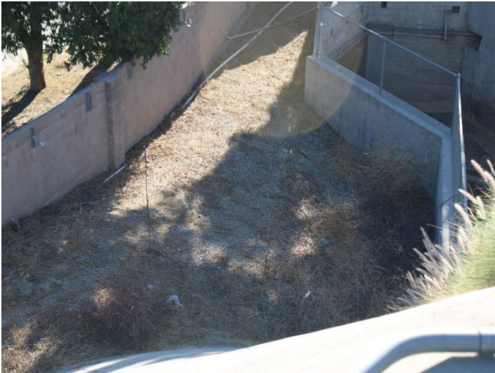
Photo 309: Terminal Basin: October 31, 2024
