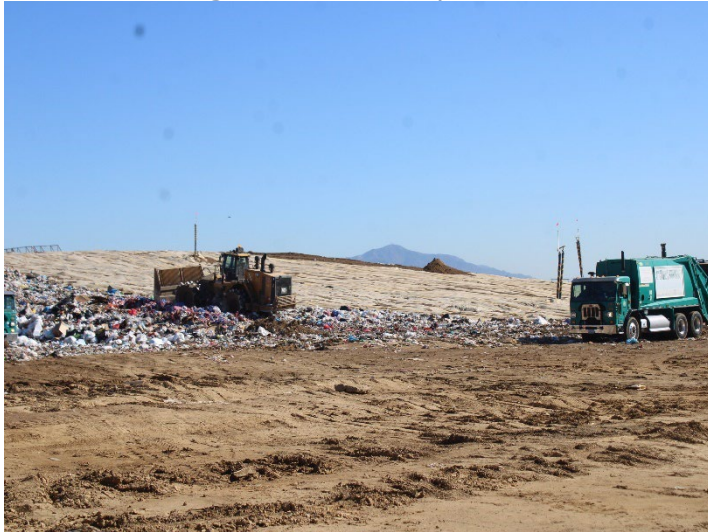
Photo 67: Working Area, CC4 Part 1/2: November 20, 2024
