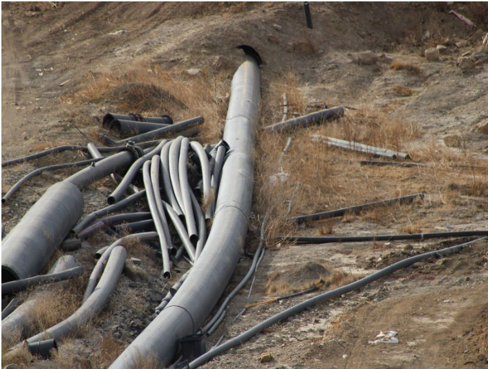
Photo 93: Working Area, CC4 Part 1/2: December 11, 2024
