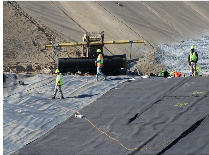
Photo 386: General Site: October 31, 2024
