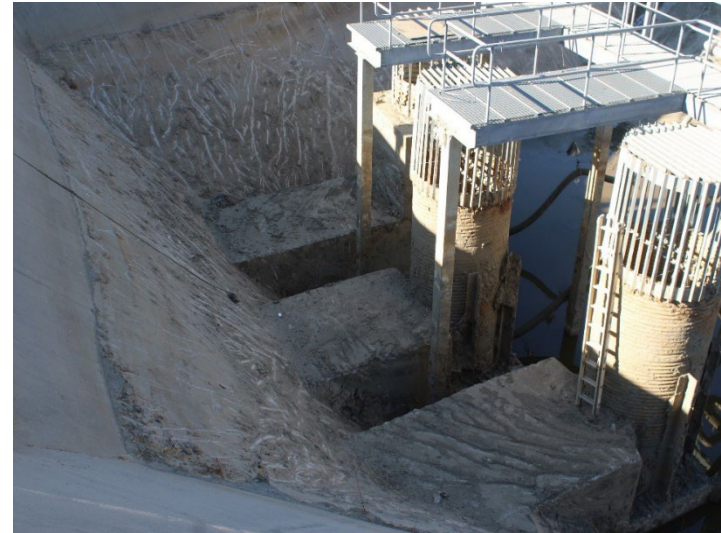
Photo 310: Terminal Basin: October 31, 2024
