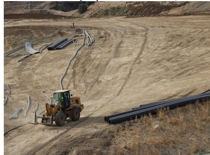
Photo 272: County Top Deck: December 11, 2024
