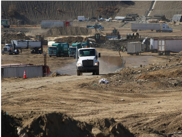
Photo 13: Working Area, CC4 Part 1/2: October 31, 2024
