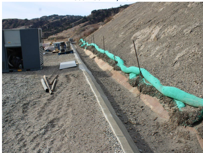
Photo 259: Flares 9, 10, 11 and Gas-to-Energy Facility: December 11, 2024
