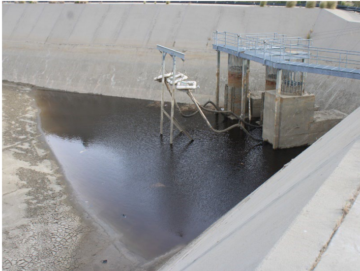
Photo 345: Terminal Basin: December 11, 2024
