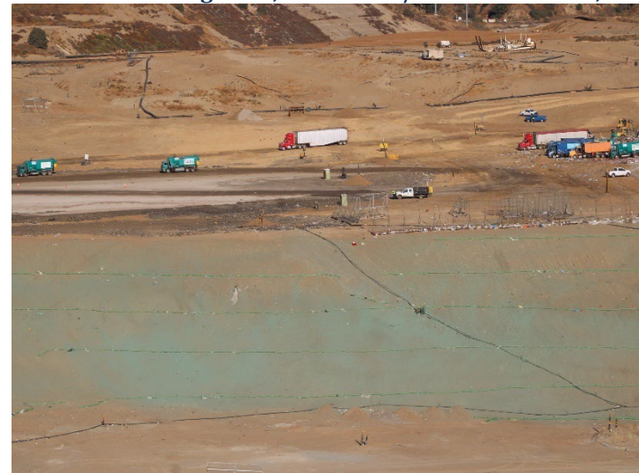
Photo 176: Working Area, CC4 Part 4/5: November 20, 2024
