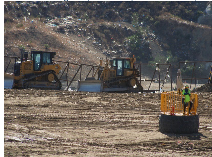
Photo 40: Working Area, CC4 Part 1/2: November 20, 2024
