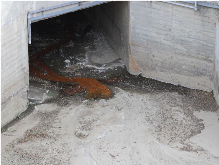
Photo 353: Terminal Basin: December 11, 2024
