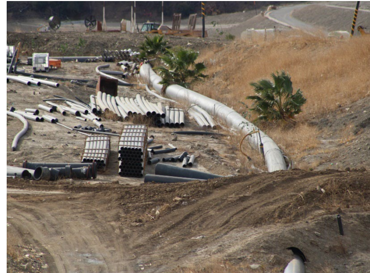
Photo 94: Working Area, CC4 Part 1/2: December 11, 2024
