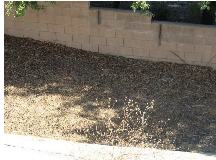
Photo 328: Terminal Basin: November 20, 2024
