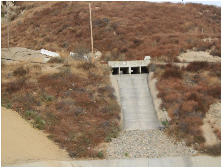
Photo 343: Terminal Basin: December 11, 2024
