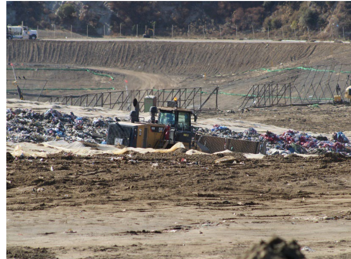
Photo 10: Working Area, CC4 Part 1/2: October 31, 2024
