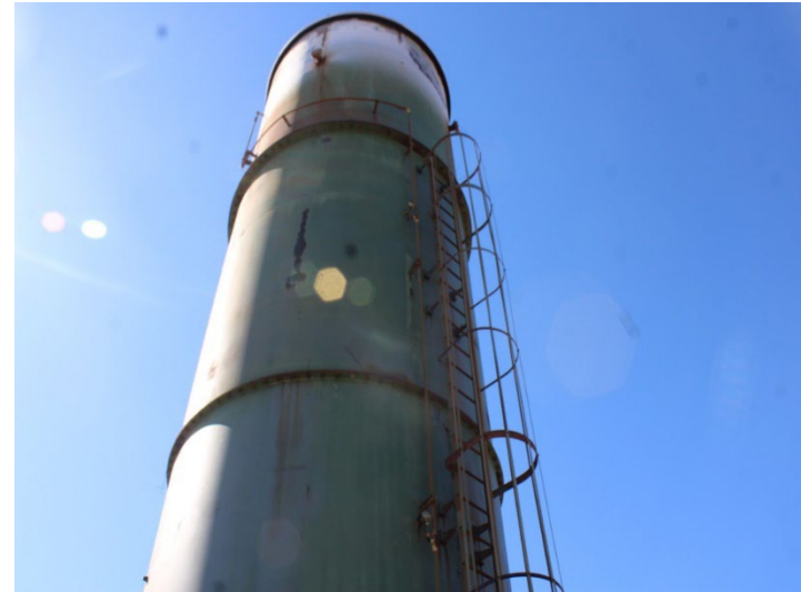
Photo 414: General Site: October 31, 2024
