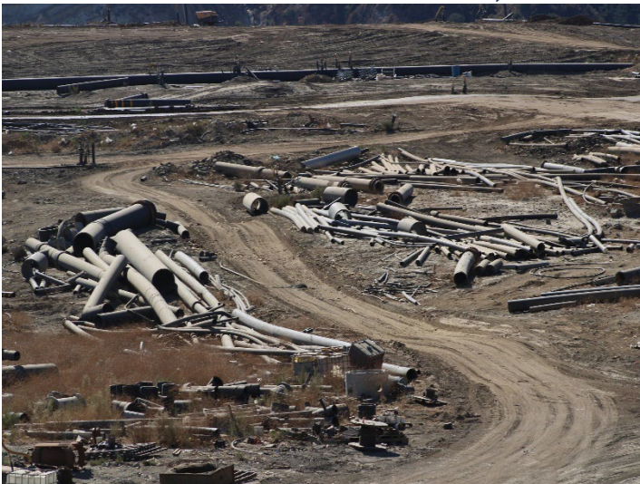
Photo 411: General Site: October 31, 2024
