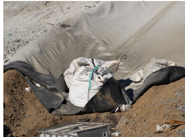
Photo 396: General Site: October 31, 2024
