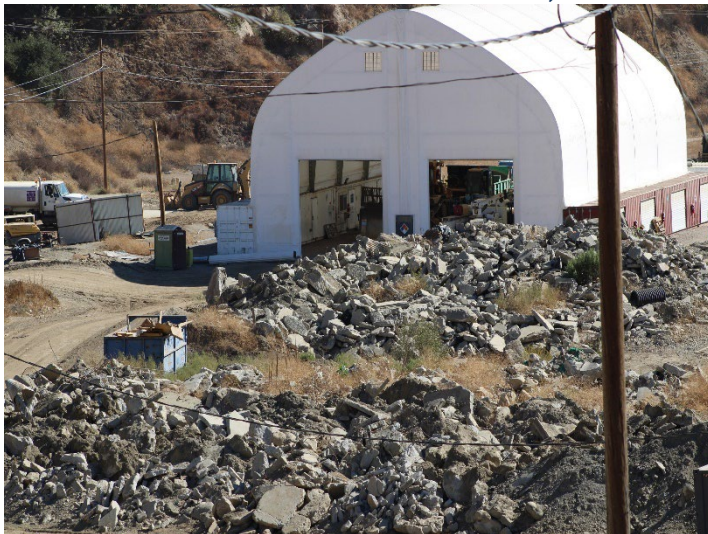
Photo 407: General Site: October 31, 2024
