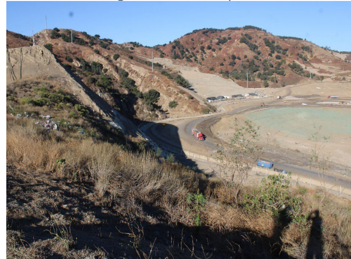
Photo 160: Working Area, CC4 Part 4/5: November 20, 2024
