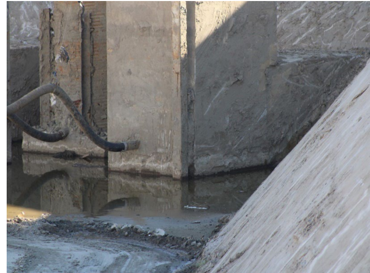
Photo 298: Terminal Basin: October 31, 2024
