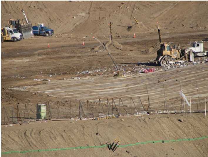
Photo 121: Working Area, CC4 Part 3: October 31, 2024
