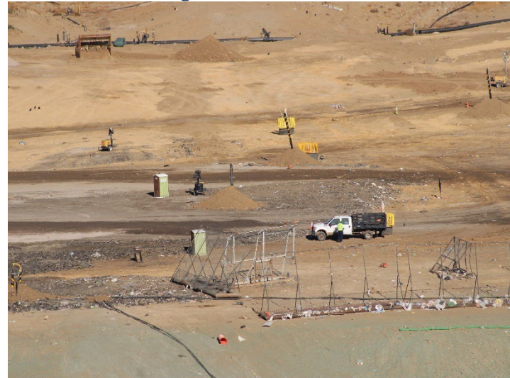
Photo 128: Working Area, CC4 Part 3: November 20, 2024
