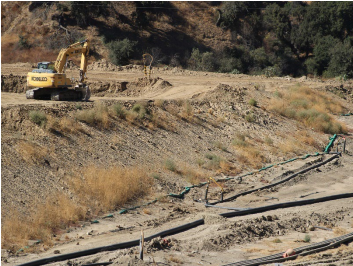
Photo 265: County Top Deck: October 31, 2024
