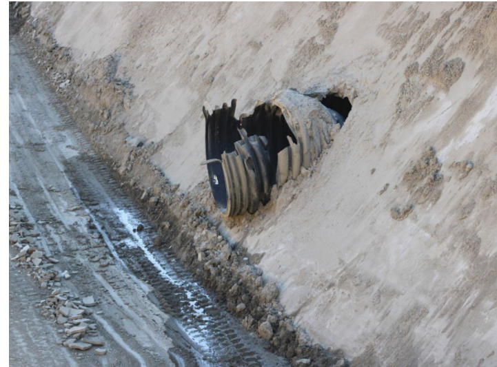
Photo 294: Terminal Basin: October 31, 2024
