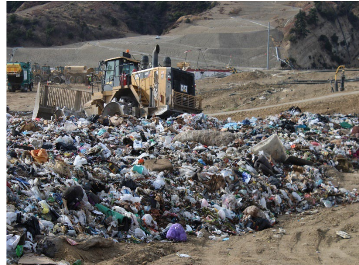
Photo 102: Working Area, CC4 Part 1/2: December 11, 2024
