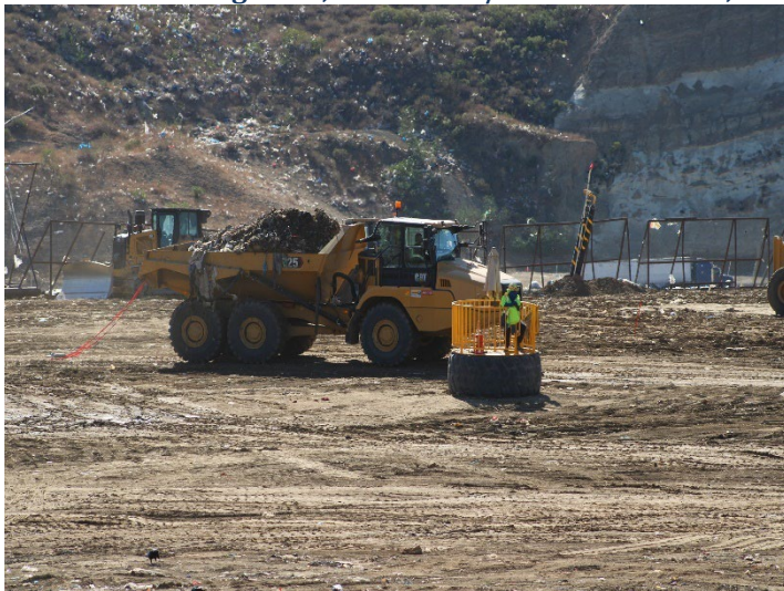
Photo 39: Working Area, CC4 Part 1/2: November 20, 2024
