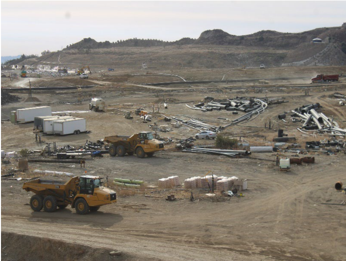
Photo 513: General Site: December 11, 2024
