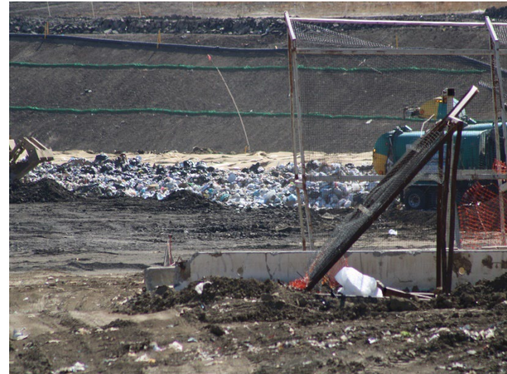
Photo 22: Working Area, CC4 Part 1/2: October 31, 2024
