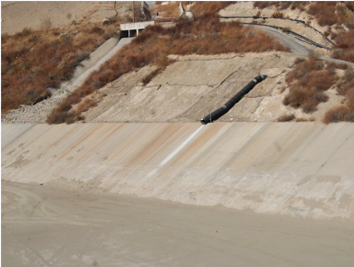
Photo 325: Terminal Basin: November 20, 2024
