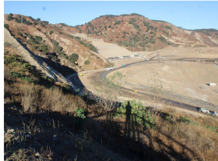
Photo 142: Working Area, CC4 Part 4/5: October 31, 2024
