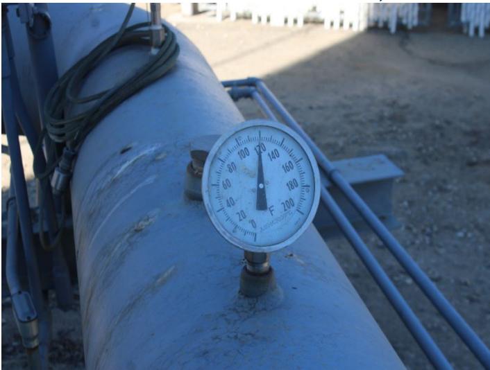
Photo 419: General Site: October 31, 2024
