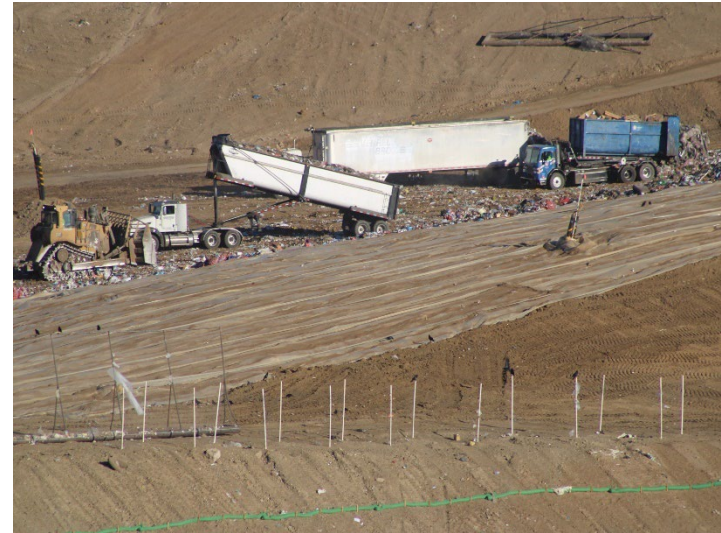
Photo 122: Working Area, CC4 Part 3: October 31, 2024
