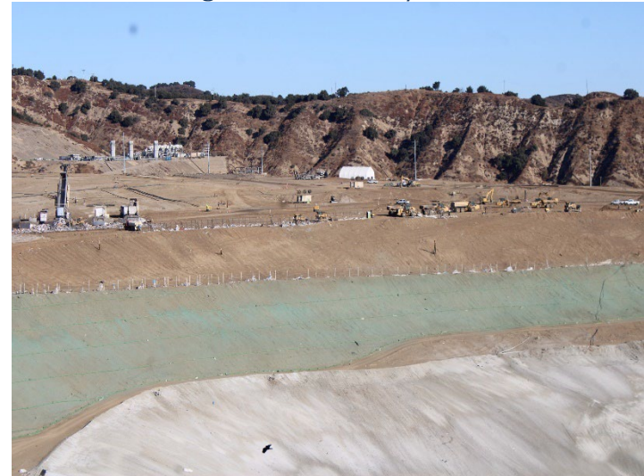
Photo 168: Working Area, CC4 Part 4/5: November 20, 2024
