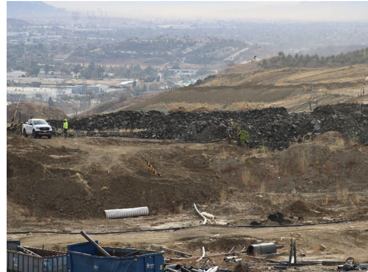
Photo 82: Working Area, CC4 Part 1/2: December 11, 2024
