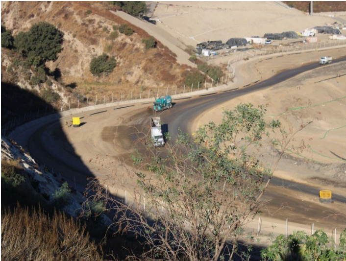
Photo 145: Working Area, CC4 Part 4/5: October 31, 2024
