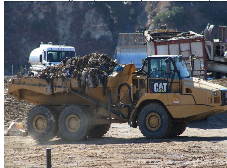
Photo 44: Working Area, CC4 Part 1/2: November 20, 2024
