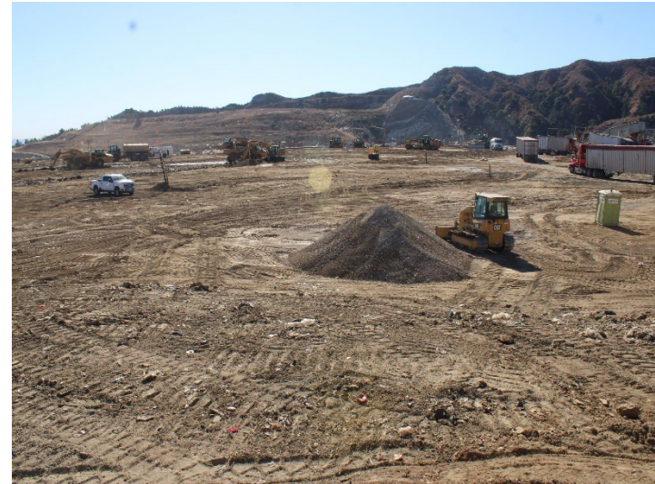
Photo 30: Working Area, CC4 Part 1/2: November 20, 2024
