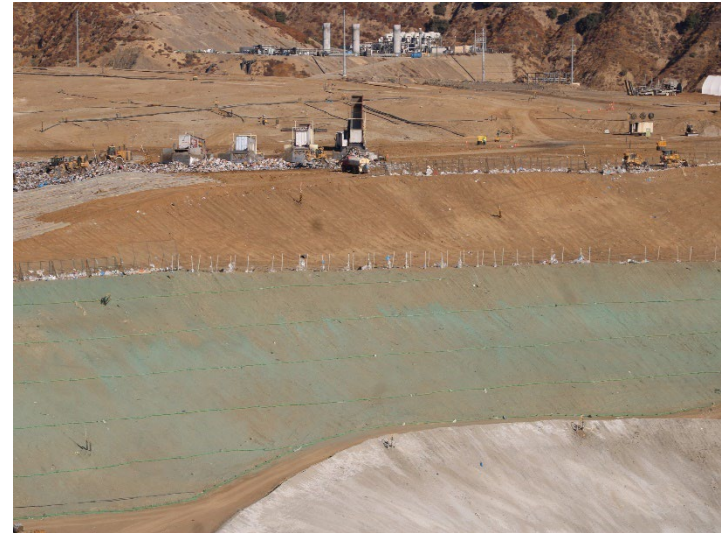
Photo 178: Working Area, CC4 Part 4/5: November 20, 2024
