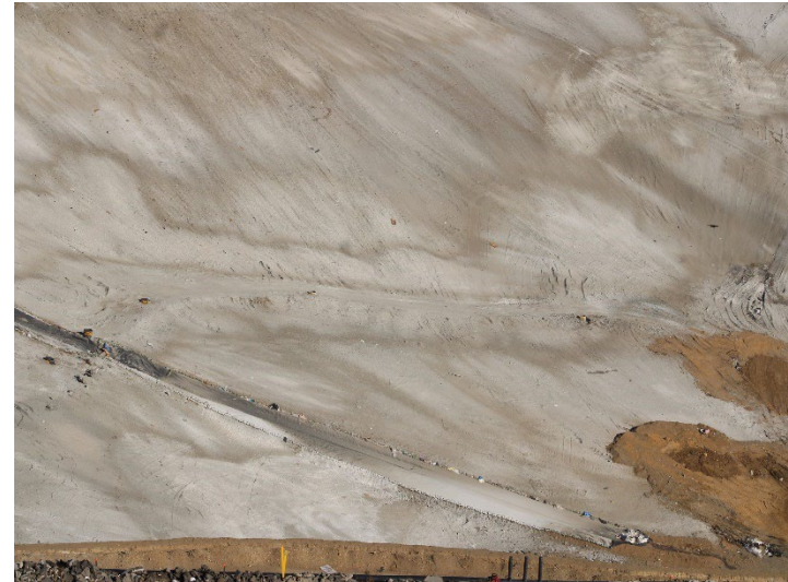
Photo 174: Working Area, CC4 Part 4/5: November 20, 2024
