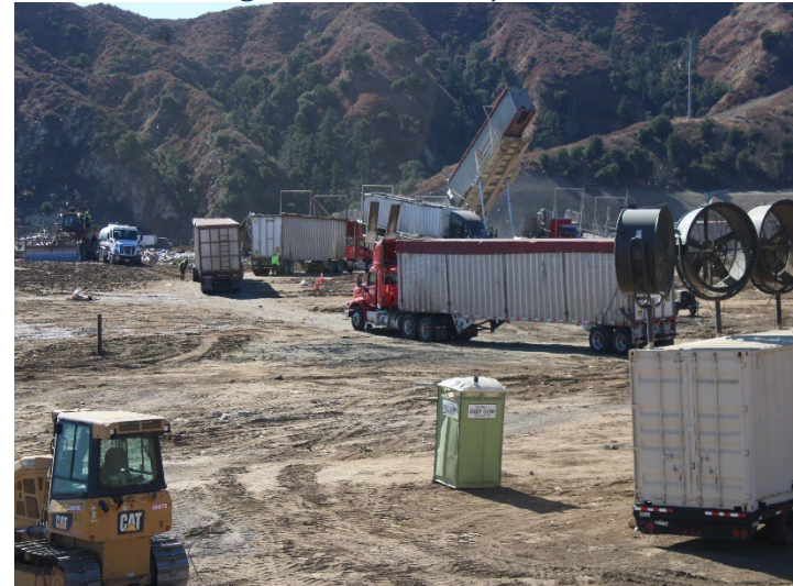
Photo 36: Working Area, CC4 Part 1/2: November 20, 2024
