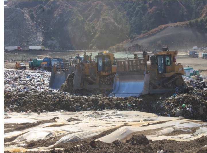
Photo 64: Working Area, CC4 Part 1/2: November 20, 2024
