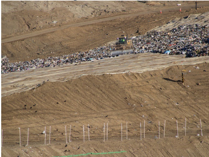
Photo 123: Working Area, CC4 Part 3: October 31, 2024
