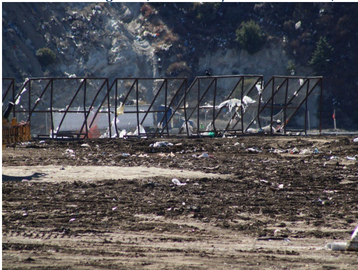
Photo 43: Working Area, CC4 Part 1/2: November 20, 2024
