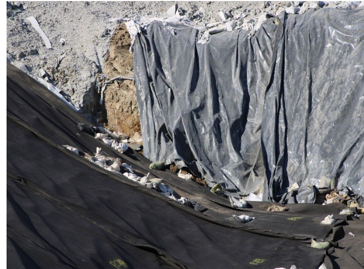
Photo 394: General Site: October 31, 2024
