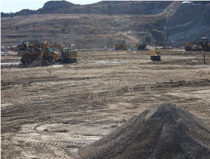
Photo 35: Working Area, CC4 Part 1/2: November 20, 2024
