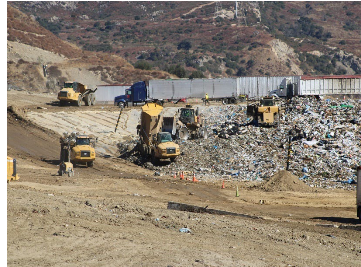
Photo 70: Working Area, CC4 Part 1/2: November 20, 2024
