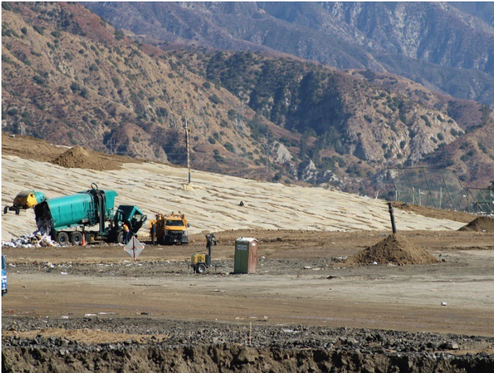
Photo 73: Working Area, CC4 Part 1/2: November 20, 2024
