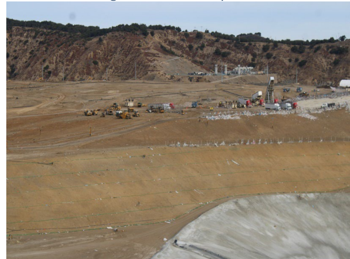
Photo 192: Working Area, CC4 Part 4/5: December 11, 2024
