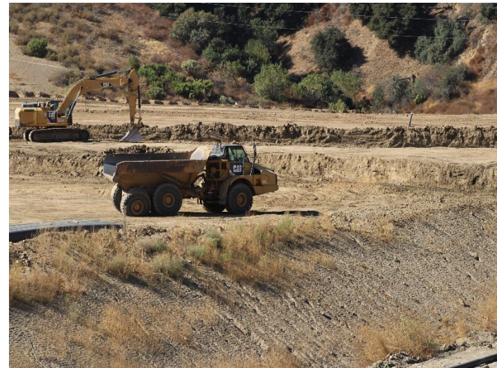
Photo 264: County Top Deck: October 31, 2024
