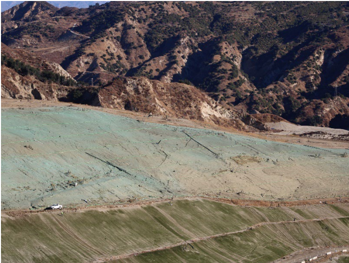
Photo 181: Working Area, CC4 Part 4/5: November 20, 2024
