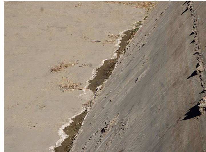
Photo 332: Terminal Basin: November 20, 2024
