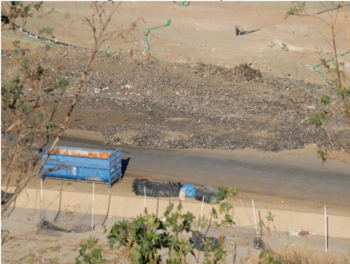
Photo 171: Working Area, CC4 Part 4/5: November 20, 2024
