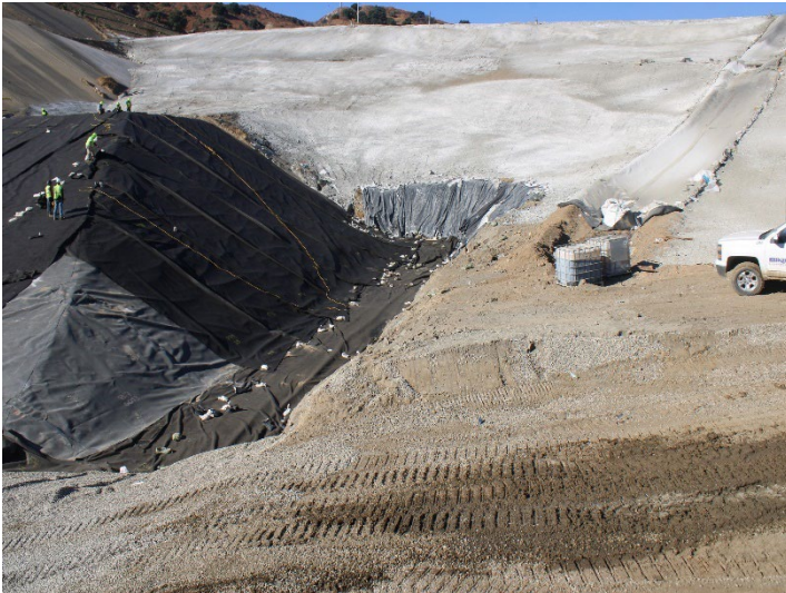
Photo 387: General Site: October 31, 2024
