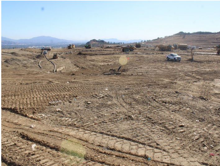
Photo 29: Working Area, CC4 Part 1/2: November 20, 2024
