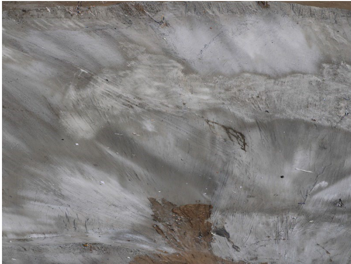
Photo 197: Working Area, CC4 Part 4/5: December 11, 2024
