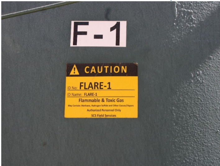
Photo 423: General Site: October 31, 2024
