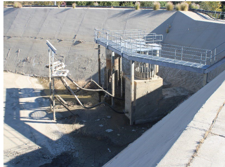
Photo 320: Terminal Basin: November 20, 2024
