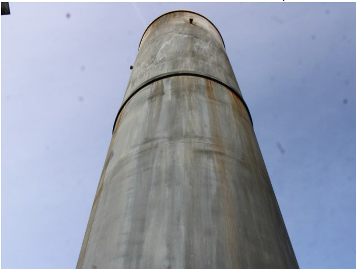
Photo 543: General Site: December 11, 2024
