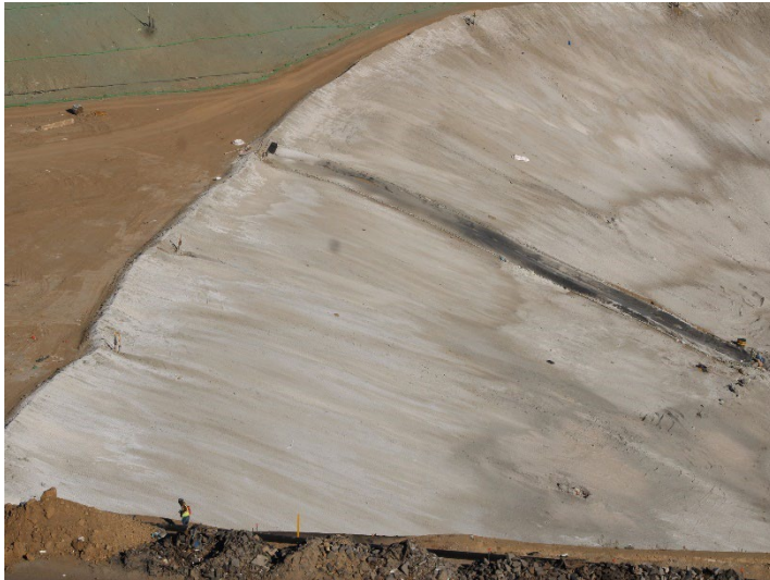
Photo 173: Working Area, CC4 Part 4/5: November 20, 2024
