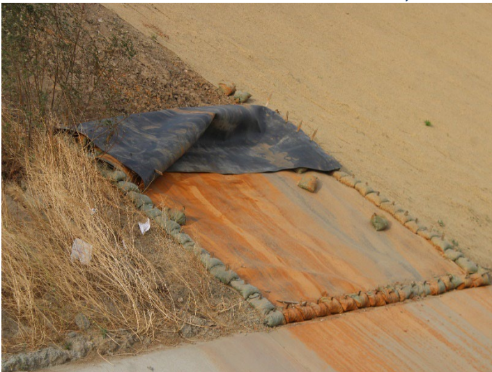
Photo 339: Terminal Basin: December 11, 2024
