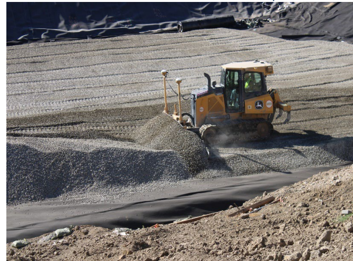
Photo 400: General Site: October 31, 2024
