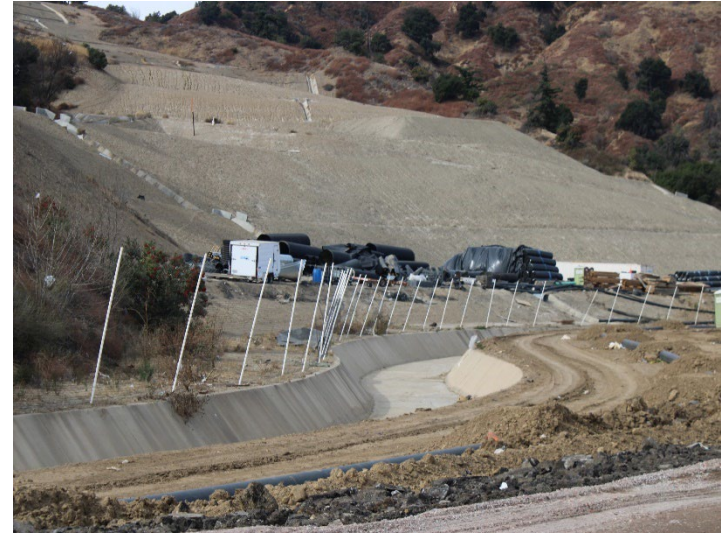
Photo 550: General Site: December 11, 2024
