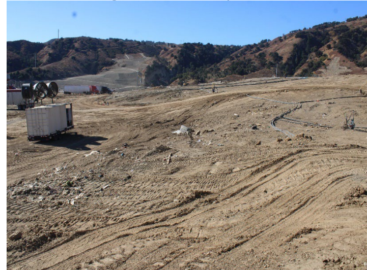
Photo 32: Working Area, CC4 Part 1/2: November 20, 2024
