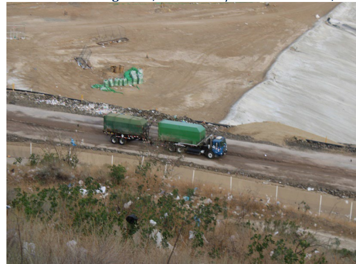
Photo 188: Working Area, CC4 Part 4/5: December 11, 2024
