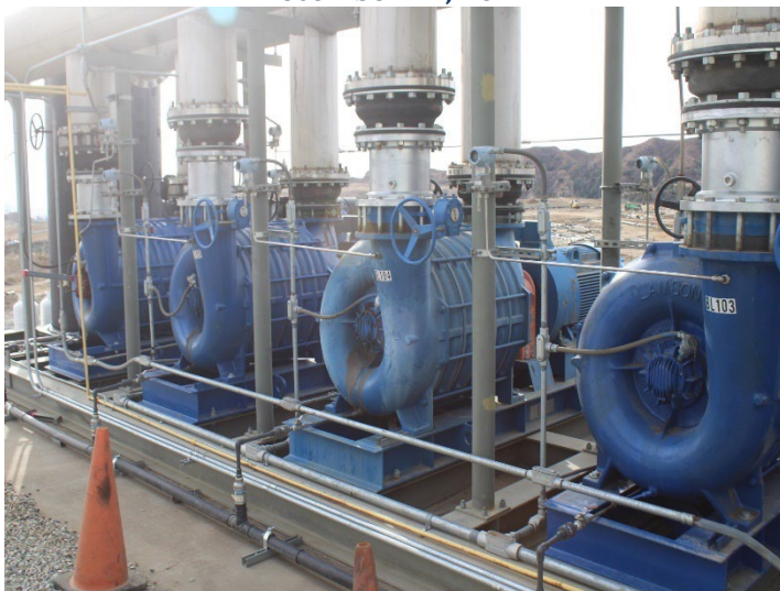
Photo 255: Flares 9, 10, 11 and Gas-to-Energy Facility: December 11, 2024
