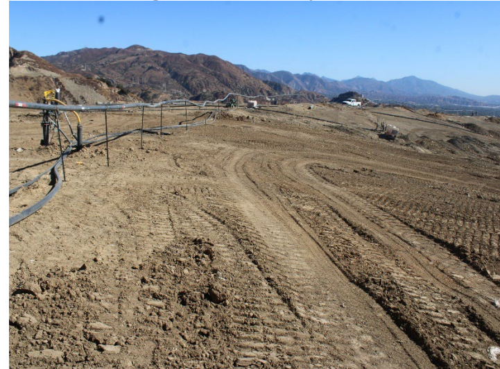
Photo 28: Working Area, CC4 Part 1/2: November 20, 2024
