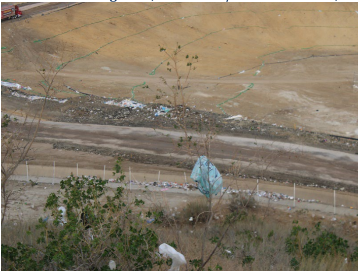
Photo 187: Working Area, CC4 Part 4/5: December 11, 2024
