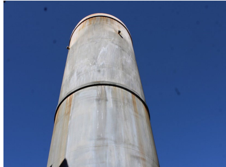
Photo 422: General Site: October 31, 2024
