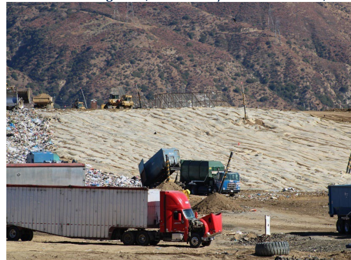
Photo 72: Working Area, CC4 Part 1/2: November 20, 2024
