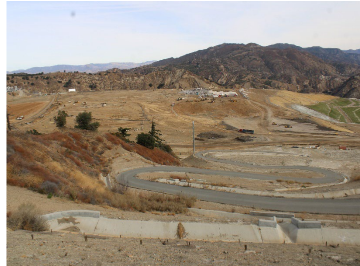
Photo 554: General Site: December 11, 2024
