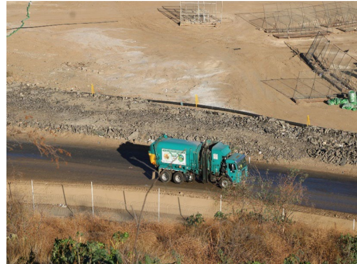
Photo 150: Working Area, CC4 Part 4/5: October 31, 2024
