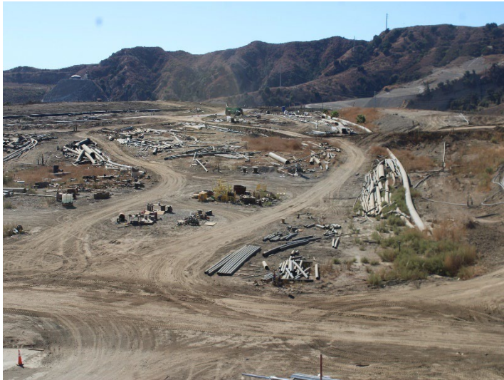
Photo 405: General Site: October 31, 2024
