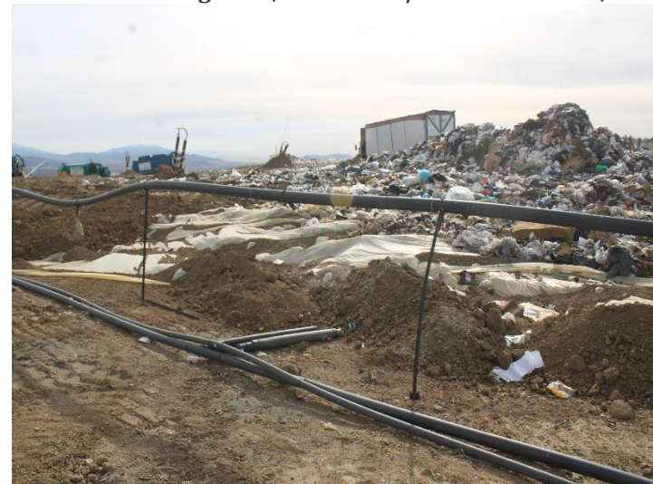
Photo 96: Working Area, CC4 Part 1/2: December 11, 2024
