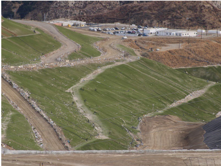
Photo 561: General Site: December 11, 2024
