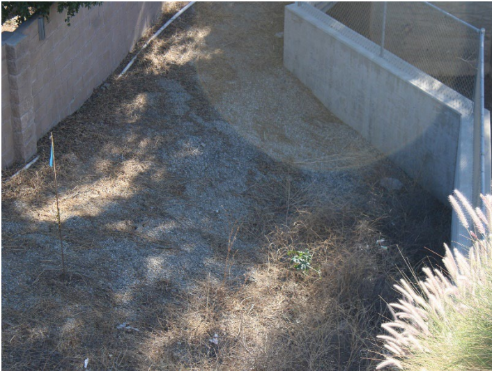
Photo 329: Terminal Basin: November 20, 2024
