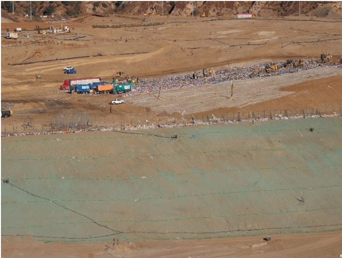
Photo 177: Working Area, CC4 Part 4/5: November 20, 2024
