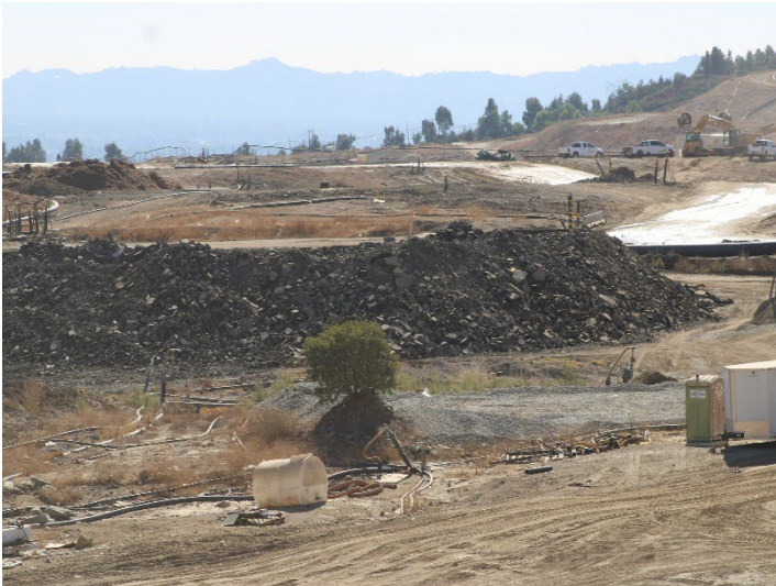
Photo 409: General Site: October 31, 2024
