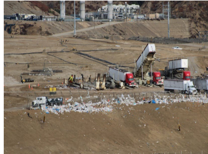
Photo 78: Working Area, CC4 Part 1/2: December 11, 2024
