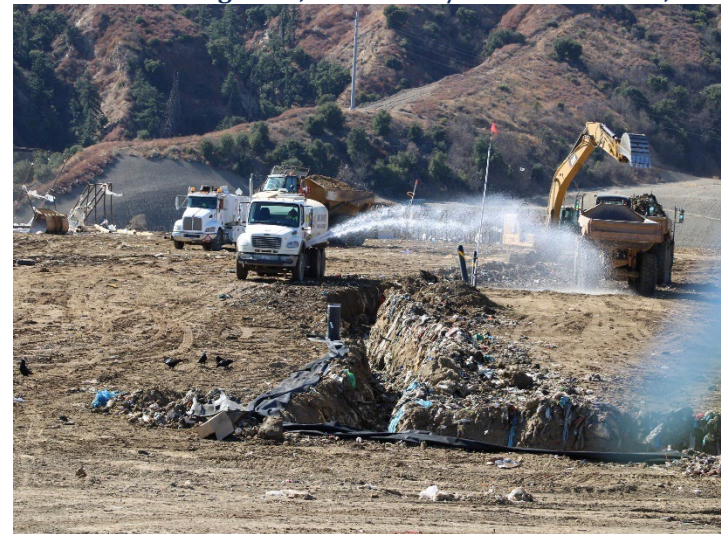
Photo 52: Working Area, CC4 Part 1/2: November 20, 2024
