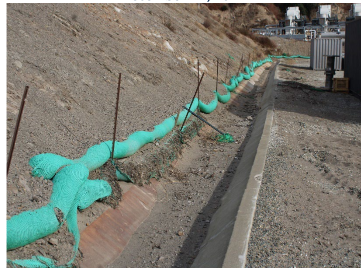
Photo 260: Flares 9, 10, 11 and Gas-to-Energy Facility: December 11, 2024
