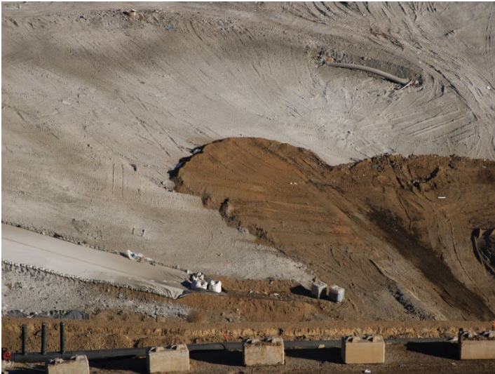
Photo 157: Working Area, CC4 Part 4/5: October 31, 2024
