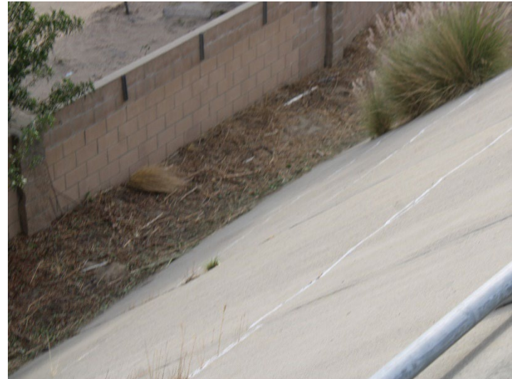
Photo 350: Terminal Basin: December 11, 2024
