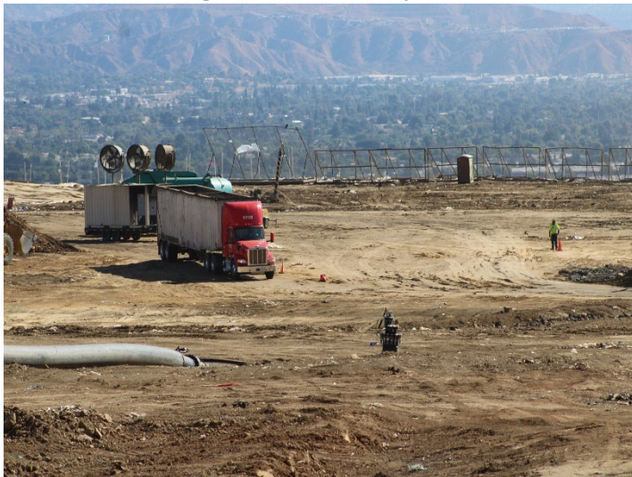
Photo 19: Working Area, CC4 Part 1/2: October 31, 2024
