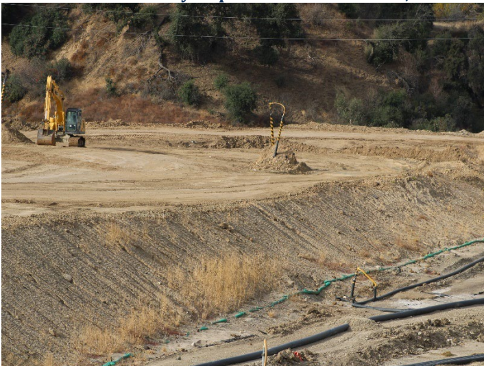
Photo 275: County Top Deck: December 11, 2024
