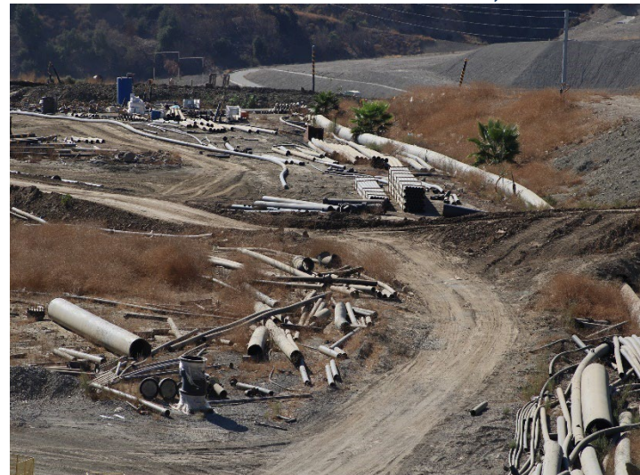
Photo 412: General Site: October 31, 2024
