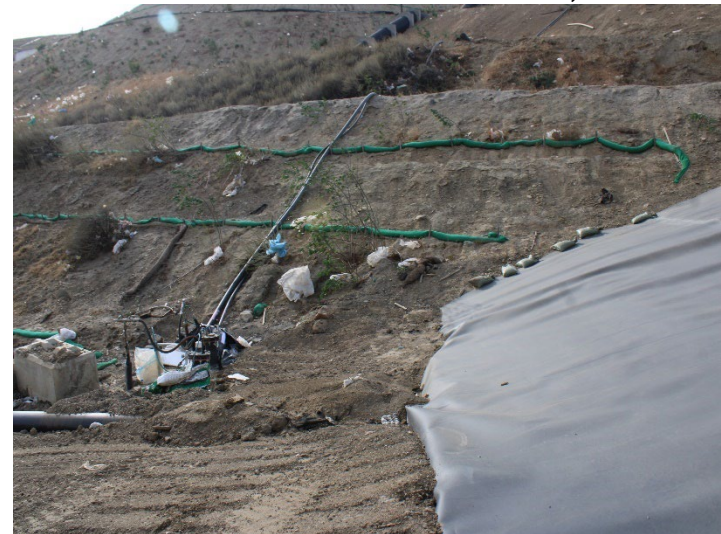
Photo 516: General Site: December 11, 2024
