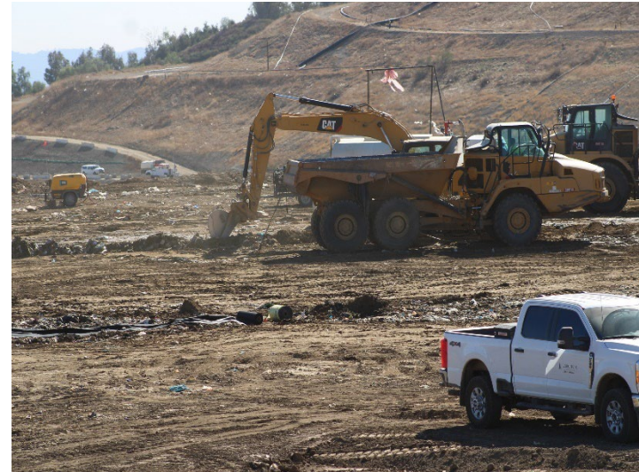
Photo 38: Working Area, CC4 Part 1/2: November 20, 2024
