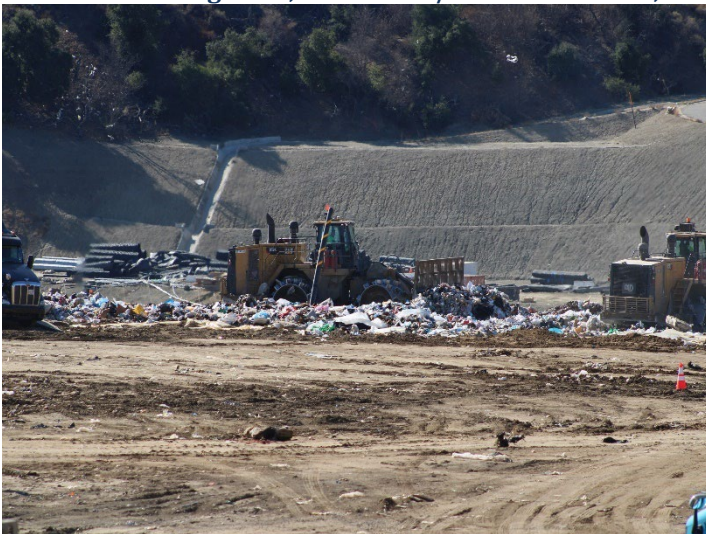
Photo 47: Working Area, CC4 Part 1/2: November 20, 2024
