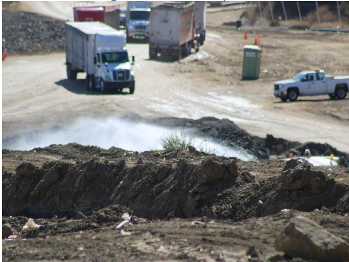
Photo 23: Working Area, CC4 Part 1/2: October 31, 2024
