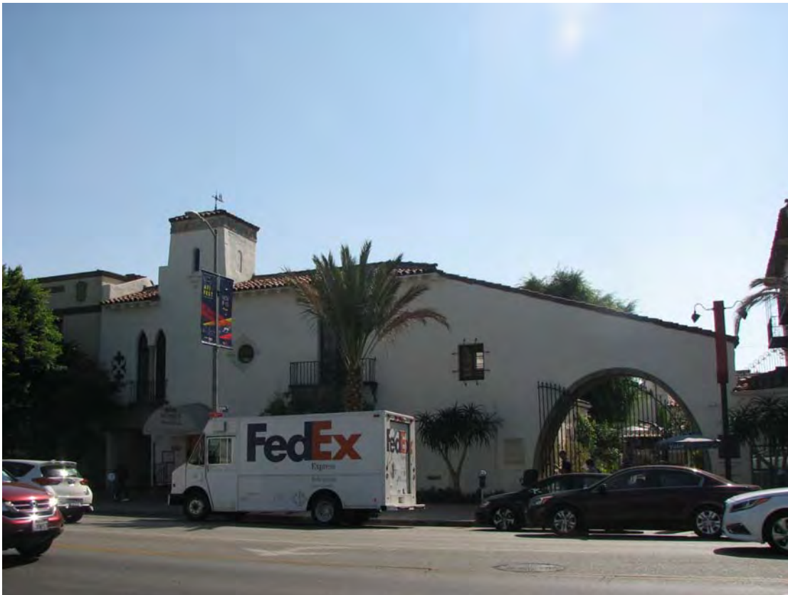
Fred C. Thomson Building, front facade, 6526-40 Sunset Boulevard, October 24, 2018, (Charles J. Fisher photo)
