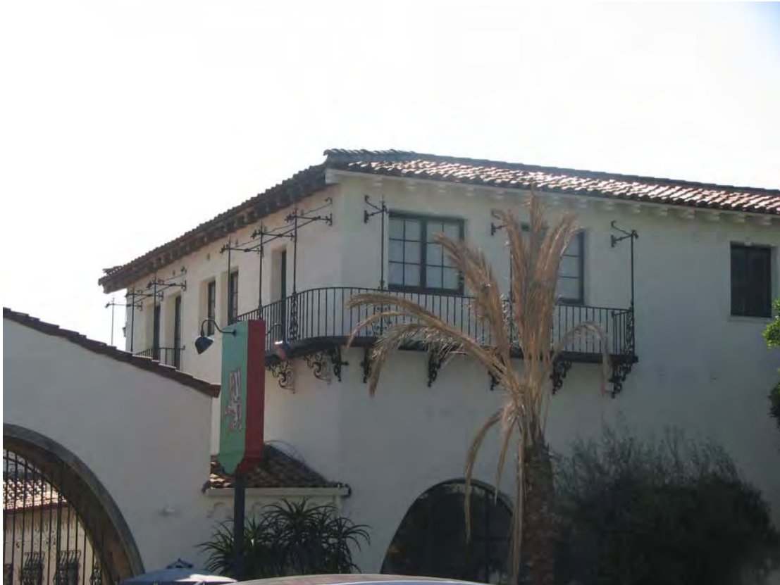
Fred C. Thomson Building, front facade, 6526-40 Sunset Boulevard, October 24, 2018, (Charles J. Fisher photo)
