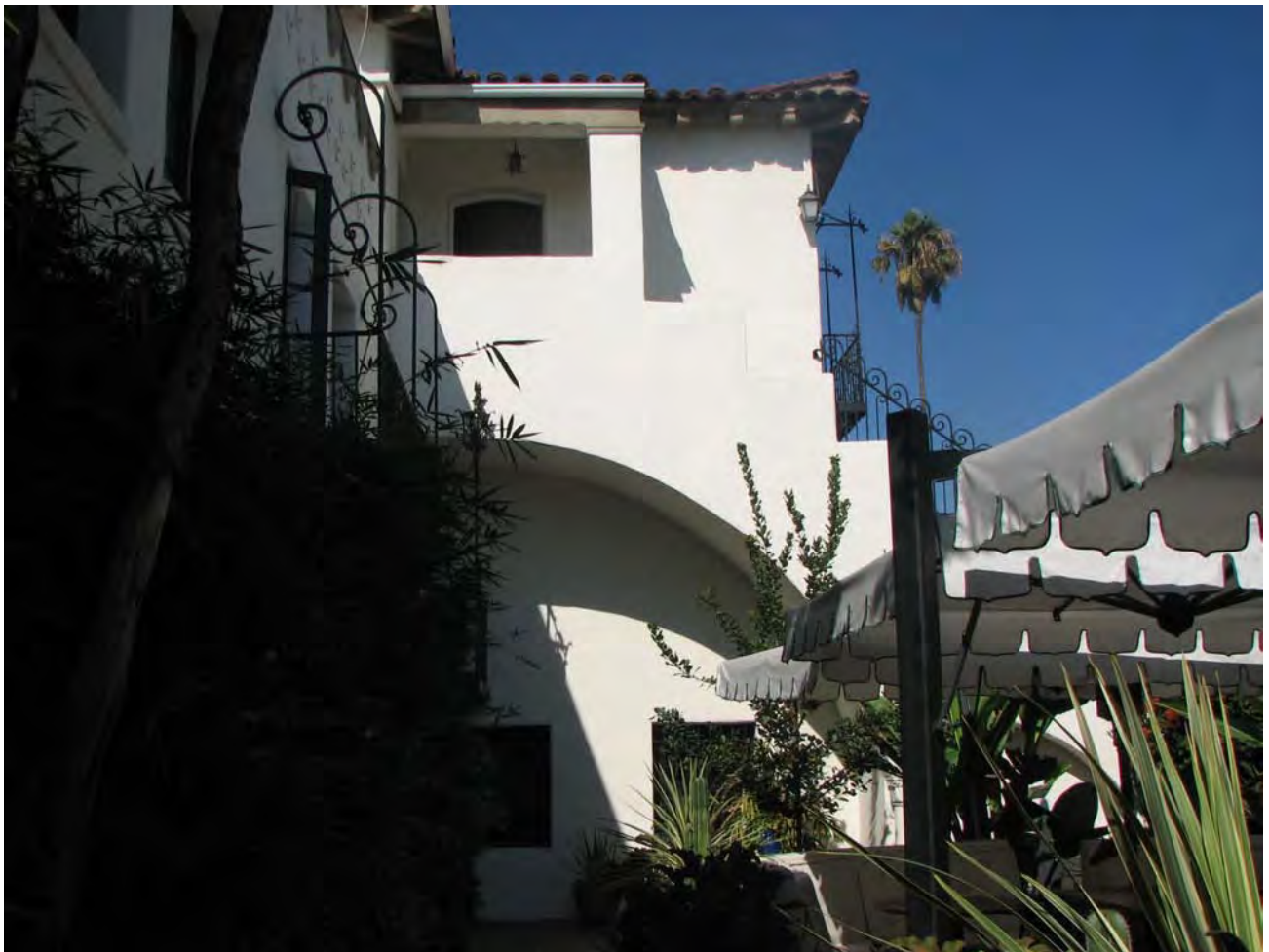
Fred C. Thomson Building, view from courtyard, 6526-40 Sunset Boulevard, October 24, 2018, (Charles J. Fisher photo)
